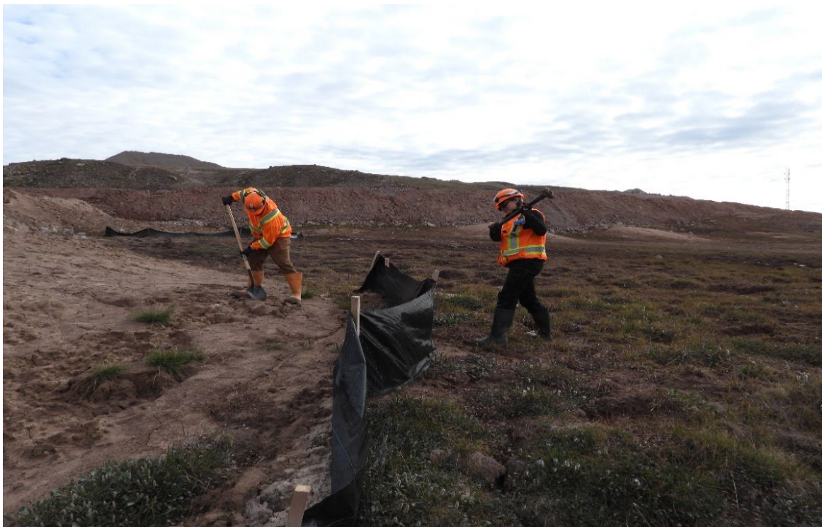
Photo 77. Silt Fence Installation along the Tote Road - August
