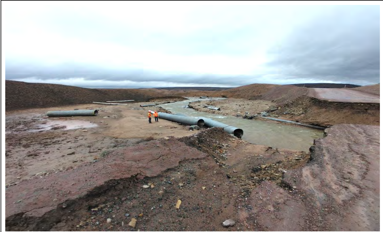
Photo 1. KM 63.5 Culverts deposited downstream from Tote Road crossing during September rain event, 2024-09-22
