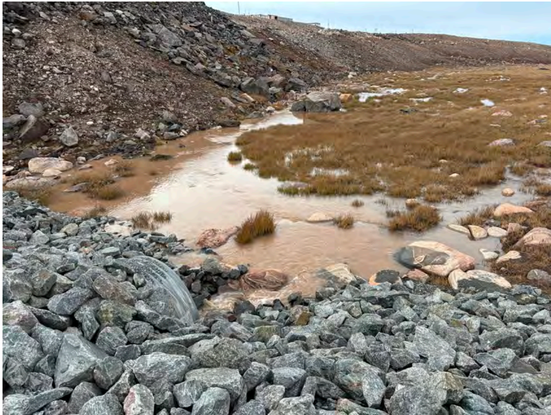
Photo 9 – Downstream of KM105 Dam looking at sediment laden runoff on the tundra (Sep 2024).
