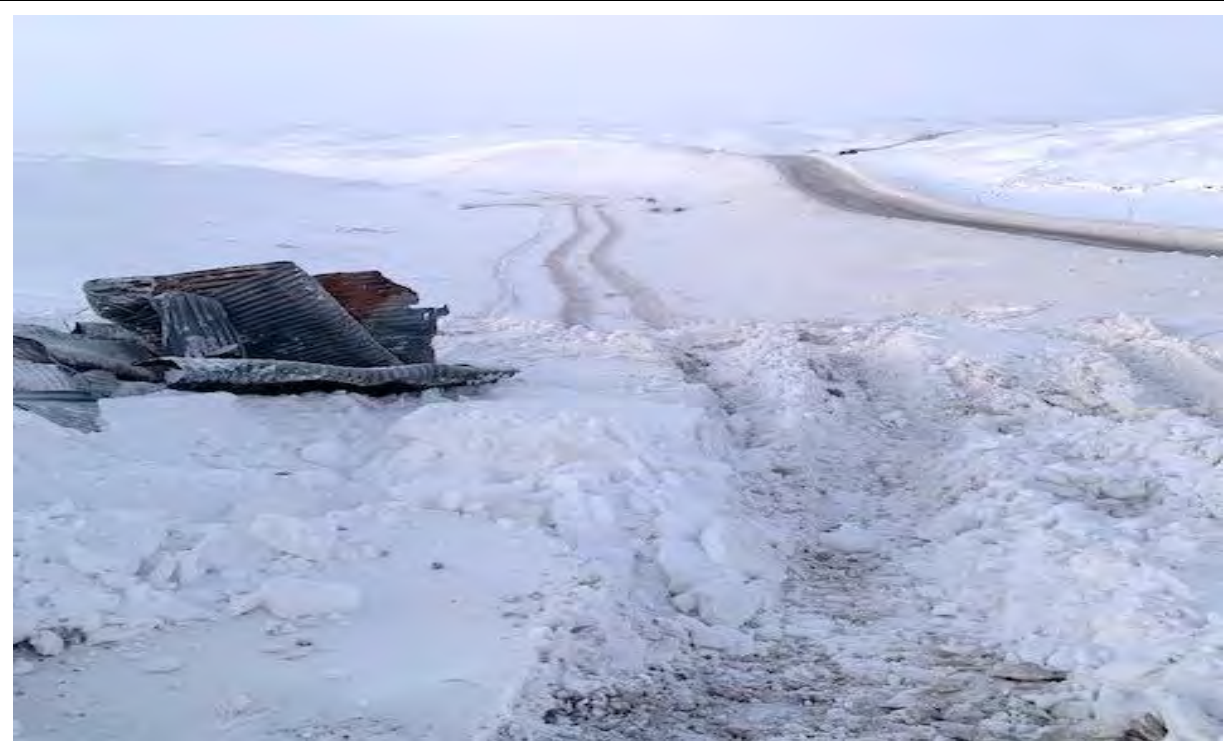
Photo 4. KM 63.5, Culverts retrieved from watercourse, staged next to Tote Road for pick-up and final disposal, 2024-11-28
