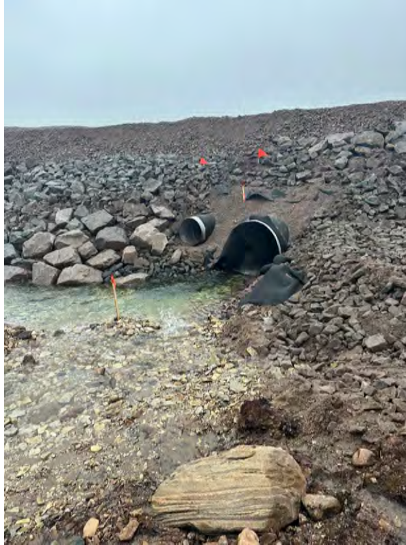
Photo 17 – Culvert replacement at ~KM63.5 (Oct 2 nd , 2024).
