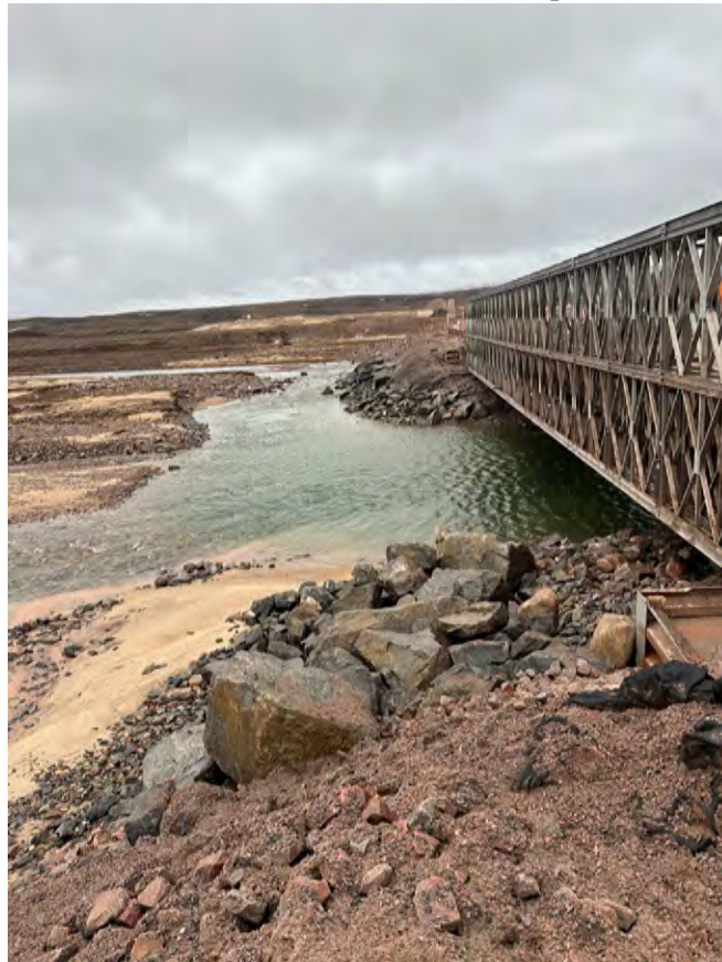
Photo 26 – Bridge close to Sailiivik Camp and sediment deposited due to erosion (Oct 2 nd , 2024)
