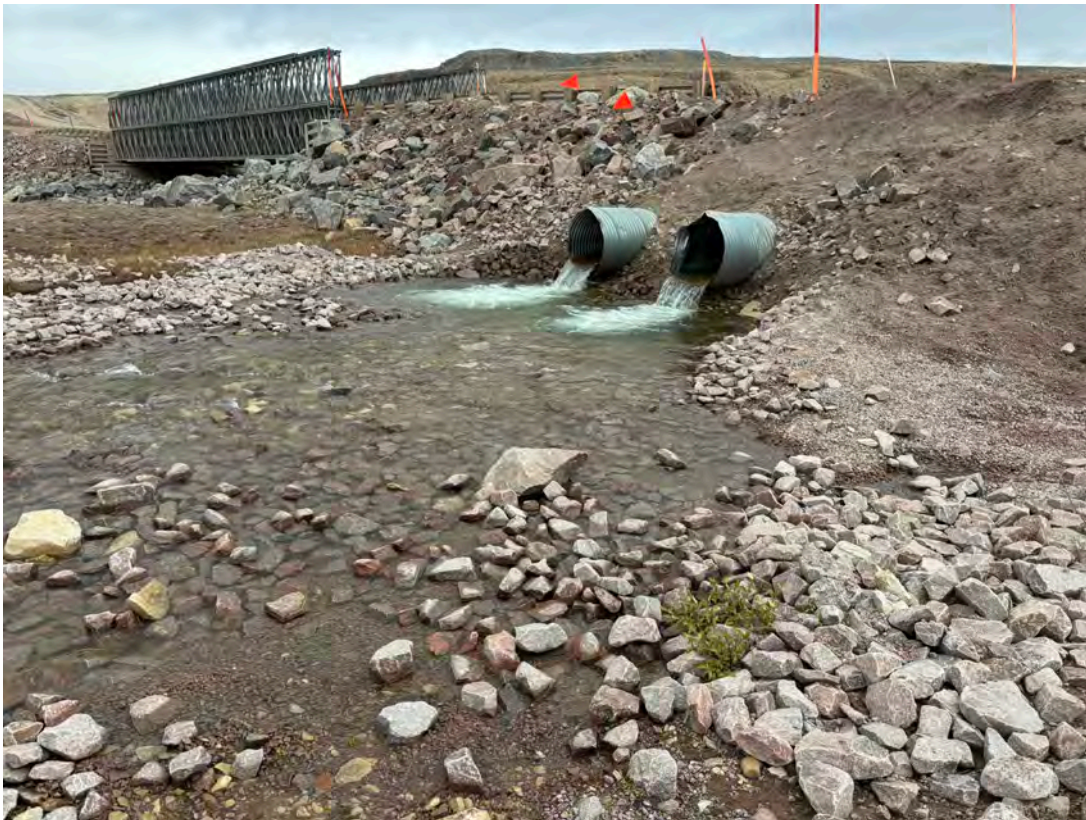
Photo 16 – KM63 watercourse crossing – perched CSP culverts (Sep 2024).
