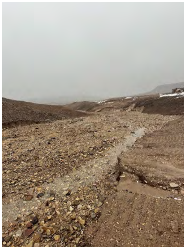
Photo 21 – Example of sediment erosion adjacent to the Tote Road (Oct 2 nd , 2024).
