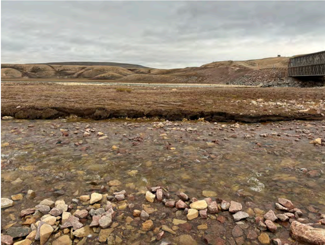
Photo 17 – KM63 watercourse crossing – streambank erosion downstream of perched CSP culverts (Sep 2024).
