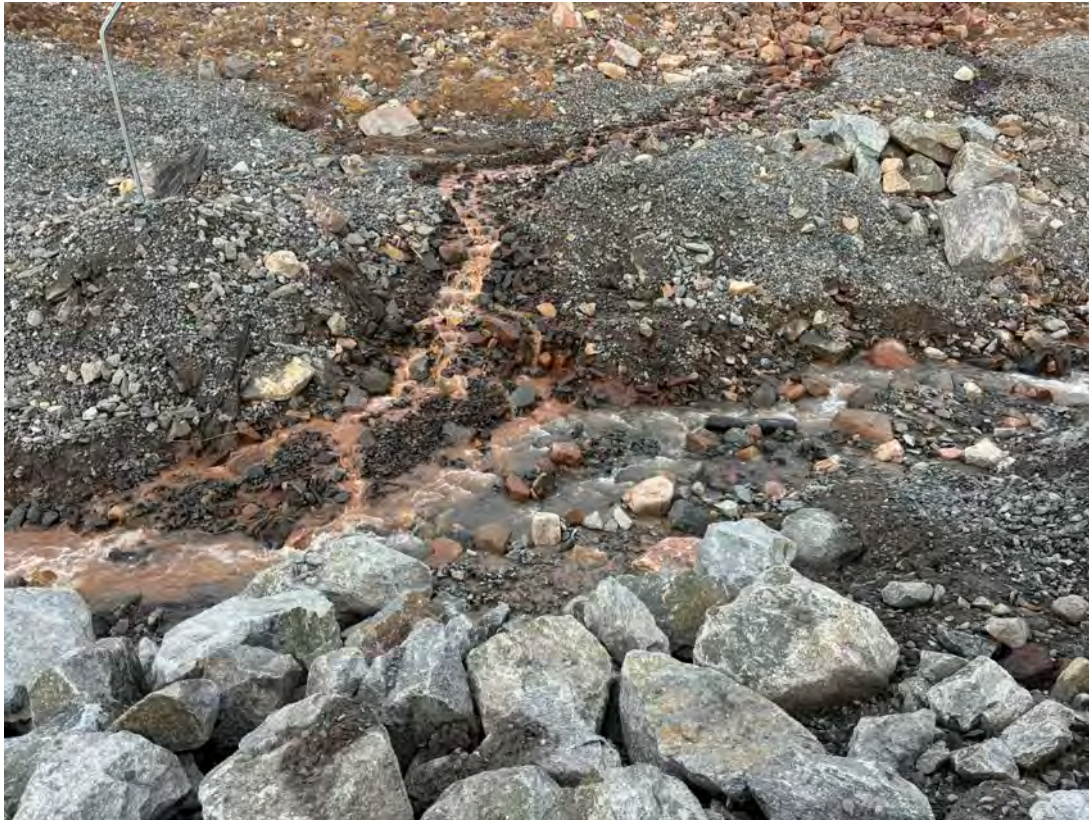
Photo 3 – Sediment laden runoff from upslope at KM106.5 (Sep 2024).
