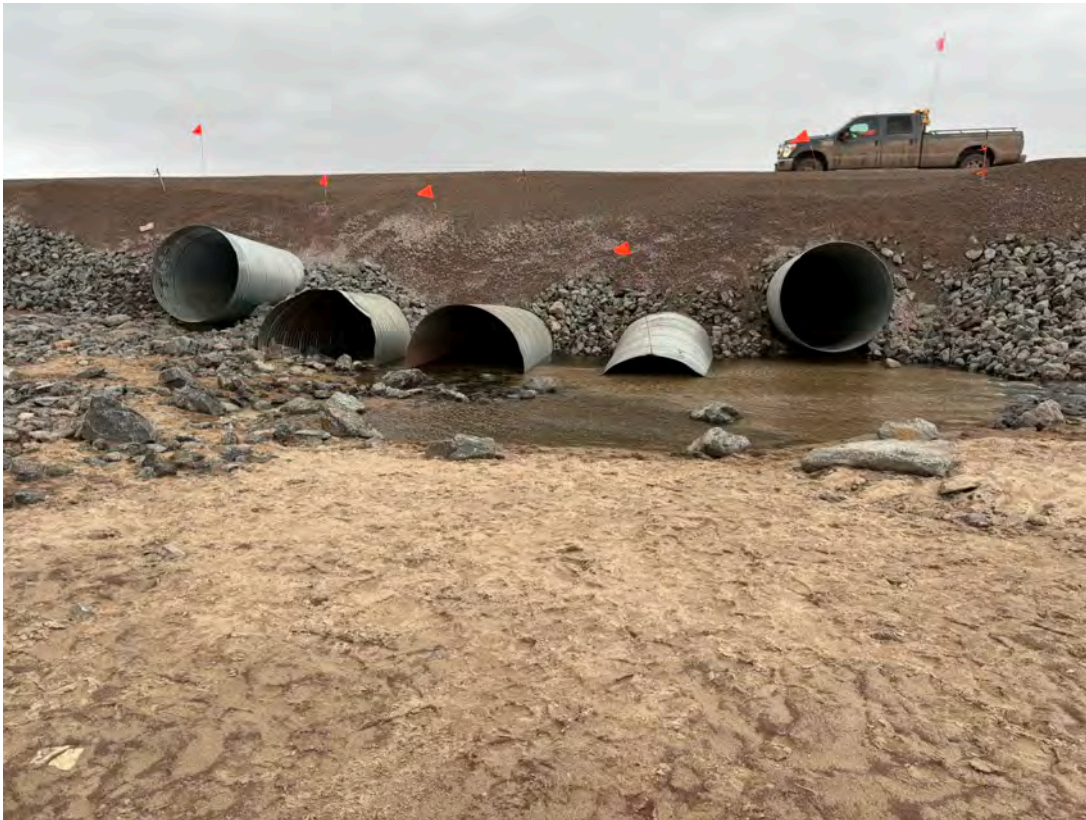
Photo 13 – KM81 watercourse crossing where road has washed out – downstream side (Sep 2024).
