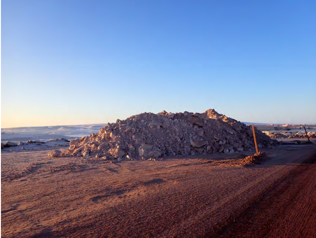
Photo 1 – Temporary snow stockpile immediately south of the mine road to be removed in order to ensure no sediment be deposited into Sheardown Lake Tributary - February 9, 2025
