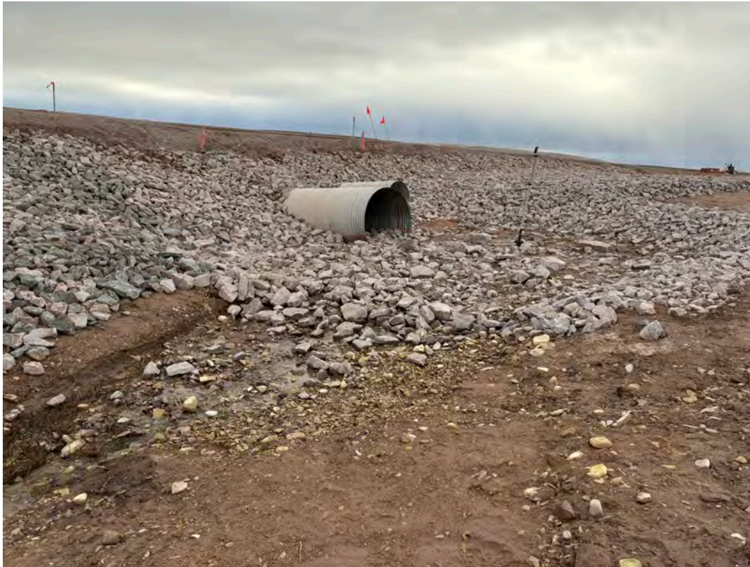
Photo 19 – KM33 watercourse crossing – flow emerging from under recently placed rocks visible (Sep 2024).
