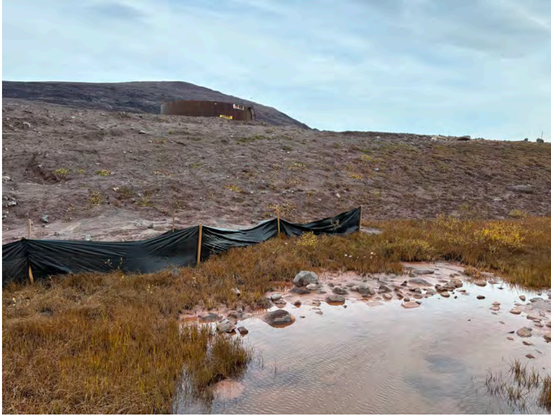
Photo 11 – Fine sediment accumulation on rocks – Sheardown Tributary east of Sailiivik Camp. Example of location where use of coir logs could be implemented (Sep 2024).
