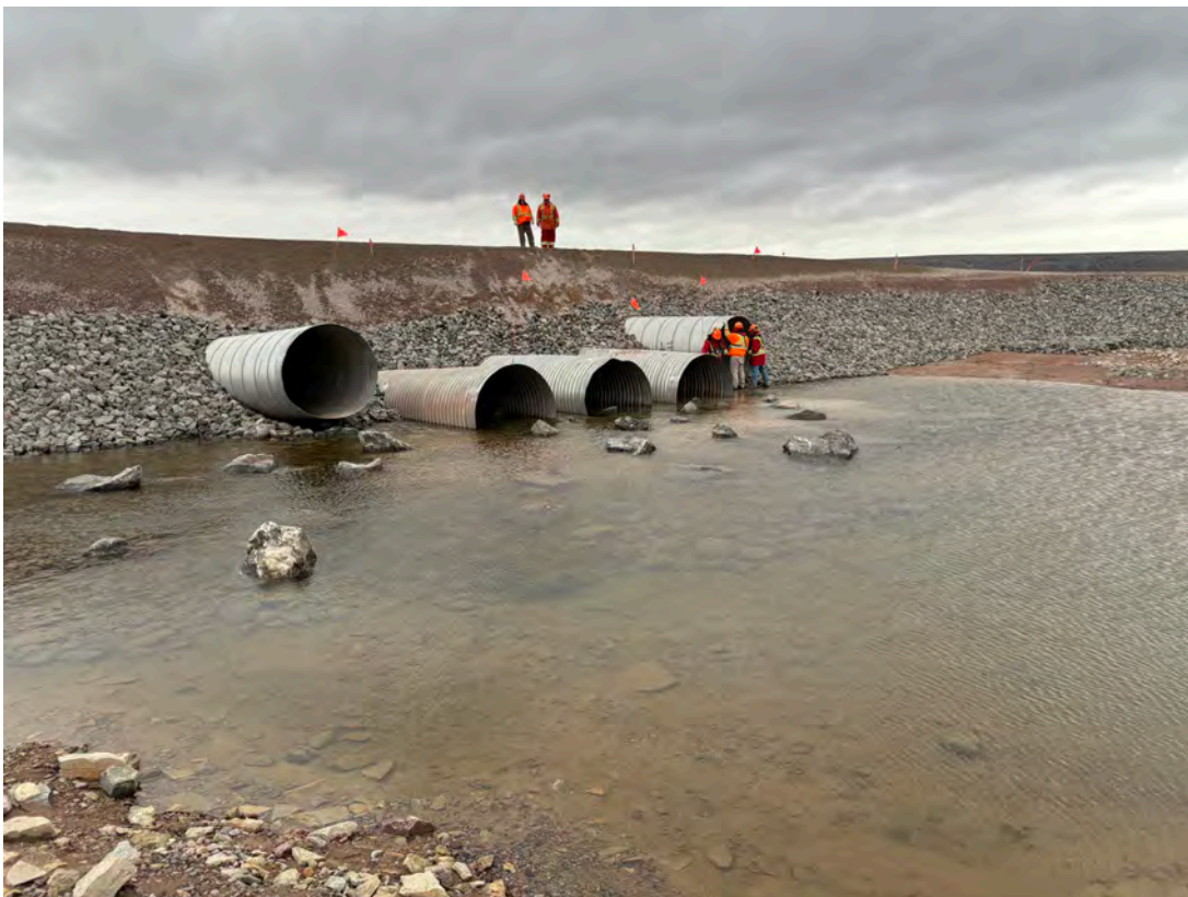
Photo 14 – KM81 watercourse crossing where road has washed out – upstream side (Sep 2024).
