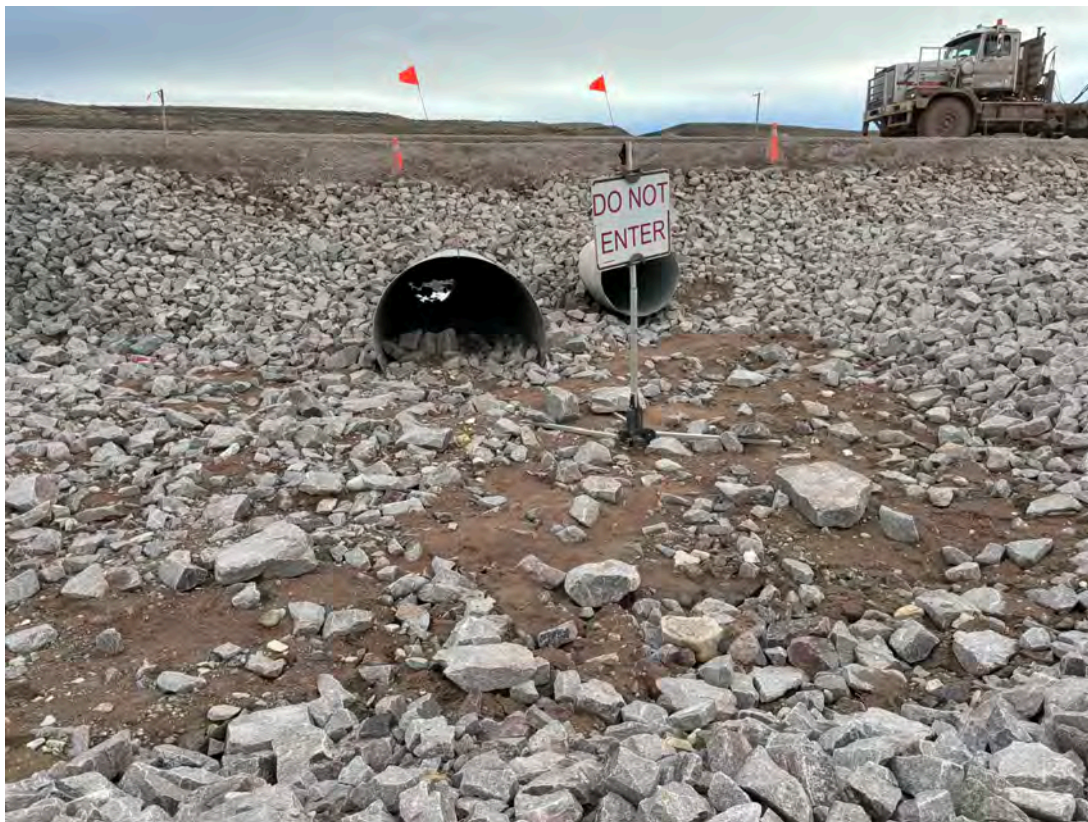
Photo 18 – KM33 watercourse crossing – flow under recently placed rocks (Sep 2024).
