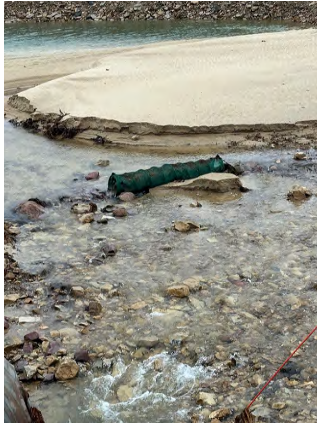
Photo 25 – Extent of erosion and increased channel size compared to erosion trap (Oct 2 nd , 2024).
