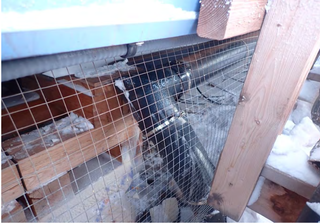
Photo 3. Influent Line (After Repair) – February 29, 2024
