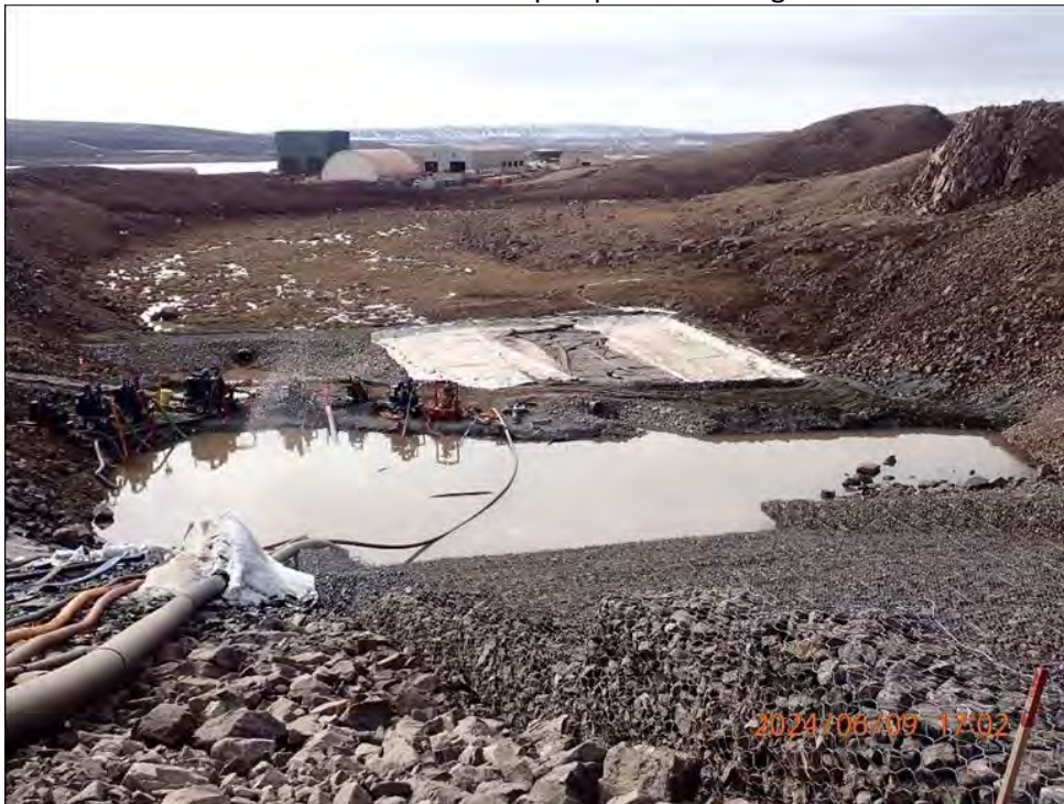
Photo 12: Reinforced earthen berm and pumps transferring water back into treatment pond, June 2024
