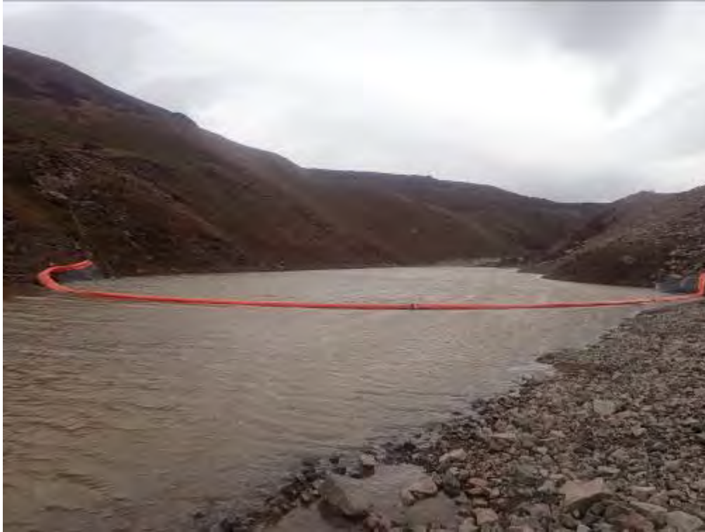
Photo 1: Installation of two (2) silt curtains upstream of the intake pumps 2022
