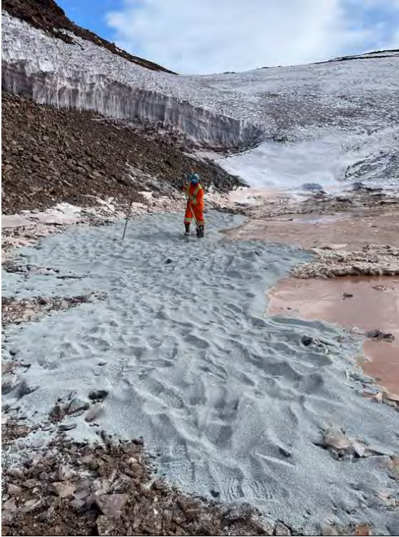
Photo 3: Attempt at sealing new seepage location utilizing bentonite plugs, 2023
