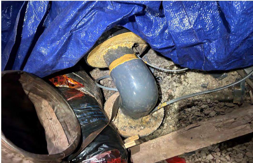
Photo 3. Influent Line (After Repair) – February 4, 2024
