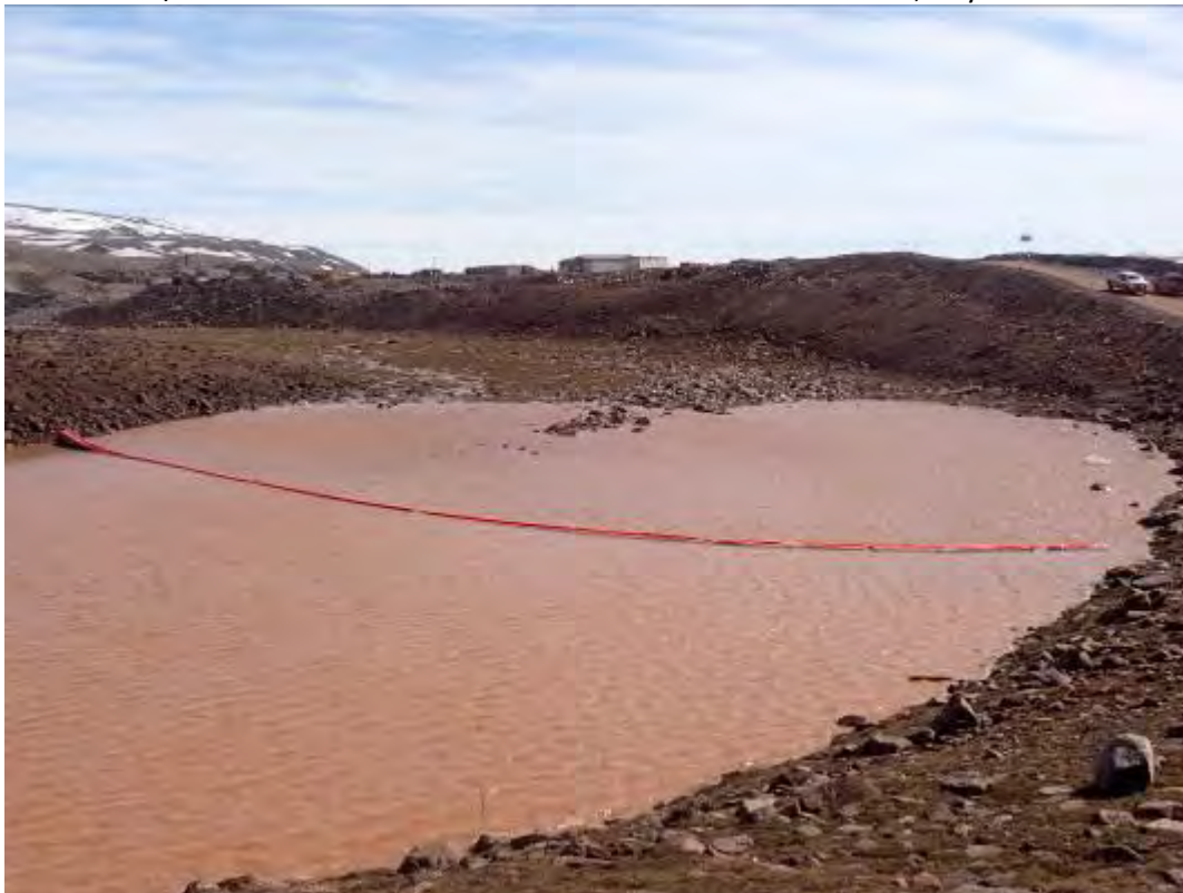
Photo 6: Silt/ Sedimentation Curtain downstream of the KM105 dam, July 2023
