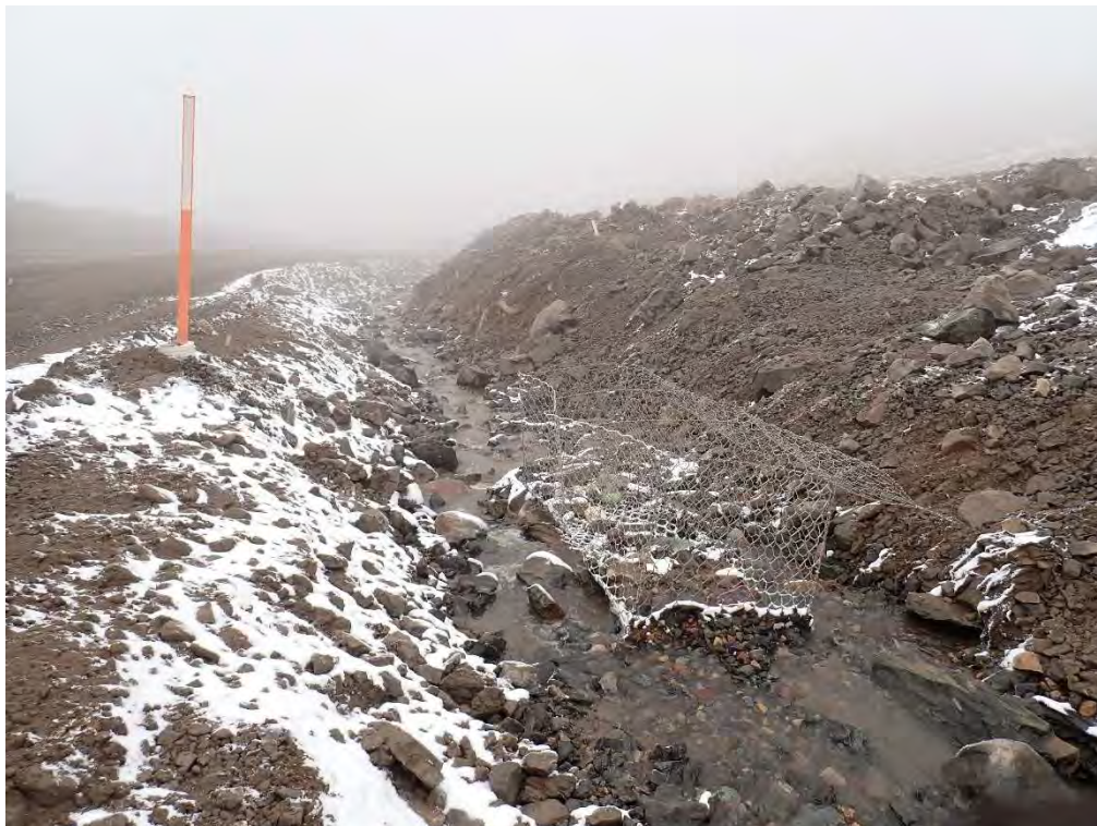
Photograph 8: Placement of Floc Blocs in drainage ditch of inflow to KM105 Pond
