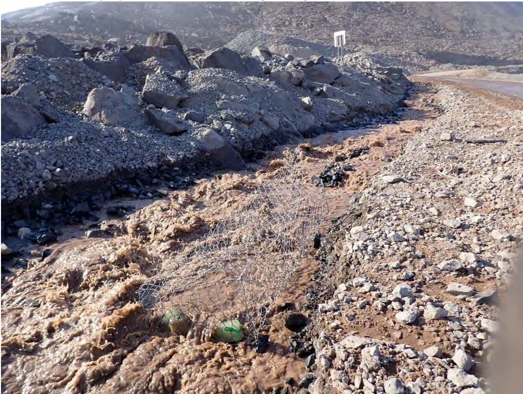
Photo 4: Passive polymer flocculent block cages, August 2023
