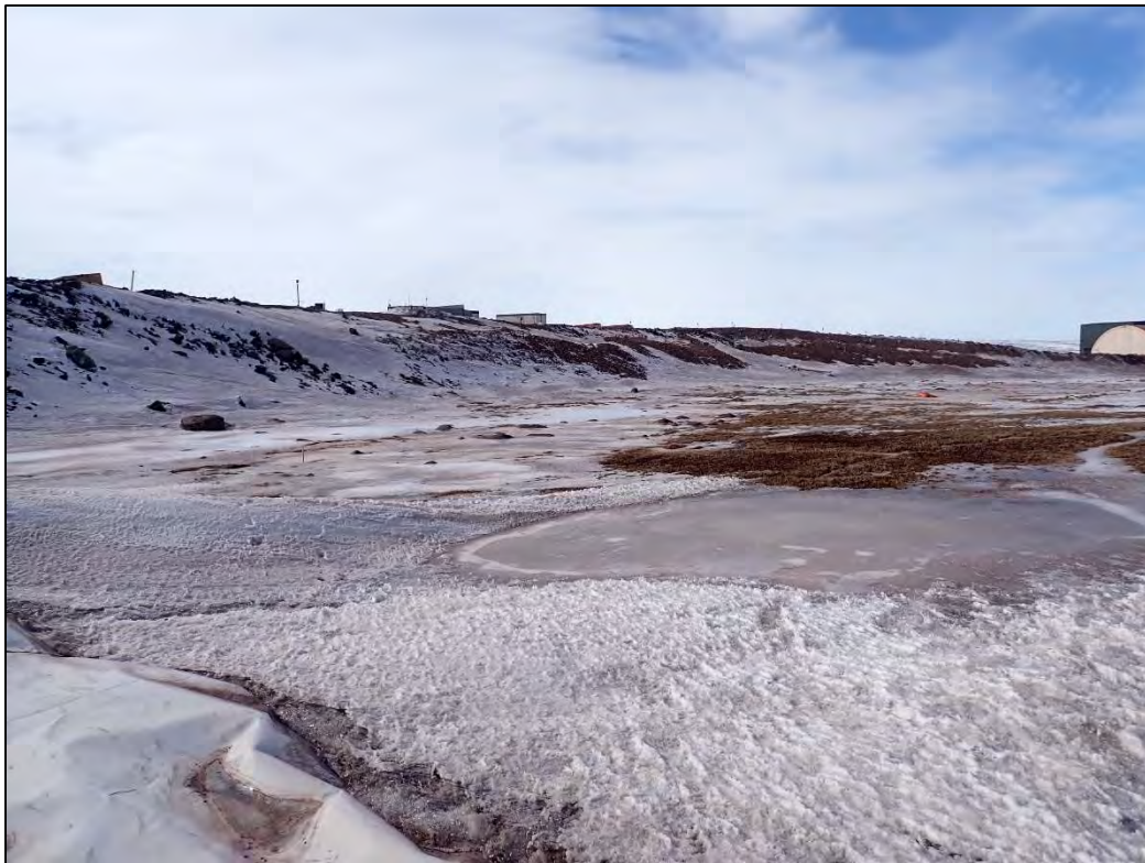
Photograph 2. Downstream showing no seepage from toe of dam to receiving environment, May 11, 2024
