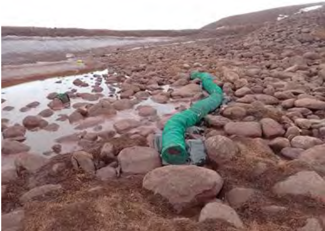
Photo 9: LDFG-OUT ESC Measures (Spring Berm/Floc Bloc) June 3, 2024
