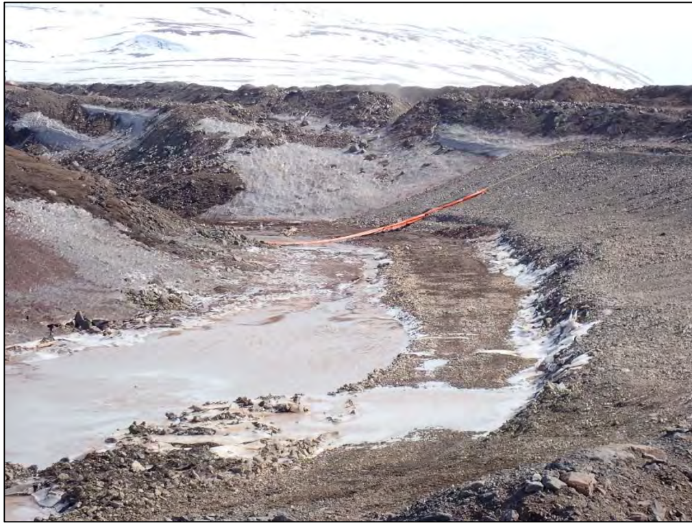
Photograph 7: Silt curtain installation
