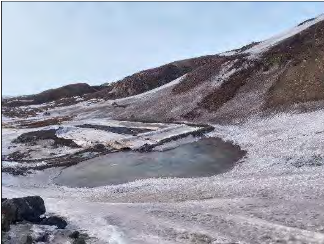
Photograph 1. Seepage from Toe of KM105 Dam on May 11, 2024
