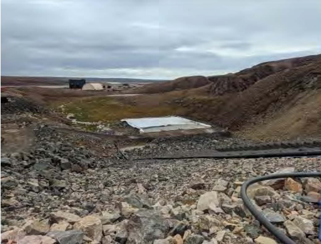
Photo 7: Construction of Geotube® Filtration System at the base of the KM105 Pond, 2023
