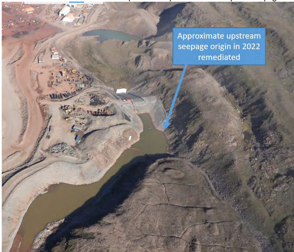
Photo 2: Remedial construction completed in September 2022 to patch seepage location
