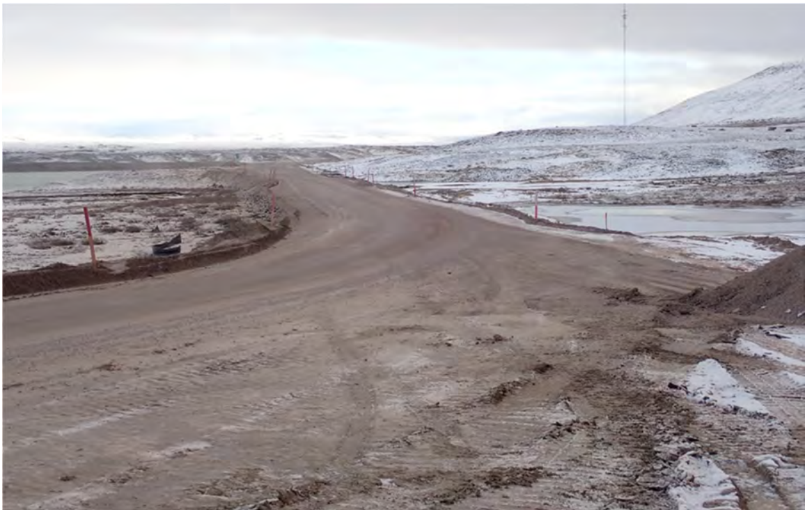
Photo 2: KM 87 Tote Road Remediated, Sand and Debris Cleared from Flood– October 9, 2024
