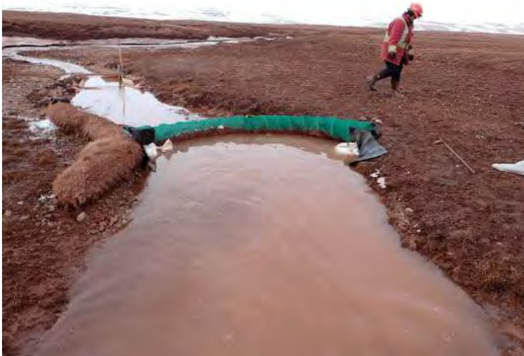
Photo 4: MP-C-B Freshet Monitoring Site with ESC (Reinforced Spring Berm) on May 30, 2024
