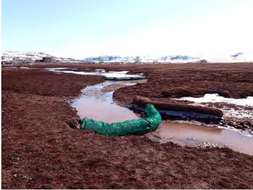
Photo 3: MP-C-B Freshet Monitoring Site with ESC (Additional Spring Berm) Installed on May 29, 2024
