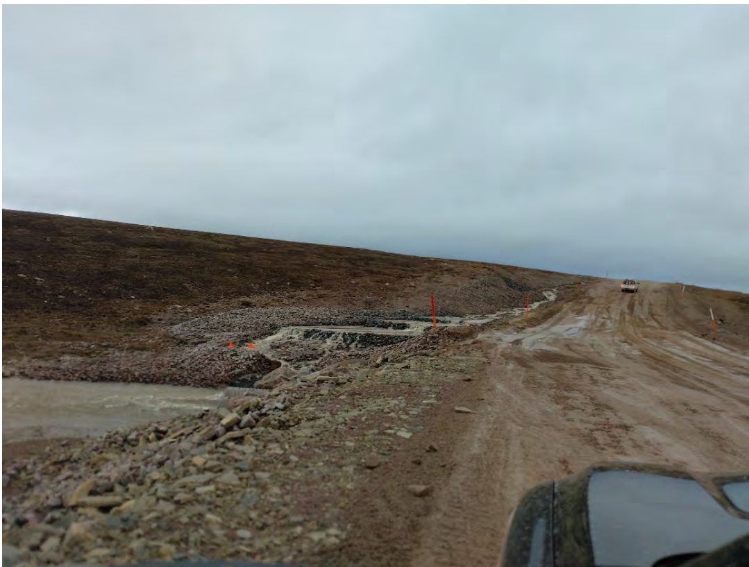
Photo 4: The KM 72 Dip Tote Road Following Road Resurfacing. Check Dams Adjacent to Road Operating as Designed – September 22, 2024
