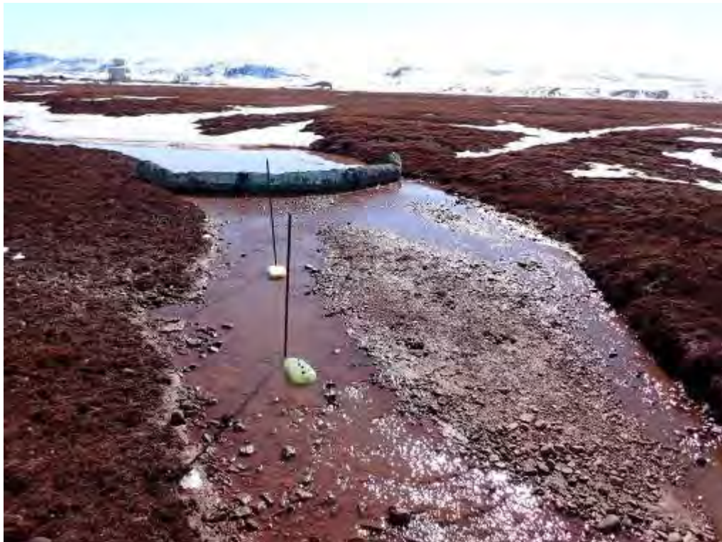
Photo 2: MP-C-B Freshet Monitoring Site with ESC (Spring Berm and Floc Blocs) Installed on May 26, 2024
