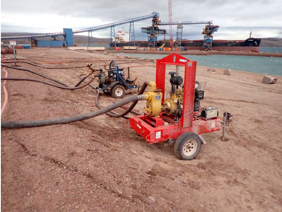
Photo 5: Controlled Discharge via Pumps Directly to Milne Inlet – September 22, 2024
