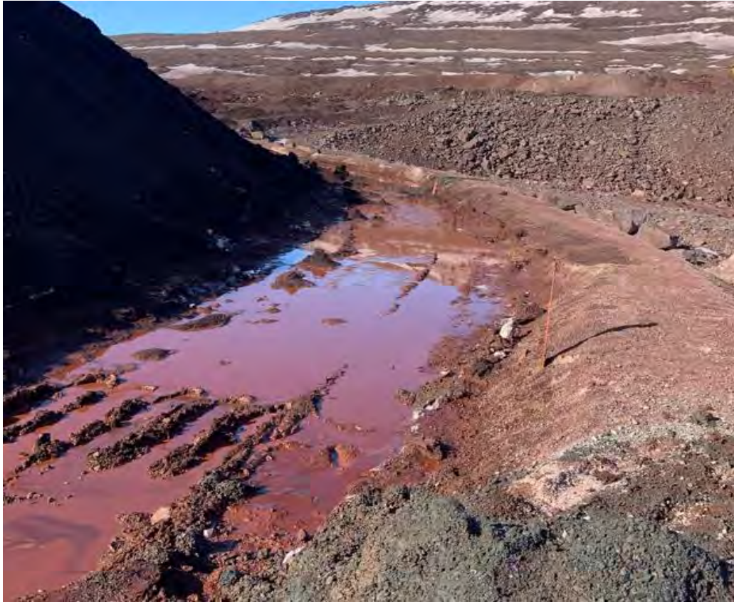
Photo 3: Embankment Berm Where Seepage Entered Perimeter Ditch – May 27, 2024
