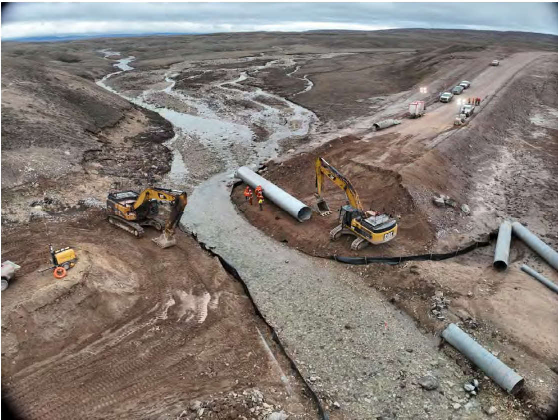
Photo 14: KM 63.5 and CV-049 Culvert Remediation - September 27, 2024
