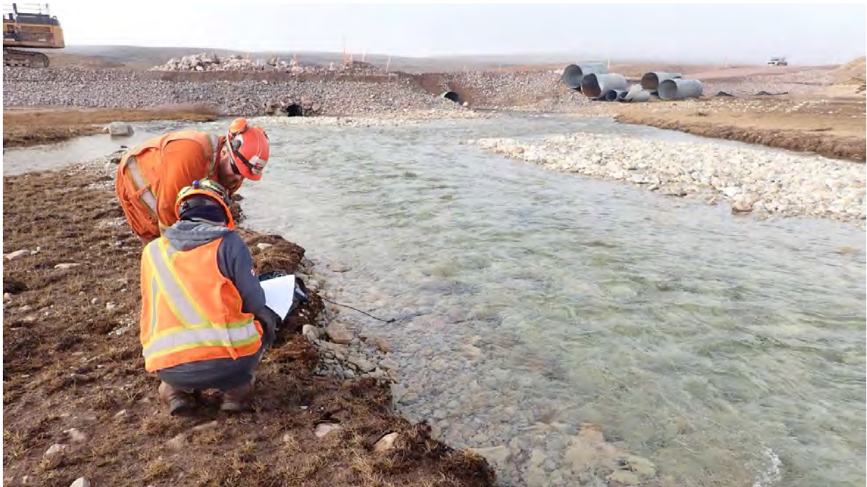
Photo 18: Rip-rap Placed along the Upstream Side of KM 51 Crossing – September 29, 2024
