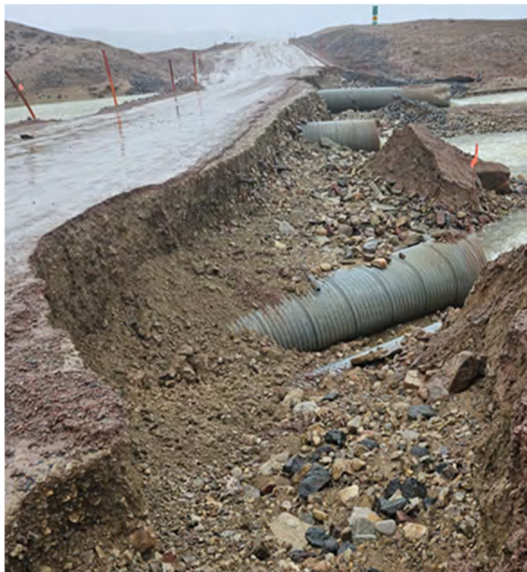
Photo 16: KM 51 Severe Road Degradation and Partial Washout – September 21, 2024
