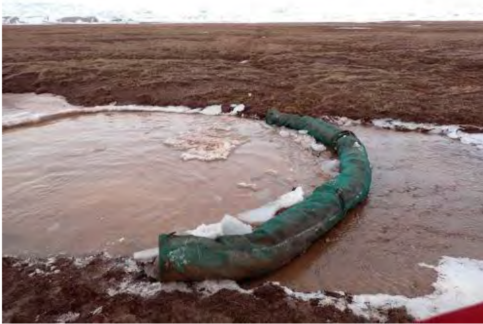
Photo 1: MP-C-B Freshet Site Upstream with ESC (Spring Berm) Installed on May 22, 2024
