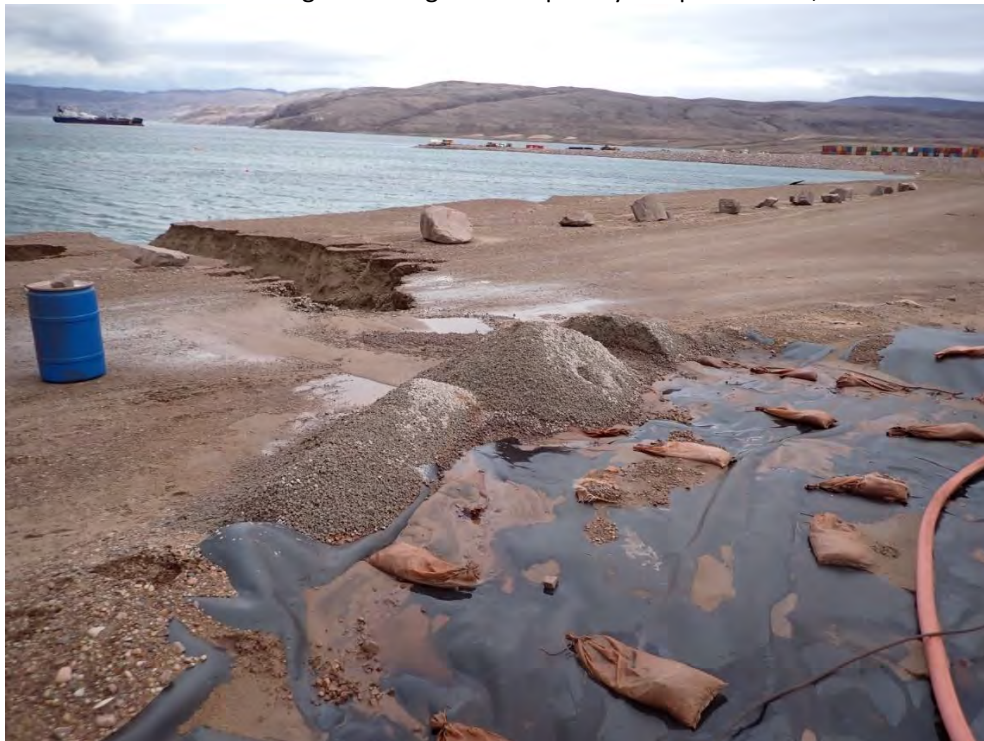
Photo 4: Erosion Down-Gradient of Engineered Spillway – September 22, 2024
