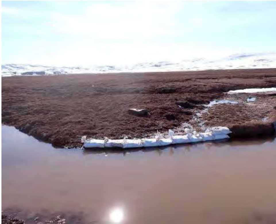
Photo 5: MP-C-B Freshet Monitoring Site with ESC (Sandbags) Installed on June 1, 2024
