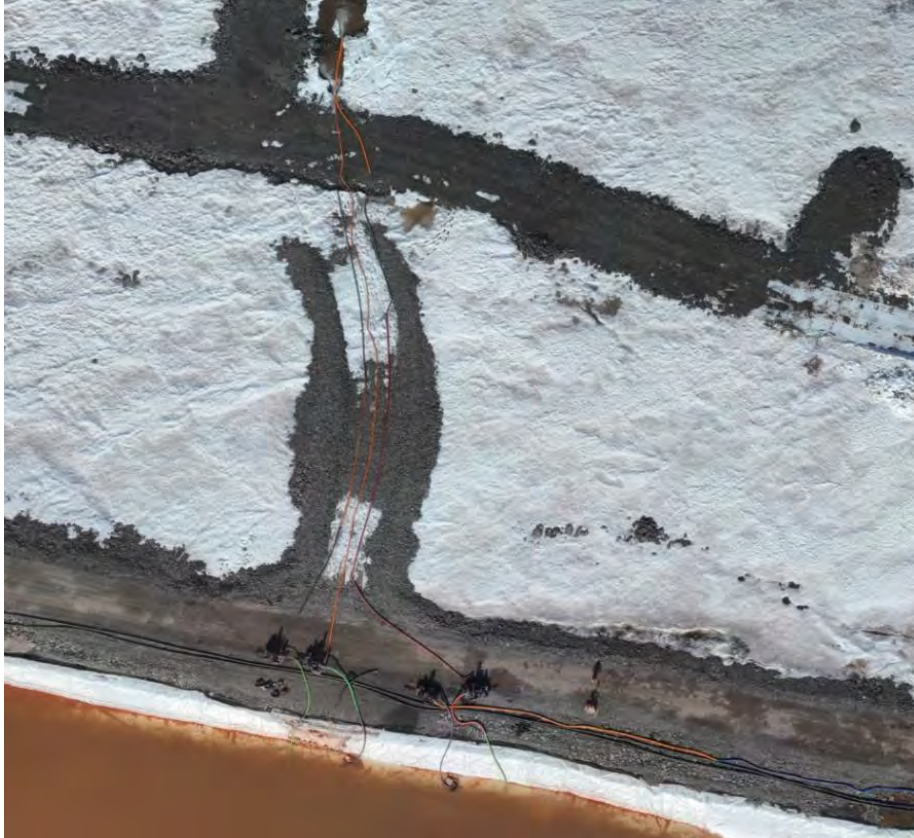
Photo 3: Additional pumps set up and discharging to lower water level in WRF Pond. June 24, 2024
