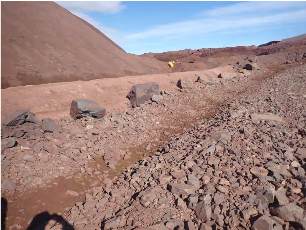
Photo 4: Reinforced Embankment Berm to Ensure Water Flows to MS-06 - June 24, 2024
