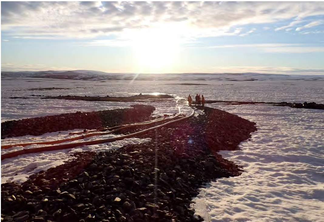
Photo 2: Discharge occurring over spill way onto frozen ground. June 24, 2024
