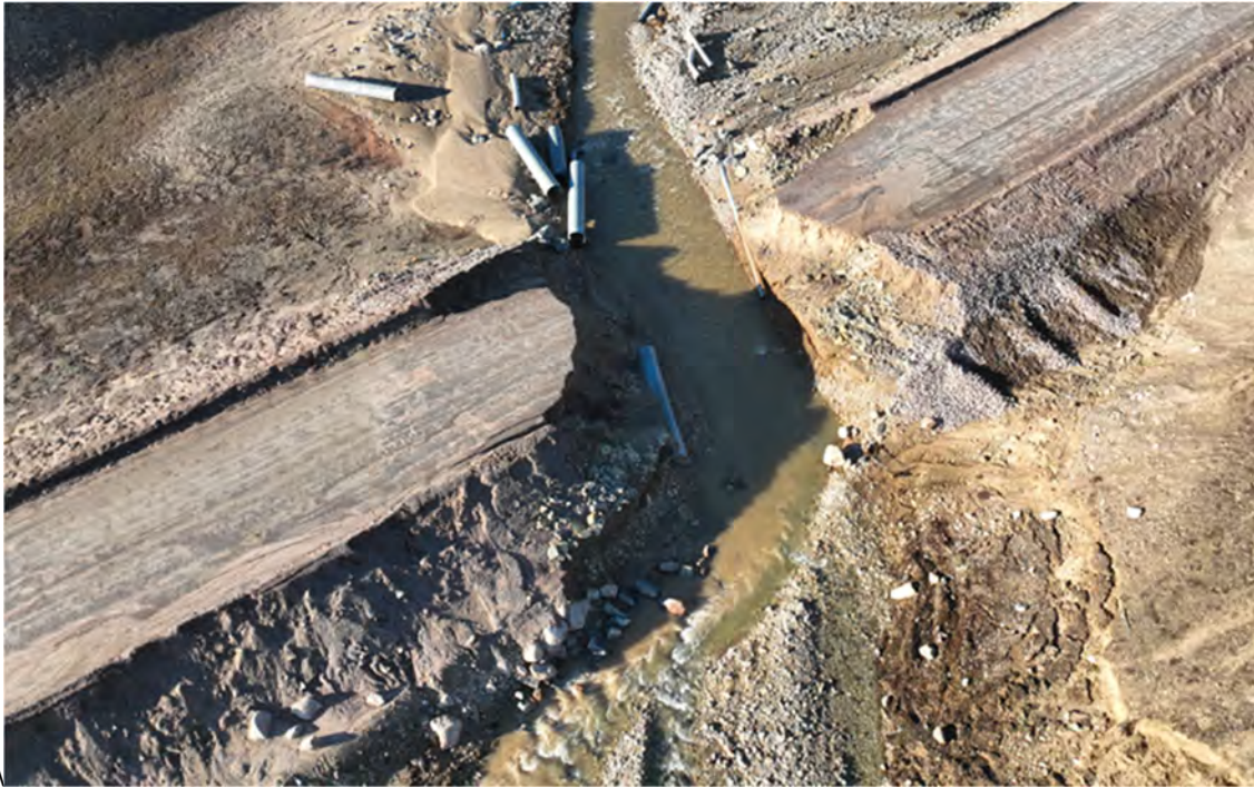
Photo 11: KM 63.5 and CV-049 Tote Road and Culverts Completely Washed Out – September 23, 2024
