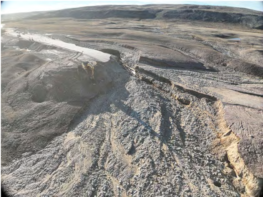
Photo 8: KM 64 Tote Road Completely Washed Out - Aerial View – September 23, 2024
