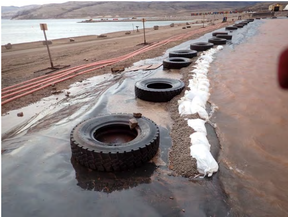
Photo 2: Sandbags Placed to Stop Uncontrolled Release at MP-05 Northwest Corner - September 22, 2024
