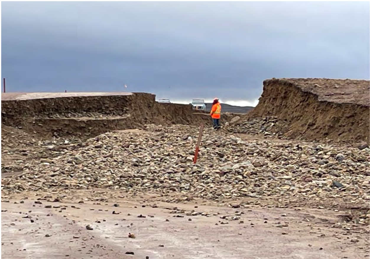
Photo 1: Complete loss of roadway at KM 63.5
