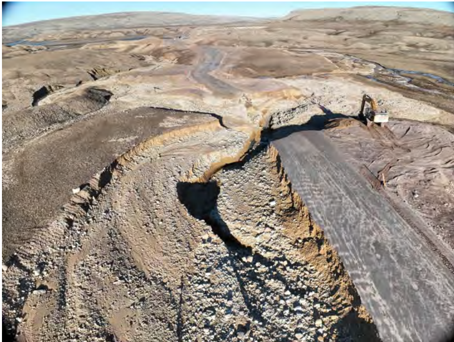
Photo 6: km 64 Aerial Photo Showing Damage to Roadway following Rainfall Event (September 23)
