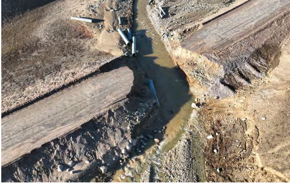
Photo 7: km 63.5 (CV-48) Aerial Photo Showing Damage to Roadway following Rainfall Event (September 23)
