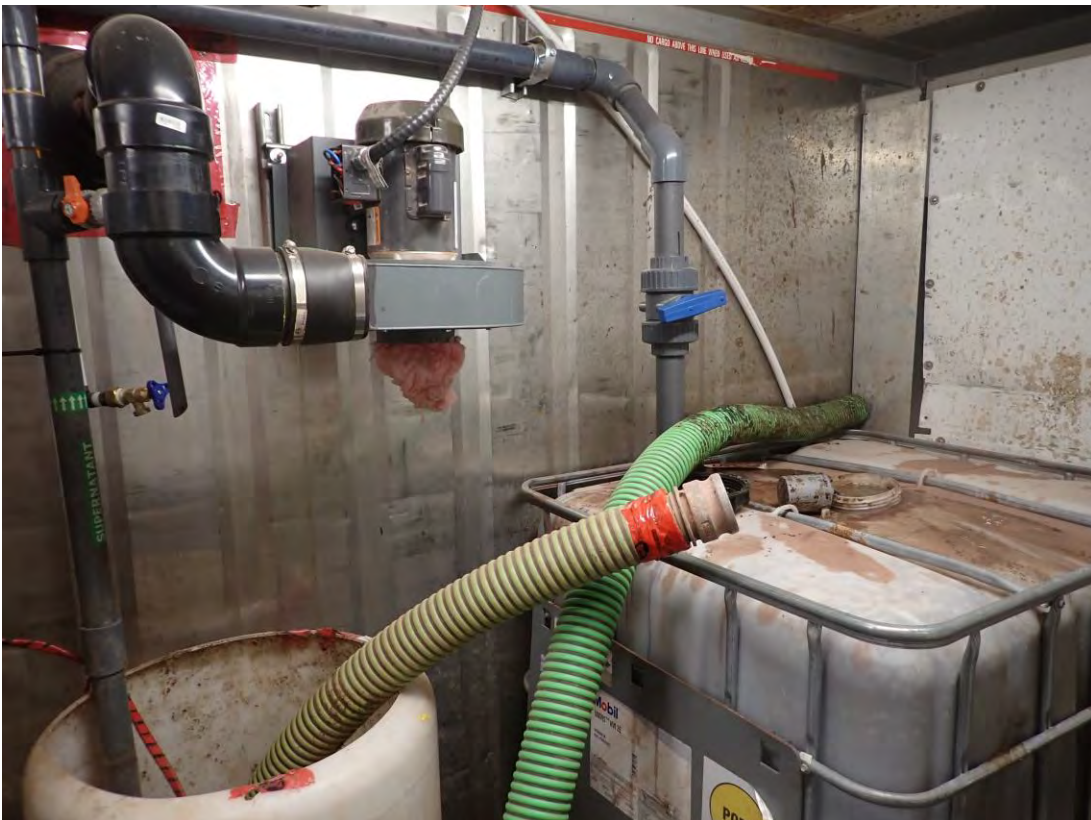
Photo 2: Tote inside Milne Port 380 WWTP that overflowed, resulting in release – December 12, 2024
