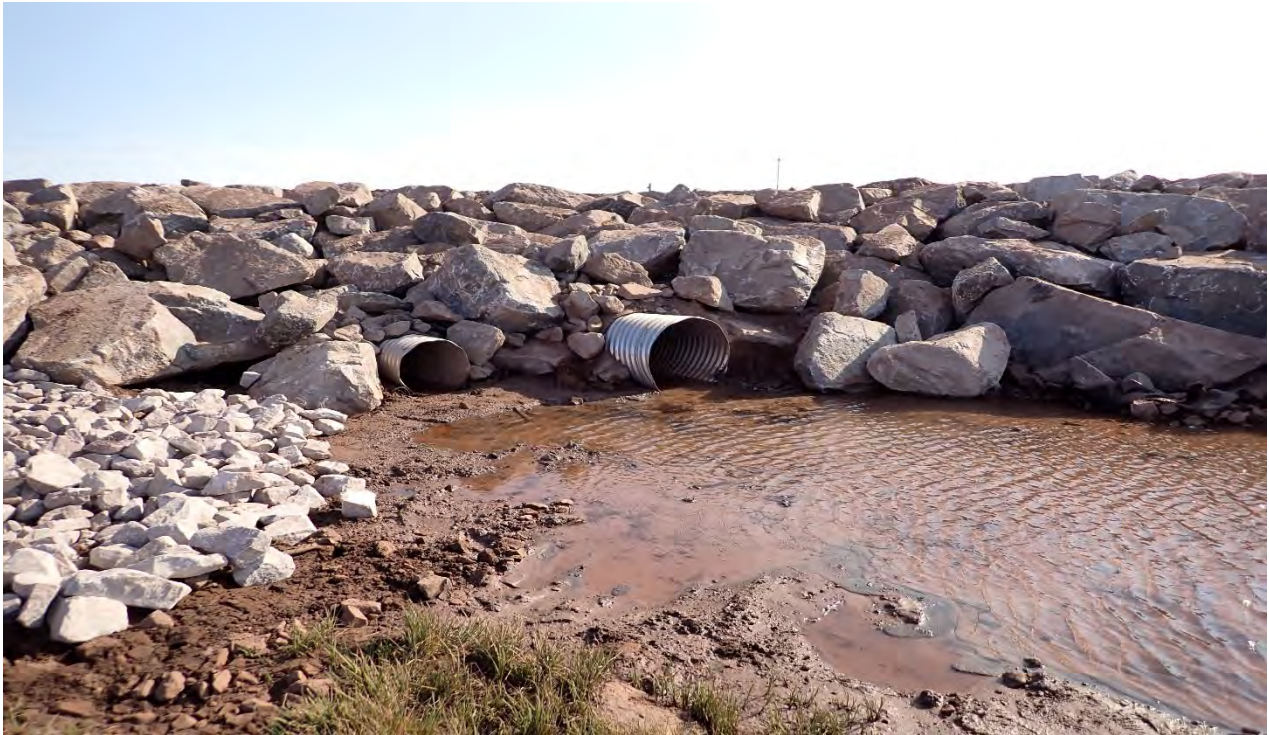
Photo 11. Downstream embankment armoured with over-sized rip rap, 2025-06-27
