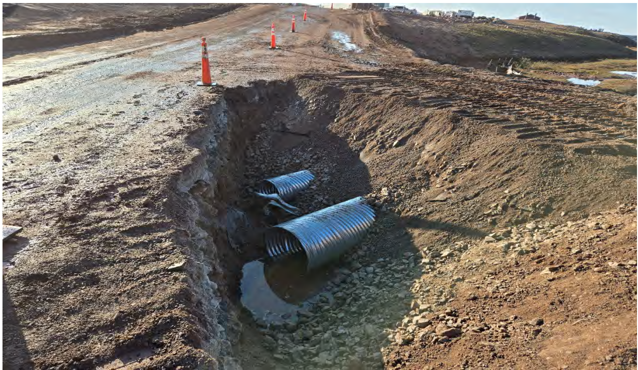
Photo 8. Upstream culverts backfilled and compacted, 2025-06-23
