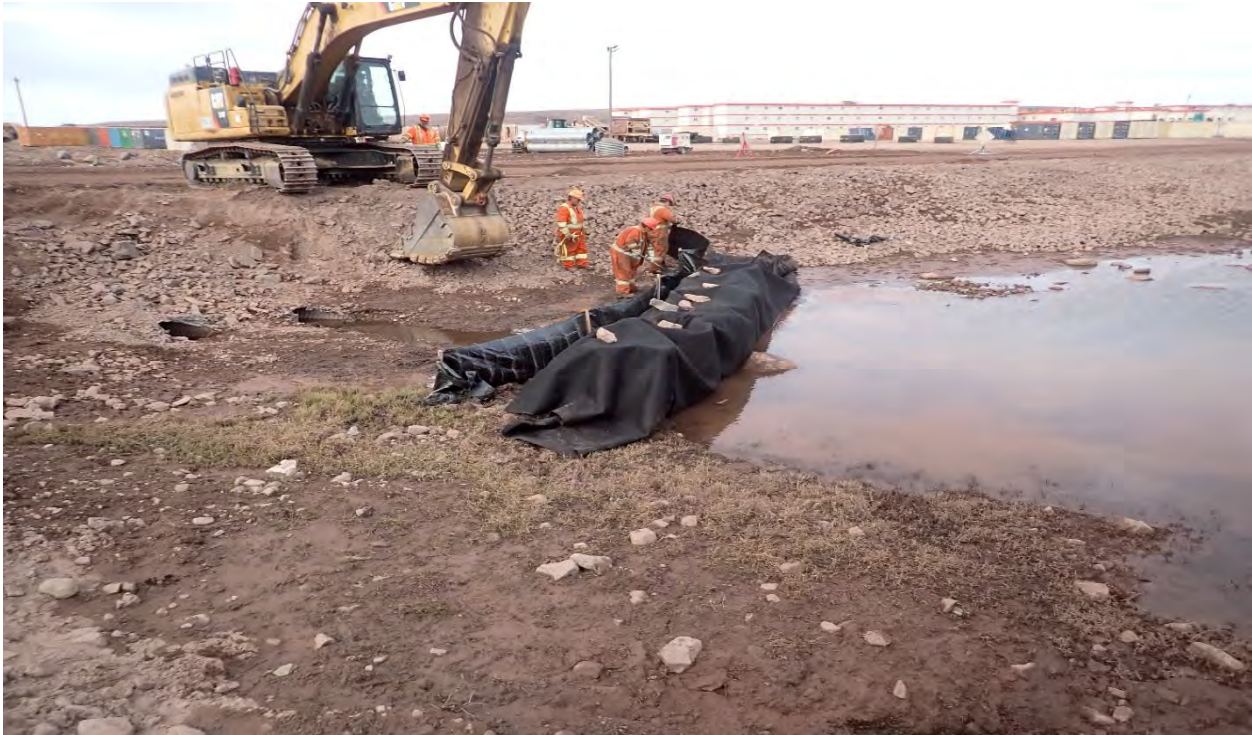
Photo 1. Downstream, looking south west, watercourse isolation and silt fence installed, 2025-06-21
