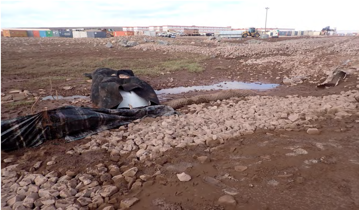
Photo 2. Upstream, looking west, watercourse isolation, silt fence and coir log installed, 2025-06-21
