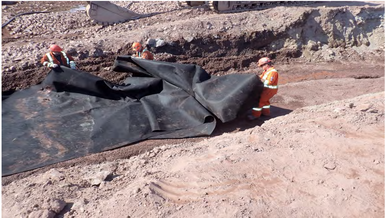
Photo 6. Installing non-woven geotextile over channel bed, prior to culvert placement, 2025-06-22
