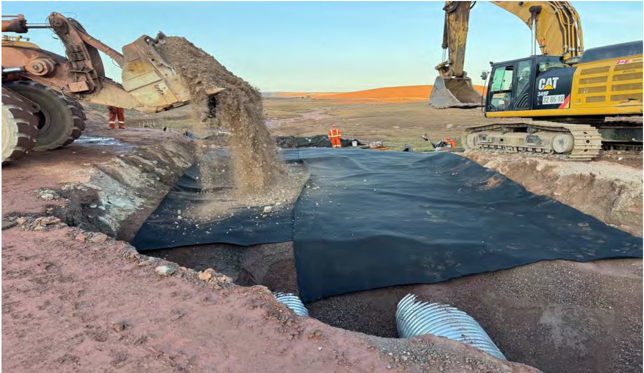
Photo 11. Placing road base aggregate over backfilled downstream culverts, 2025-06-24
