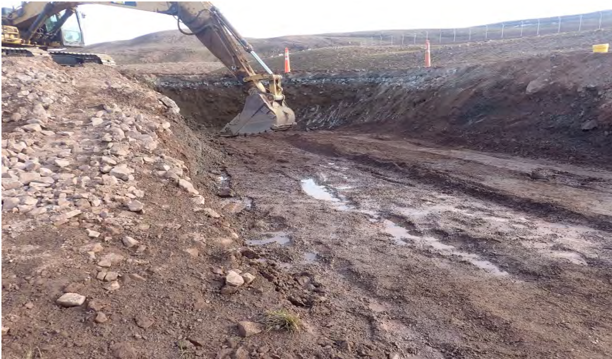
Photo 4. Upstream looking north, \frac{3}{4} " minus aggregate placement for crossing foundation, 2025-06-22
