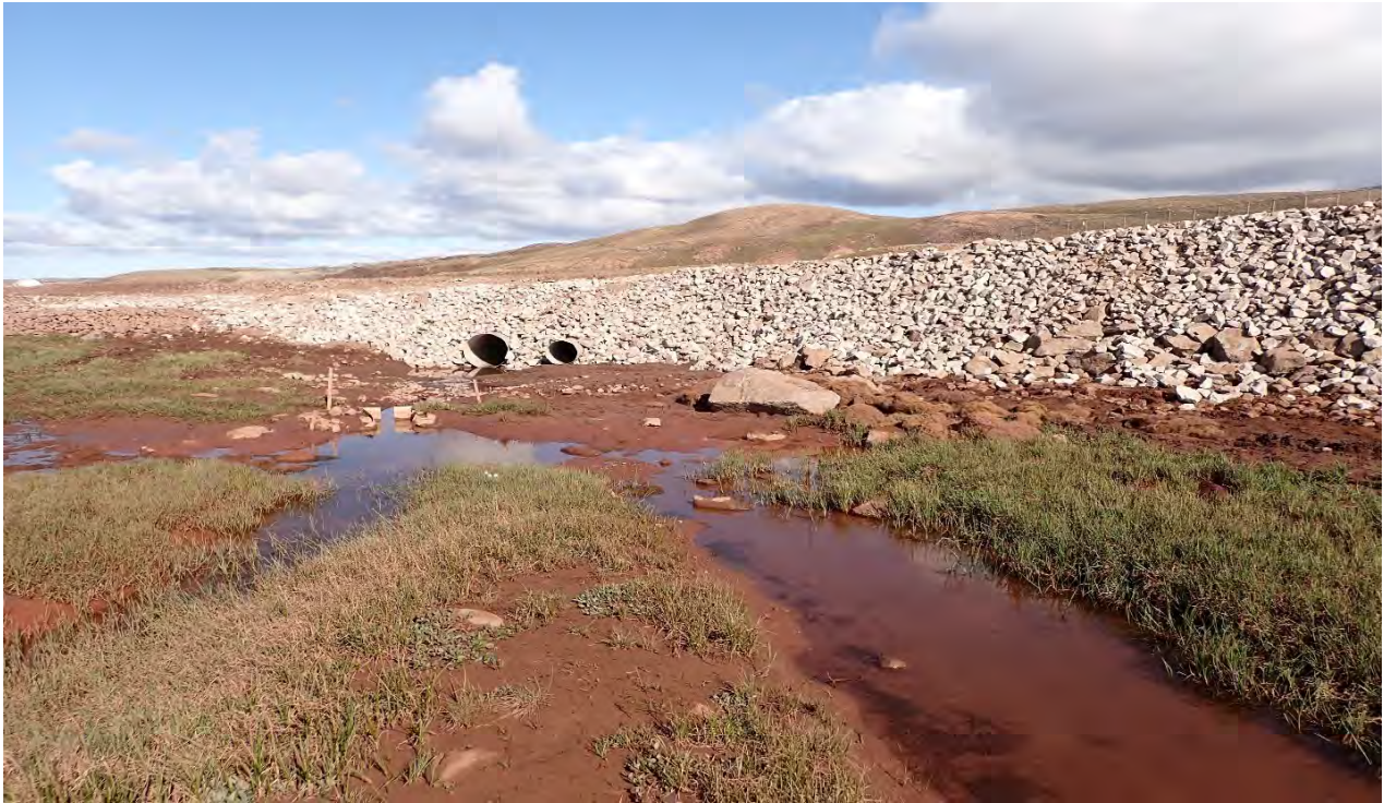
Photo 13. Upstream embankment armoured with 12" minus rip rap, 2025-06-29
