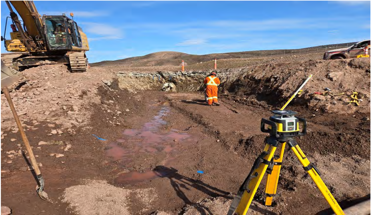
Photo 5. Survey and grading of channel to achieve proper slope for culverts, 2025-06-22
