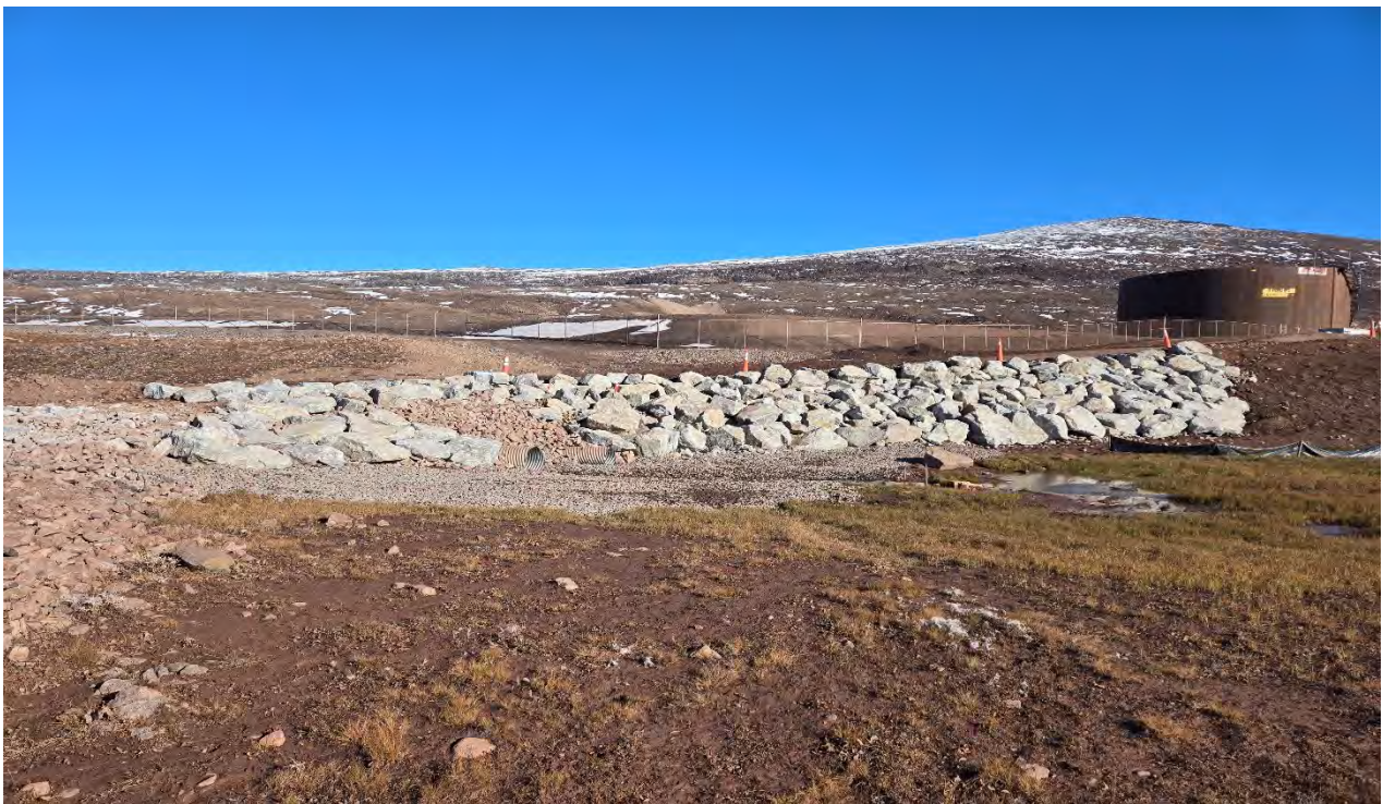
Photo 14. Upstream embankment re-armoured with over-sized rip rap, 2025-09-09
