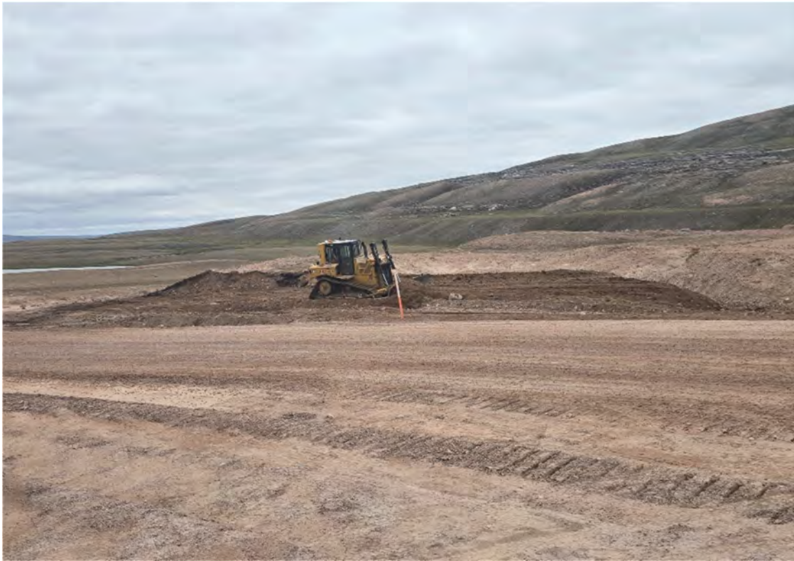
Figure D1. Regrading of Borrow Pit 71 using a CAT D6 dozer, July 2025
