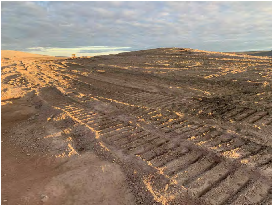
Figure C2. Post-reclamation site, surface grading, August 2025
