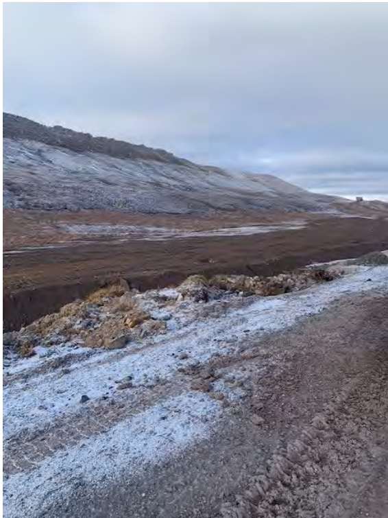
Figure B3. Site 14 and Site 14A after Reclamation Work, September 2025
