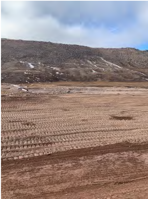
Figure B5. Site 14 and Site 14A after Reclamation Work, September 2025
