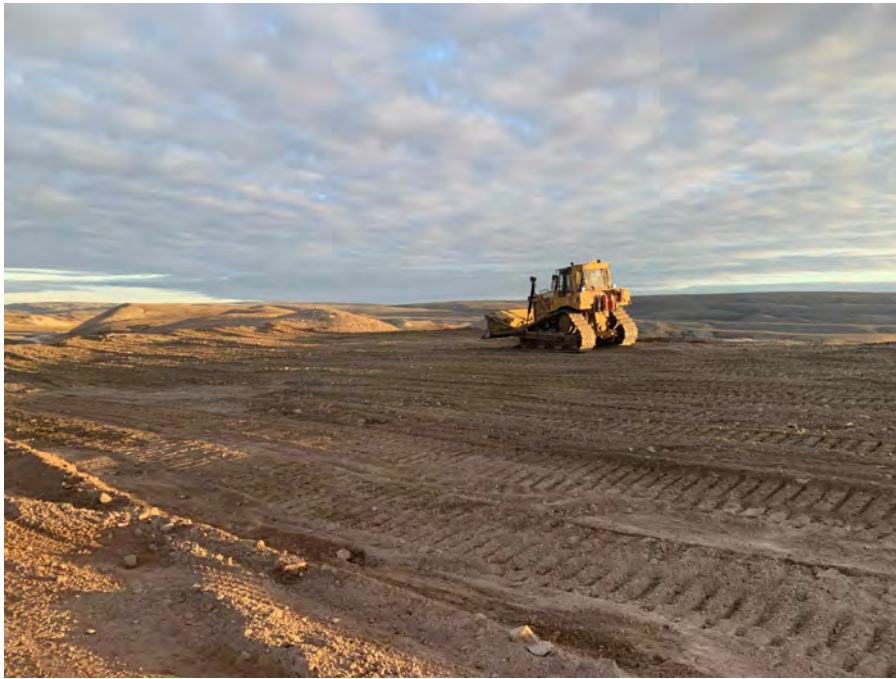
Figure C1. Regrading of Borrow Pit 41 using a CAT D6 dozer, August 2025
