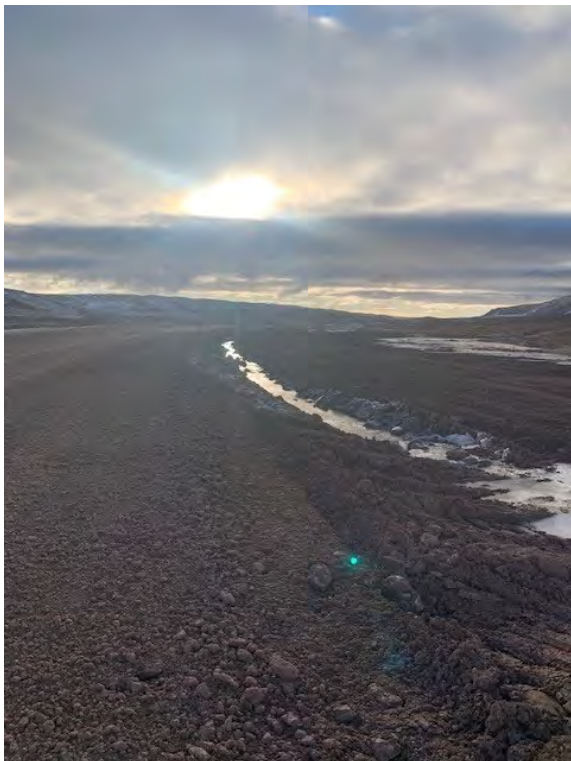
Figure B4. Site 14 and Site 14A after Reclamation Work, September 2025
