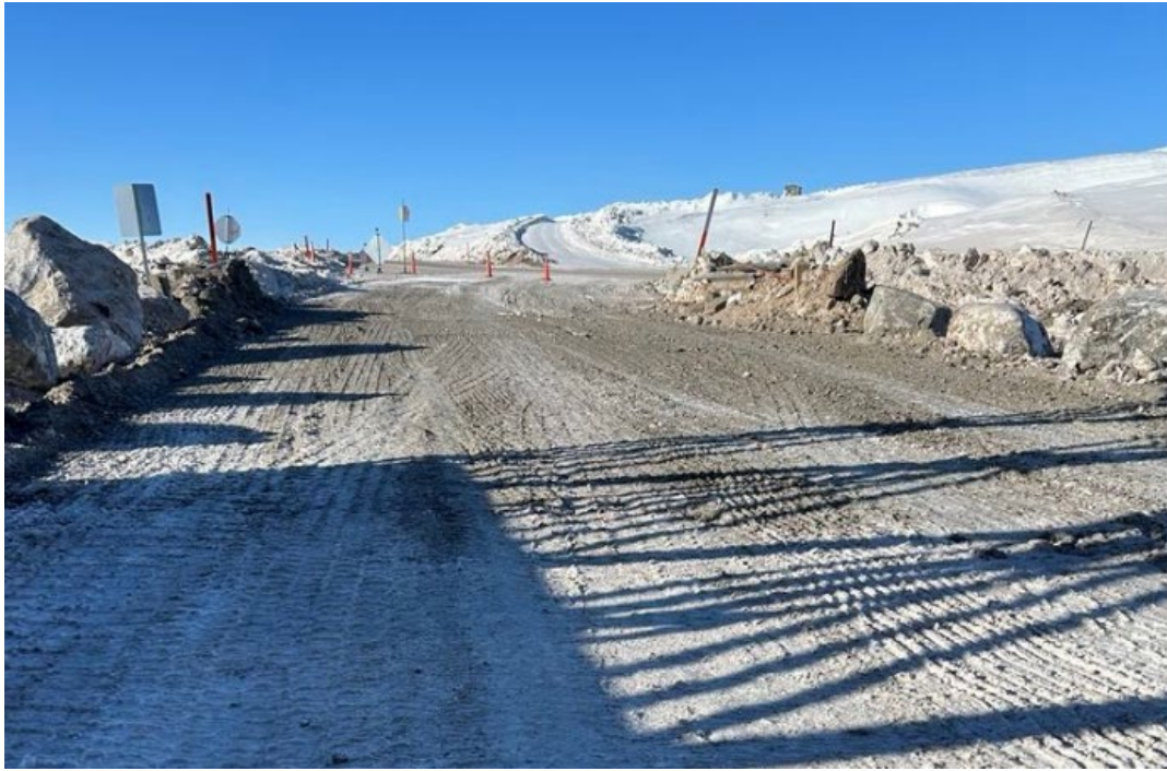
Photo 7. Bridge access road fully restored.
