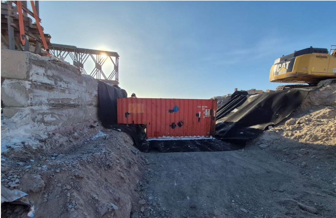
Photo 3. Typical Abutment support – customized 20' Seacan
