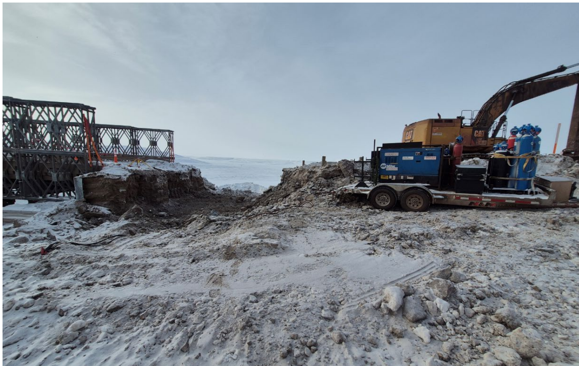
Photo 2. Typical excavation of abutment area
