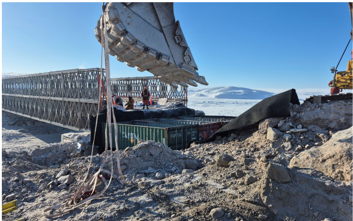
Photo 4. Four custom abutment anchors installed, awaiting rockfill.
