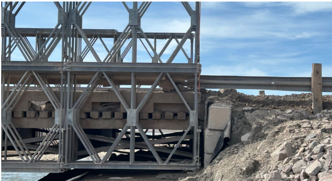
Photo 8. Post-construction condition of bridge sliding end
