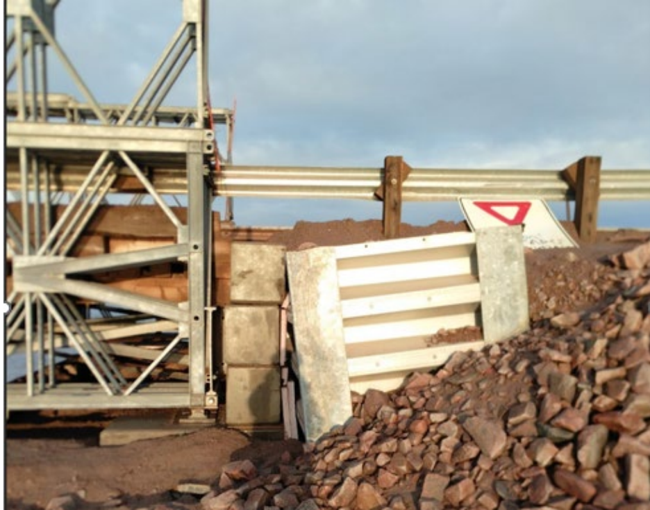
Photo 1. Pre-construction condition of bridge sliding end (typical)
