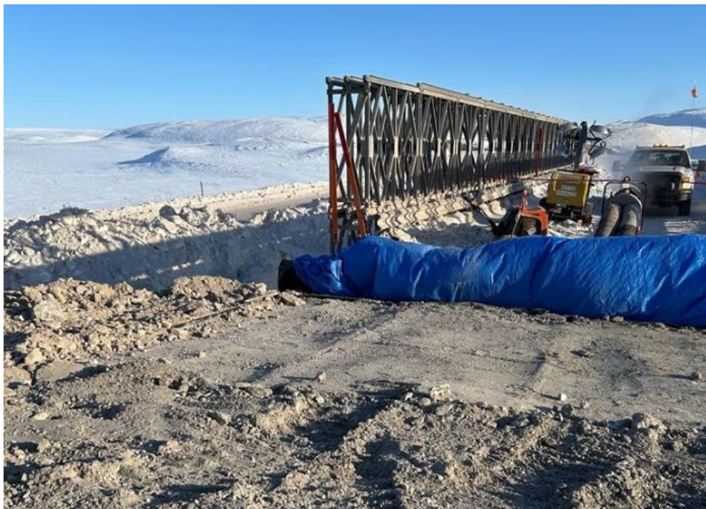
Photo 6. Abutment anchors fully backfilled
