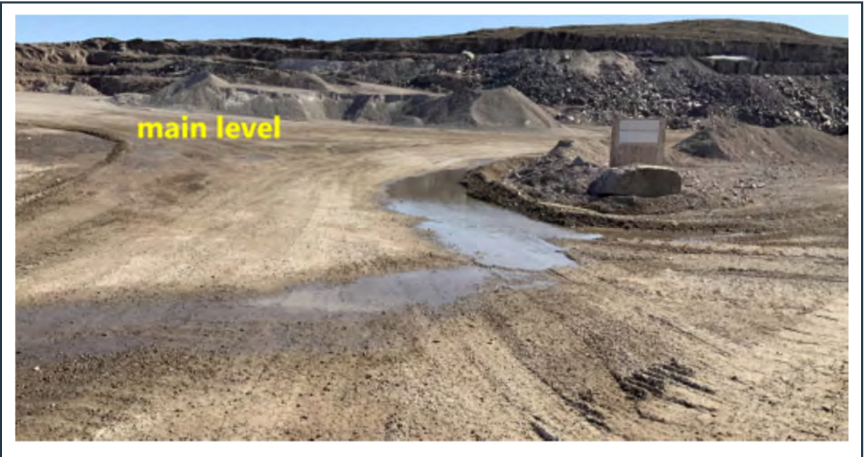
Figure 61: View of ponding and flowing water in many areas of the lower (main) level of the Q01 rock quarry. The drainage problem should be rectified prior to restarting the operation in the quarry.
