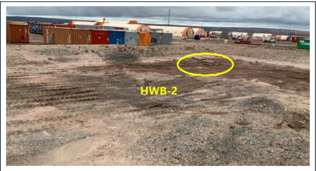
Figure 17: View of the stable berms around the currently empty HWB-2 cell. Debris from the cell (yellow circle) should be removed.
