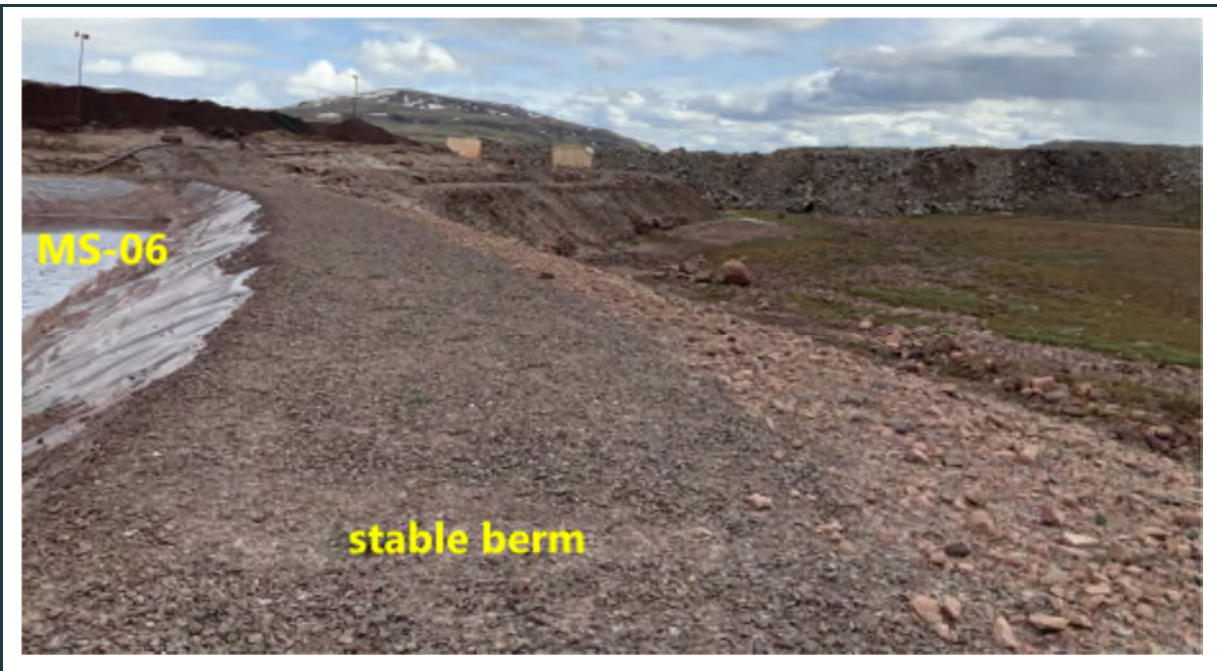
Figure 26: View of the robust, stable berm around the MS-06 pond, with intact liner.
