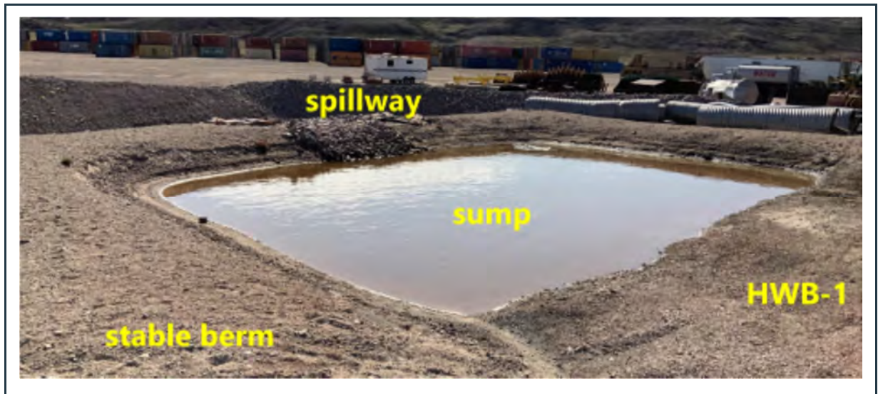
Figure 49: View of the sump and emergency spillway at the back of the HWB-1 cell with stable berm.
