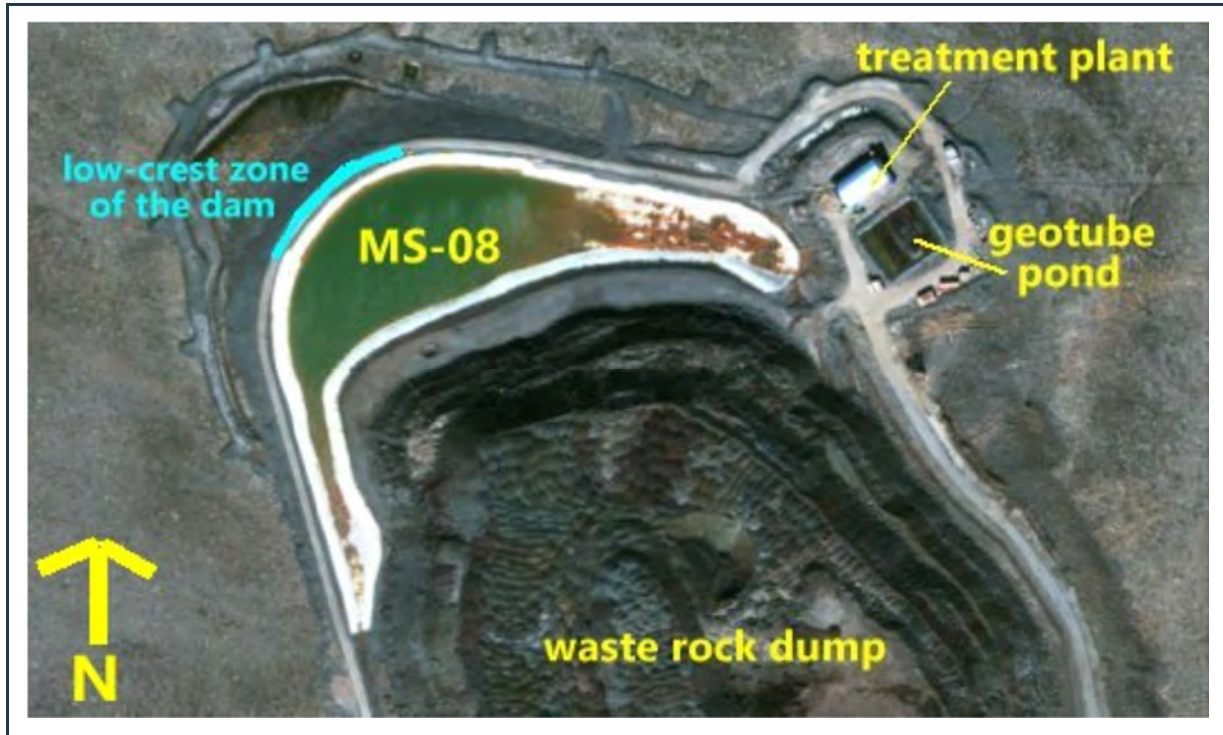
Figure 3: Mary River Mine Site Layout Map – North-Eastern Zone – Waste rock stockpile facility's sedimentation pond (MS-08) and geotube ponds - © 2023 Digital Globe, Inc.
