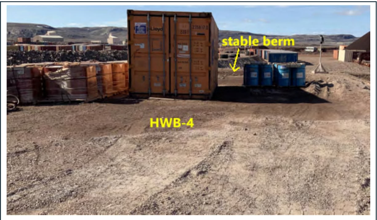
Figure 51: View of stable berm around the HWB-4 cell, storing jet fuel and a shipping container. Note the improved granular base within the cell, protecting the geomembrane liner.
