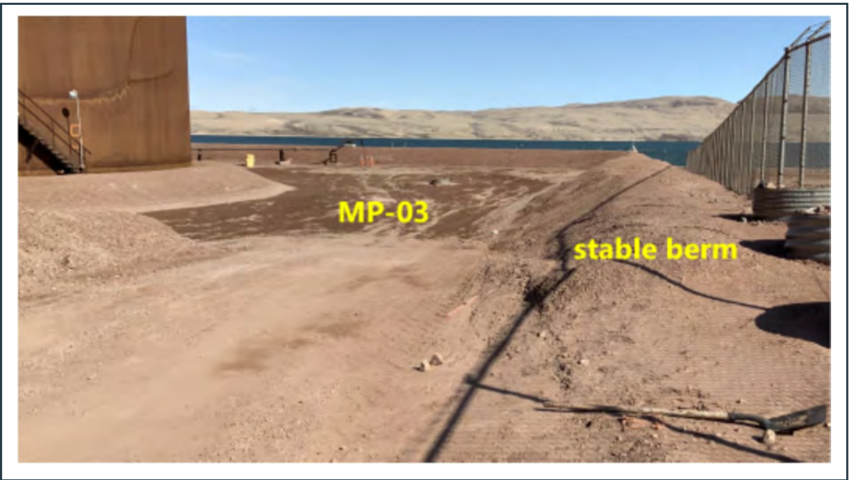
Figure 53: View of the well-maintained stable perimeter berm around the lined MP-03 fuel tank farm. Ponding water was recently removed from the facility.
