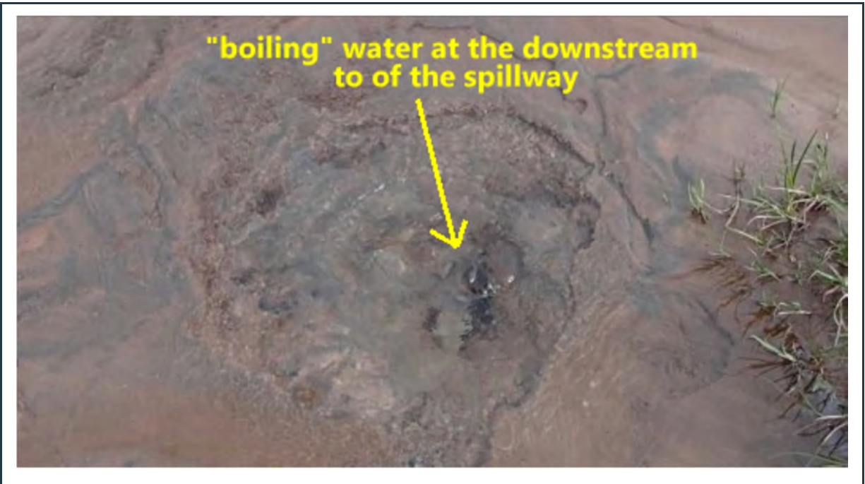
Figure 34: View of boiling water at the downstream toe of the spillway of the main dam at MS-11.
