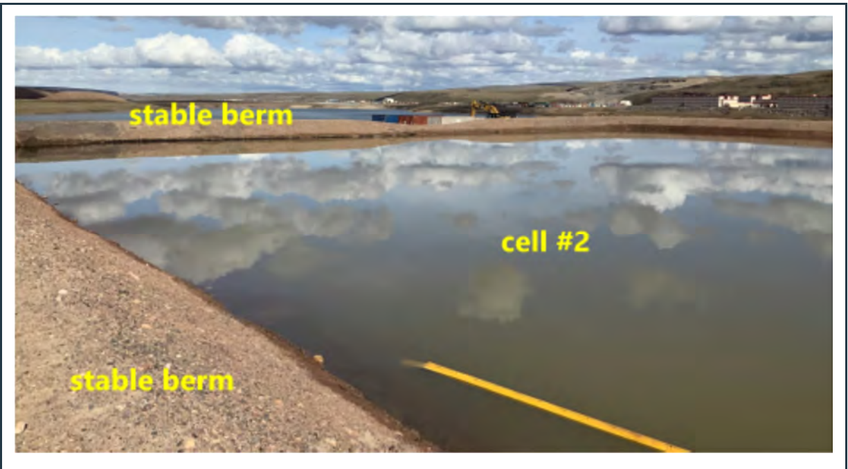
Figure 44: View of the stable berm around the currently empty, flooded cell #2 of the landfarm. The ponding water indicates good liner performance.
