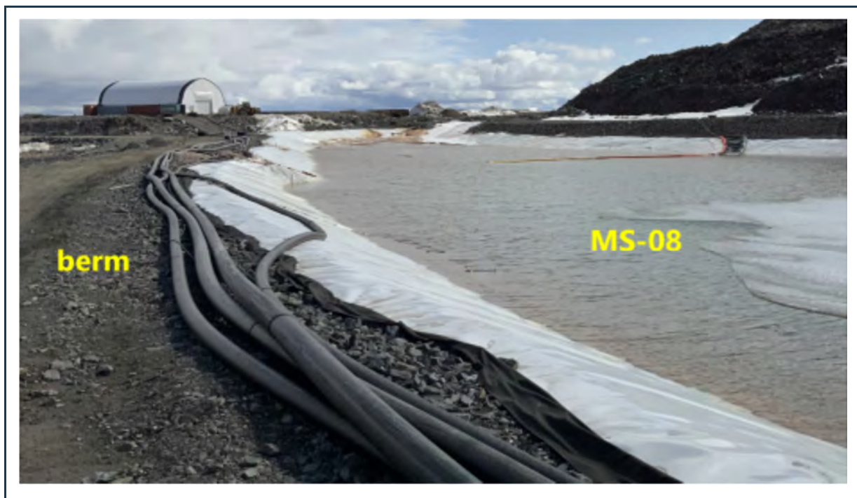
Figure 29: View of the stable, robust berm and intact liner at the MS-08 pond.
