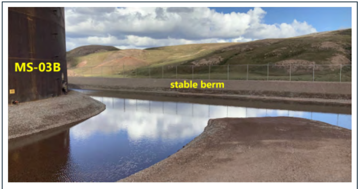
Figure 41: View of the well-maintained stable berm and interior granular fill over the liner at the new fuel tank farm. Note the ponding water in the cell, indicating good liner performance.
