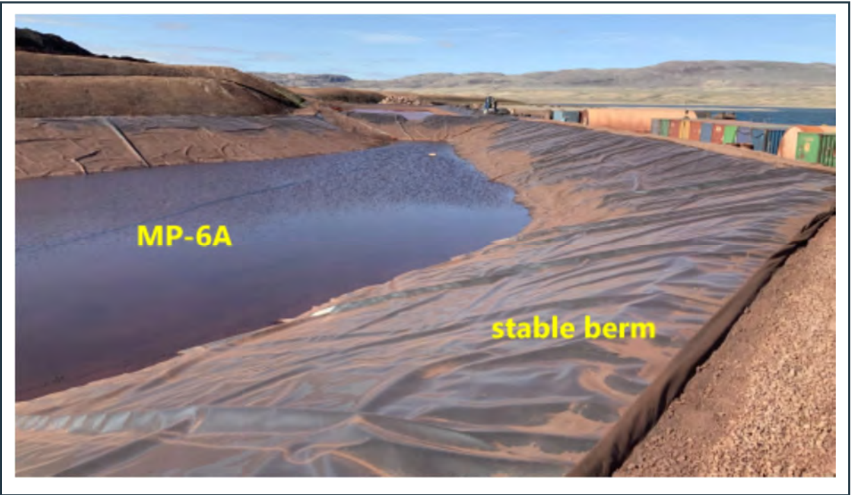
Figure 60: View of the lined MP-06A overflow pond with robust stable berms.
