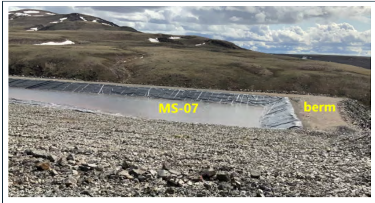
Figure 28: View of the robust, stable perimeter berm and intact liner at the MS-07 surface-water management pond at KM106.
