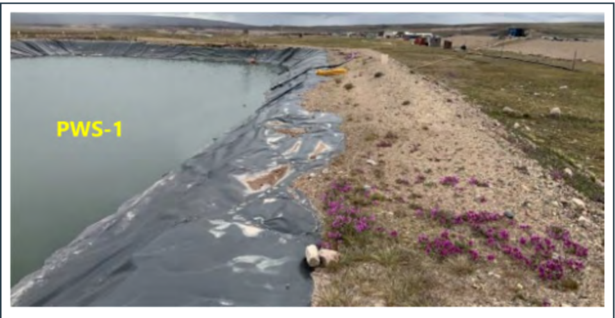
Figure 13: PWS pond #1. Well-maintained, stable perimeter berm and intact liner at the pond (July 2025).
