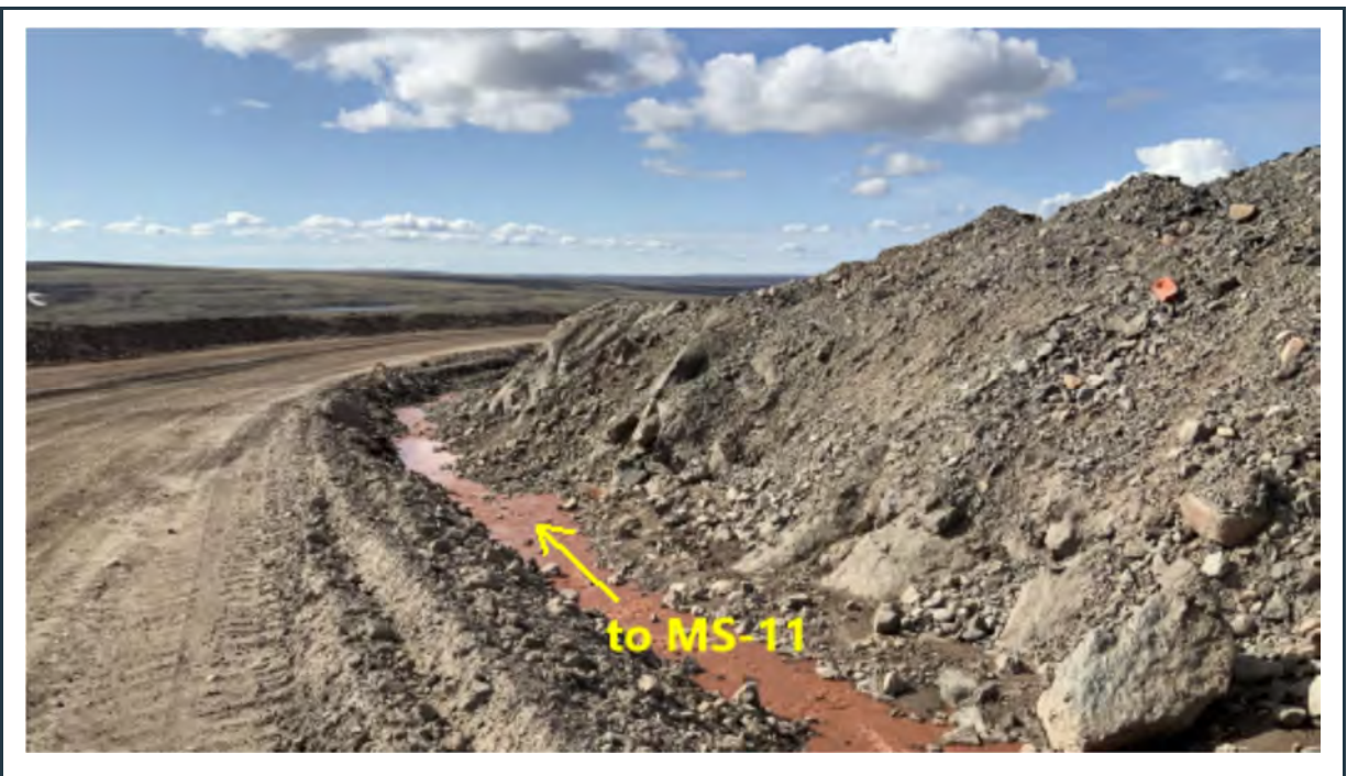
Figure 35: View of the side-ditch along the haul road draining surface water into the MS-11 sedimentation control pond. Note the muddy water in the ditch, entering the pond.
