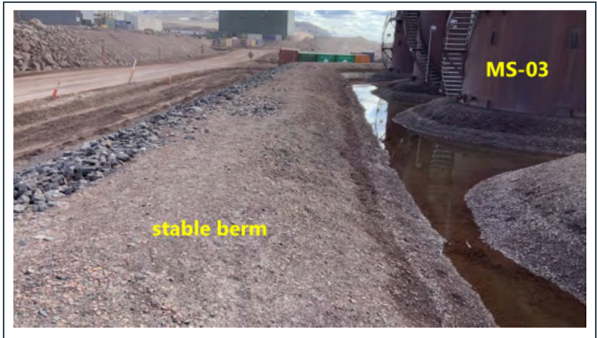
Figure 40: Well-maintained, stable berm around the MS-03 diesel fuel farm, with some ponding water, which is indication of good liner performance.
