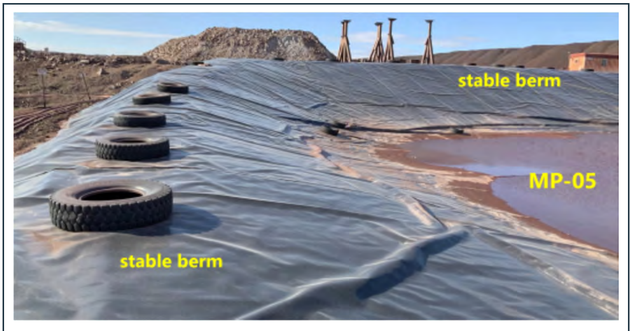
Figure 57: View of the robust, stable perimeter berm and intact liner at the MP-05 pond.
