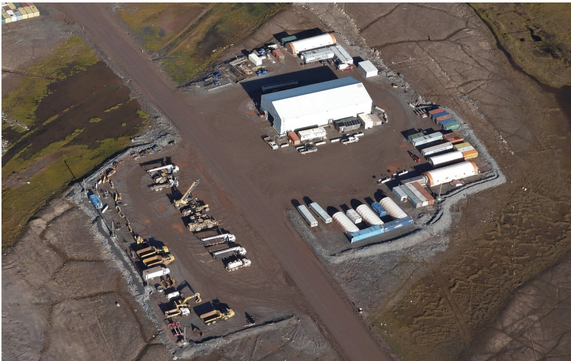
Photo 62. Site Services Building and Laydown – August
