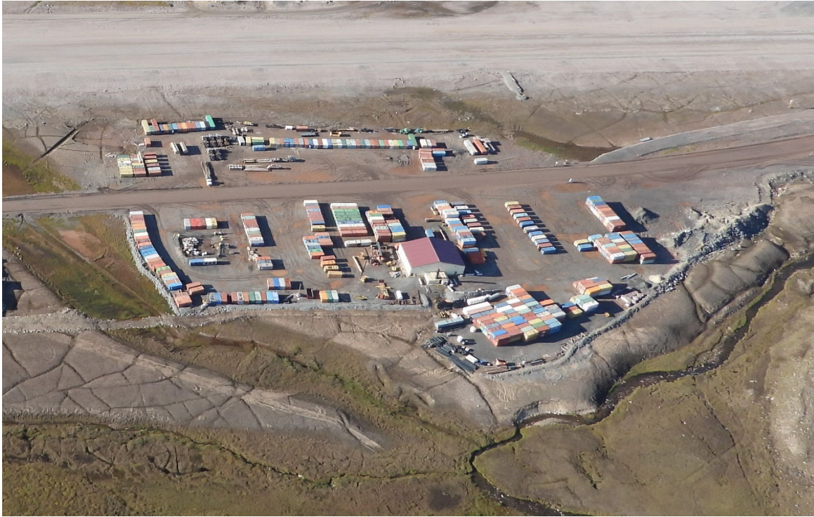
Photo 59. Incinerator Facility and Laydown – August
