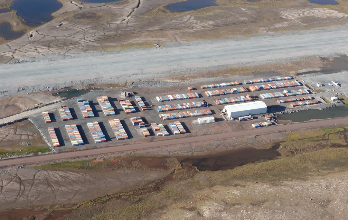
Photo 63. Warehouse Building and Laydown - August
