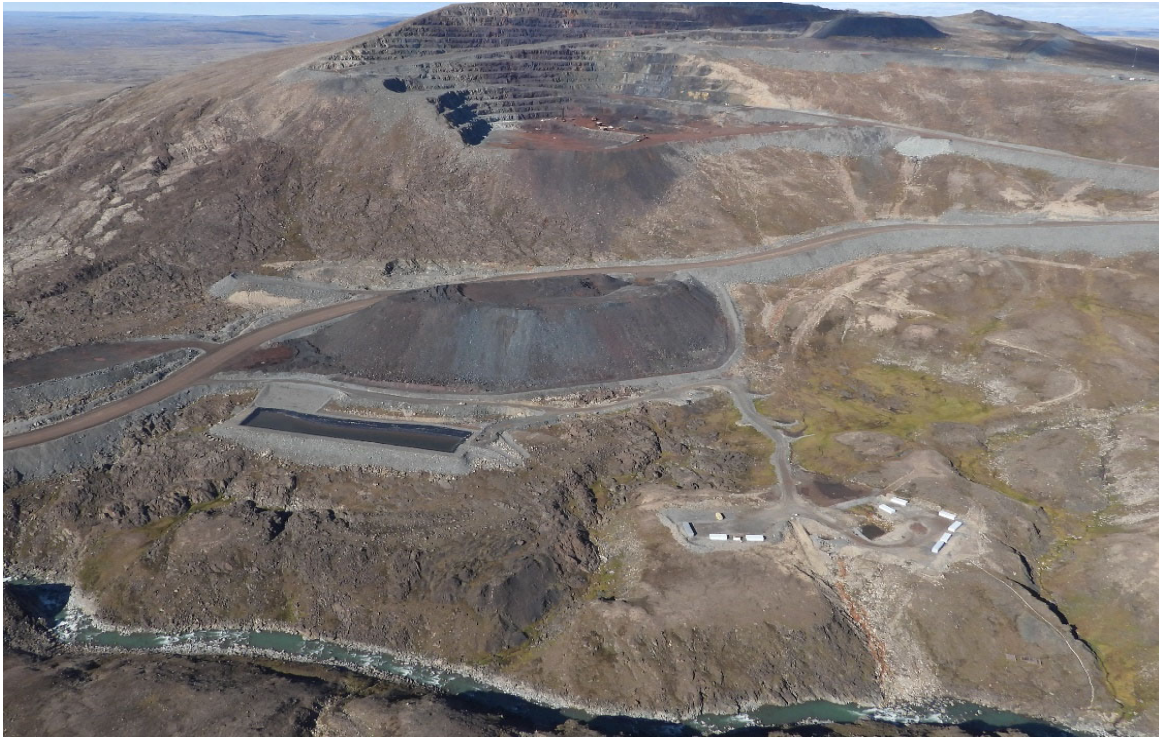
Photo 23. Run of Mine Ore Stockpile Facility - August
