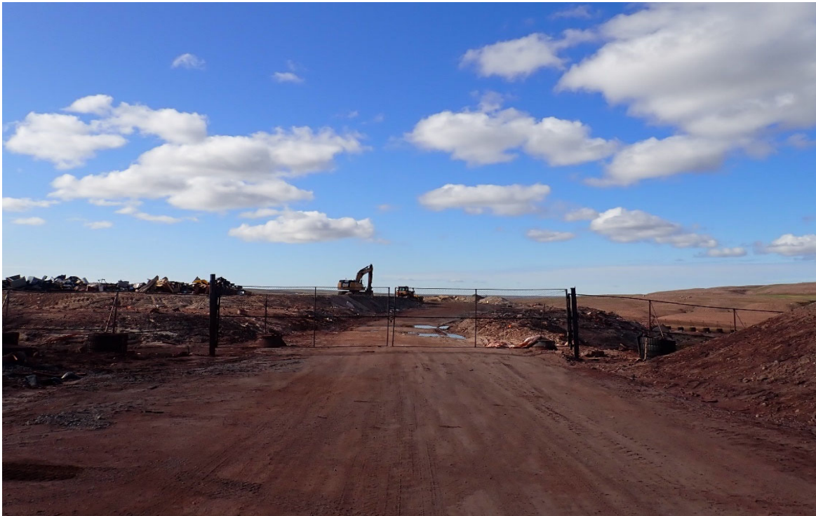
Photo 51. Non-Hazardous Waste Landfill Entrance – July
