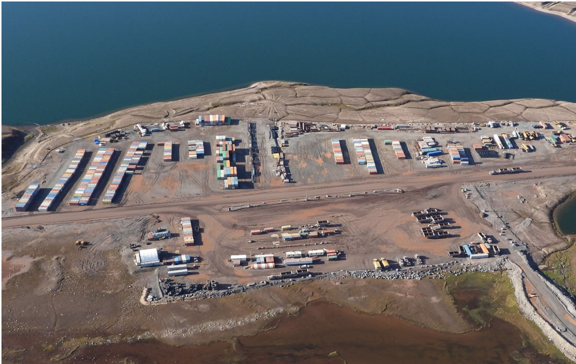
Photo 57. OHT Laydown and Laydown 2 – August
