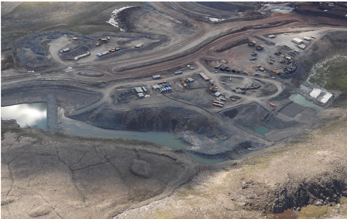
Photo 32. KM 105 Surface Water Management Pond (MS-11) - June
