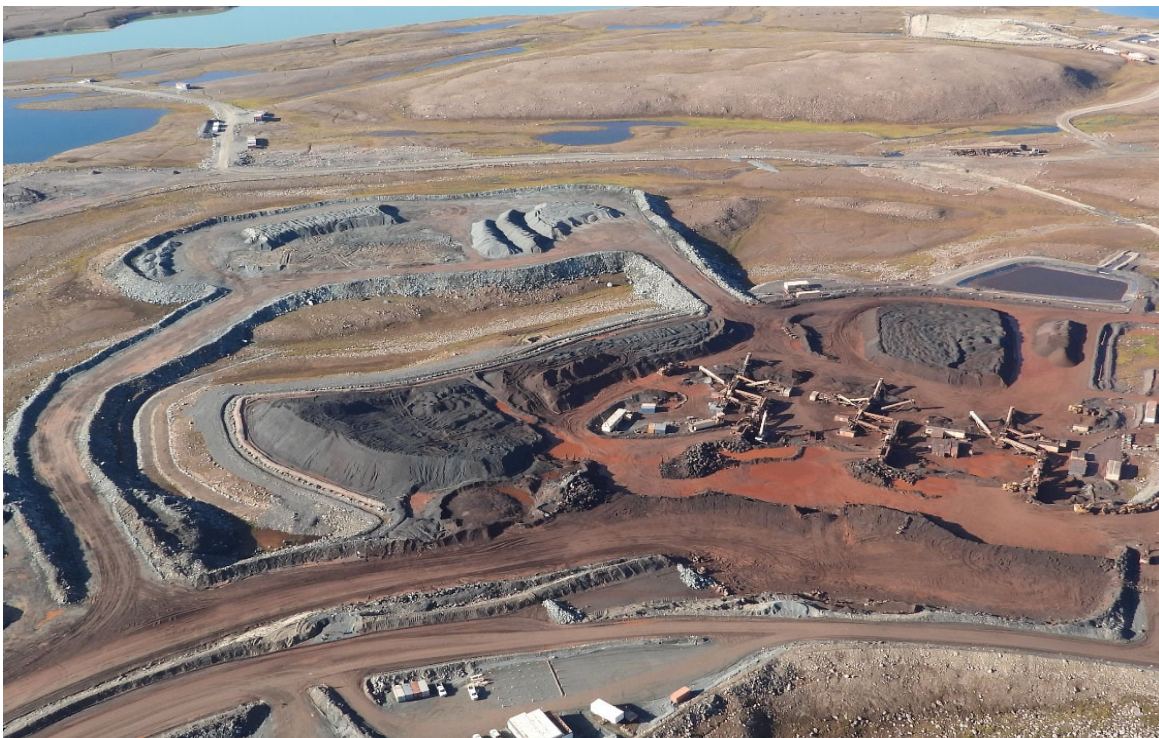
Photo 40. Ore Crushing Facility and KM 105 Steensby Aggregate Pad – August
