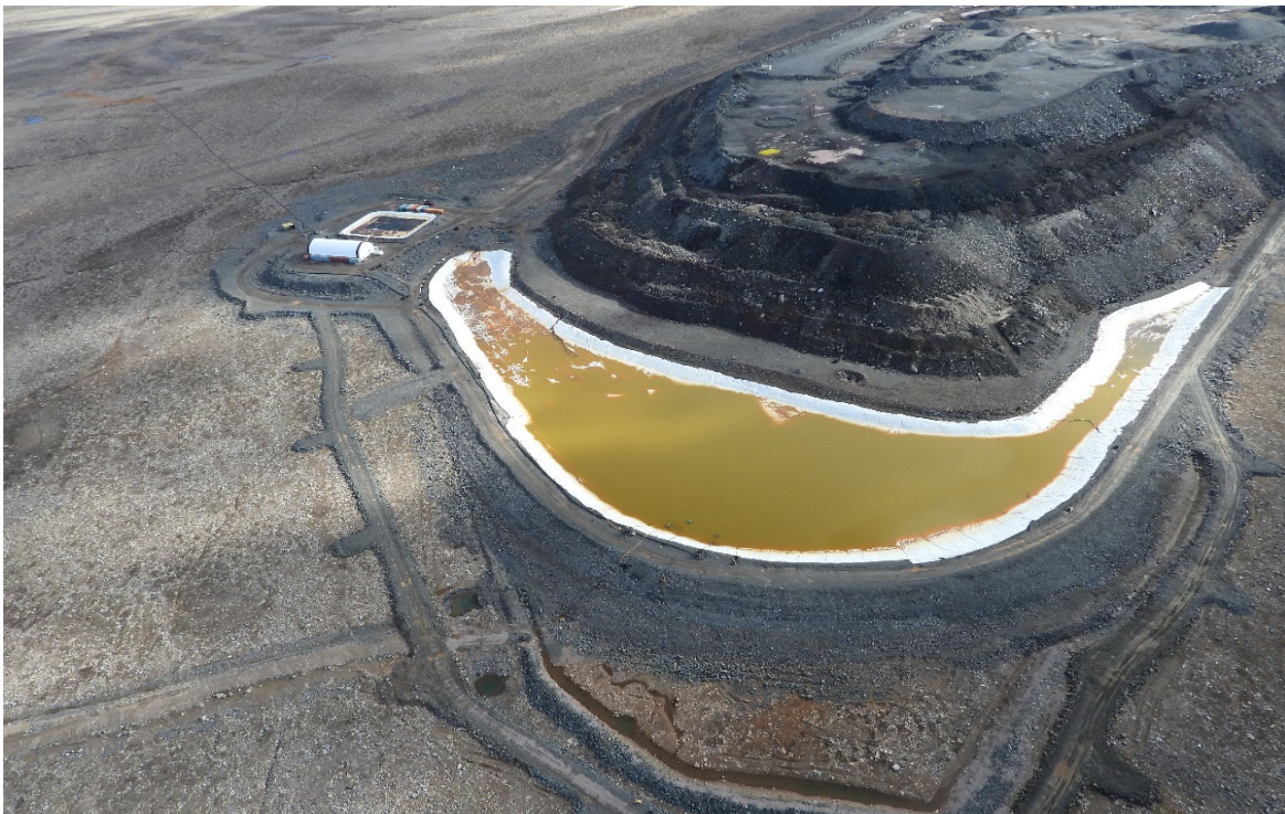
Photo 14. Waste Rock Facility Surface Water Management Pond (MS-08) - August
