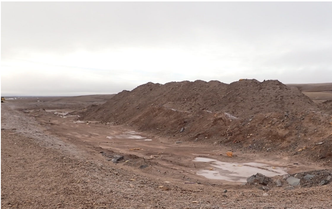
Photo 52. Soil Windrows in the Landfarm Facility Cell 1 - September
