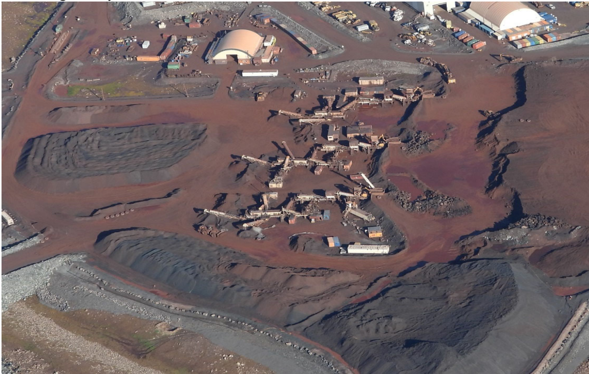
Photo 39. Stacked Lump and Fines at the Ore Crushing Facility – August
