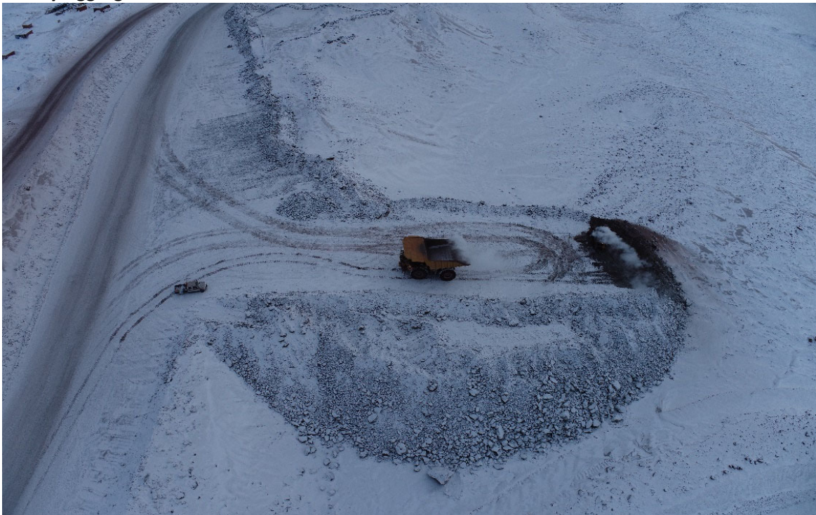
Photo 34. KM 105 Steensby Aggregate Pad Construction – February
