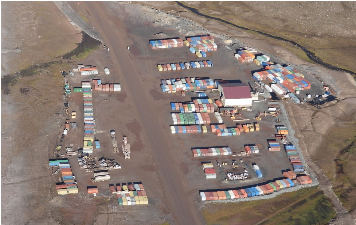
Photo 60. Incinerator Facility and Laydown – August
