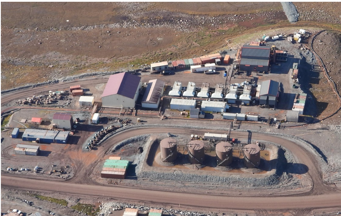
Photo 46. Bulk Fuel Storage Facility (MS-03) and Power Generation Facility – August
