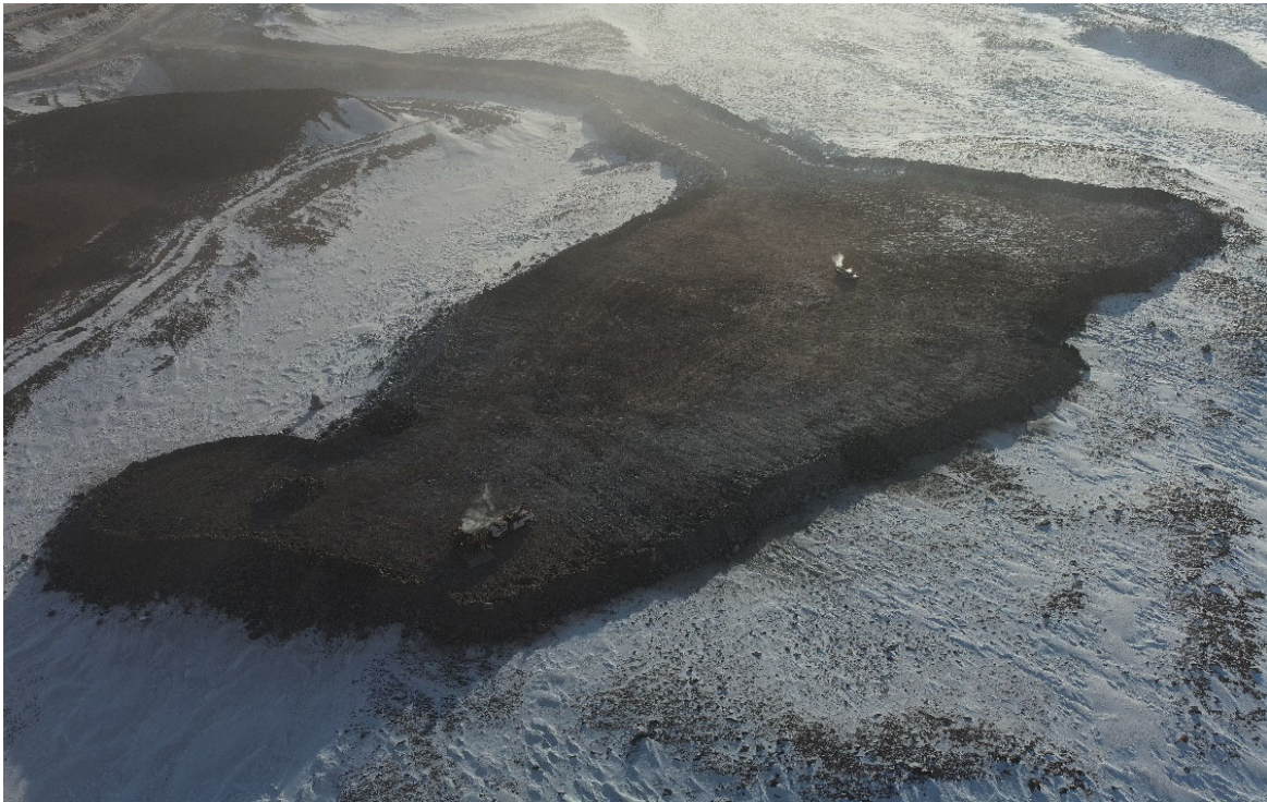
Photo 35. KM 105 Steensby Aggregate Pad Construction – April
