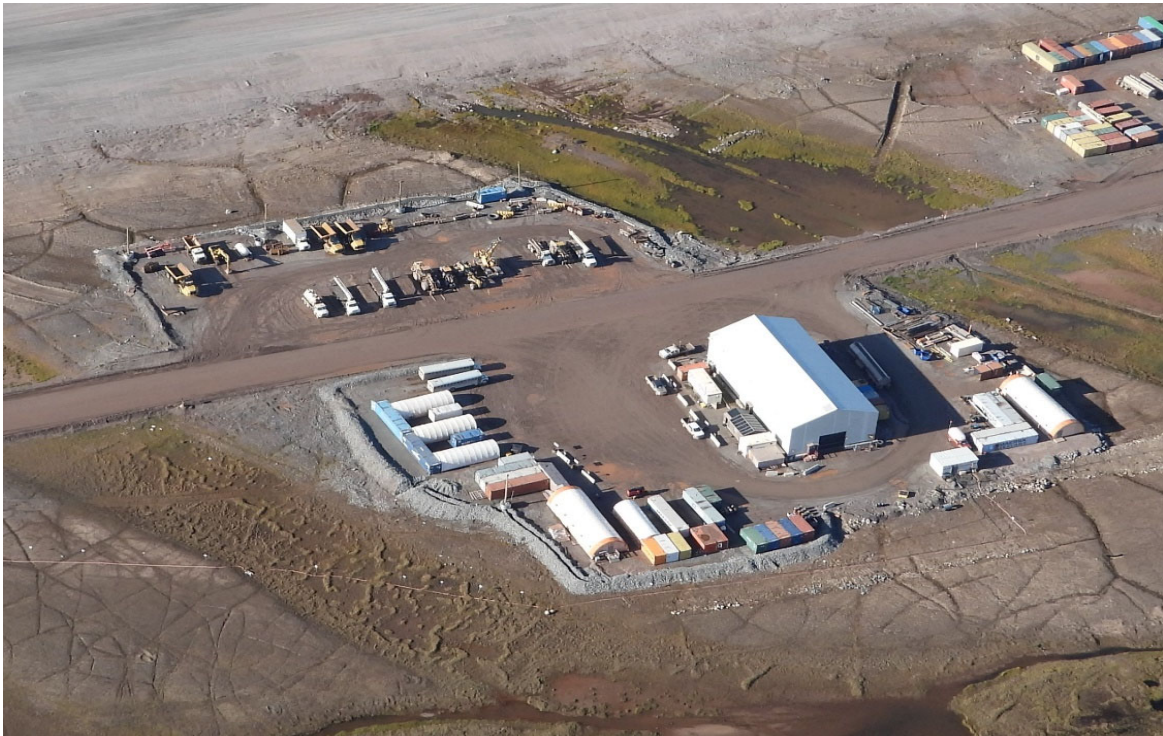
Photo 61. Site Services Building and Laydown – August
