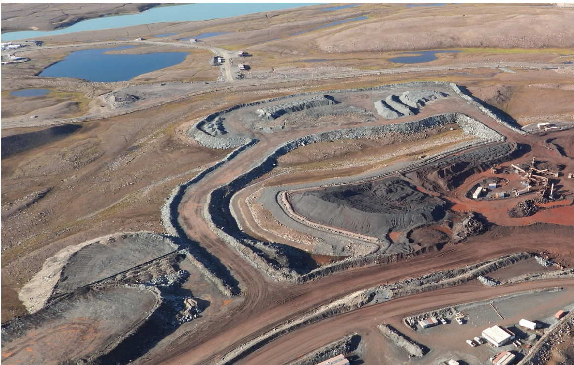
Photo 38. KM 105 Steensby Aggregate Pad – August
