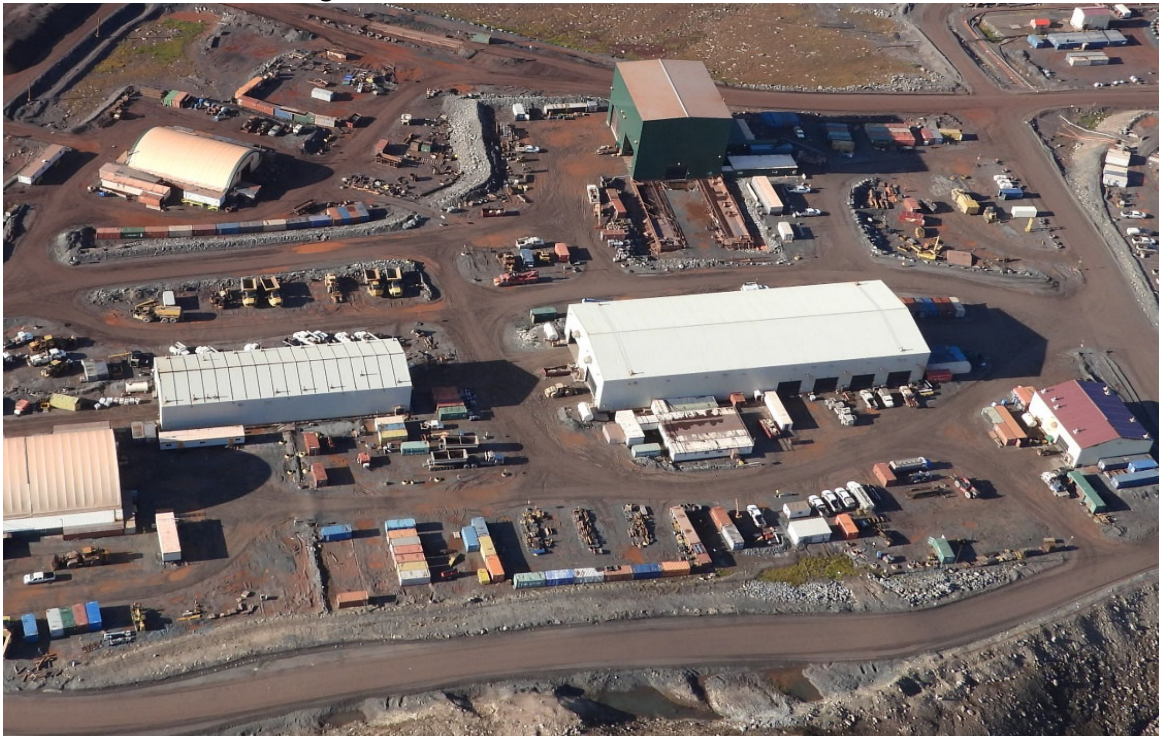
Photo 43. Mobile Maintenance Buildings - August
