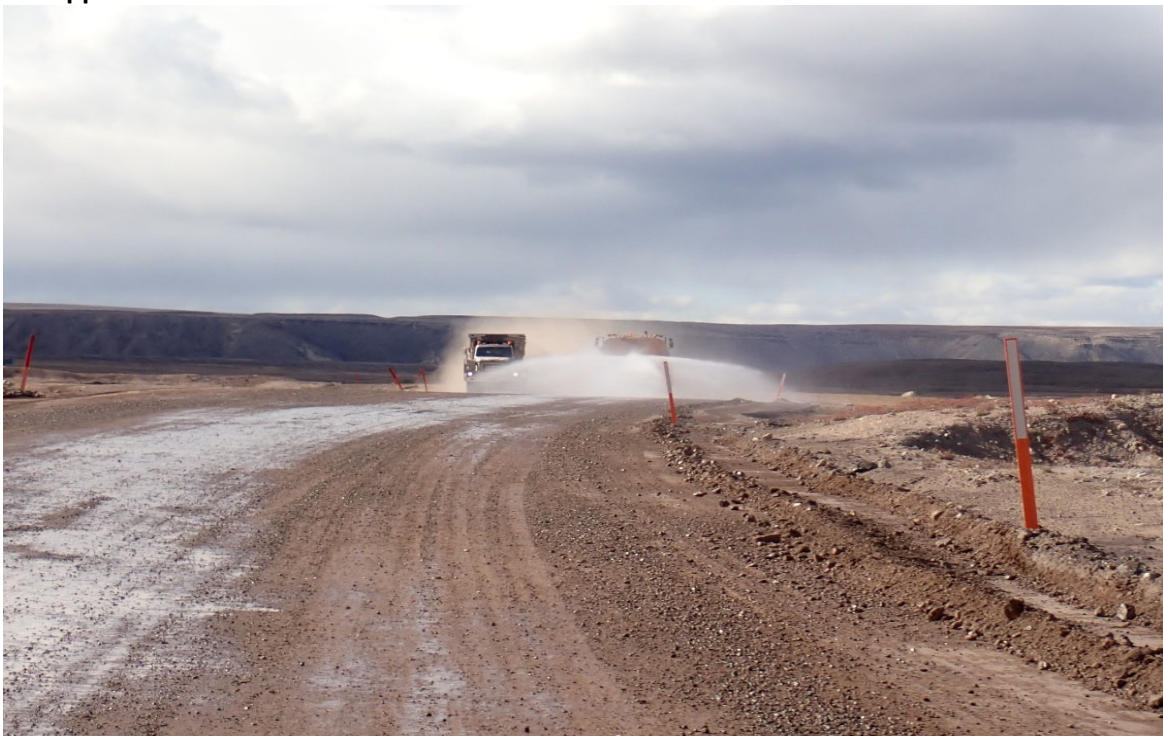
Photo 102. Applying Water to Site Roadways as Dust Suppression – August
