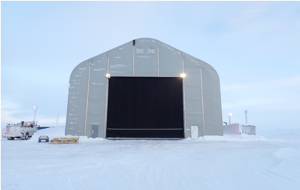
Photo 19. Maintenance Shop at KM 110 - November
