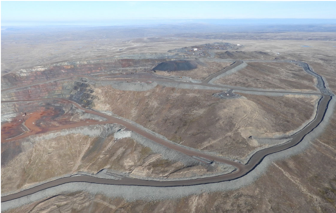
Photo 21. Mine Haul Road – July
