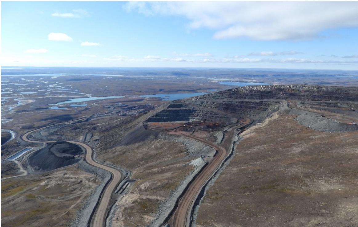
Photo 5. Deposit 1 and the Mine Haul Road - August
