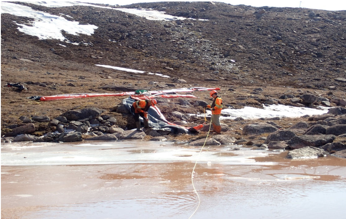
Photo 94. Silt Curtain Installation Downstream of MS-C-F – May
