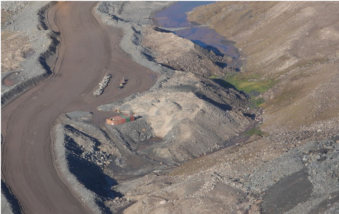
Photo 31. Water Treatment Plant Upstream of the KM 105 Surface Water Management Pond (MS-11) – August
