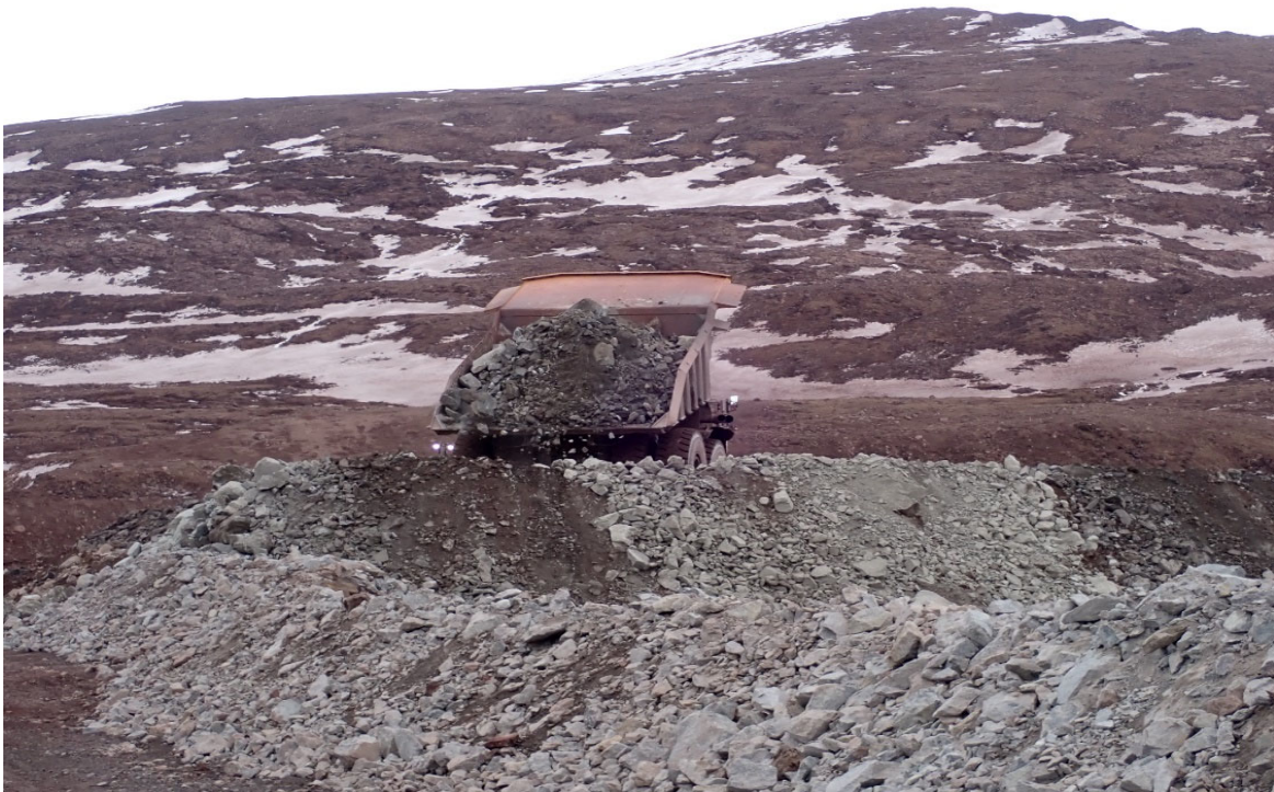
Photo 37. Road Expansion at the KM 105 Steensby Aggregate Pad – May
