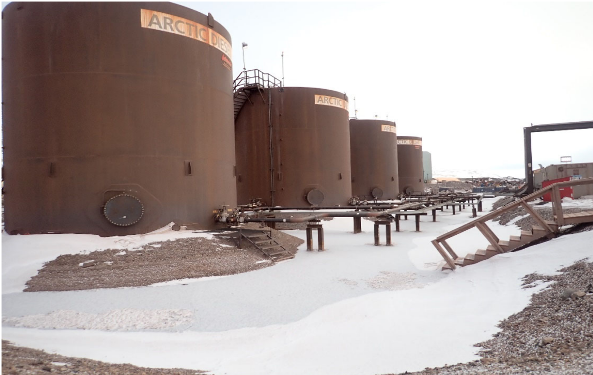
Photo 45. Mine Site Bulk Fuel Storage Facility (MS-03) for Vehicle and Equipment Re-fuelling - October
