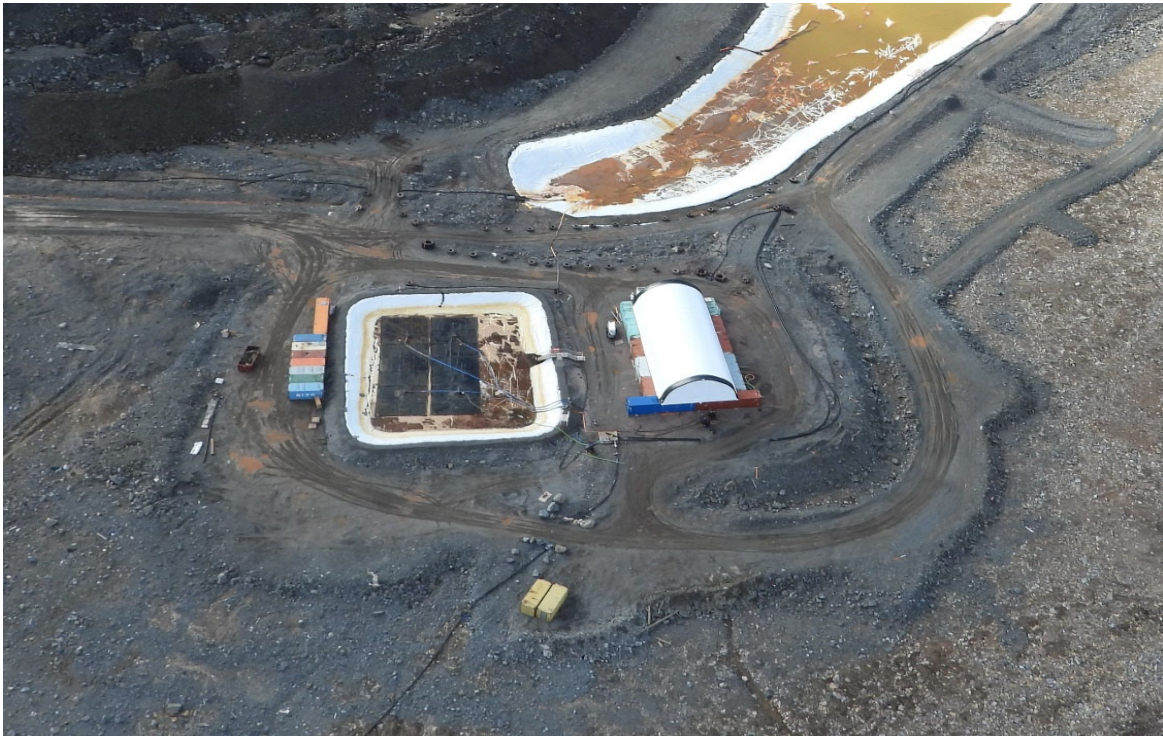
Photo 13. Geotube Pond at the Waste Rock Facility Water Treatment Plant – August
