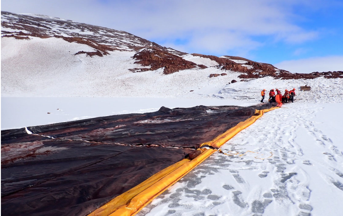
Photo 93. Silt Curtain Installation at MS-C-F – May
