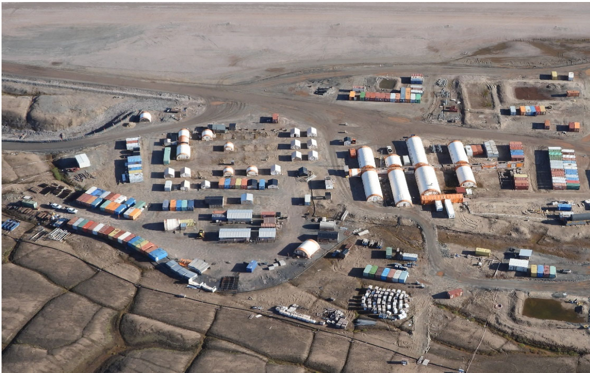
Photo 70. Weatherhaven Complex - August
