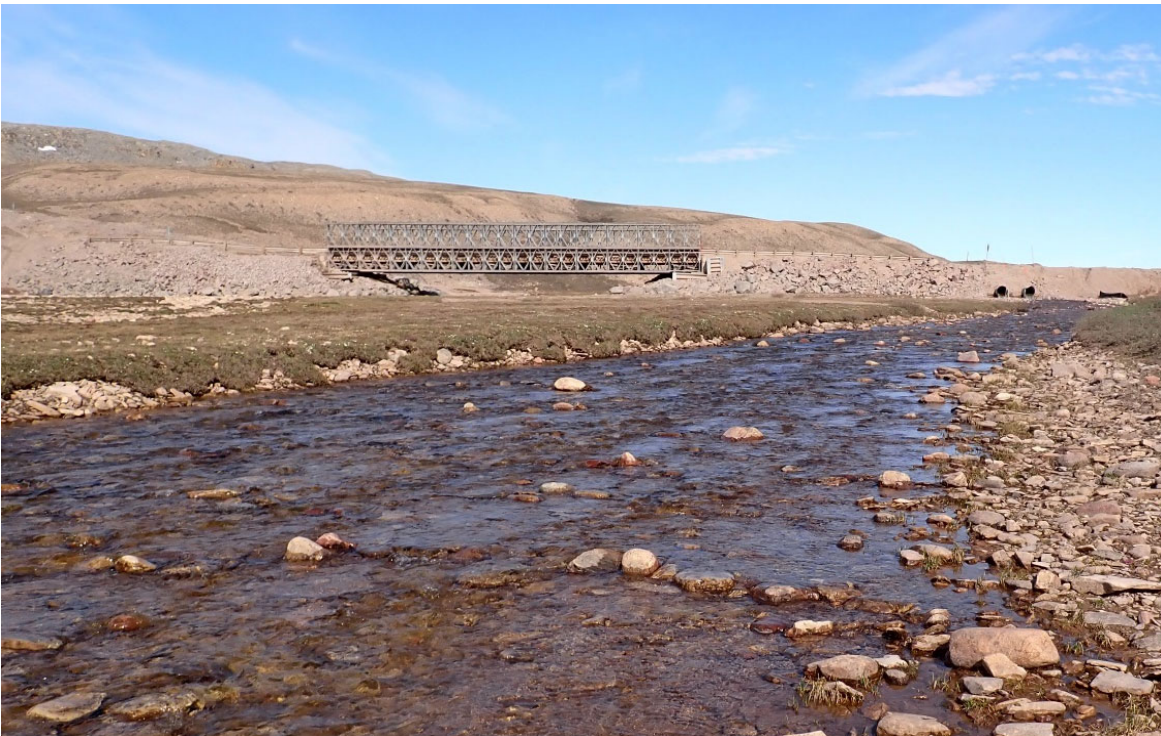
Photo 20. KM 63 Bridge, looking upstream - June
