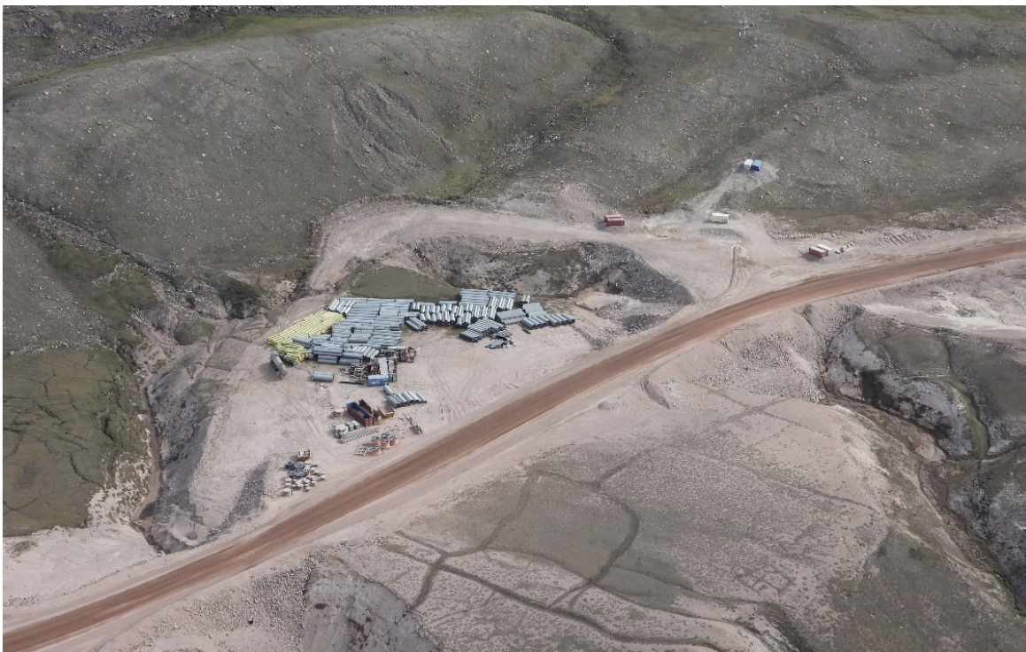
Photo 4. KM 7 R3 Laydown and Communications Tower – July
