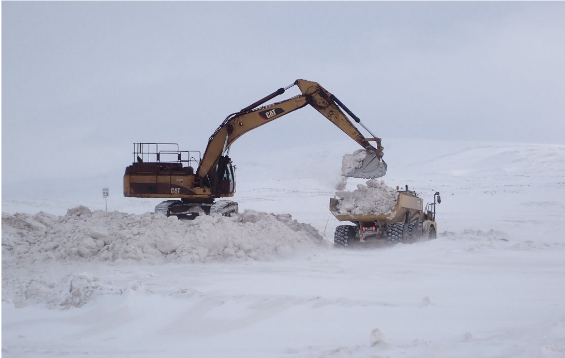
Photo 43. KM 17 Ice Bridge Removal - May
