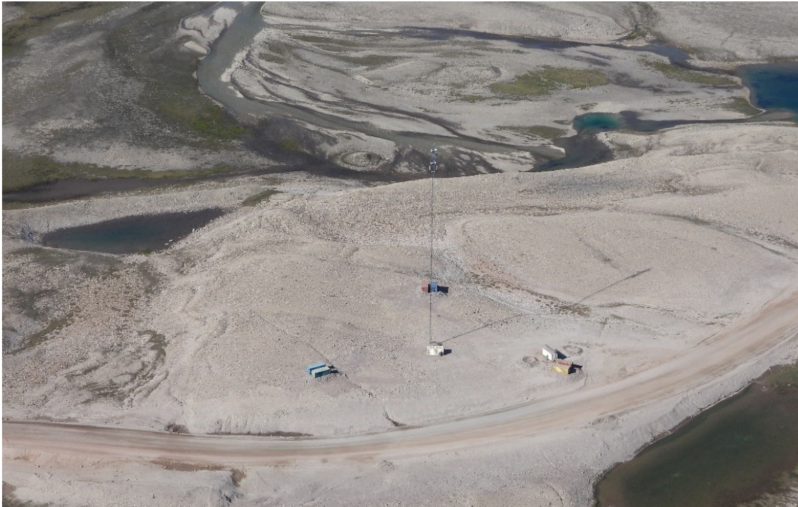
Photo 15. KM 49 Communications Tower – July
