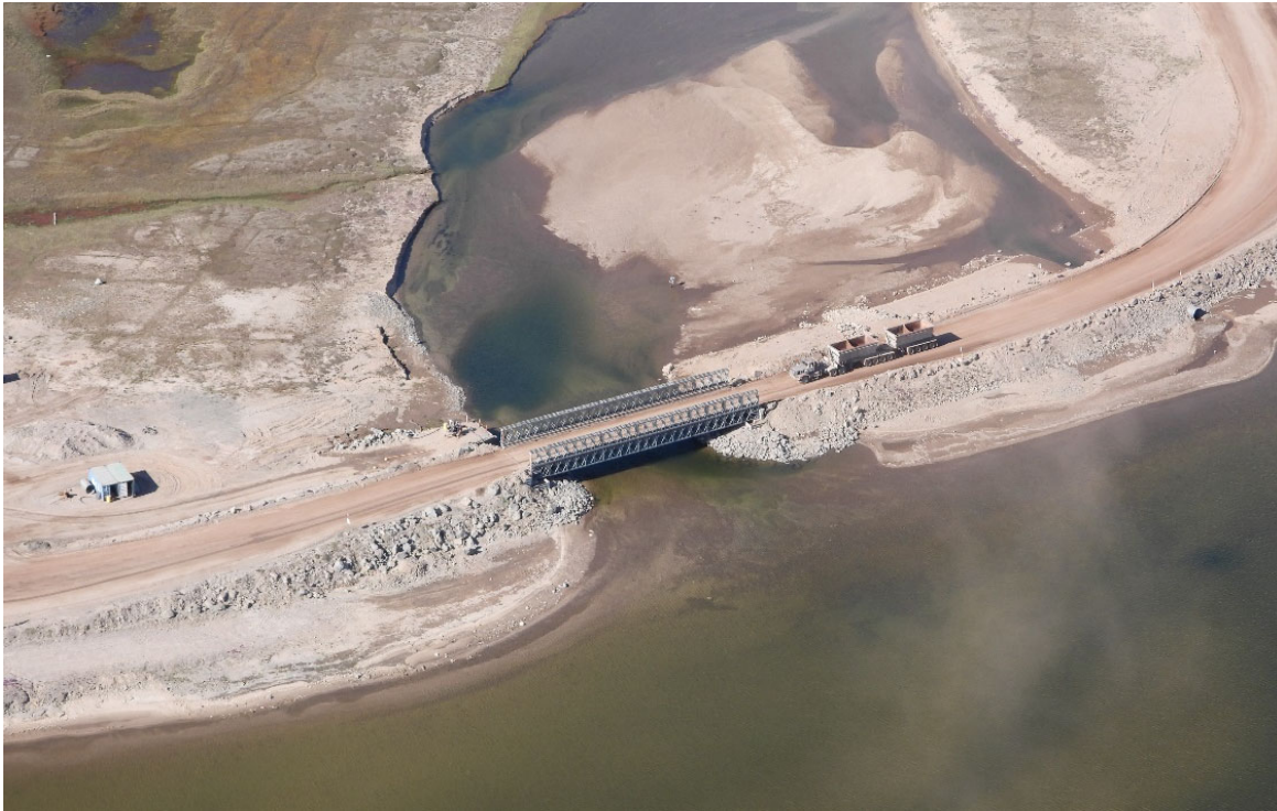
Photo 57. OHT crossing KM 80 Bridge - July
