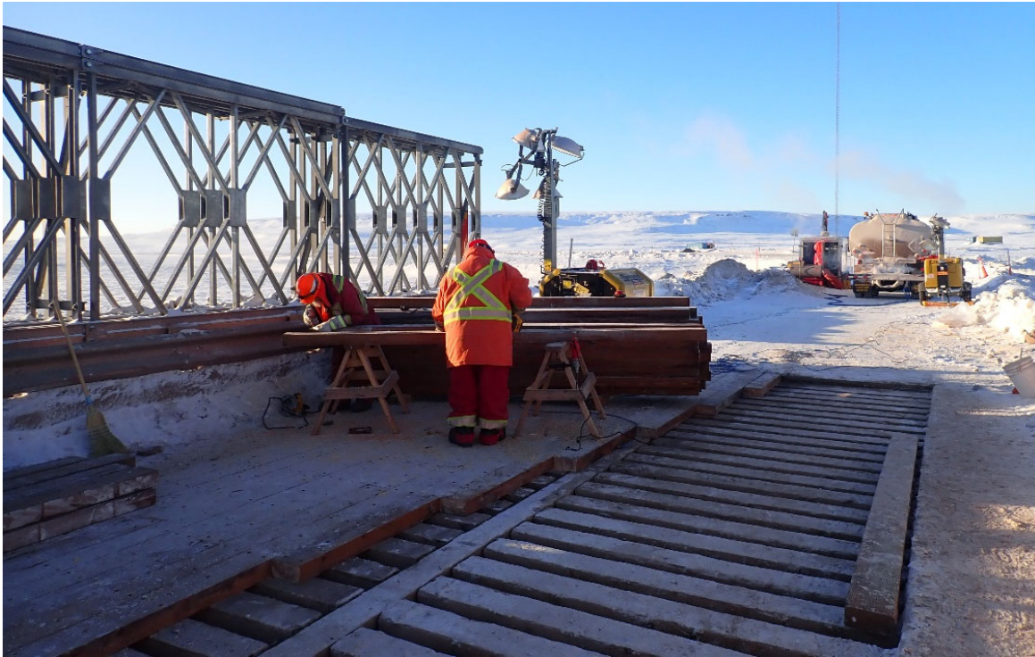
Photo 45. Redecking of KM 80 Bridge - March
