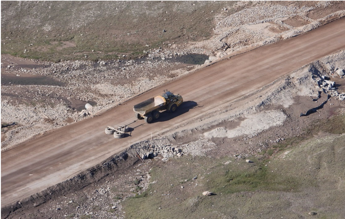
Photo 55. Tire Drag Working at KM 72.5 - July
