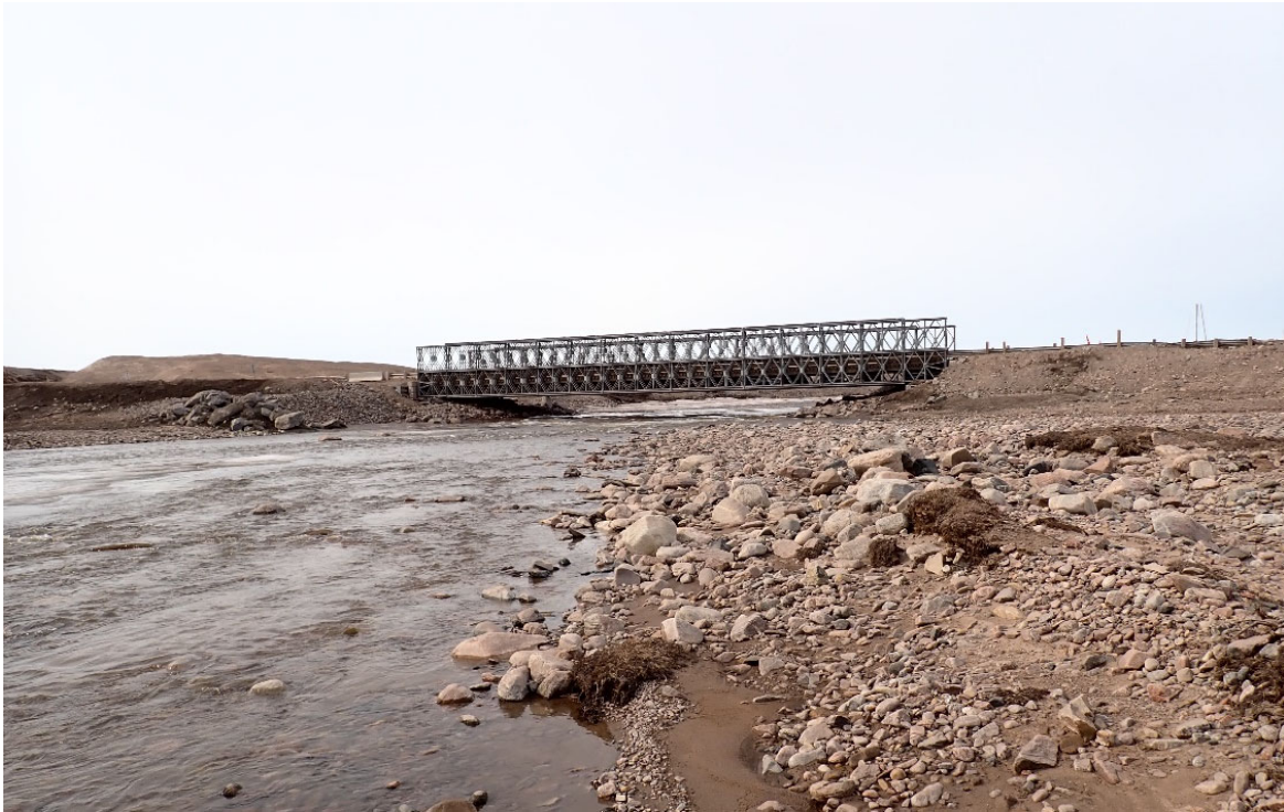
Photo 37. KM 97 Bridge looking upstream- June
