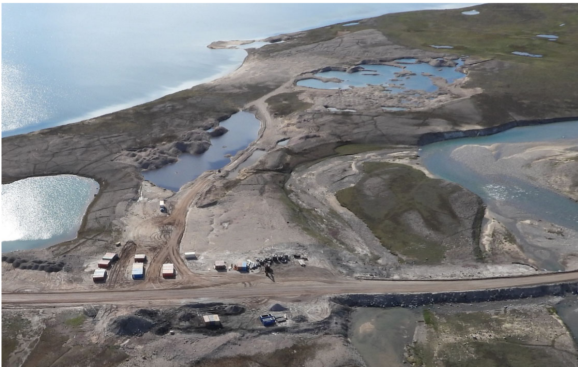
Photo 40. KM 97 Borrow Pit West for Dust Suppression Mixing - July
