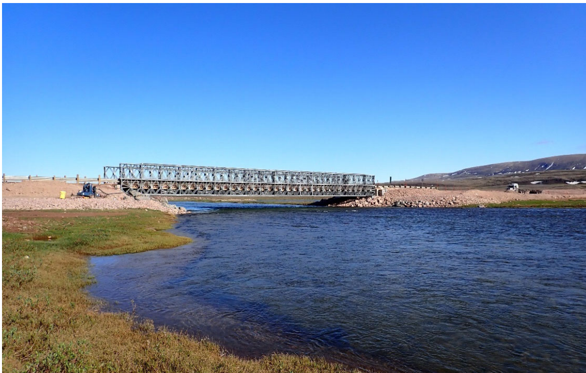
Photo 5. KM 17 Bridge looking upstream- June
