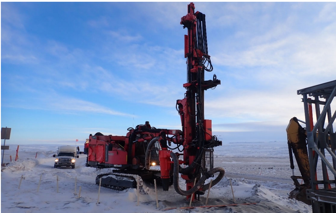
Photo 60. Drilling KM 97 Bridge Abutments for Replacement - February
