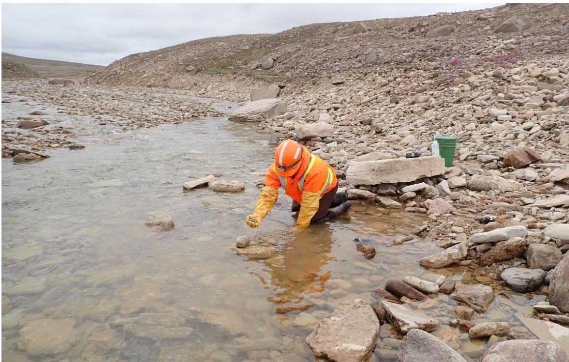
Photo 66. Installation of In-flow Sediment Traps at KM 38 (CV-099) - July
