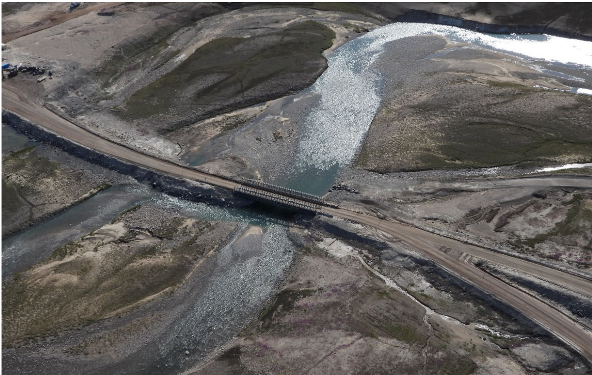
Photo 38. KM 97 Bridge - July
