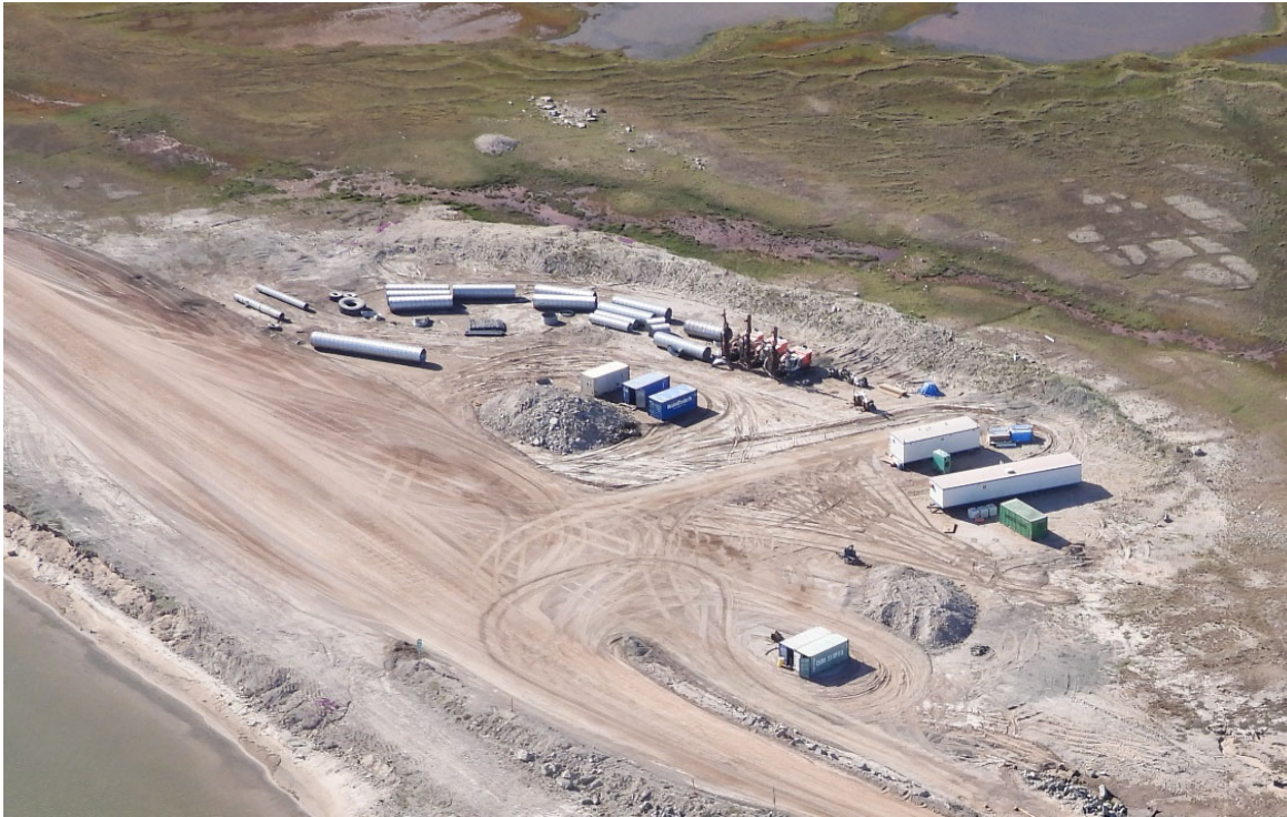
Photo 31. KM 80 Laydown – July
