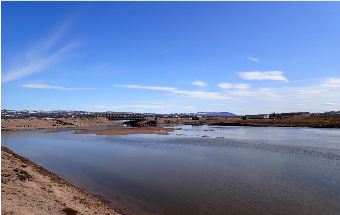
Photo 29. KM 80 Bridge looking downstream - June
