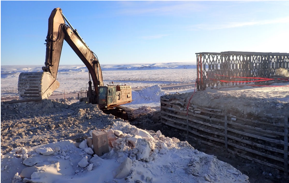
Photo 49. Removal of Southern Abutment of KM 97 Bridge – March
