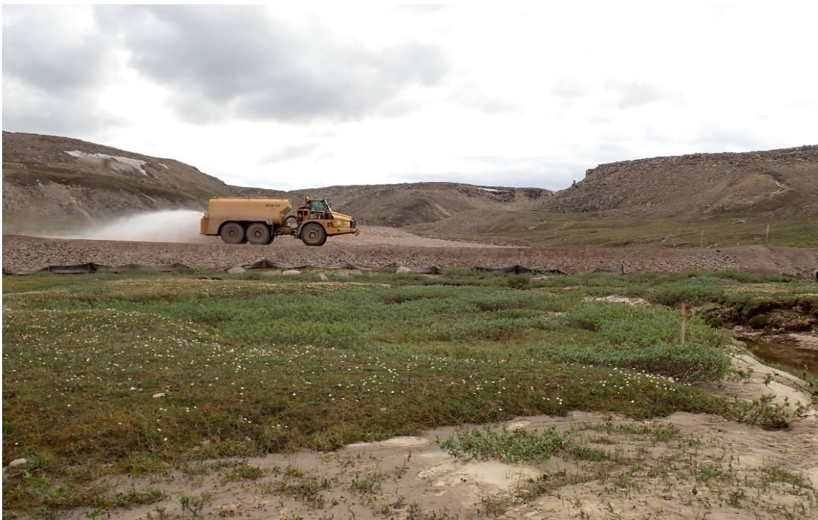
Photo 58. Water Buffalo Applying Dust Suppressant at KM 88 - July
