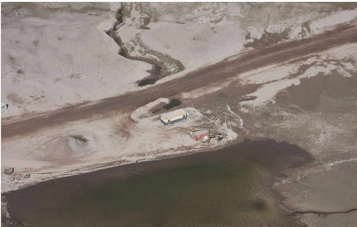
Photo 12. KM 33 Laydown – July
