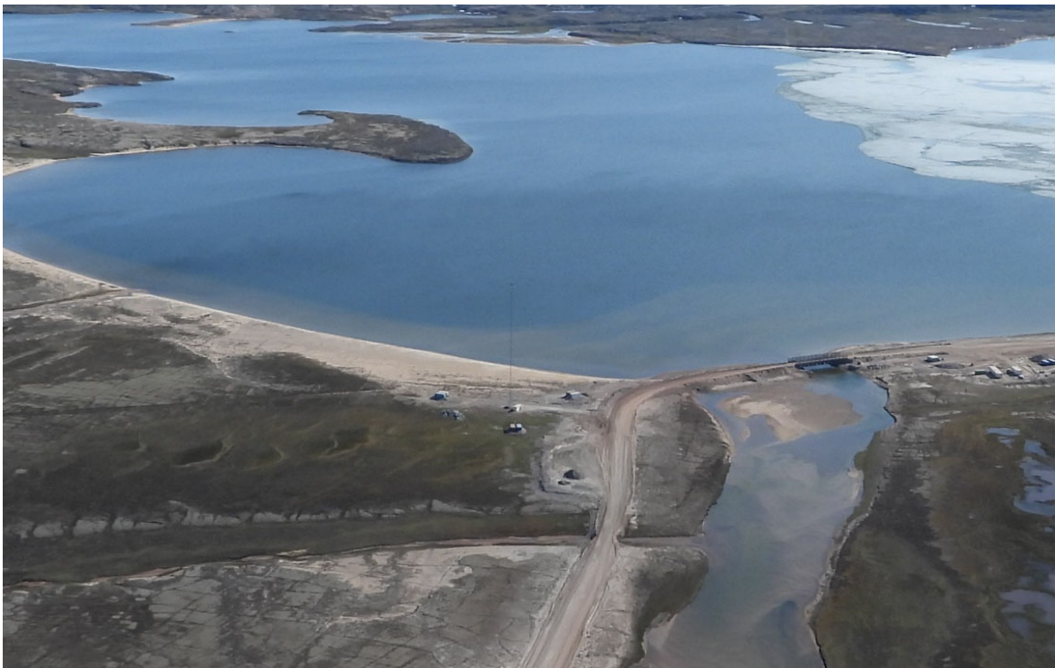
Photo 28. KM 80 Communications Tower – July
