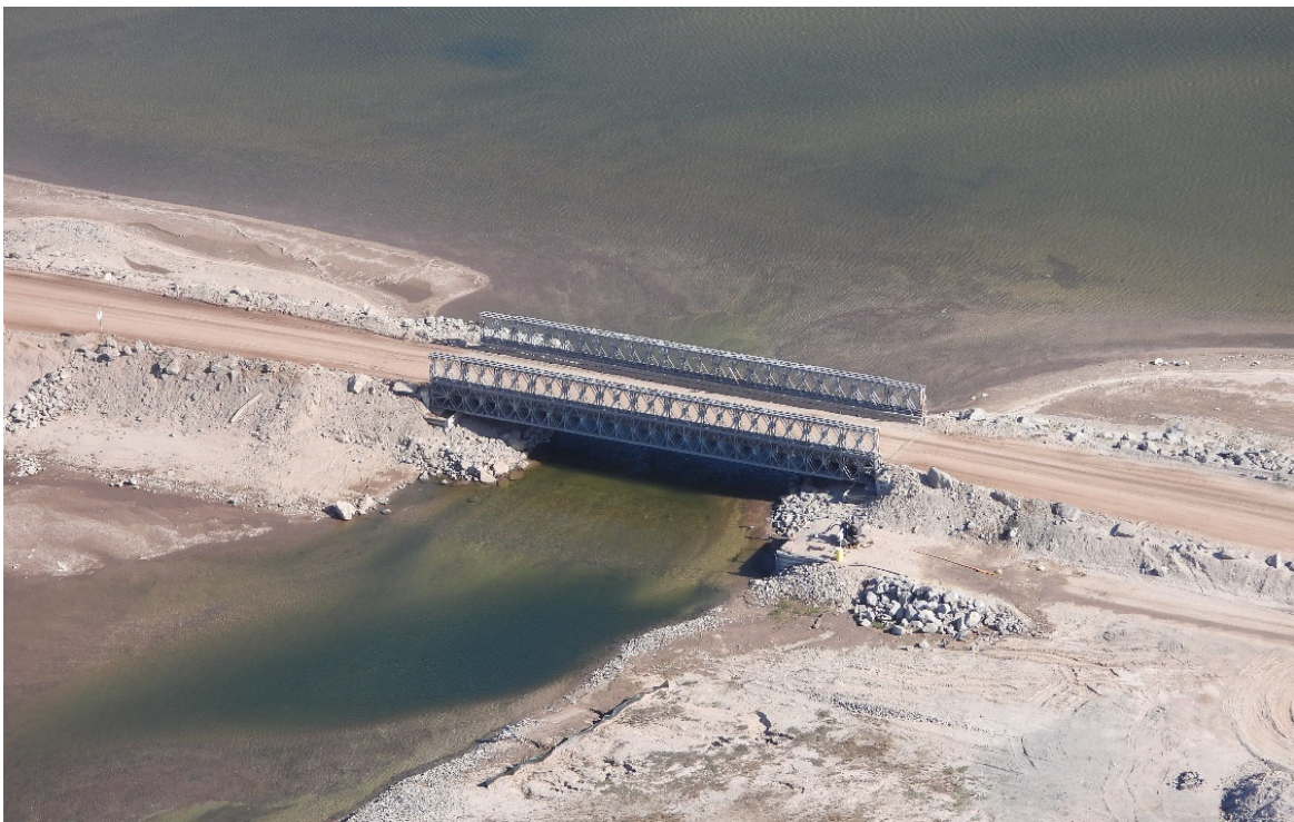
Photo 30. KM 80 Bridge – July
