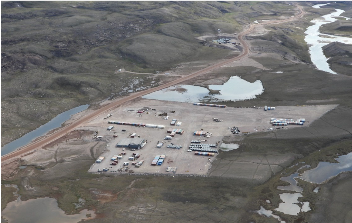
Photo 3. KM 6.5 L2 Laydown – June
