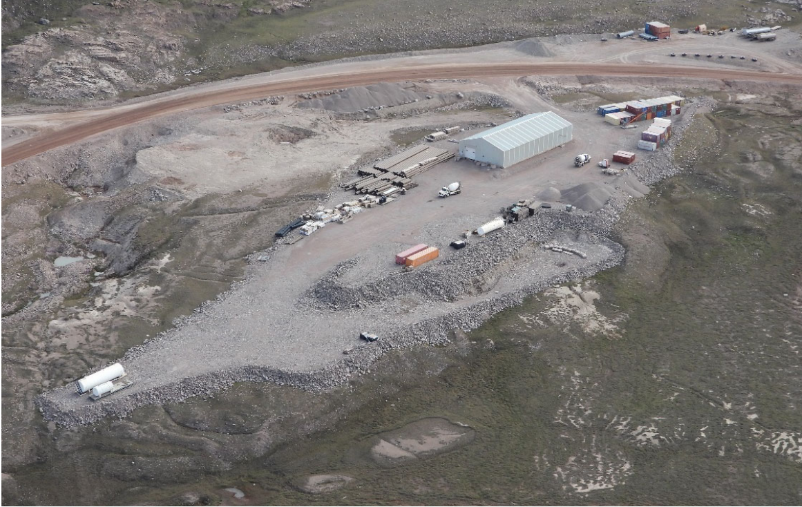
Photo 1. KM 4 R1 Laydown – July
