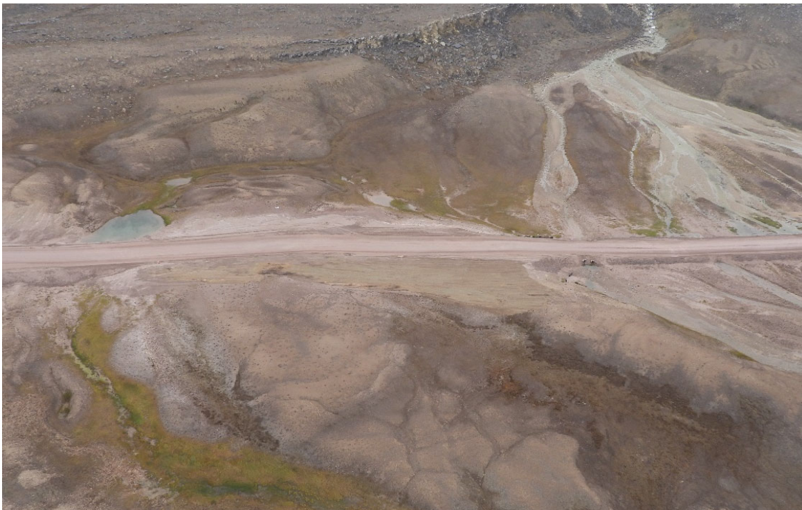
Photo 16. KM 50 Borrow Pit Remediation - August
