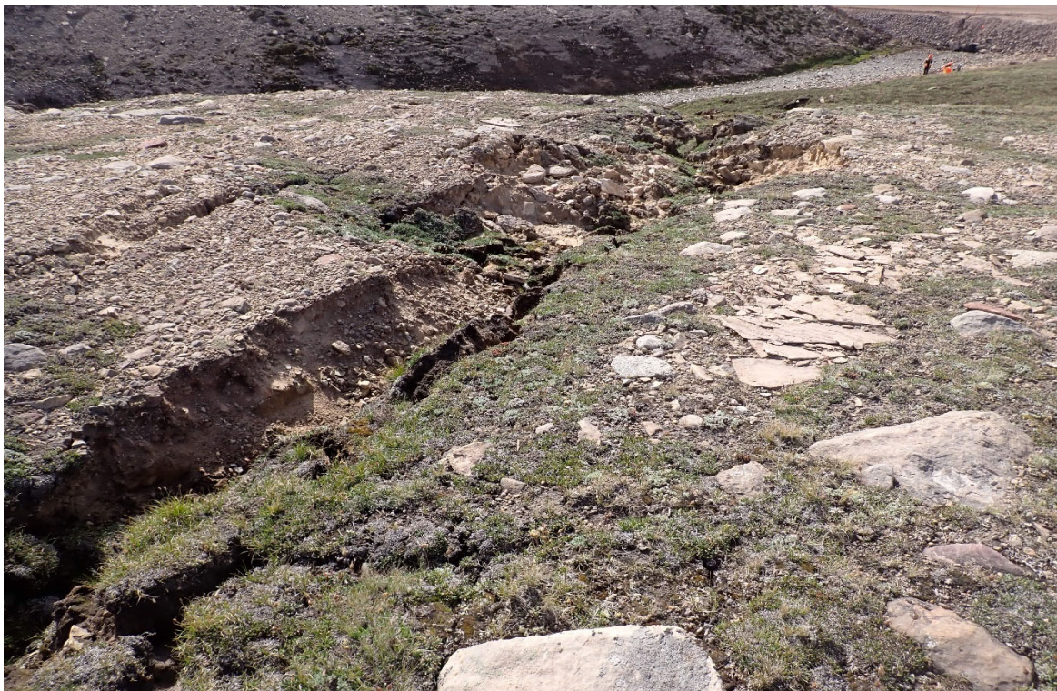
Photo 72. Erosion gully and ground slumping upstream of CV-111 (KM 32) - August
