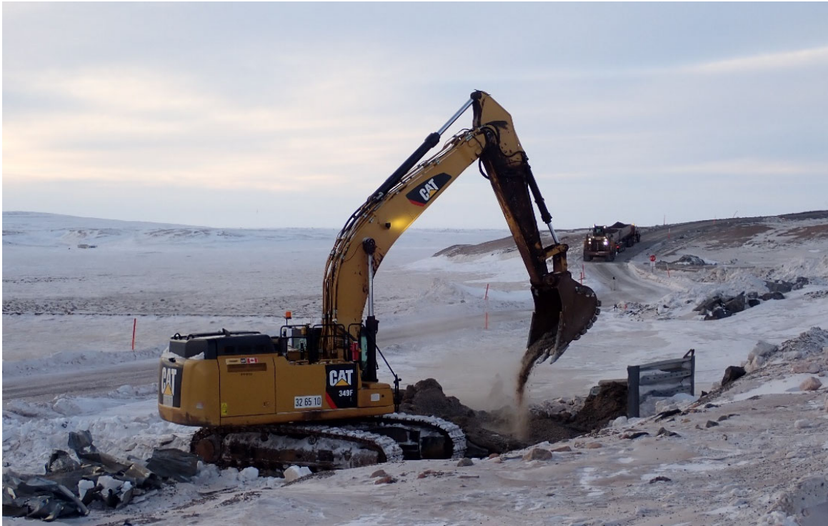
Photo 61. Excavator Removing KM 97 Bridge Abutment - February
