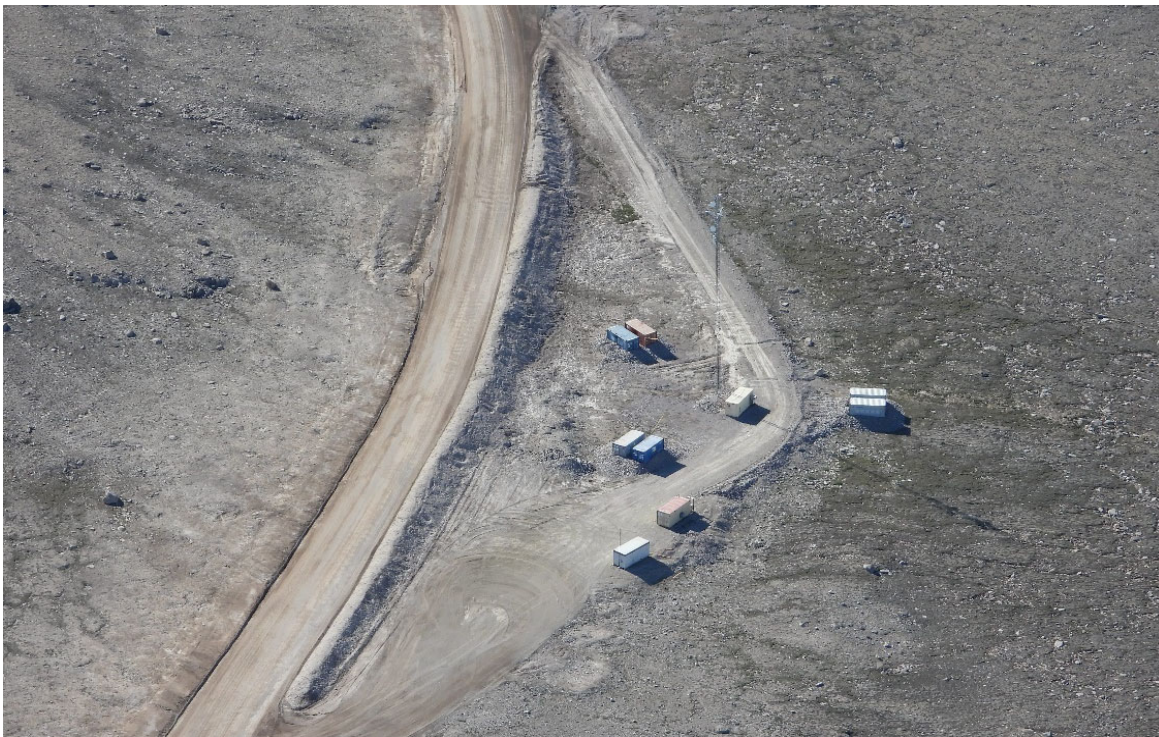
Photo 14. KM 40 Communications Tower – July
