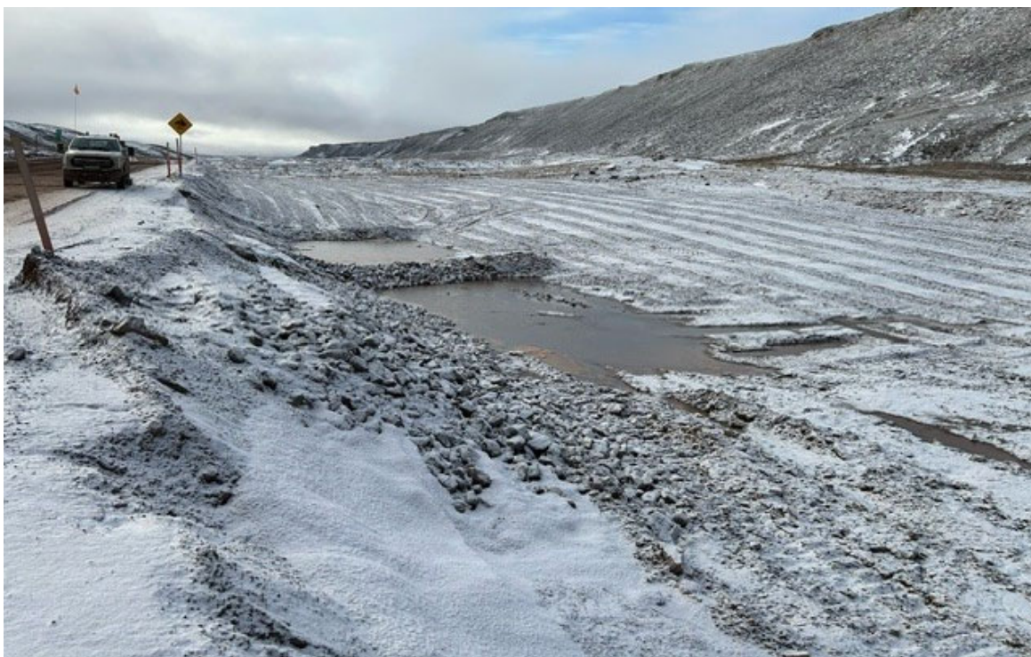
Photo 48. Borrow Pit 14A Remediation at KM 89 - September
