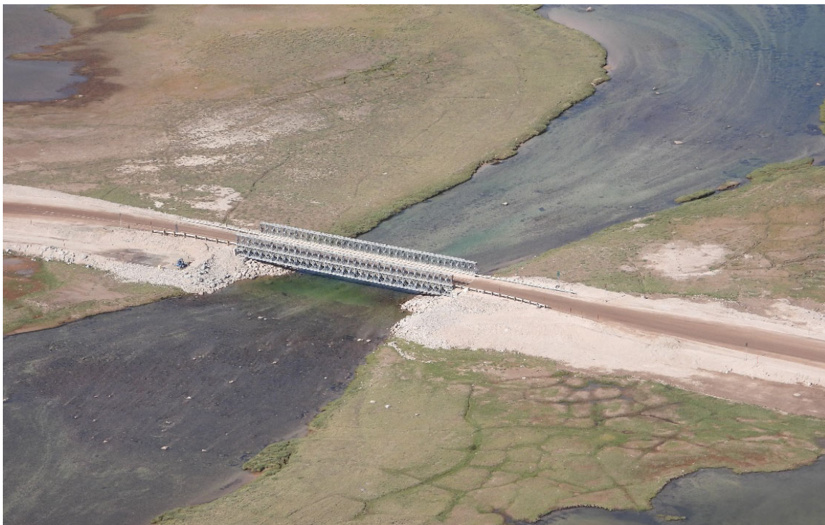
Photo 6. KM 17 Bridge – July
