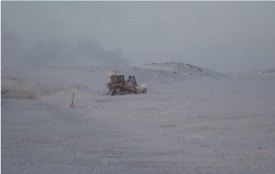
Photo 59. Dozer Feathering Snowbanks into Tundra at KM 95 - February
