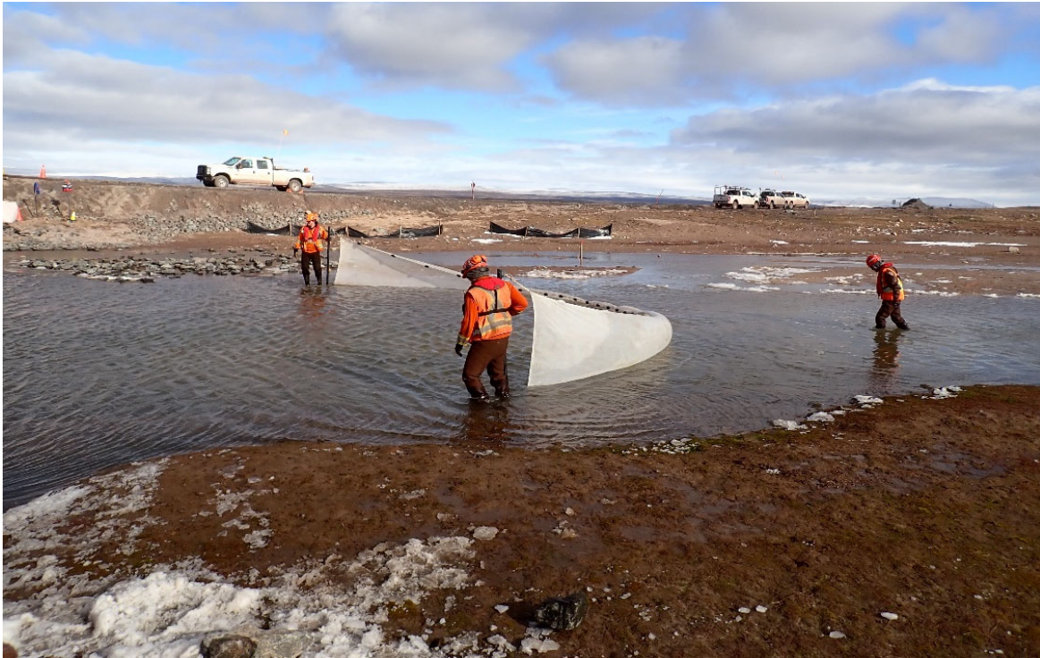
Photo 69. Pre-construction Fish Salvage at KM 81 (CV-216) - August
