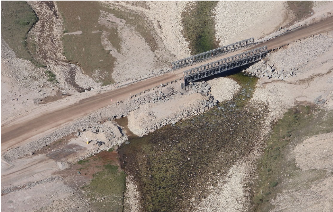
Photo 21. KM 63 Bridge – July
