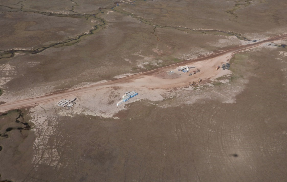
Photo 19. KM 60 Laydown – July
