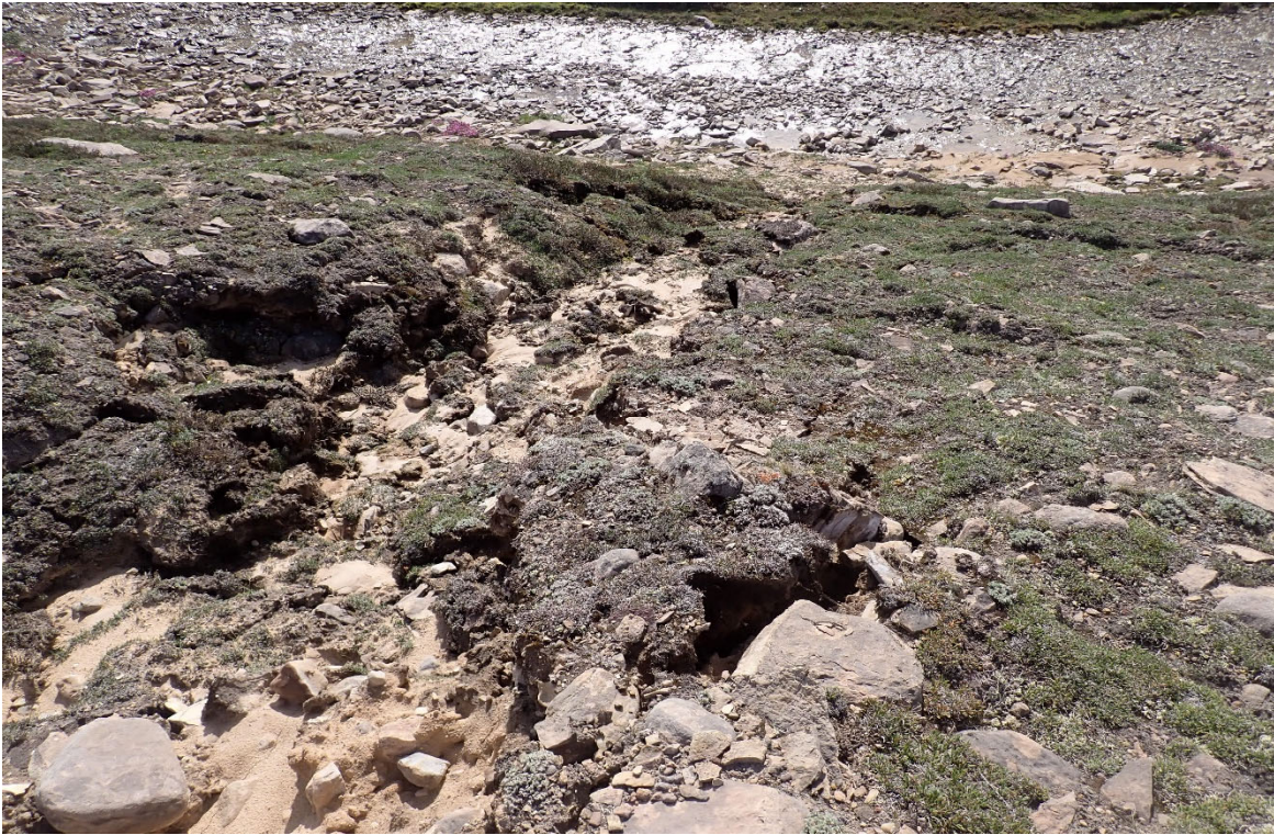
Photo 73. Erosion gully and sediment deposition into watercourse, upstream of CV-111 (KM 32) - August
