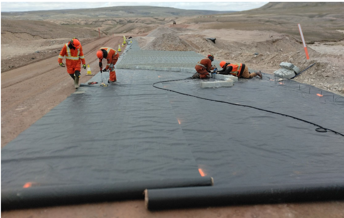
Photo 44. Installation of Geo Cell at KM 64 – July
