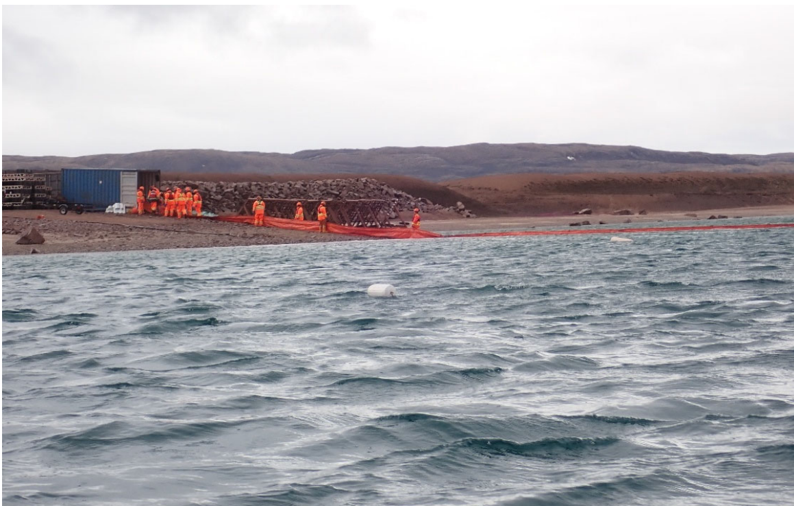
Photo 24. Oil Pollution Emergency Plan (OPEP) Boom Deployment – July
