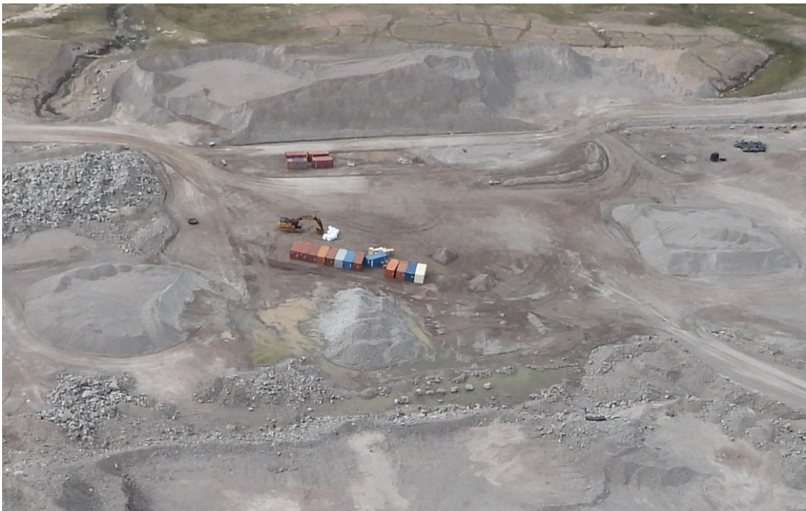
Photo 16. Quarry (Q1) Stockpile and Facilities – July
