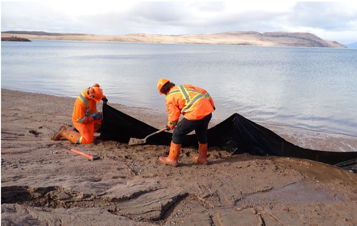
Photo 40. Silt Fence Installation at Bulk Fuel Manifold – July
