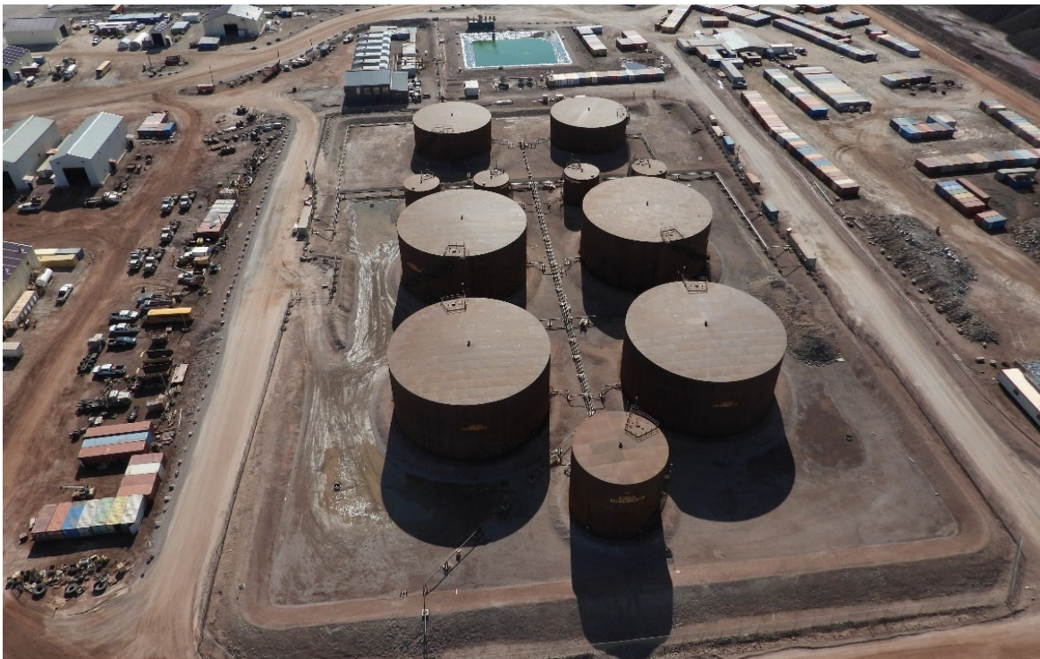
Photo 10. Bulk Fuel Storage Facility (MP-03) - August
