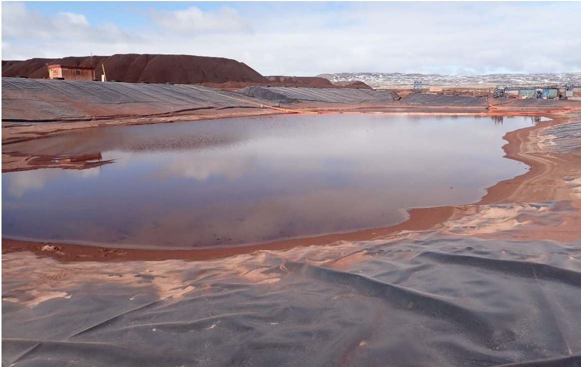
Photo 7. Surface Water Management Pond (MP-05), East Ore Stockpile Pad – June
