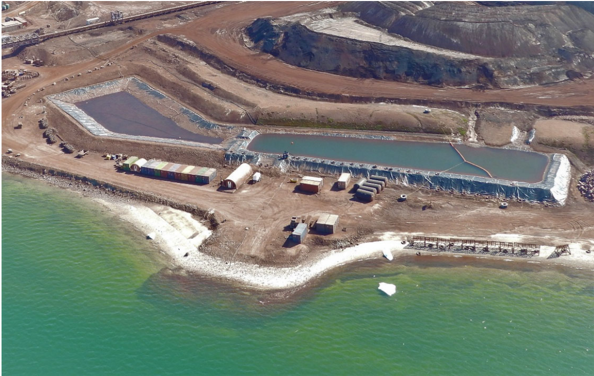
Photo 3. Surface Water Management Pond (MP-06), West Ore Stockpile Pad – July
