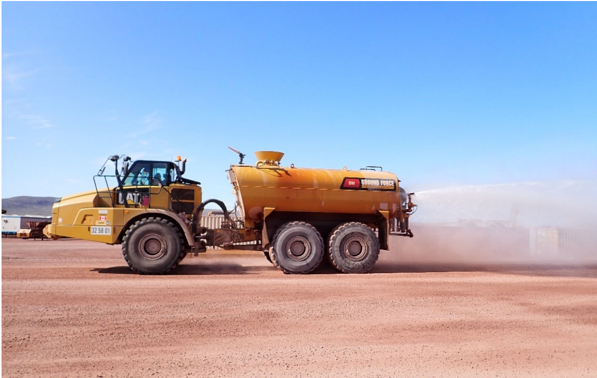
Photo 23. 740 Water Truck Applying Water as Dust Suppressant at Milne Port – June
