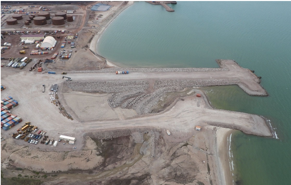
Photo 11. Freight Dock and Sealift Ramp – July
