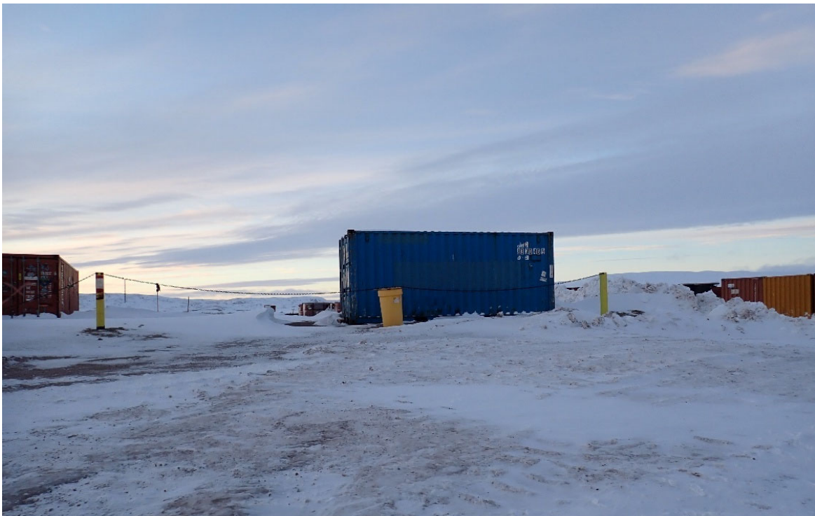
Photo 14. Hazardous Water Berms 3 & 4 Entrance (chained) - November
