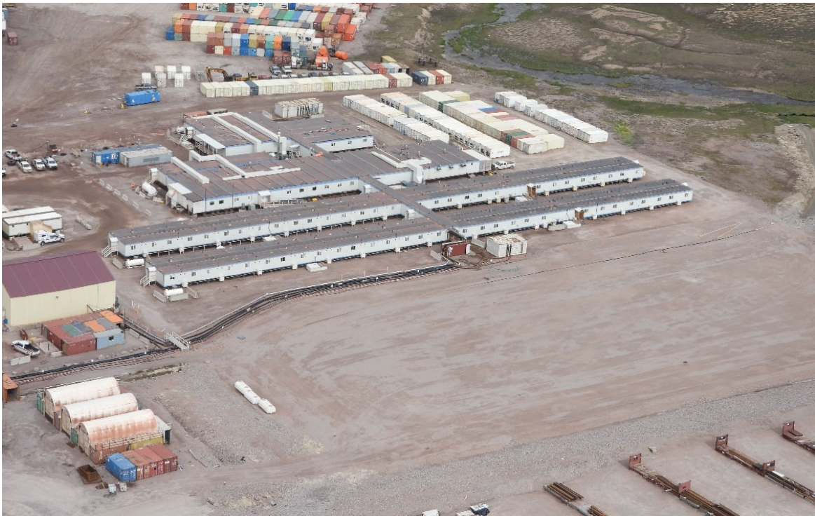
Photo 18. Milne Port Accommodation, Port Site Complex – July
