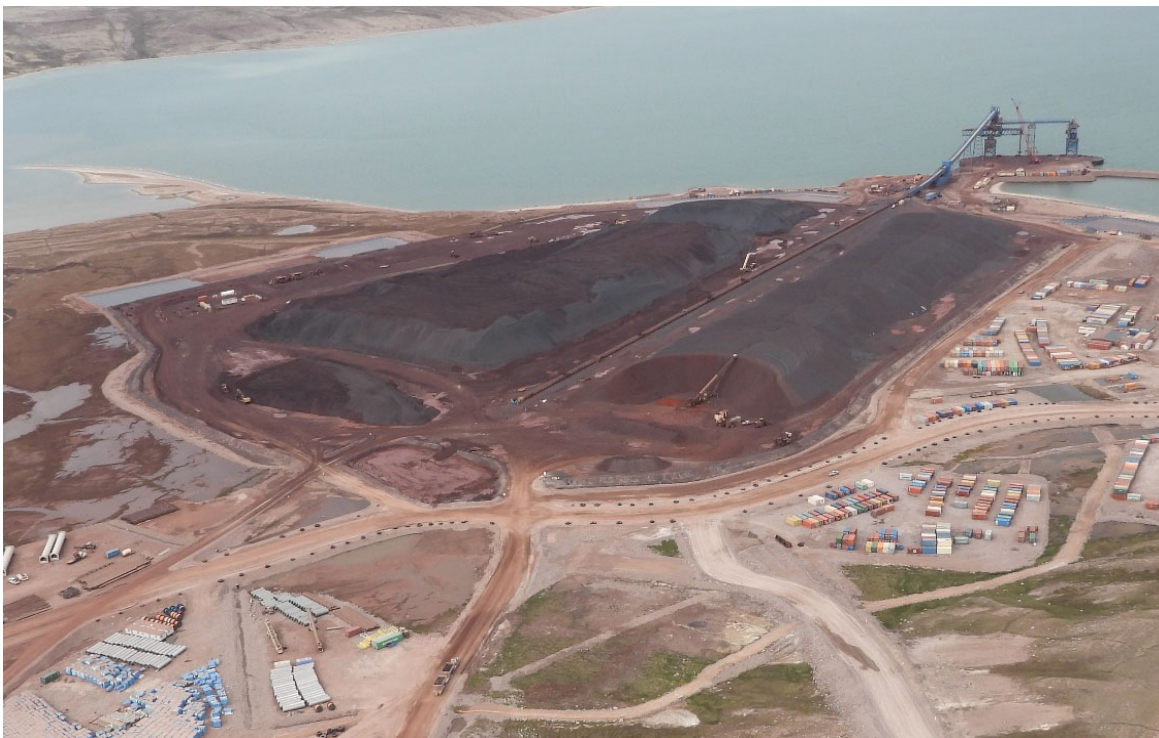
Photo 2. Milne Port Ore Stockpile Pad and Facility Infrastructure - July
