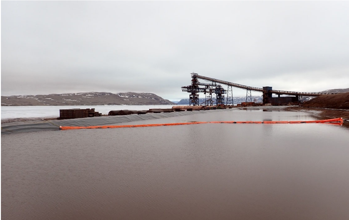
Photo 43. Silt Curtain Installation in Surface Water Management Pond (MP-06) – June
