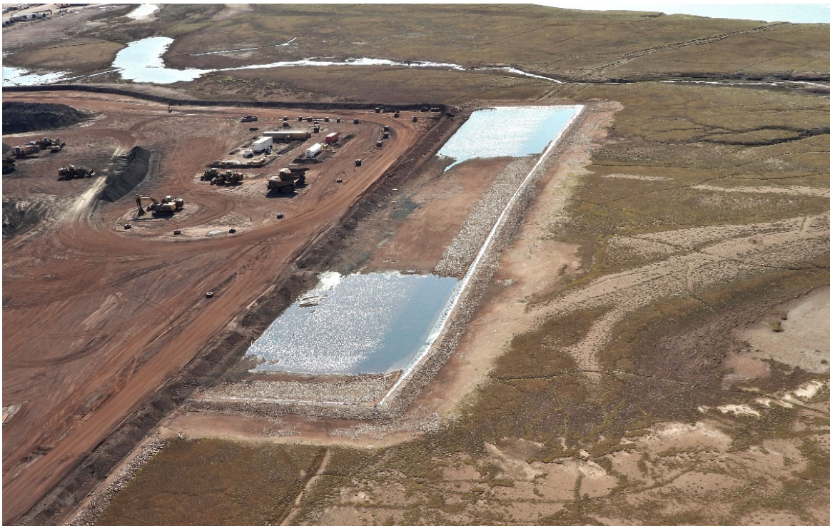
Photo 8. Surface Water Settling Pond (Pond-3), West Ore Stockpile Pad – September
