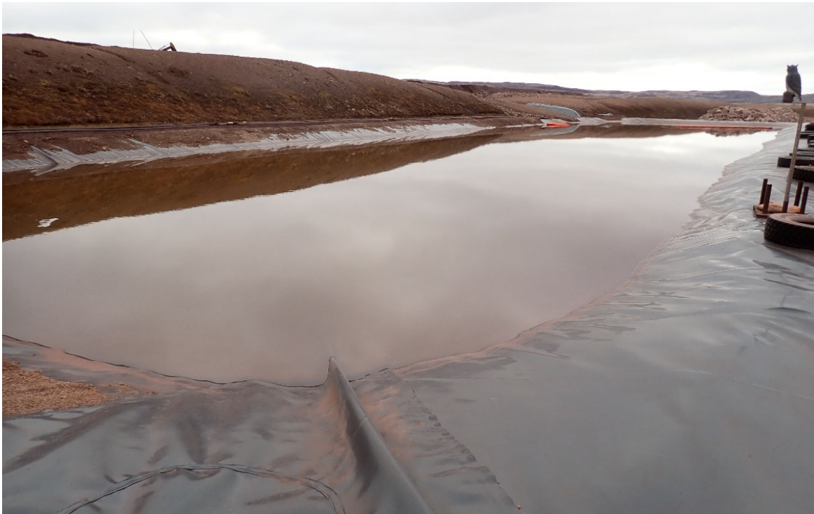
Photo 4. Surface Water Management Pond (MP-06), Northwest Cell of Ore Stockpile Pad - September
