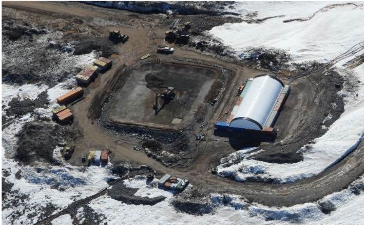
Photo 1. Geotube® Replacement at the Waste Rock Facility Water Treatment Plant - June
