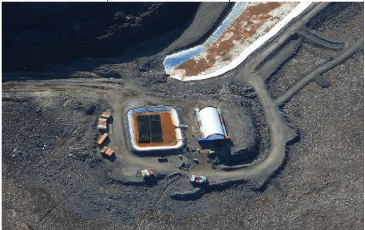
Photo 2. Geotube® Replacement Completed at the Waste Rock Facility Water Treatment Plant - August
