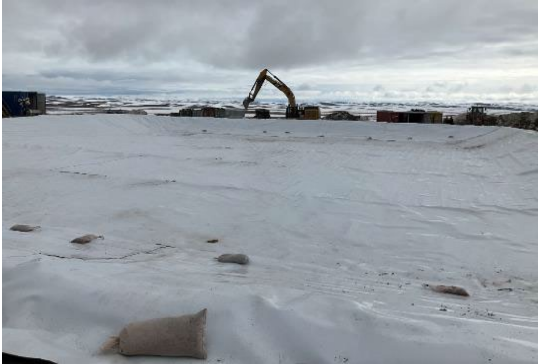
Photo 7. Liner Installation Nearly Complete - June 30
