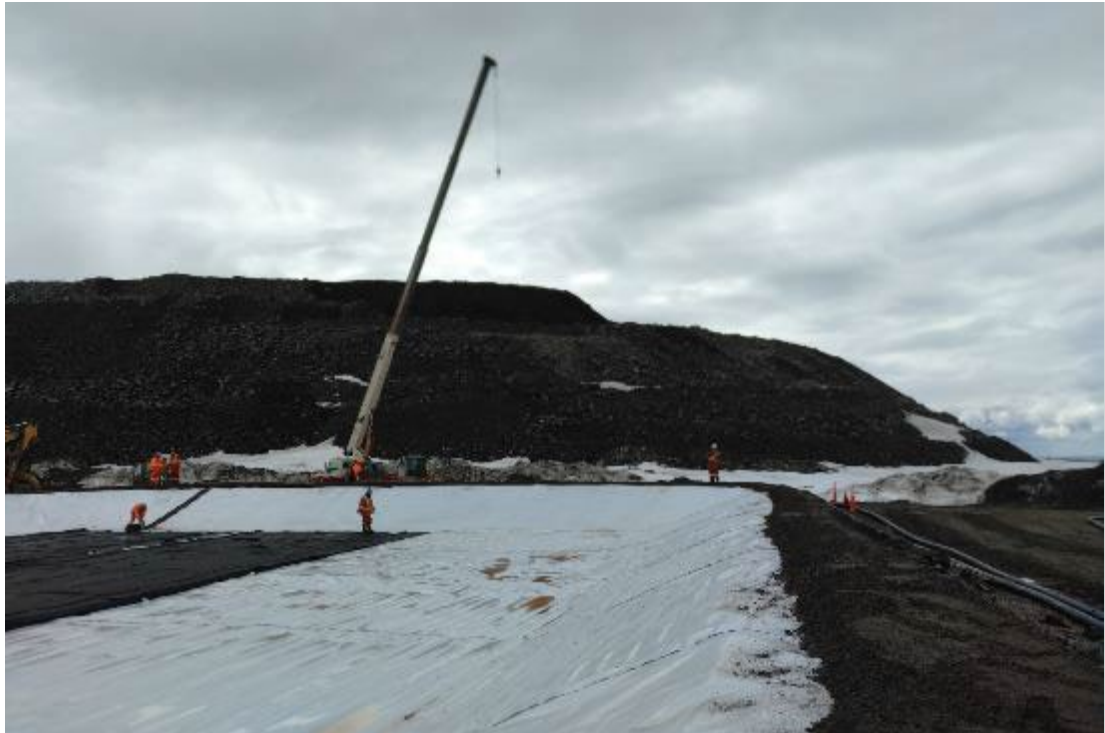
Photo 8. Liner tie-in complete and Geotube® installed – June 30
