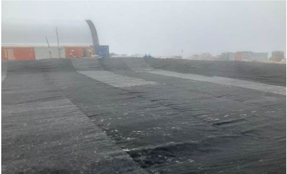
Photo 5. Subgrade covered by non-woven Geotextile Cloth – June 28
