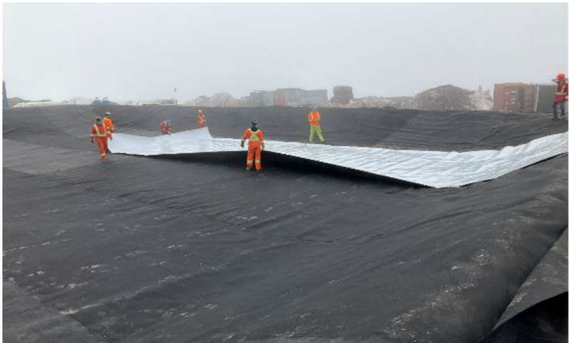
Photo 6. Liner installation begins – June 28
