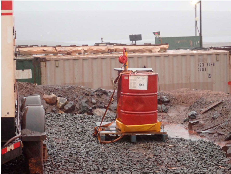
Photo 3. Drums placed within secondary containment – September 23, 2025
