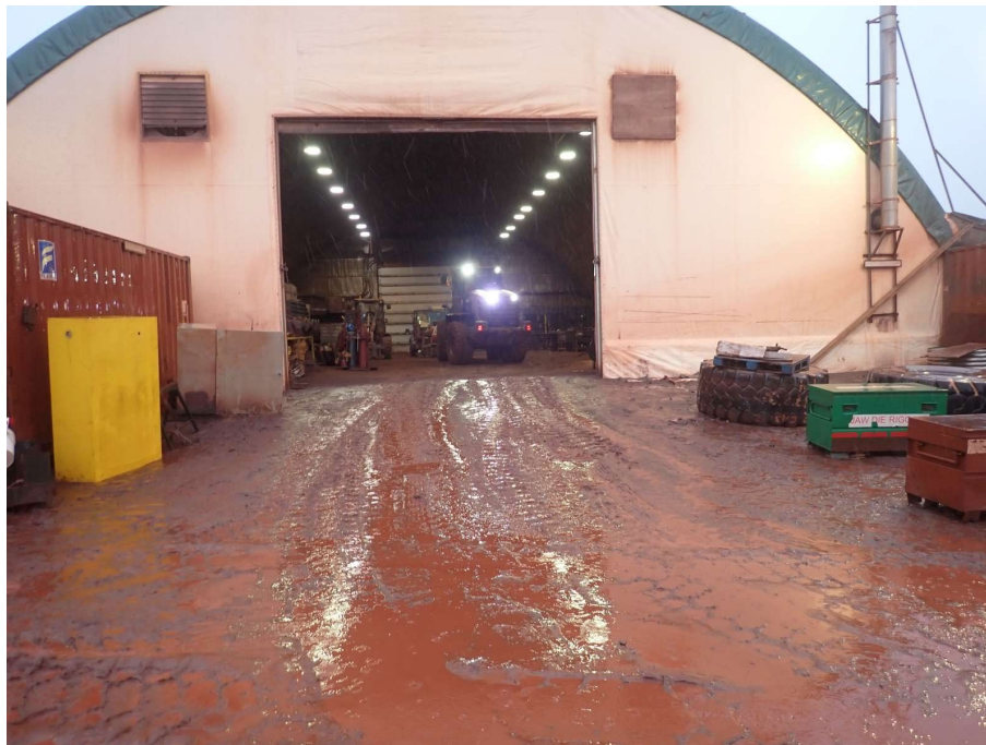
Photo 2. Materials removed from in front of Crusher Shop – September 23, 2025
