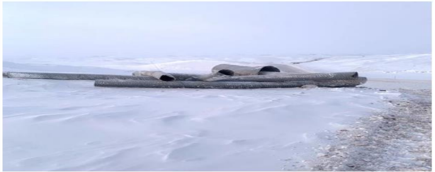
Photo 5. KM 63.5, Culverts retrieved from watercourse, staged next to Tote Road for pick-up and final disposal, 2024-11-28
