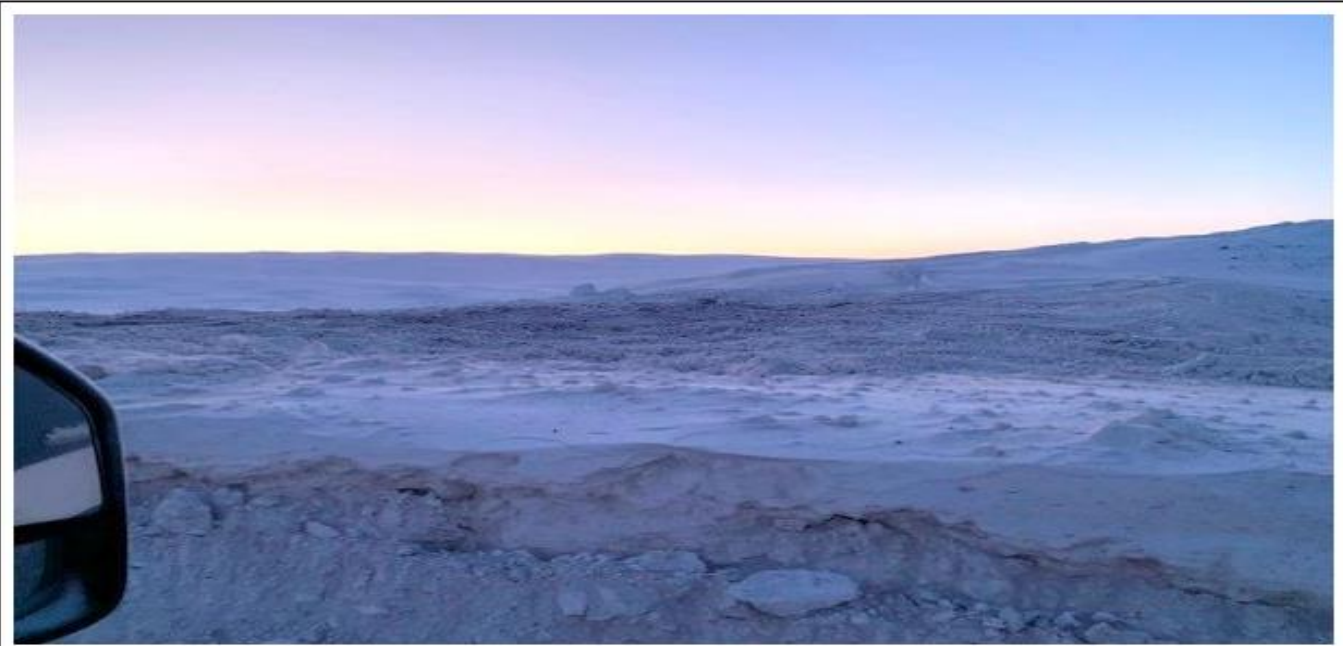
Photo 7. KM 63.5, Culvert staging area empty, after transporting culvert debris for disposal, 2024-11-29
