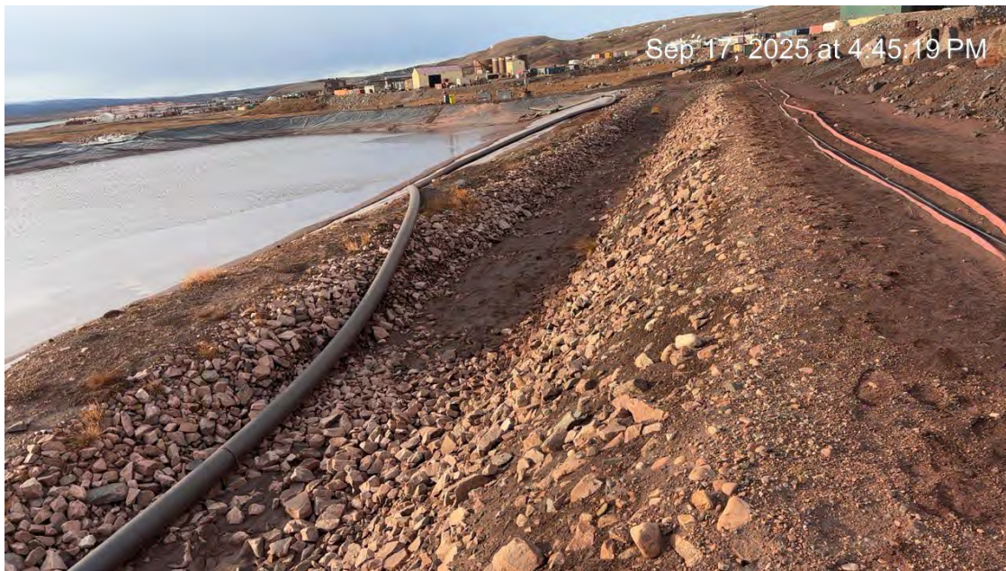
Photo 14 – Berm and ditches surrounding the Crusher Pond (September 17, 2025).
