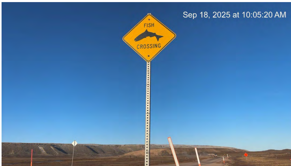
Photo 30 – Example of newly installed 'Fish Crossing' sign at KM95 (September 18, 2025).
