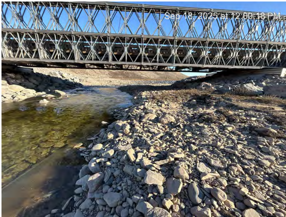
Photo 46 – Clear, flowing water at KM63 bridge (September 18, 2025).
