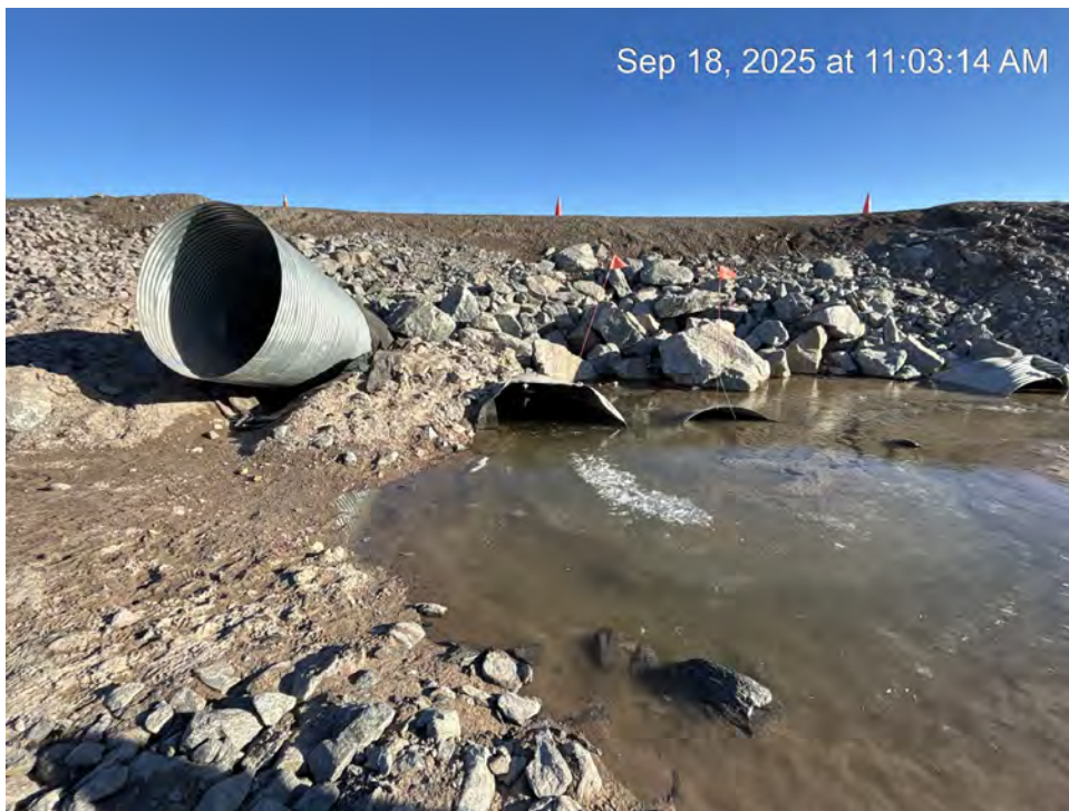
Photo 38 – Compressed culverts at KM216 (September 18, 2025).
