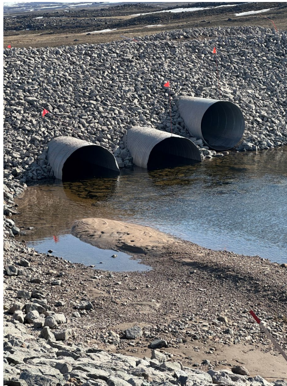
Photo 21 – Culvert replacement on the Tote Road (June 19 th , 2025).
