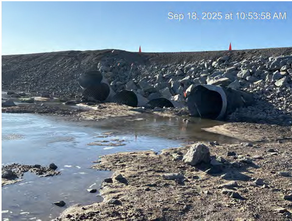
Photo 37 – Compressed culverts at KM216 (September 18, 2025).
