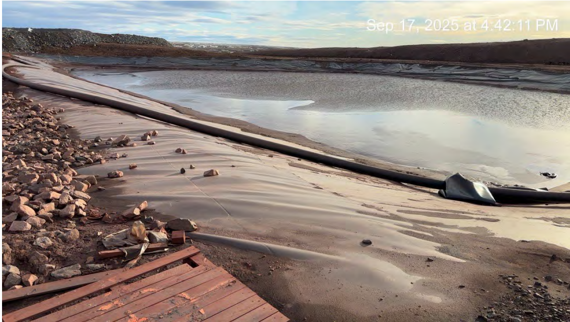
Photo 13 – Low water levels in the Crusher Pond (September 17, 2025).
