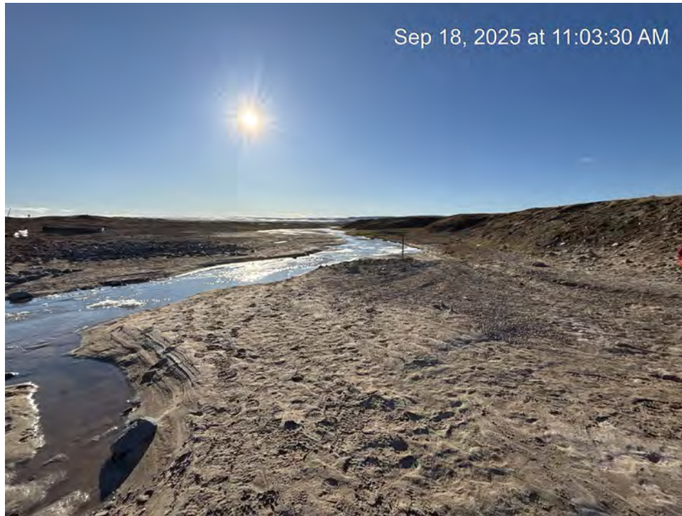
Photo 39 – Location of Tote Road relocation 30 m south of existing culverts at KM81 (September 18, 2025).
