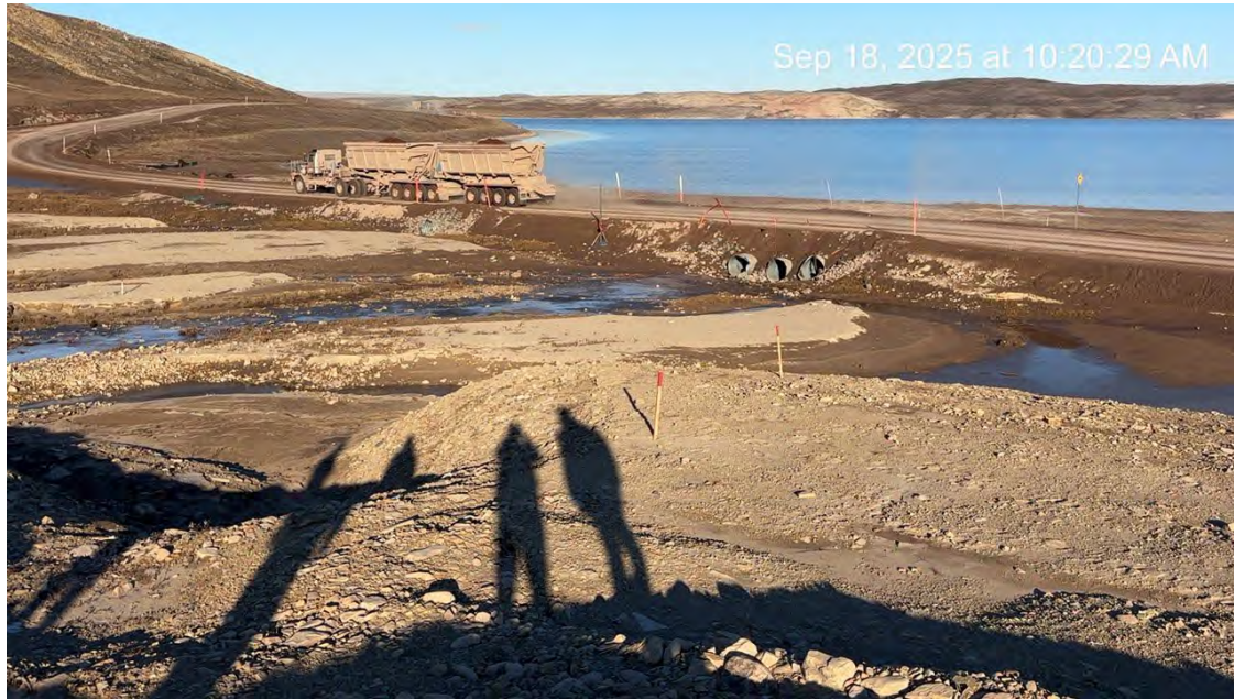
Photo 33 – Area of erosion (KM87.5) adjacent to David's Lake (September 18, 2025).
