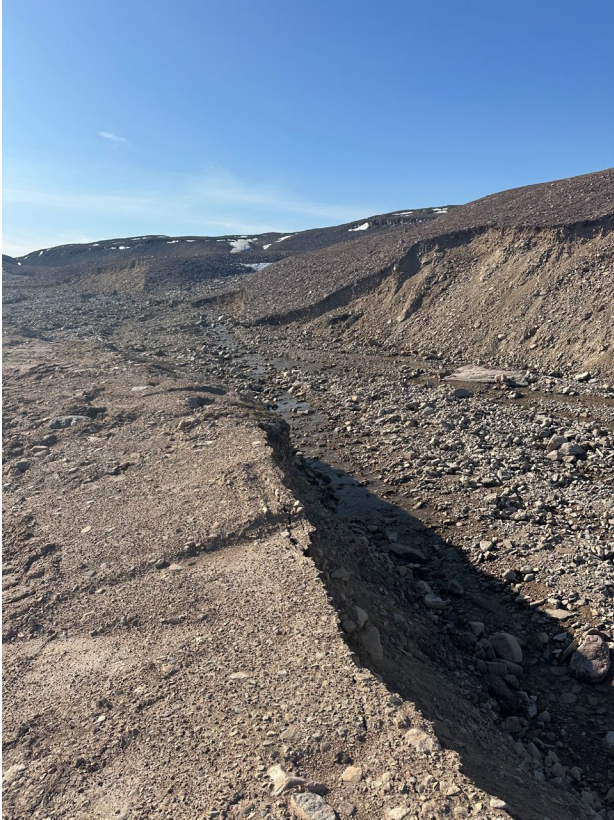
Photo 23 – KM63.5 washout (June 19 th , 2025).
