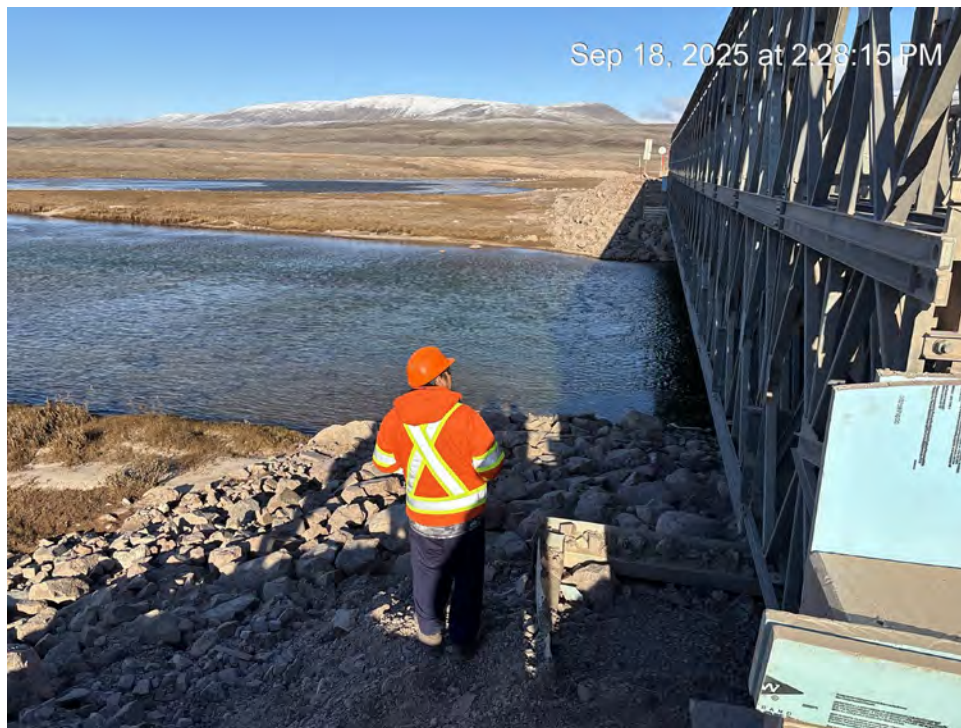
Photo 50 – Corner of buried sea can used to reinforce KM17 bridge (September 18, 2025).
