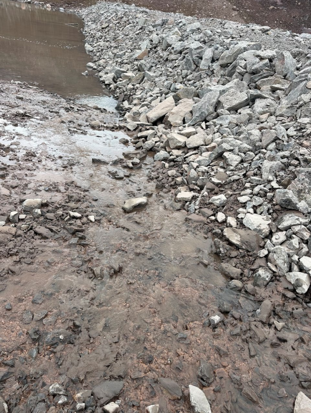
Photo 9 – Horizontal view of the new filter berm (June 18 th , 2025).
