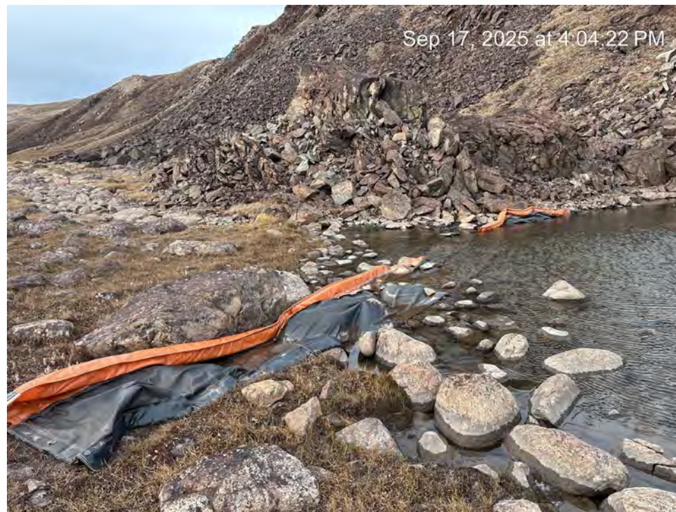
Photo 10 – Final discharge point and location of proposed weir structure downstream of KM105 (September 17, 2025).
