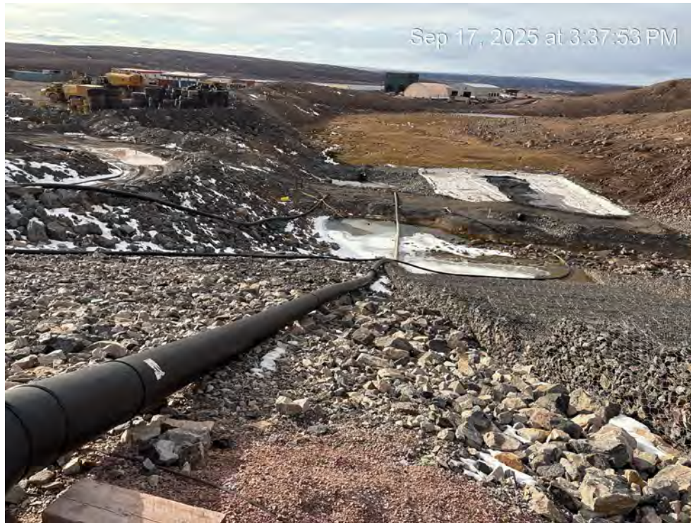
Photo 7 –Geotube infrastructure in place but not in use downstream of KM105 dam (September 17, 2025).
