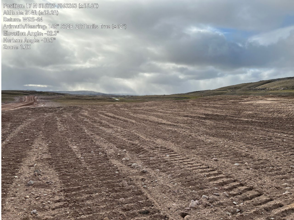
Figure 3.13: Reclaimed borrow area adjacent to Tote Road at KM 37
