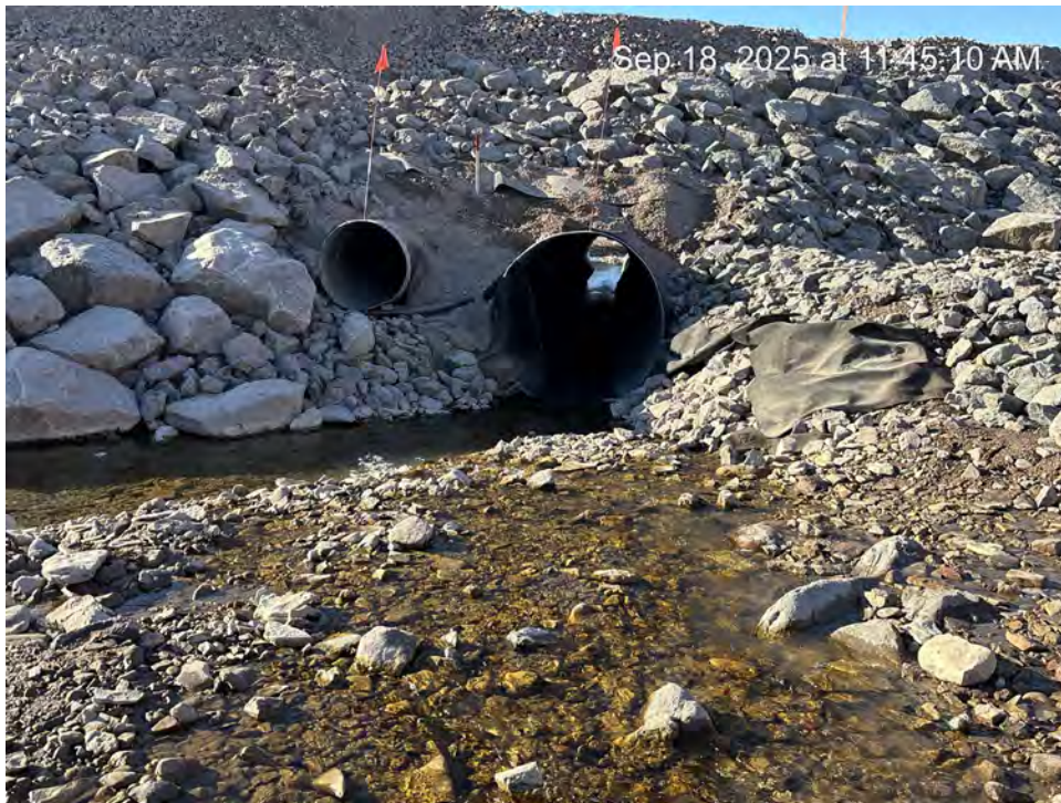
Photo 42 – Culverts at KM64 (September 18, 2025).
