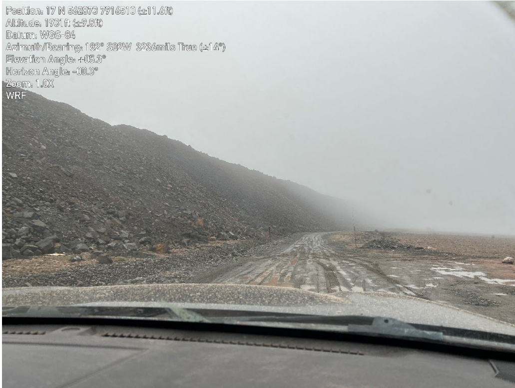
Figure 3.2: Eastern slope of WRF. No erosional or stability concerns noted.
