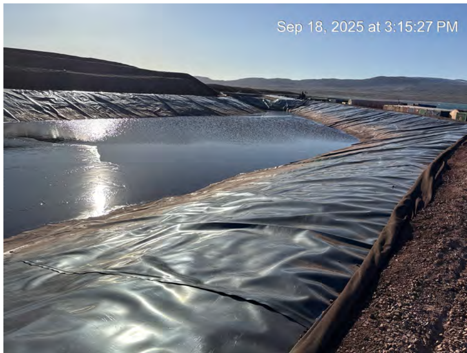
Photo 52 – West stockpile discharge pond (September 18, 2025).
