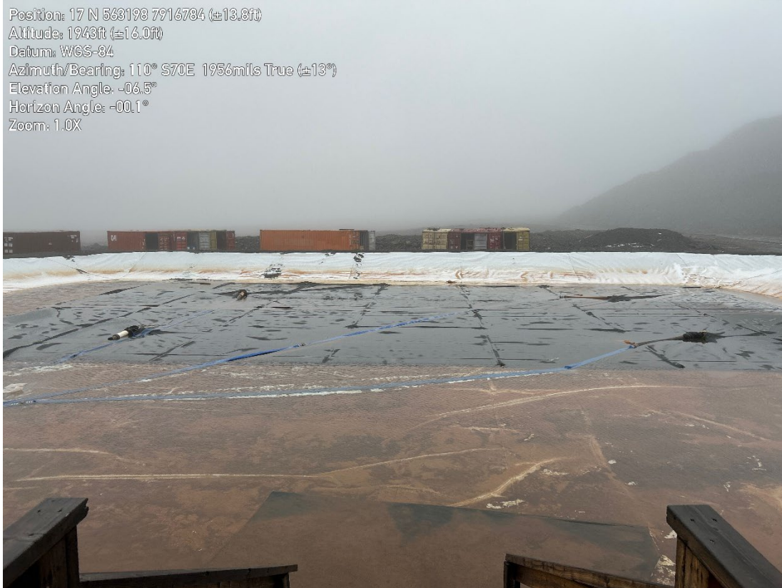
Figure 3.3: Geobags at water treatment plant (installed in 2024)
