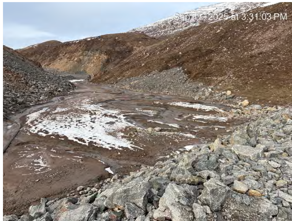
Photo 6 – Accumulation of sediment downstream of second filter berm at KM105 pond (September 17, 2025).
