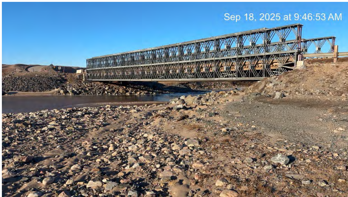
Photo 28 – Reinforced bridge at KM97 (September 18, 2025).
