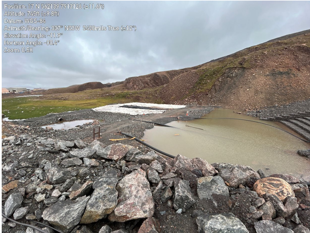
Figure 3.11: Downstream check dam and water treatment area downstream of KM 105 embankment
