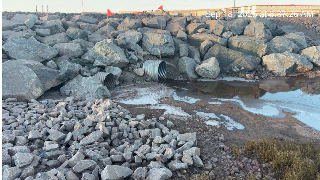
Photo 19 – CV187 replaced in June 2025 (September 18, 2025).
