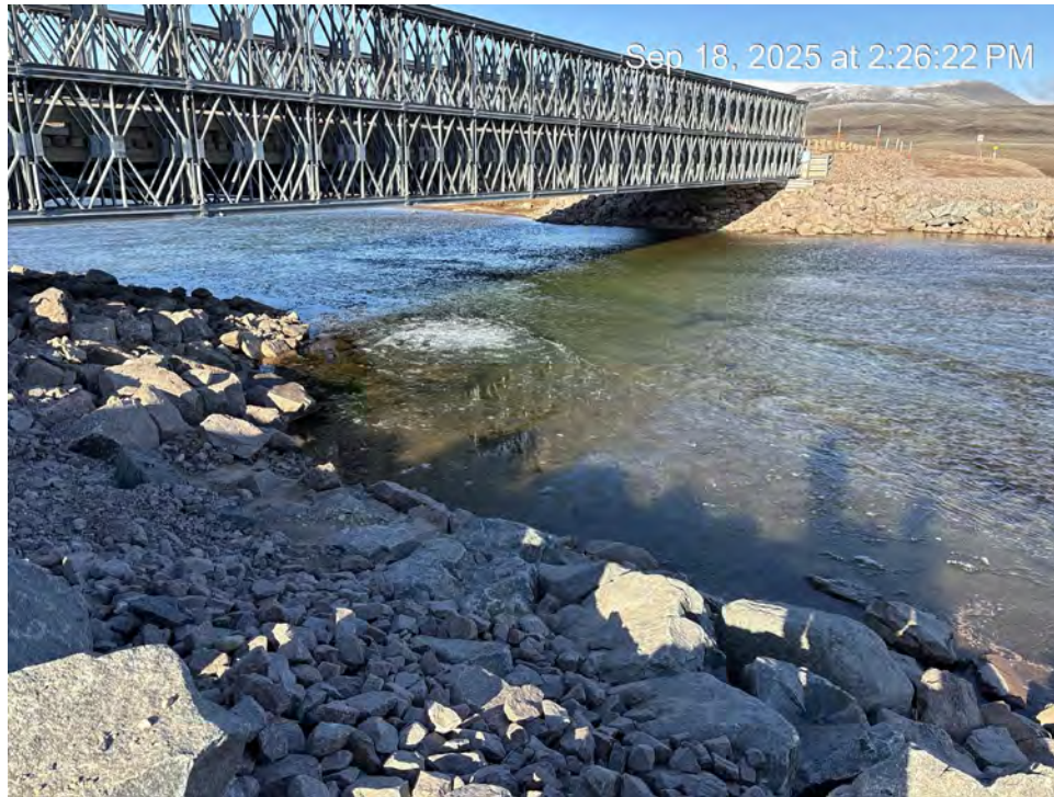
Photo 49 – Clear flows under KM17 bridge (September 18, 2025).
