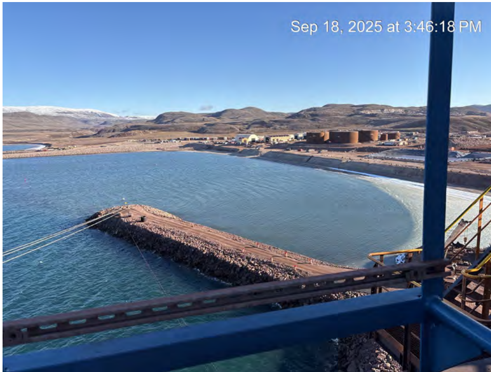
Photo 53 –View of Milne Port infrastructure from the ship loader (September 18, 2025).
