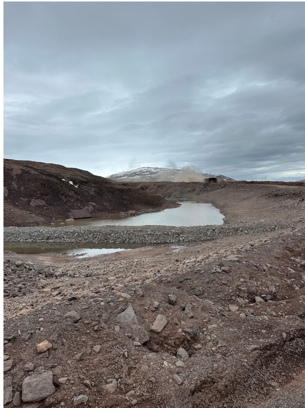
Photo 7 – New filter berm upstream of KM105 (June 18 th , 2025).
