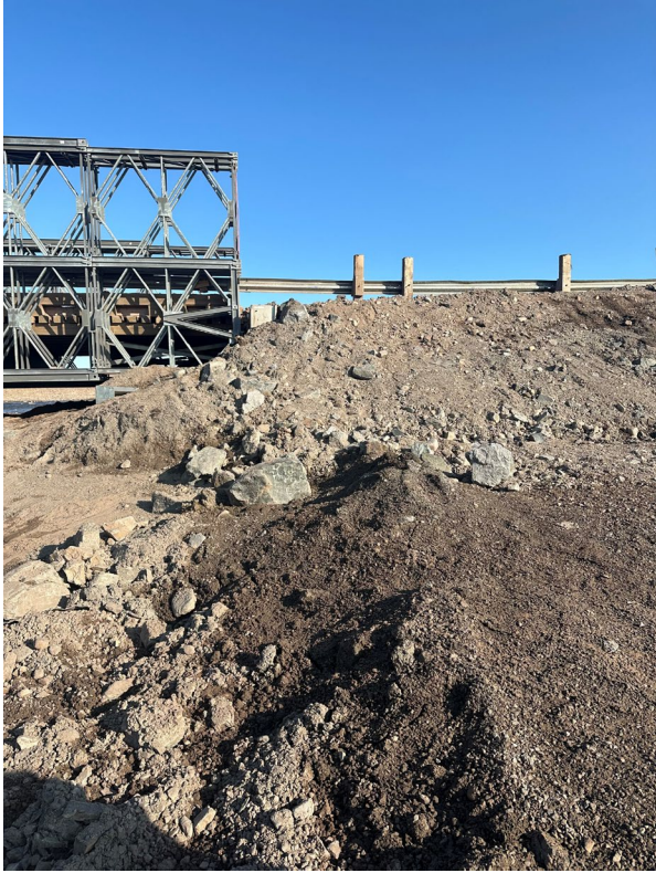
Photo 19 – KM97 Bridge crossing reinforced during winter 2025 (June 19 th , 2025).
