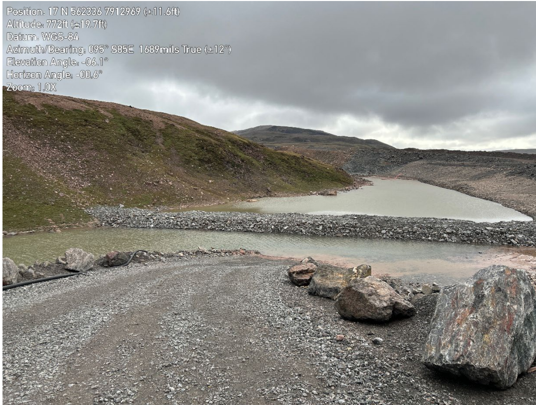
Figure 3.10: Upstream check dam installed for TSS settlement
