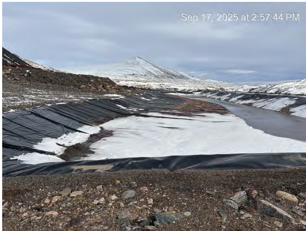
Photo 3 – Low water levels in KM 106 pond (September 17, 2025).
