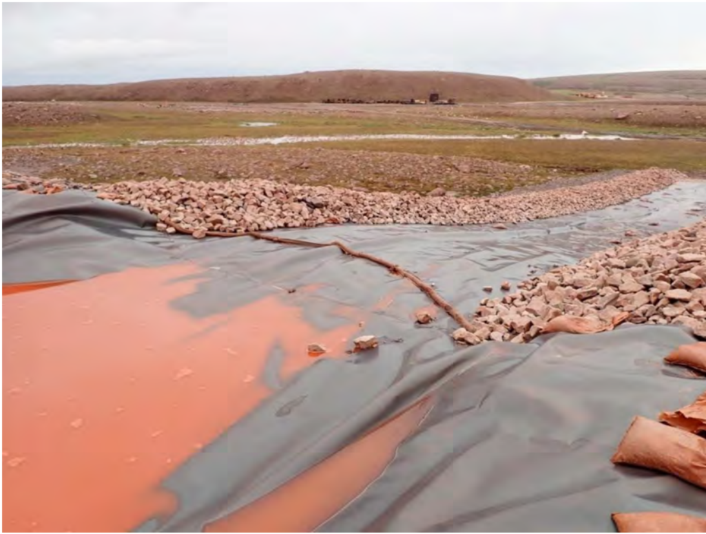
Photo 1: Effluent Emerging onto Emergency Spillway of MS-06 Pond at 19:30hrs – July 16, 2025
