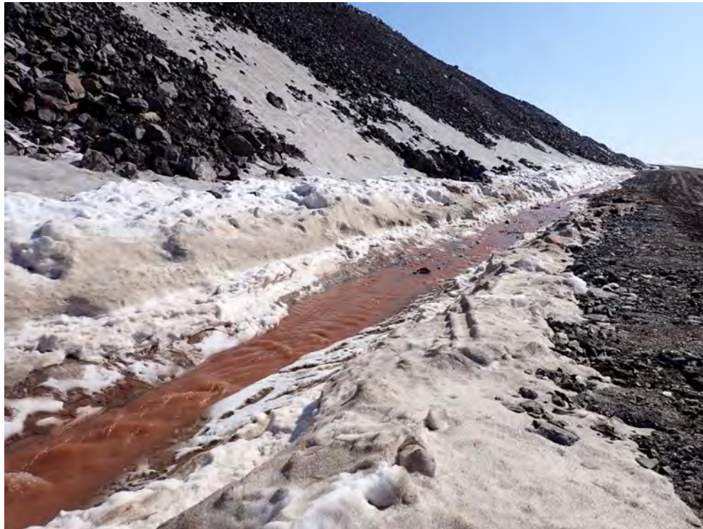
Photo 4: Snow Cleared from West Perimeter Ditch Restoring Proper Ditch Gradient and Improving Water Flow, June 21, 2025
