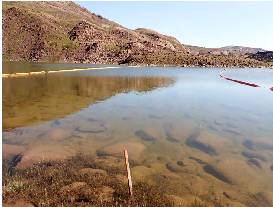
Photo 13. Silt Curtains inside the MS-C-F Settling Pond – July 20, 2025
