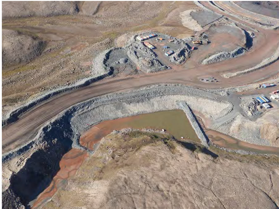
Photo 4 Filter Berm within the KM 105 Valley – August 23, 2025
