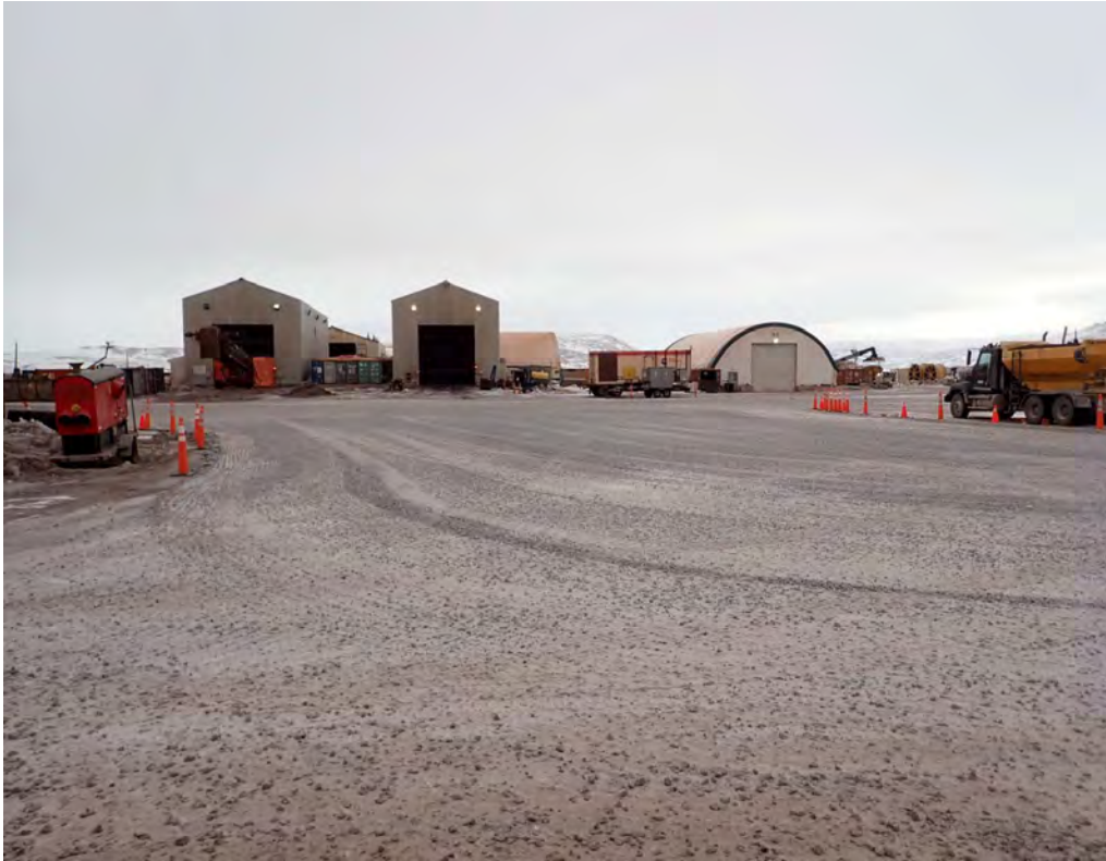
Photo 5: Clean Fill Material Placed and Area Regraded – May 12, 2025
