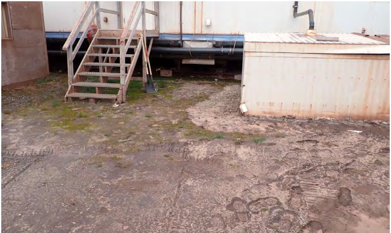
Photo 2: MSC Lift Station Release Following Clean Up – August 14, 2025
