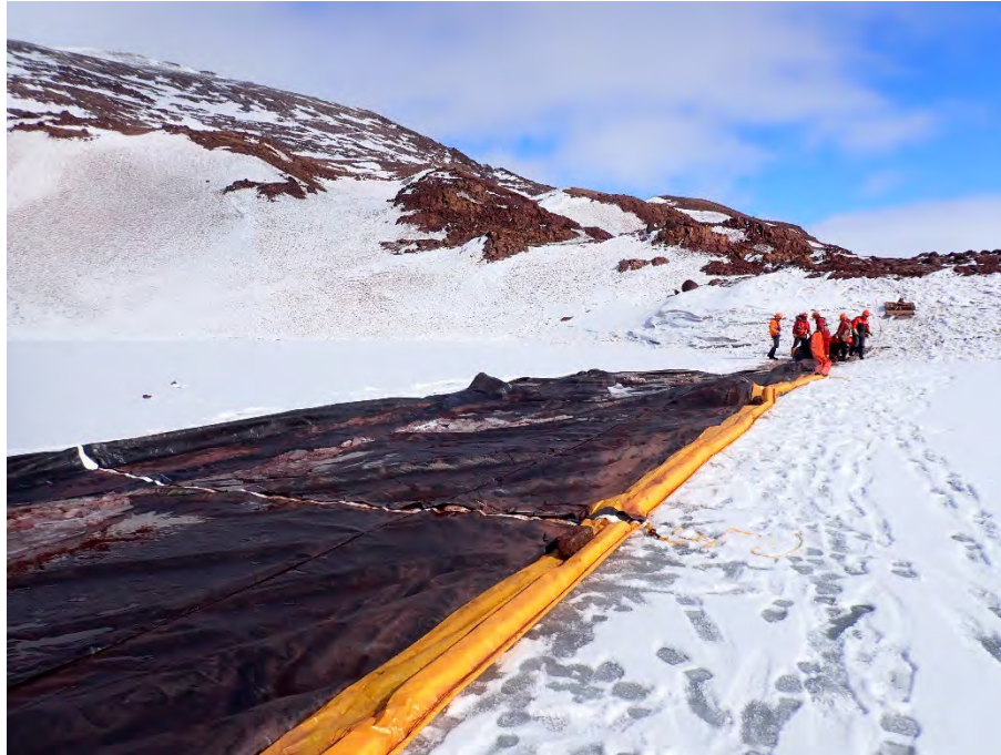
Photo 7. Maintenance and Preparation of Silt Curtains at MS-C-F Settling Pond Downstream of KM 105 – May 18, 2025
