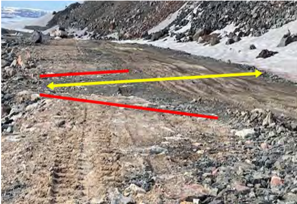
Photo 3: Course Rock Fill Material Perpendicular to WRF Road Previously Placed to Repair Road Settlement
