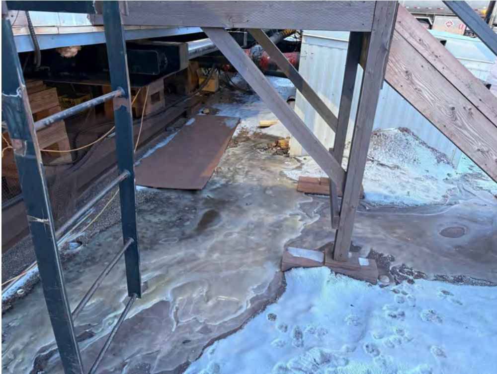
Photo 1: Mine Site Complex Laundry Lift Station Spill Location – Spilled Sewage Frozen on Ground - March 29, 2025
