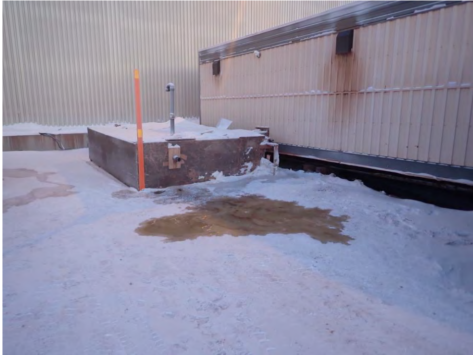
Photo 1: Milne Port South Maintenance Shop Lift Station - Sewage Spilled onto Snow, February 1, 2024
