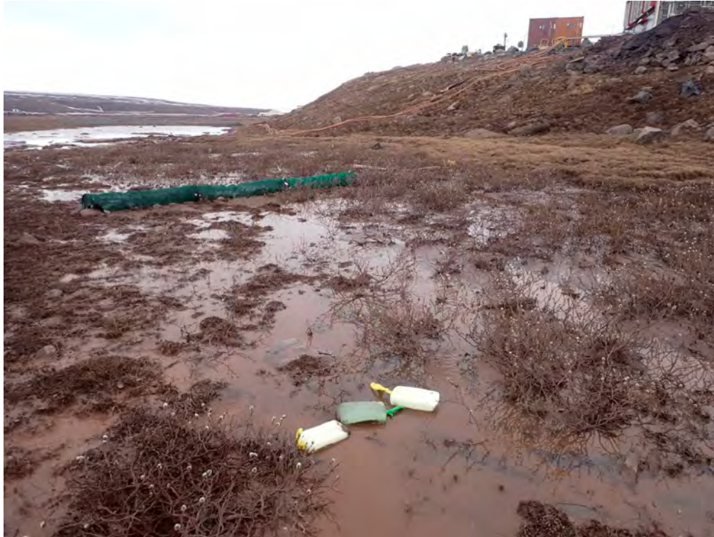
Photo 11: Spring Berms Deployed Upstream of Filter Berm C With Additional Floc Blocs – May 26, 2025
