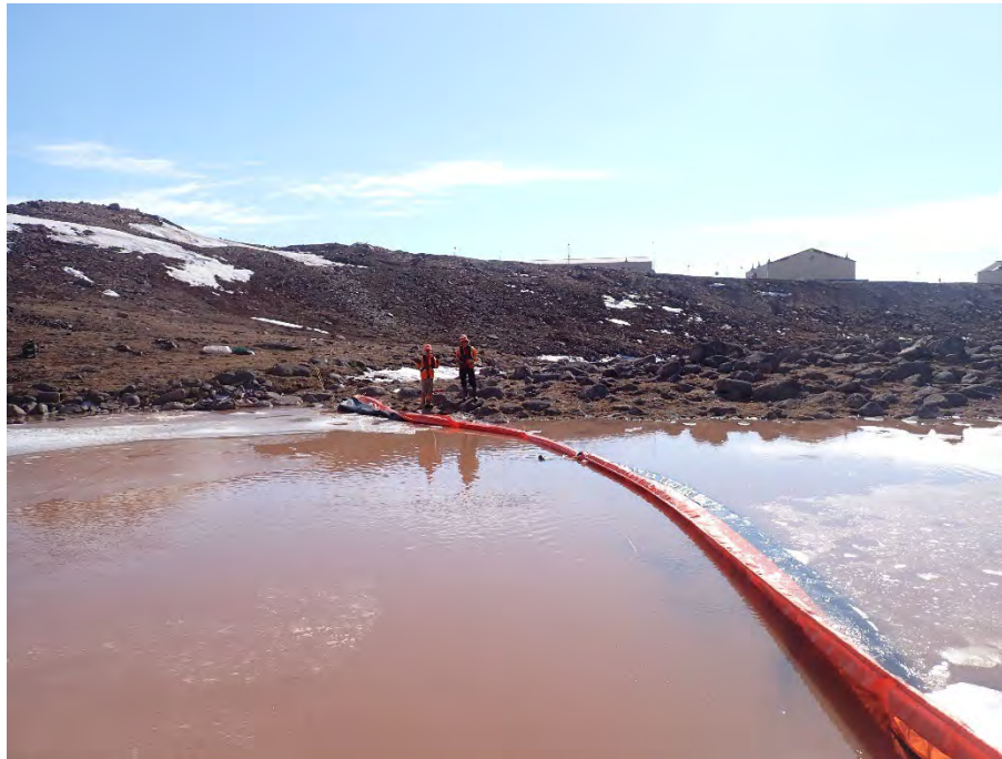
Photo 11. Installation of Silt Curtain Upstream of the Proposed MS-11 Discharge Location – May 23, 2025
