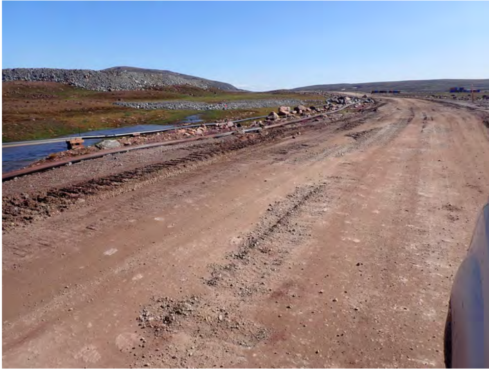
Photo 5: Dedicated Discharge Line Installed for the MS-06 Pond, Running Beside the WWTP Effluent Line to the Outfall Location – July 20, 2025
