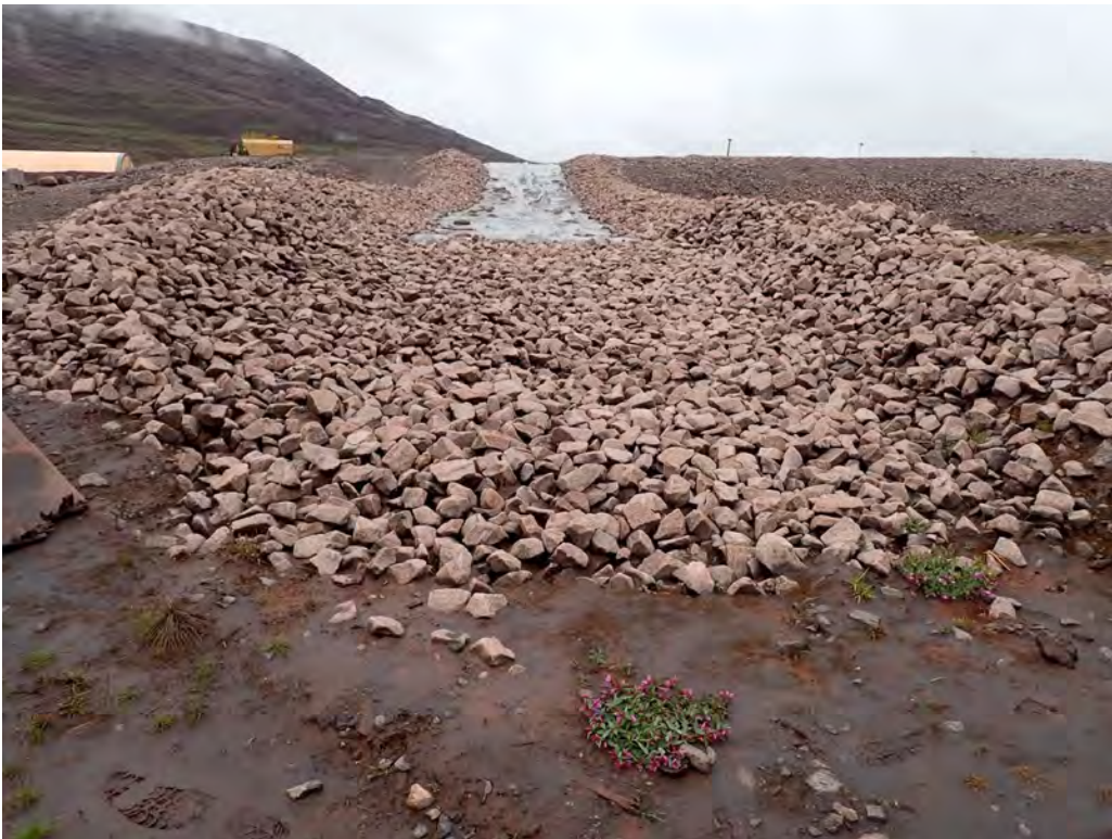
Photo 2: Tundra View of Slow Release into Rip Rap below the Emergency Spillway – July 16, 2025
