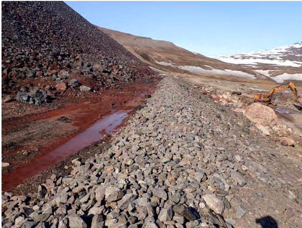
Photo 1: Water Pooling on the Upgradient Side of the Diversion Berm – June 6, 2025
