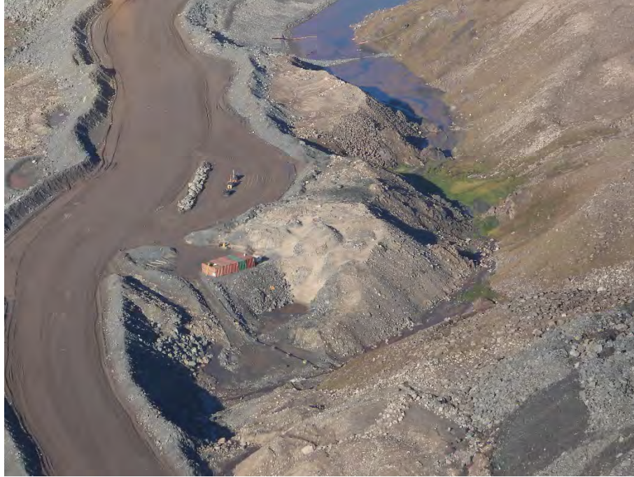
Photo 3. KM 105 Valley Inflow Pre-dosing Plant – August 23, 2025
