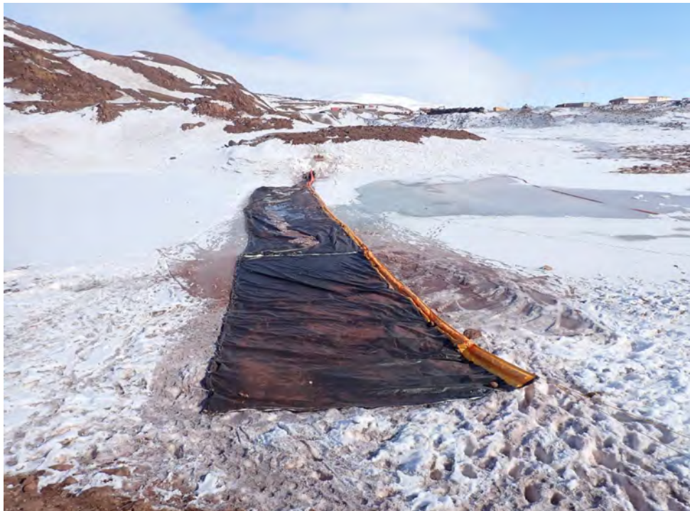
Photo 6: Maintenance and Preparation of Silt Curtains at MS-C-F Settling Pond Downstream of the Dam - May 18, 2025
