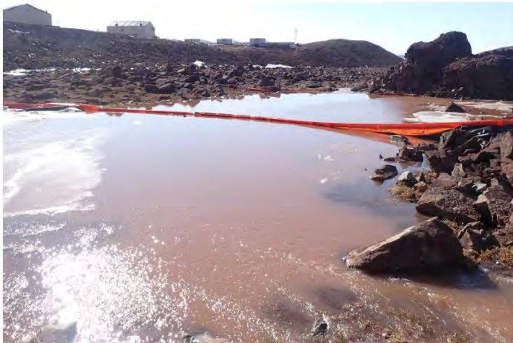
Photo 8: Installation of Silt Curtain Upstream of the Proposed MS-11 Discharge Location - May 23, 2025
