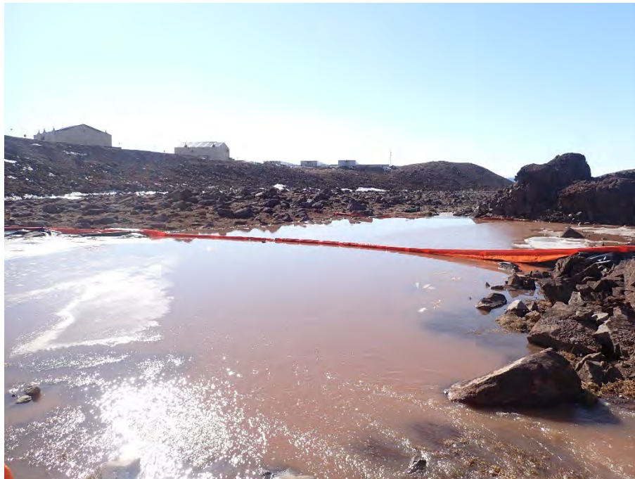
Photo 10. Installation of Silt Curtain Upstream of the Proposed MS-11 Discharge Location – May 23, 2025
