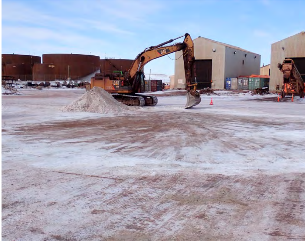
Photo 3: Excavation of Contaminated Snow & Ice – May 4, 2025
