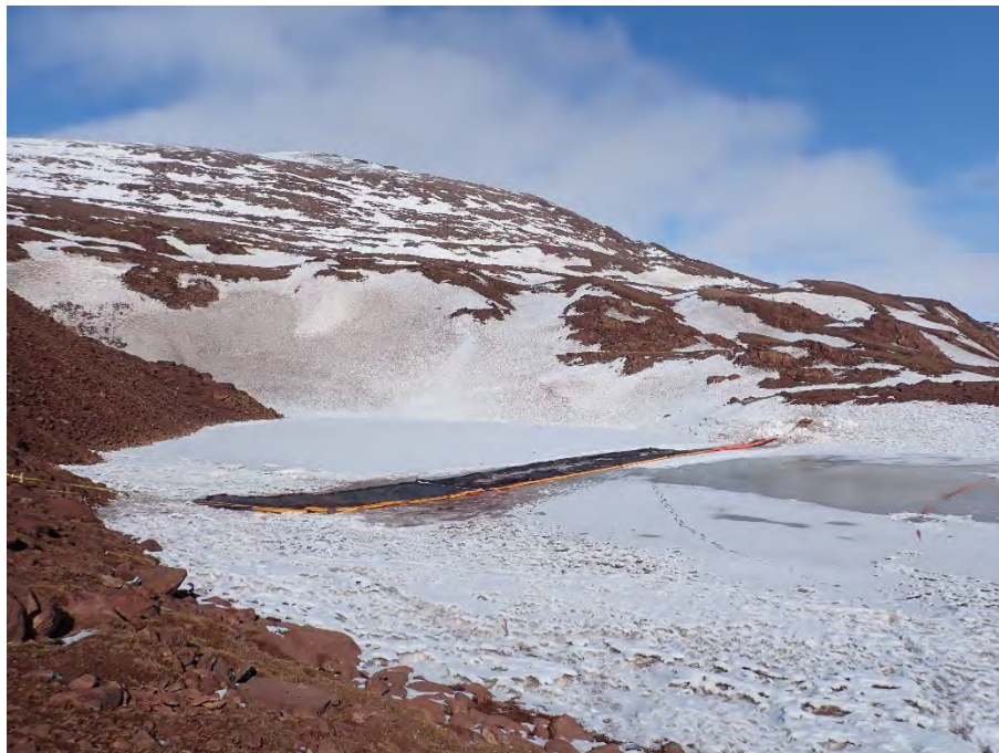
Photo 8. Maintenance and Preparation of Silt Curtains at MS-C-F Settling Pond Downstream of KM 105 – May 18, 2025
