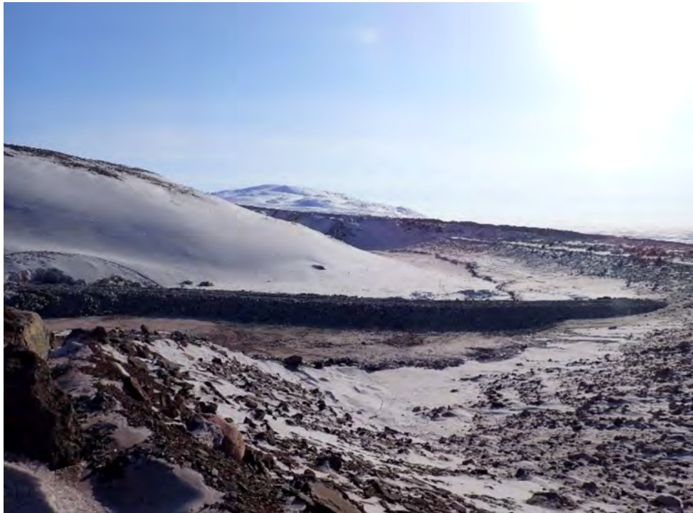
Photo 7: Filter Berm within KM 105 Valley Water Management Infrastructure - March 31, 2025
