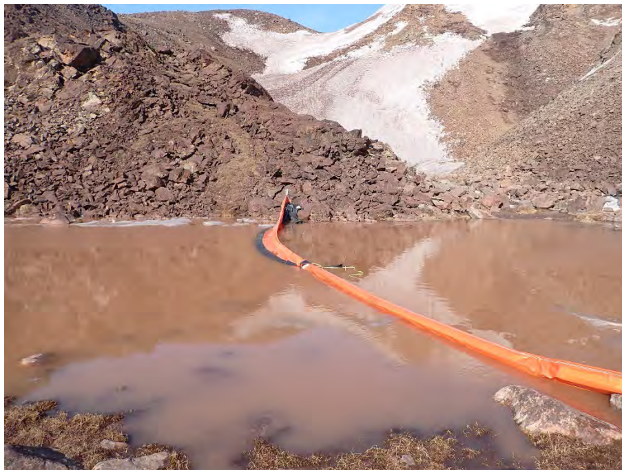
Photo 12. Installation of Silt Curtain Upstream of the Proposed MS-11 Discharge Location – May 23, 2025
