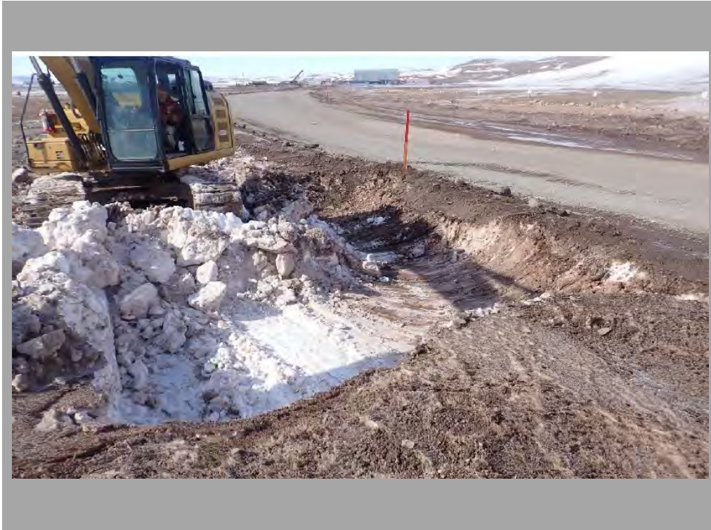
Photo 14: Excavator clearing dust impacted snow from a culvert inlet May 11 2025
