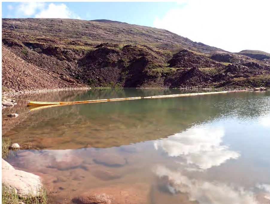
Photo 14. Silt Curtain inside the MS-C-F Settling Pond – July 7, 2025
