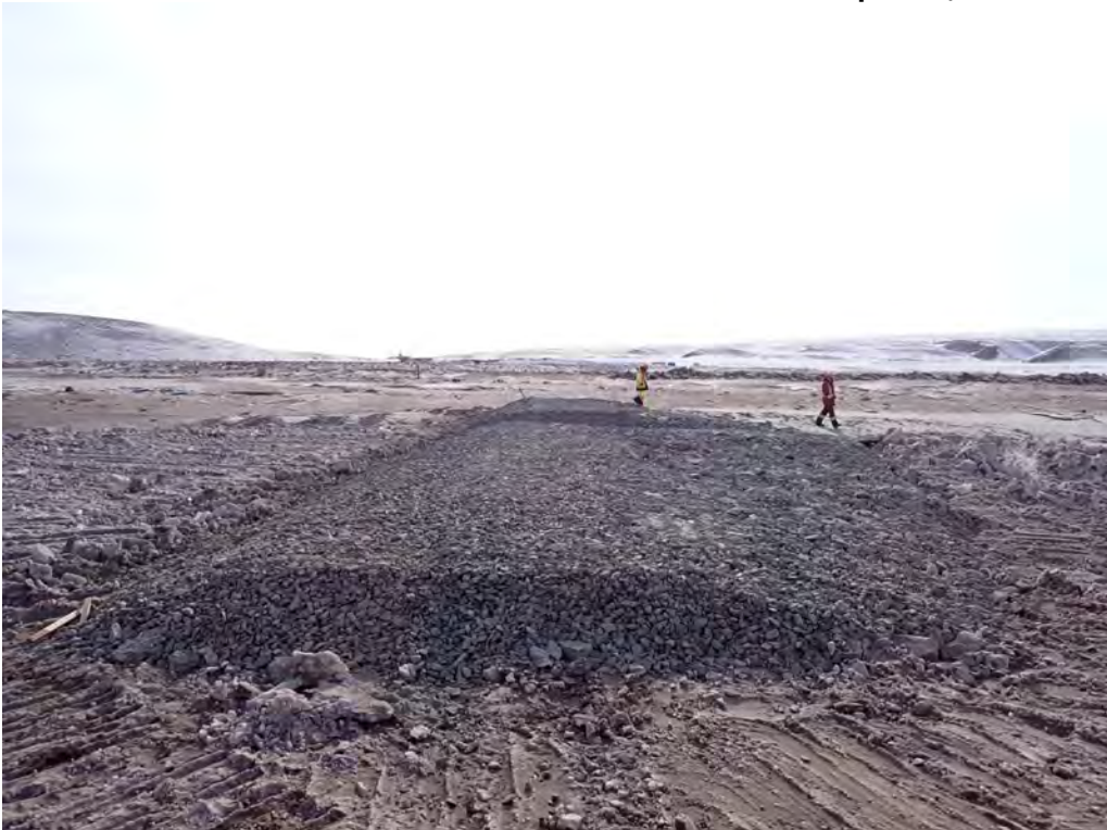
Photo 4: Rock Filter Berm B Installed Within SDLT - April 18, 2025
