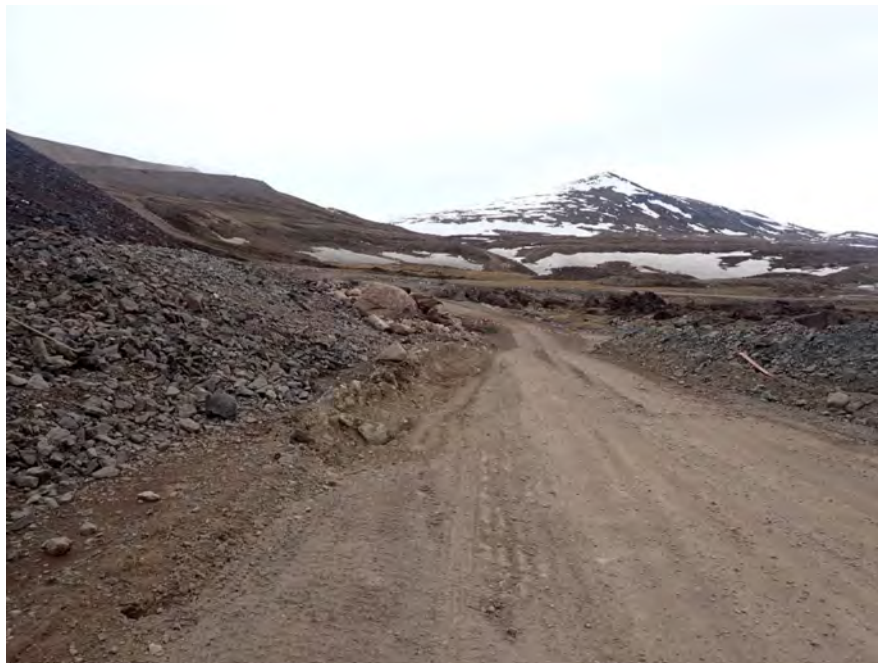
Photo 6: Conditions at MS-106OS-07 During Routine Monitoring Showing Secondary Seepage Collection Ditch Below Diversion Berm – June 18, 2025
