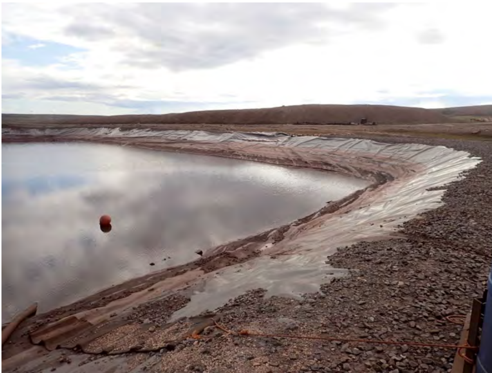
Photo 4: Pond Level in MS-06 Reduced to Low Level – July 28, 2025
