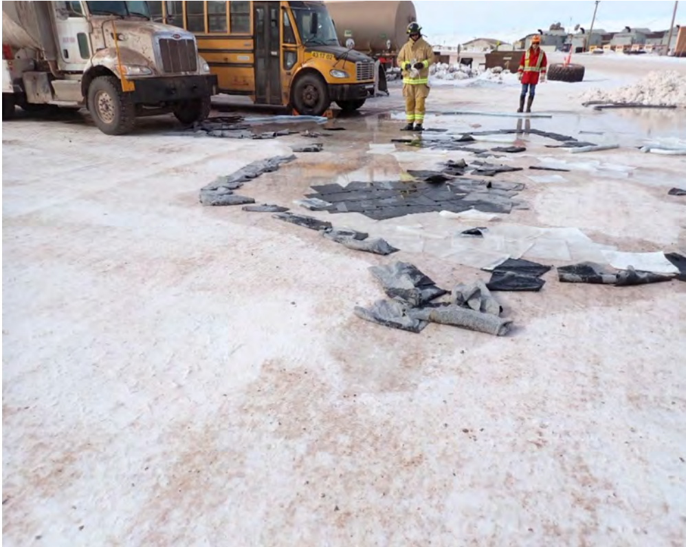
Photo 1: Initial Spill Response; Visible Diesel on Ground Being Absorbed By the Pads – May 4, 2025
