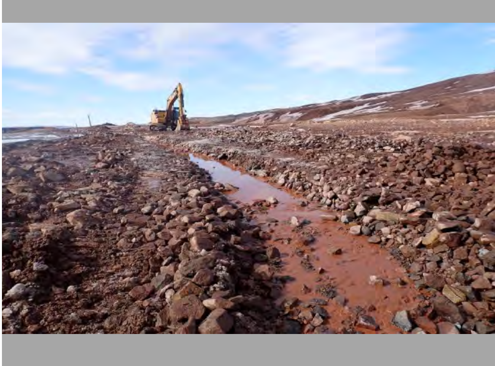
Photo 7: Water Management via Shallow Rip Rapped Ditch Installation to Direct Water Flow Towards Check Dam System at CV-186 Above SDLT - May 23, 2025
