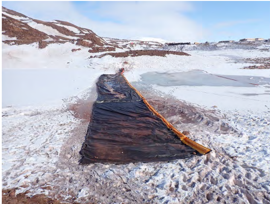
Photo 9. Maintenance and Preparation of Silt Curtains at MS-C-F Settling Pond Downstream of KM 105 – May 18, 2025
