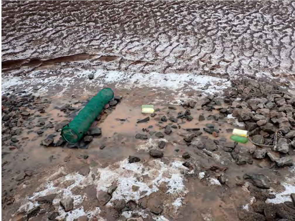
Photo 18: CLSP-OUT Spring berm and Floc Blocs Deployed in the Flow Path – May 26, 2025
