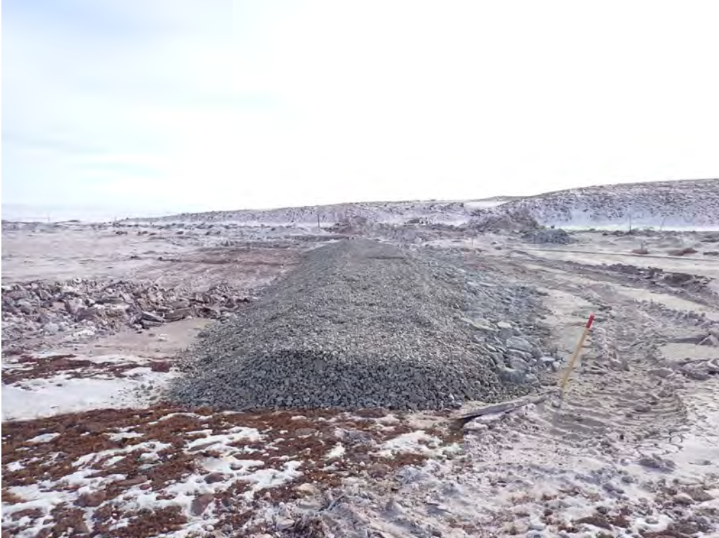
Photo 3: Rock Filter Berm A Installed Within SDLT - April 18, 2025
