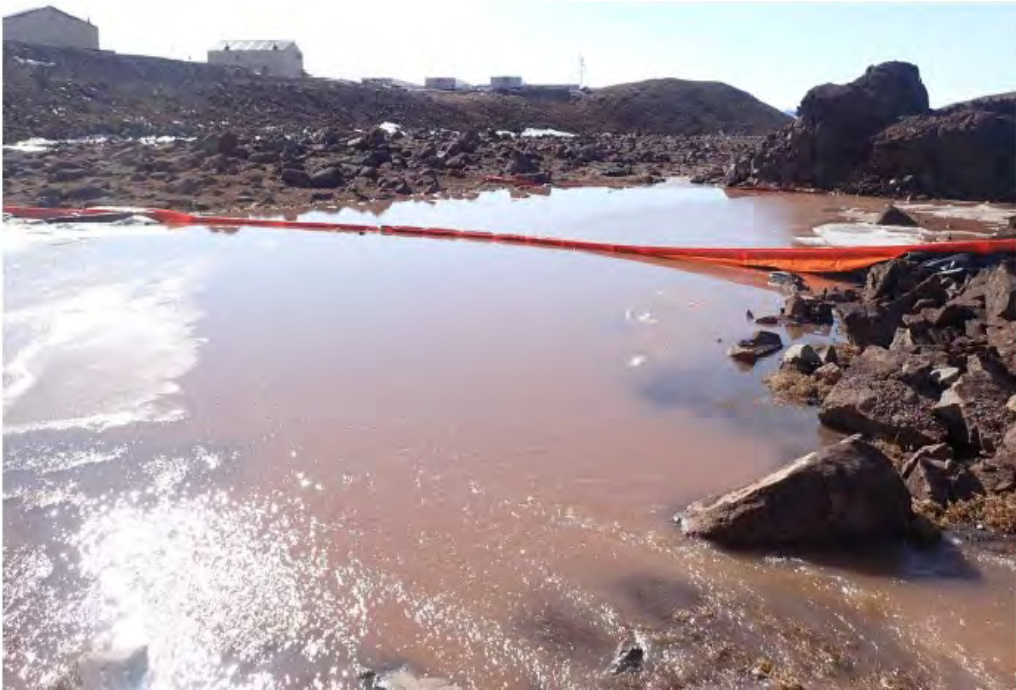
Photo 9: Silt Curtain Installed Within Km 105 Valley Infrastructure Above SDLT May 23 - 2025
