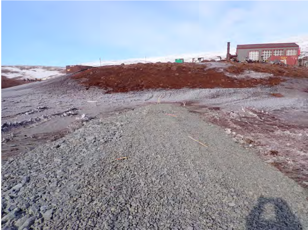
Photo 5: Rock Filter Berm C Installed Within SDLT - April 18, 2025
