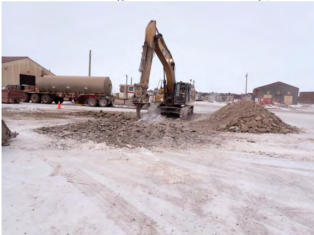
Photo 4: Excavation via Ripper of Contaminated Surface Soils – May 7, 2025
