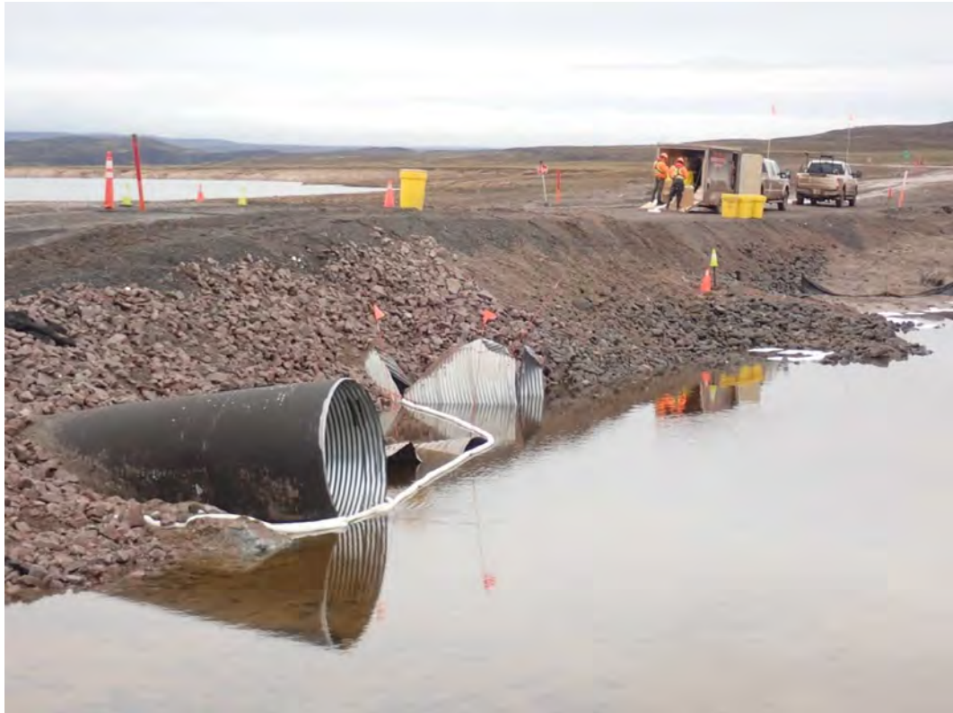
Photo 3: Spill Boom Placed Upstream Around Unobstructed Culverts – July 16, 2025
