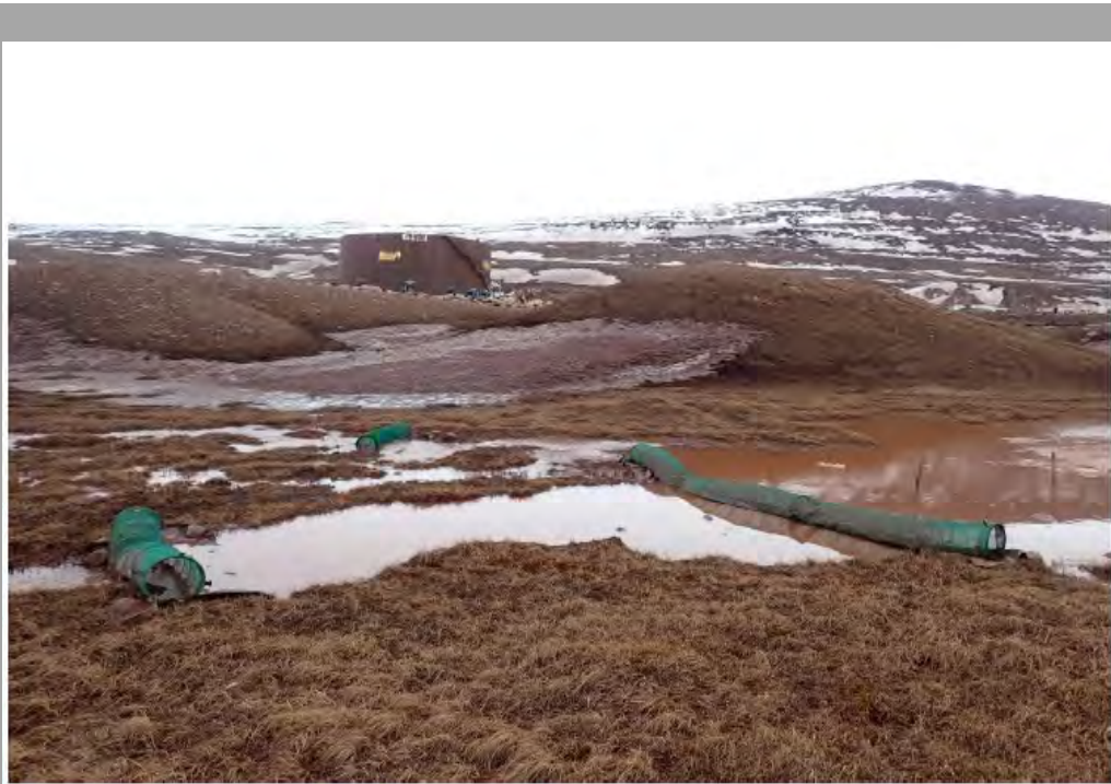
Photo 9: Silt Curtain Installed Within Km 105 Valley Infrastructure Above SDLT May 23 - 2025
