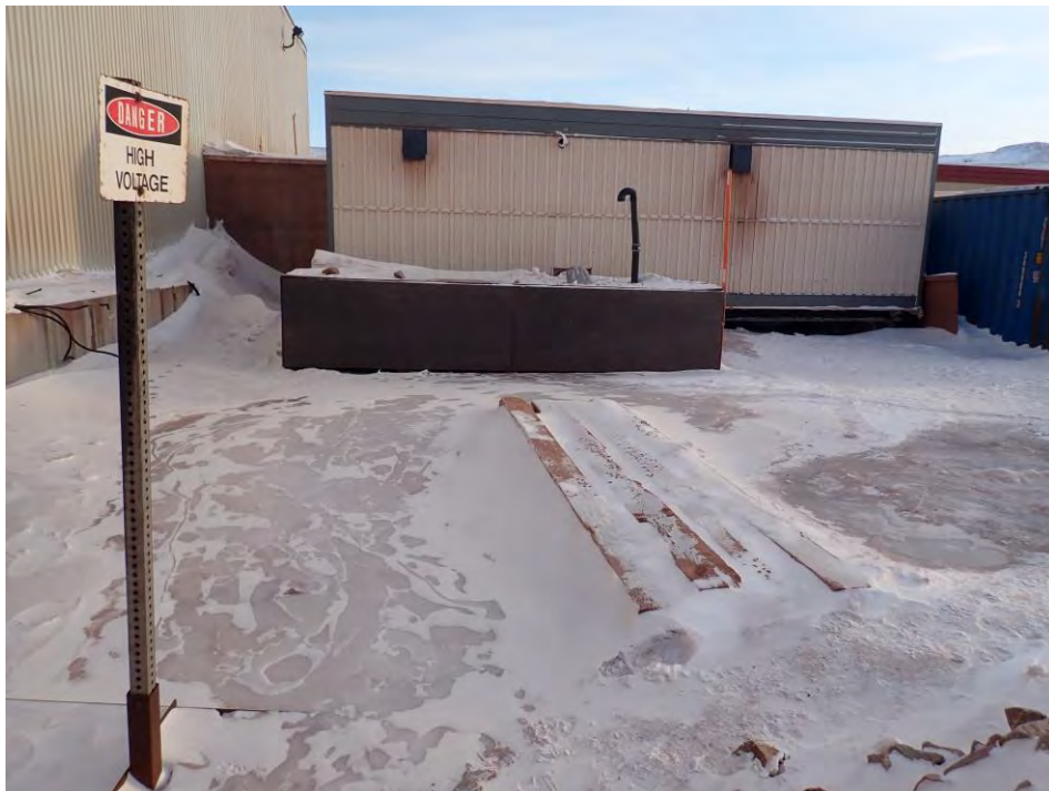
Photo 2: Milne Port South Maintenance Shop Lift Station - Clean Potable water is visible February 27, 2024
