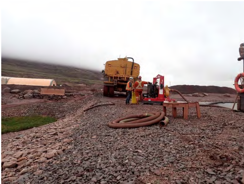
Photo 3: Pond-to-Pond Effluent Transfers via Water Truck in Progress – July 16, 2025
