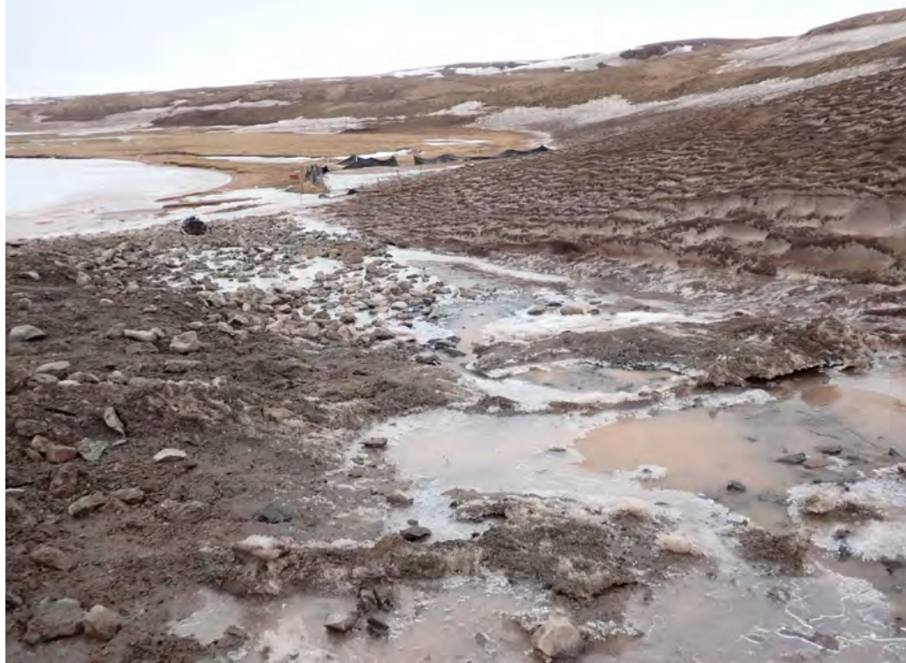
Photo 19: CLSP-OUT Silt Fence Installed Adjacent to Sample Location Preventing Sediment from Snowmelt from Entering Camp Lake – May 24, 2025
