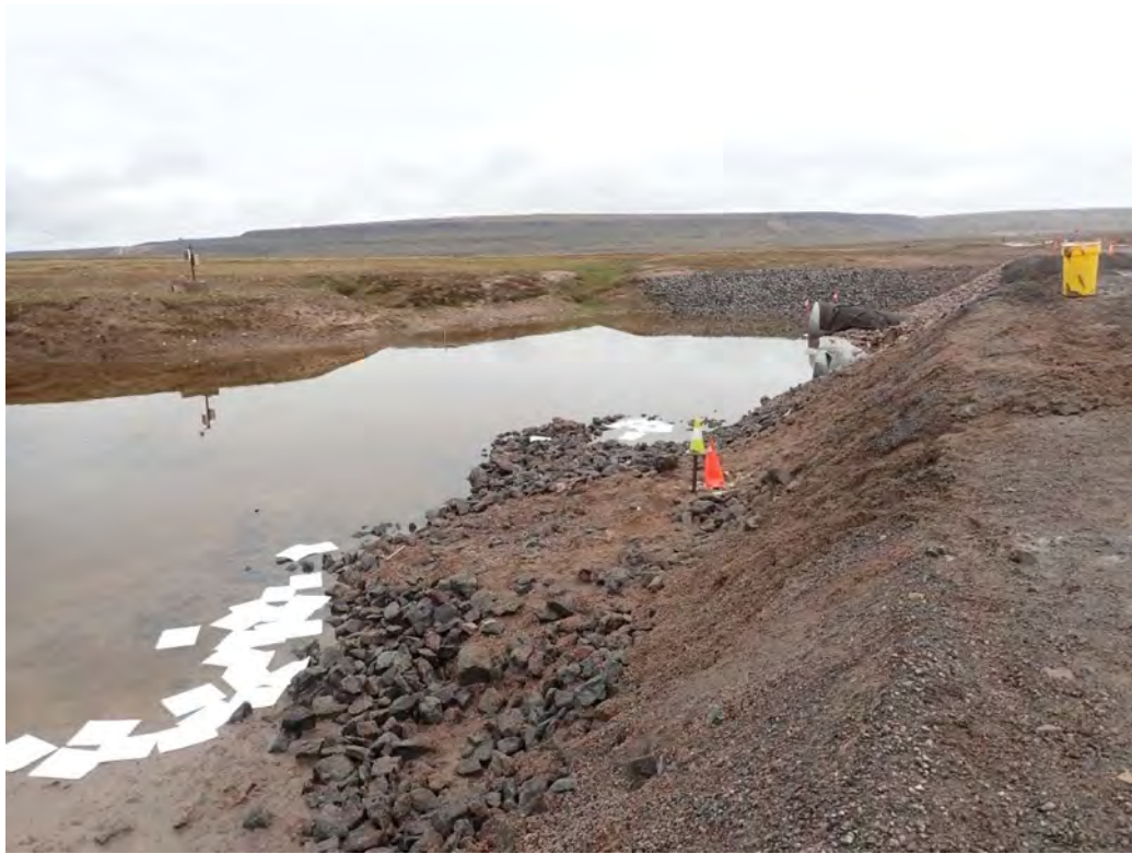
Photo 1: Spill Pads Placed on Contaminated Soil and Surface of the Water Upstream of CV-216 – July 16, 2025
