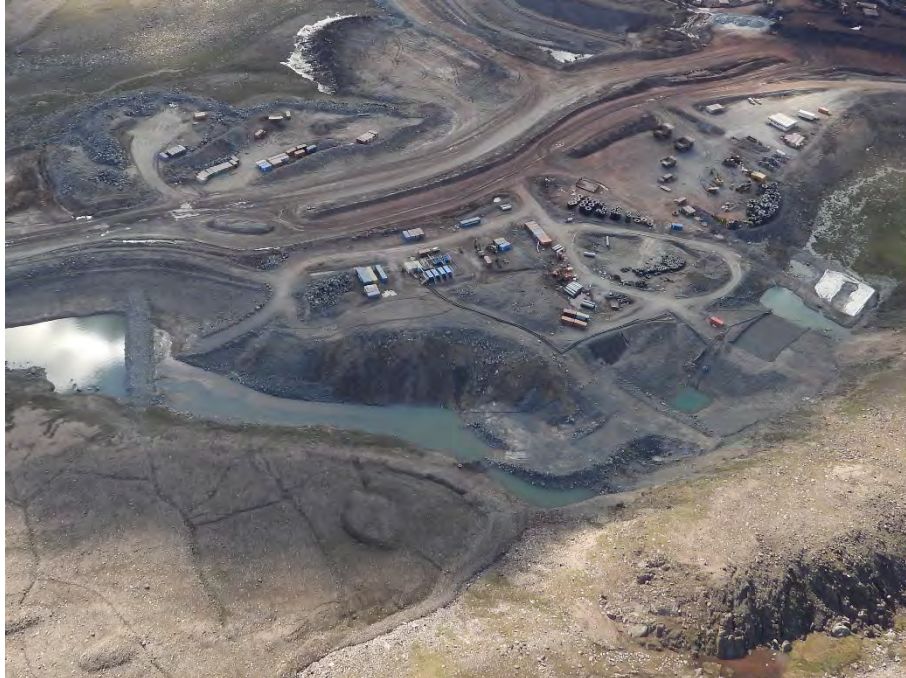
Photo 2. Filter Berm and Downstream Infrastructure within the KM 105 Valley – June 29, 2025
