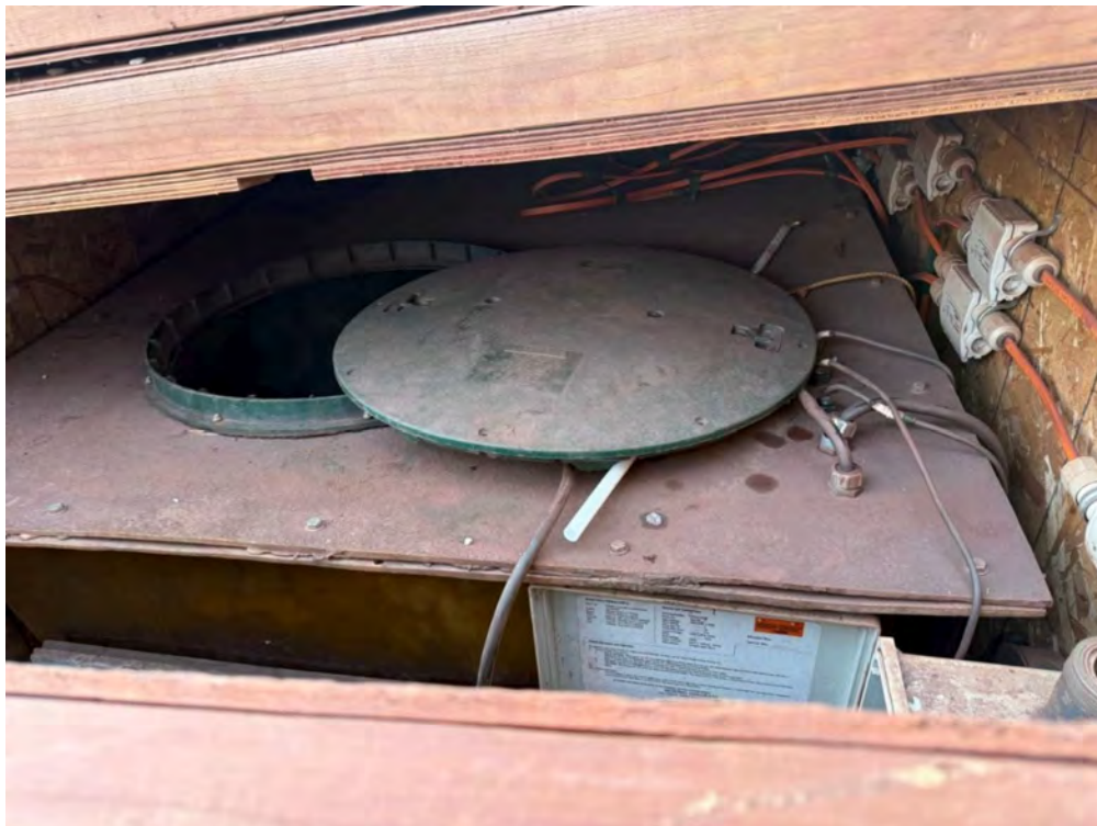
Photo 4: Mine Site Complex Laundry Lift Station - March 29, 2025
