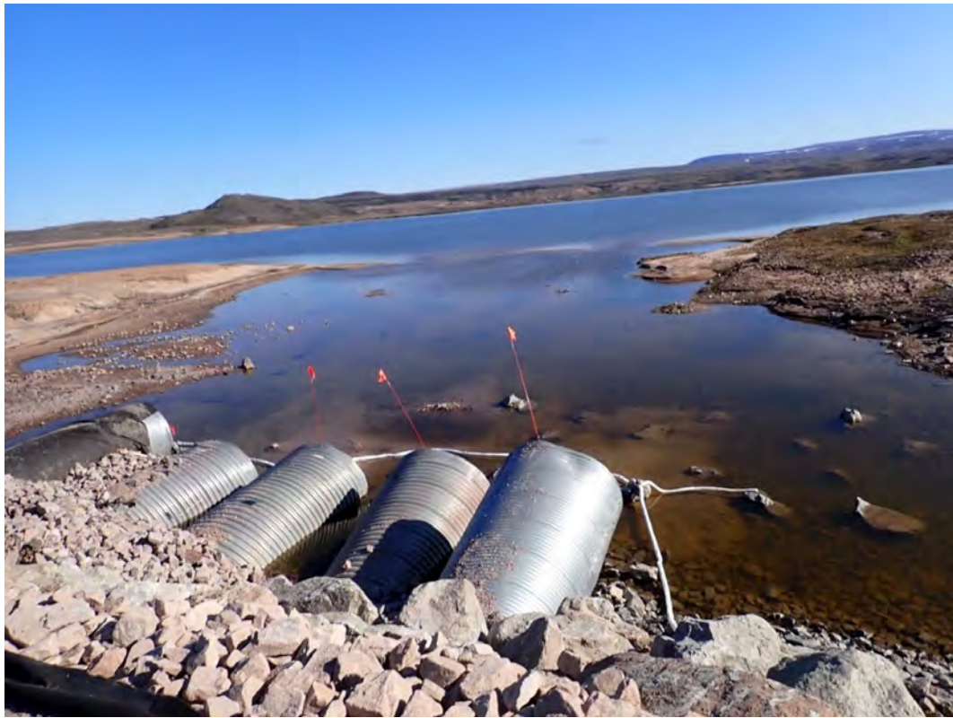
Photo 7: Downstream Conditions Prior to Removal of Spill Response Equipment – July 20, 2025
