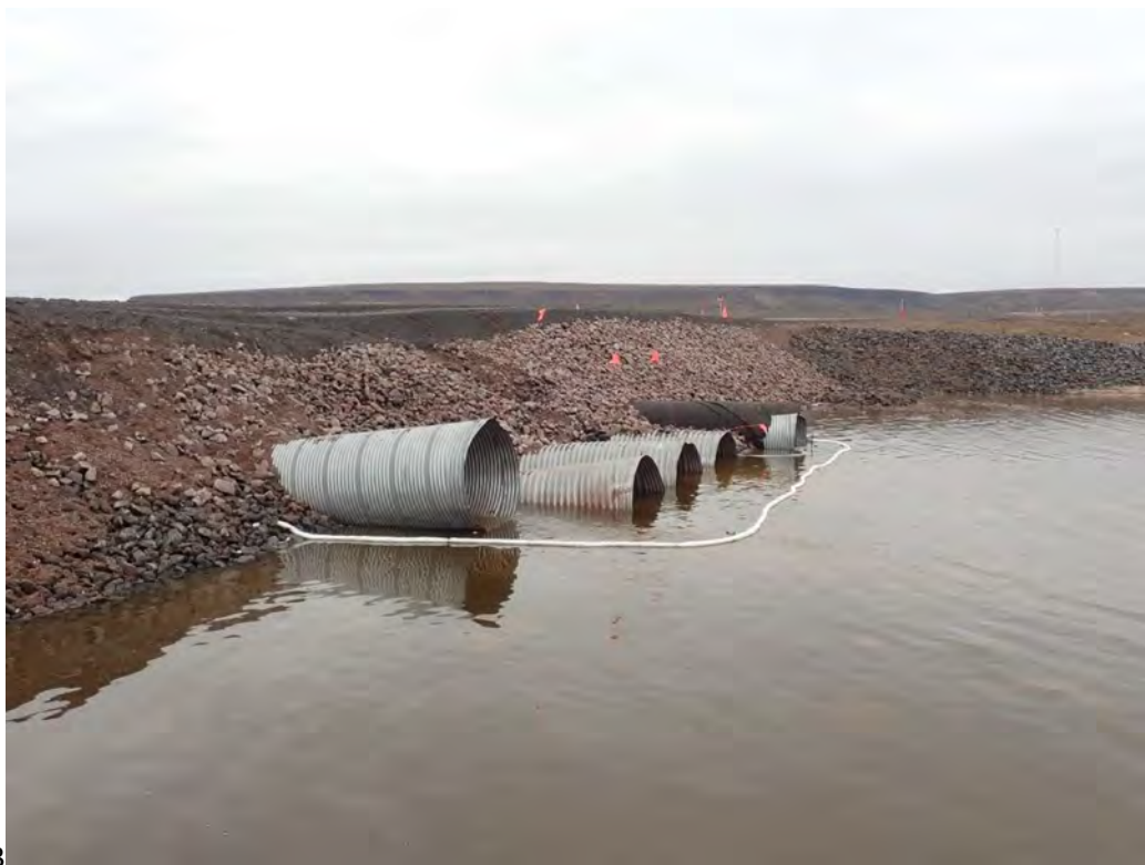
Photo 2: Spill Boom Placed Downstream – July 16, 2025
