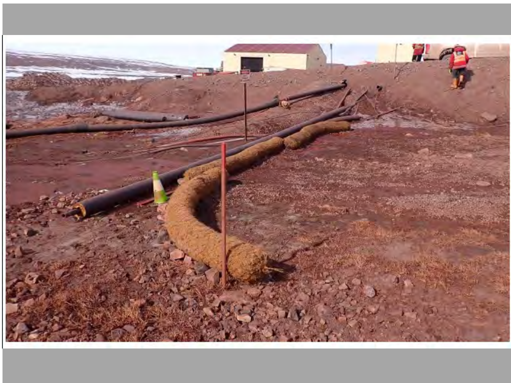
Photo 6: Coir Logs Installed Upstream of SDLT-OUT near MS-C-C and MS-C-D - May 20, 2025
