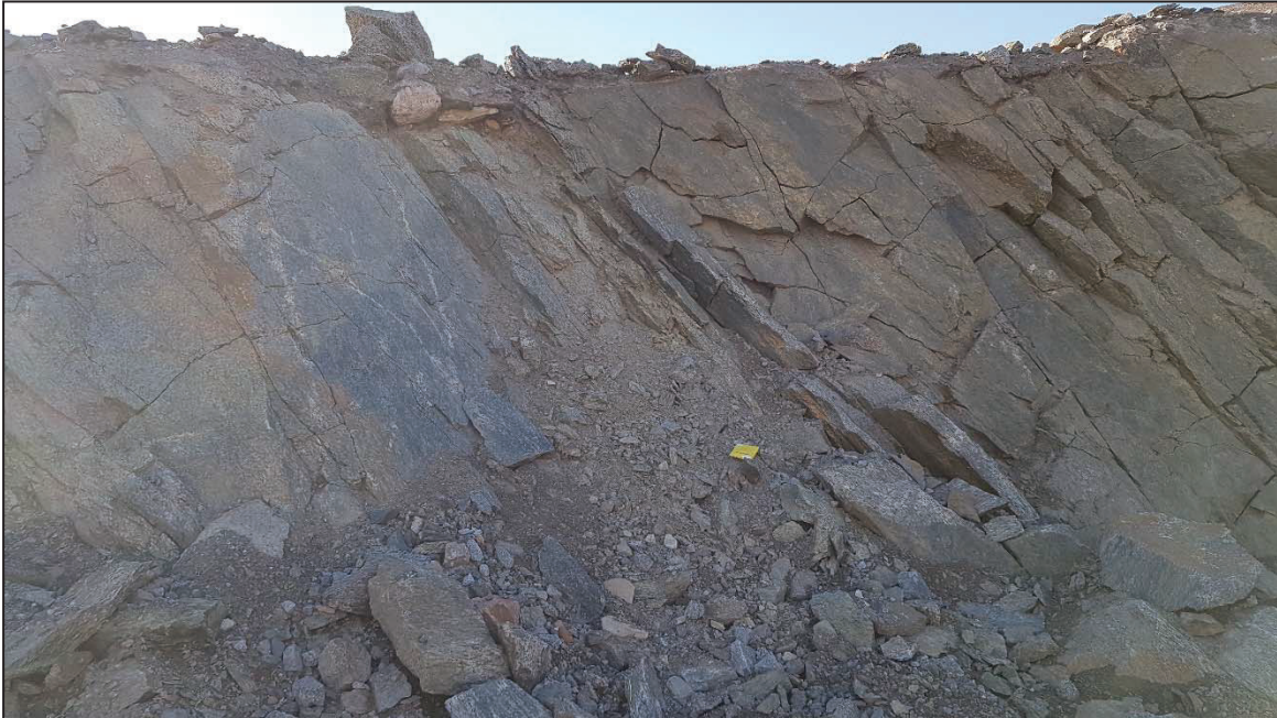
PHOTO 8 – Lower Quarry Area - Loose blocks at crest of wall
