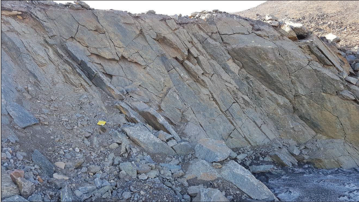
PHOTO 5 – Lower Quarry Area - Three main structural sets in north wall
