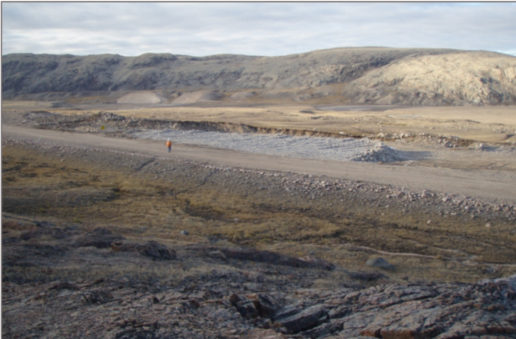
Photo 8: Borrow pit, sample pit @ 4km
