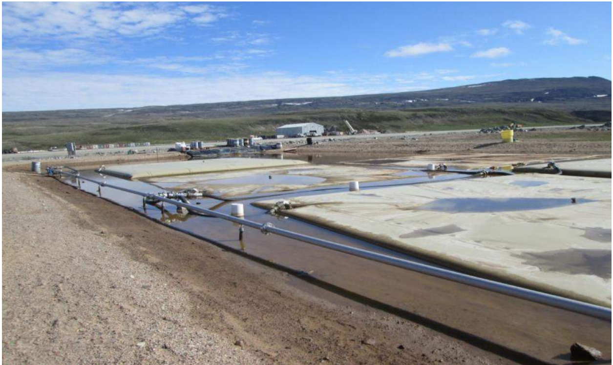
Bulk Fuel Storage Containment.
