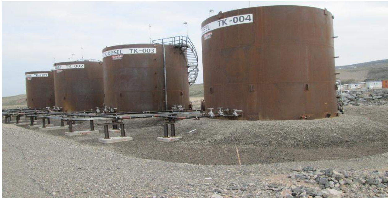
Minesite Steel Fuel Tank Farm Containment
