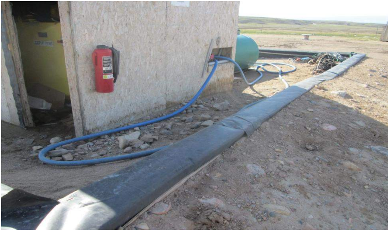
Helicopter Fuel Tank Containment.
