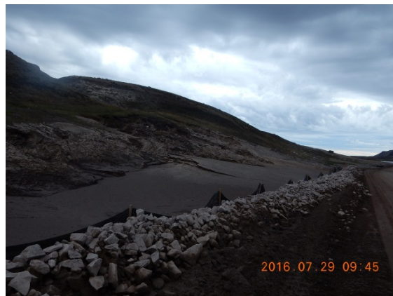
Figure 16: A View of a Problematic Section of the Tote Road. Ground sloughing – Sand/Silt Deposit with Steep Slopes
