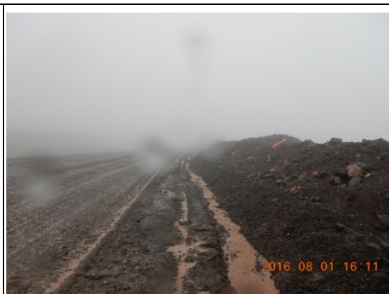
Figure 15: A View of the Drainage Along the Berm Side of Mine Haul Road
