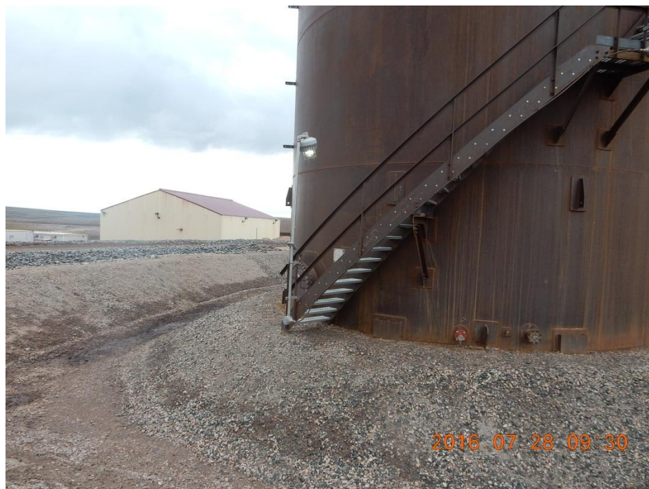
Photo 2: Typical Conditions of the Secondary Containment Base and the Dike
