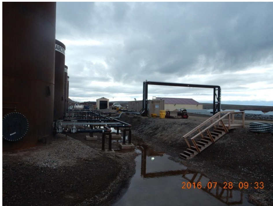
Photo 1: Bulk Fuel Storage Tank Farm Mine Site - Secondary Containment Dike
