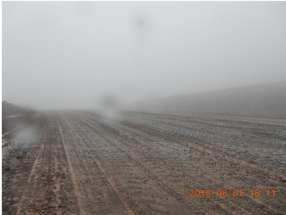
Photo 38: Mine Haul Road – During Rainfall Event
