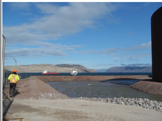
Figure 4: A view of the Milne Port Bulk Fuel Storage Facility's Secondary Containment Berm/Dam
