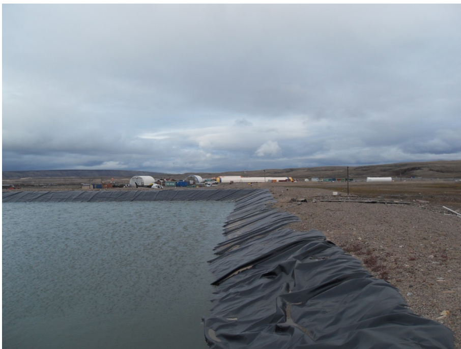
Photo 8: A close-up view of the exposed liner and embankment conditions of PSPW ponds at Mine Site
