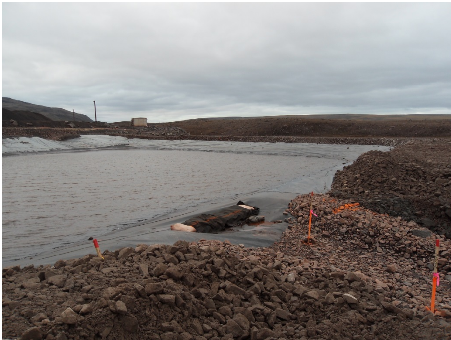
Photo 6: A view of the Emergency Spillway, Intake Channel to Sedimentation Pond and perimeter dam raising in progress associated with the Crusher Pad Area at Mine Site
