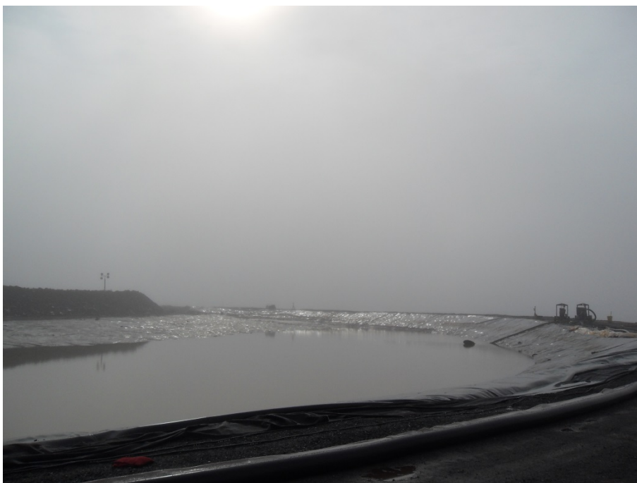
Photo 16: A view of the Mine Waste Rock Storage Facility collection pond liner and embankment/berm
