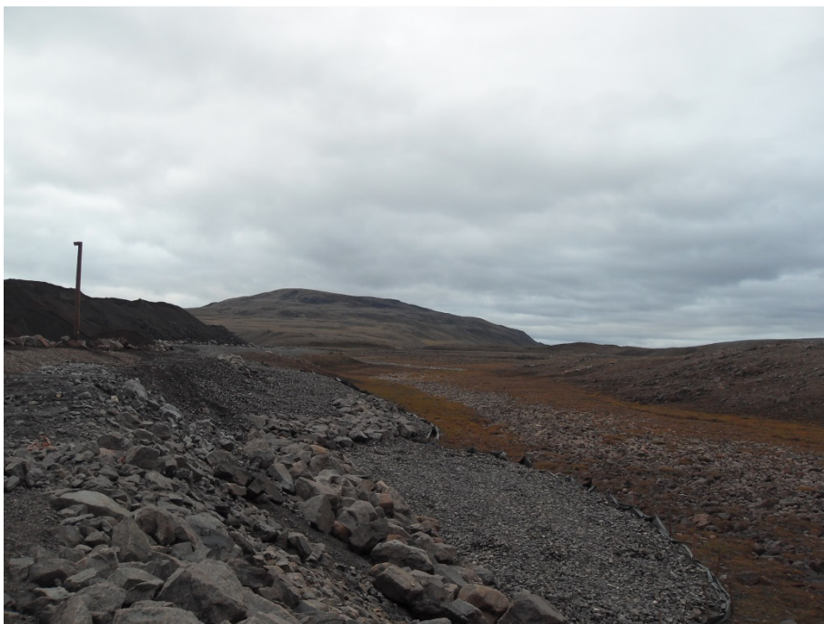
Photo 2: A view of the Crusher Pad expansion adjacent to an existing natural water course (potential for interferences with water course during an extreme flood)
