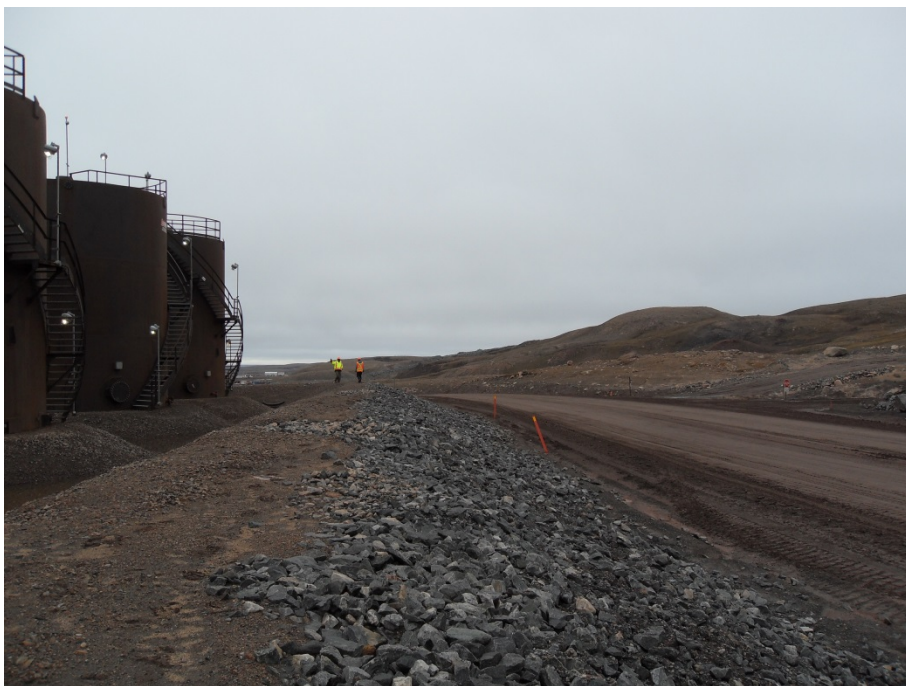
Photo 22: A view of the mine site Bulk Fuel Storage Facility – Perimeter Embankment
