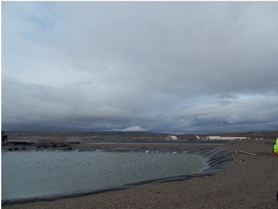
Photo 7: A view of the exposed liner on PSPW ponds at Mine Site
