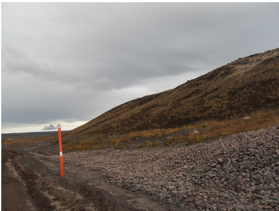
Photo 28: A view of the tote road slope improvement (granular fill slope protection)
