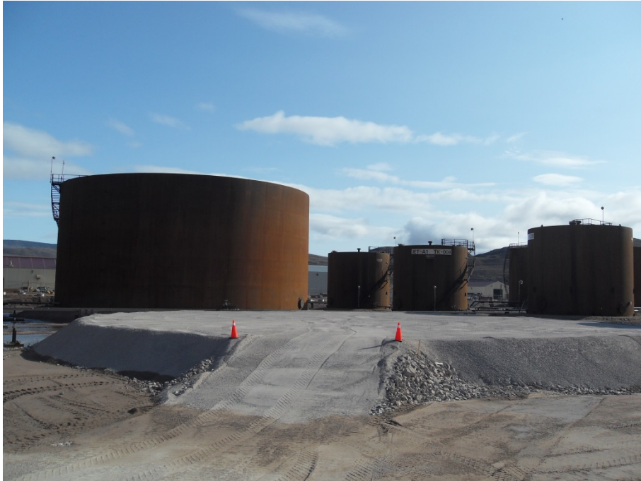
Photo 37: A view of the bulk fuel storage at port site – additional tank pad being constructed
