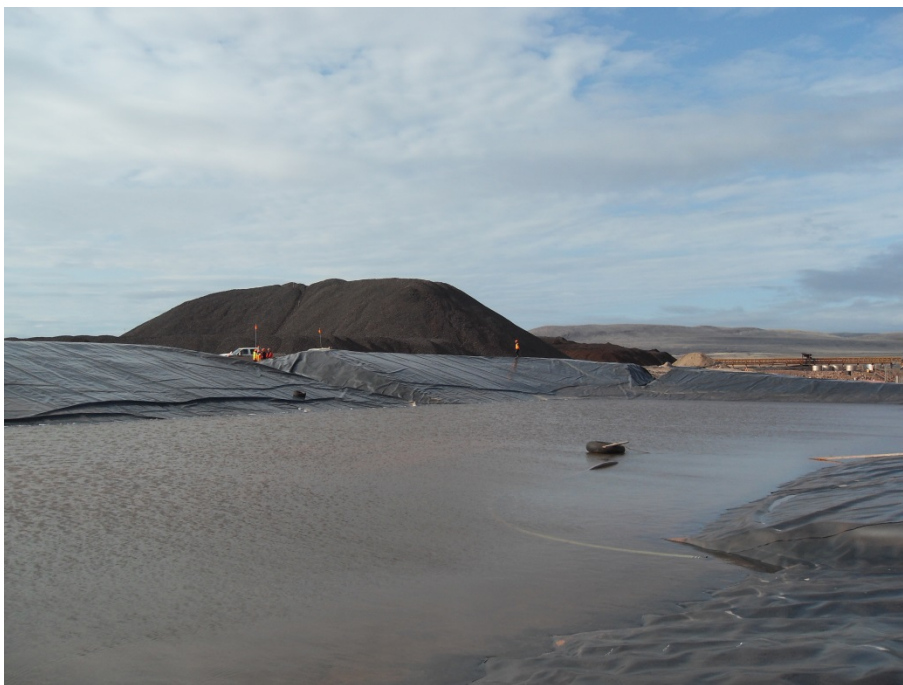
Photo 33: A view of the ore stockpile sedimentation pond (East Pond) showing liner conditions, water level and intake arrangements
