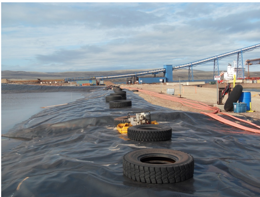
Photo 34: A view of the ore stockpile sedimentation pond (Esat Pond) showing emergency spillway section
