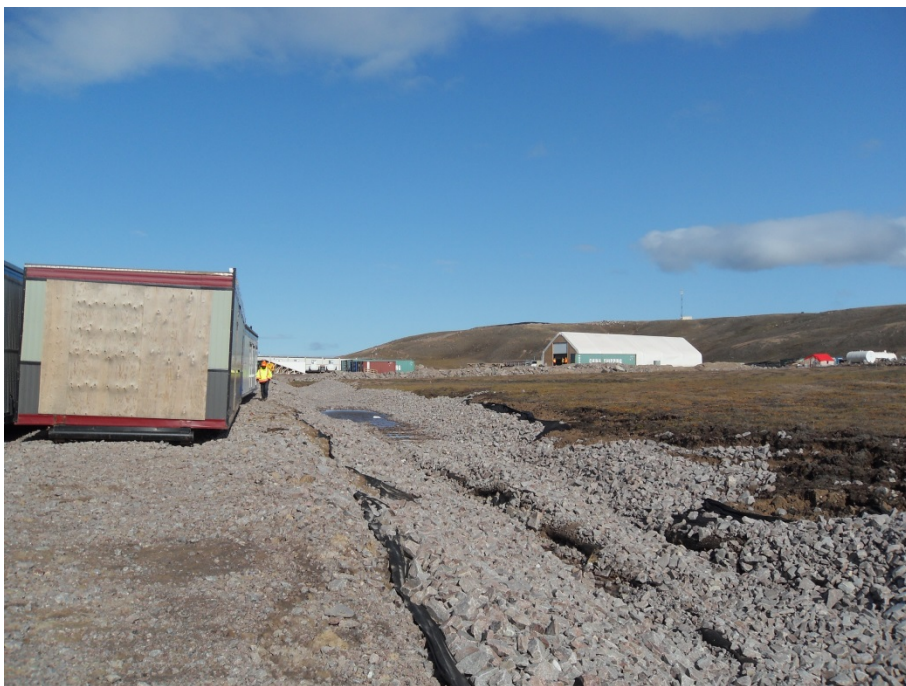
Photo 44: A view of the diversion drain at port site laydown area – local slogging
