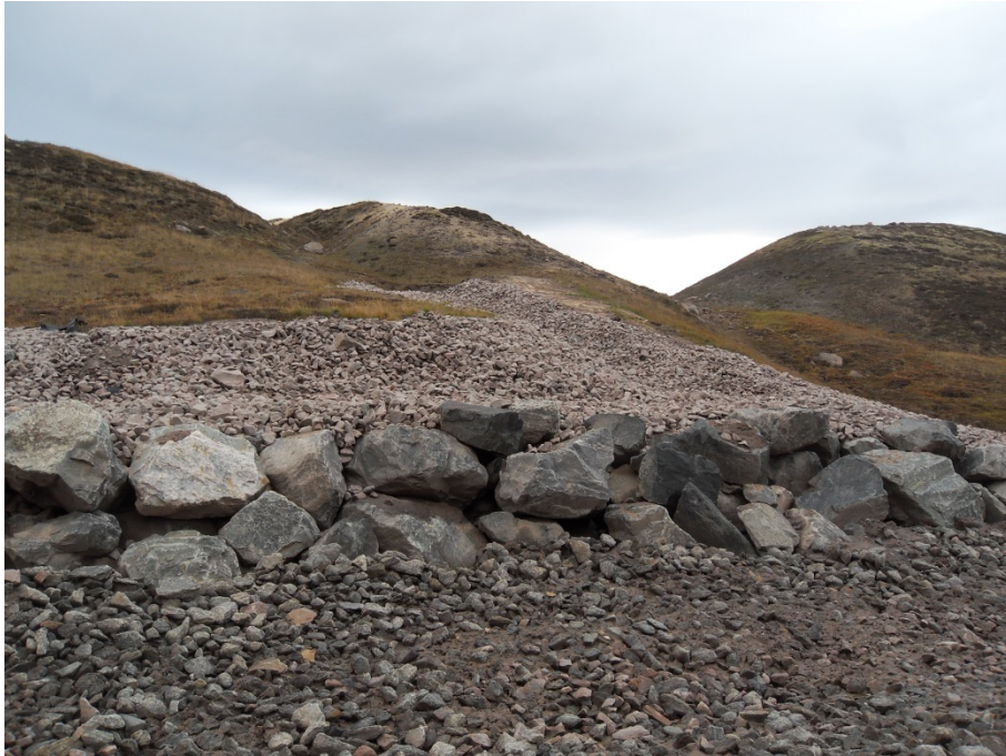
Photo 27: A view of the tote road slope improvement (Rockfill buttress)
