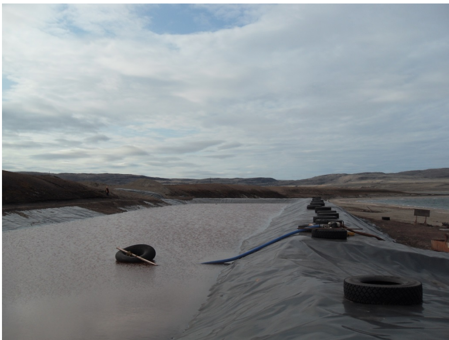
Photo 32: A view of the ore stockpile pond (West) – depressed section on right corner is emergency spillway
