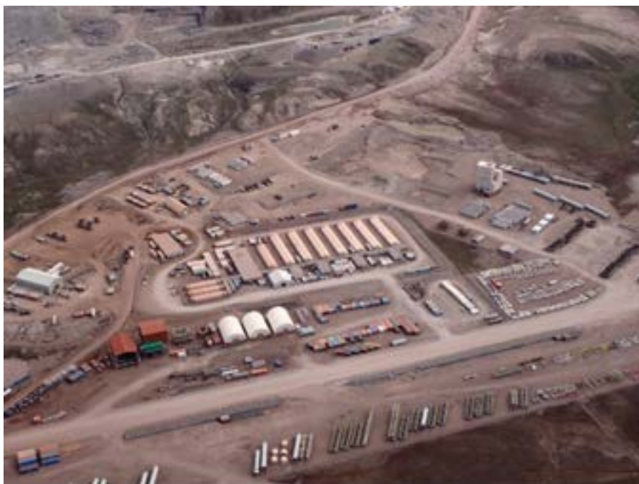
Aerial View of the 380 Person Camp (July 2023)
