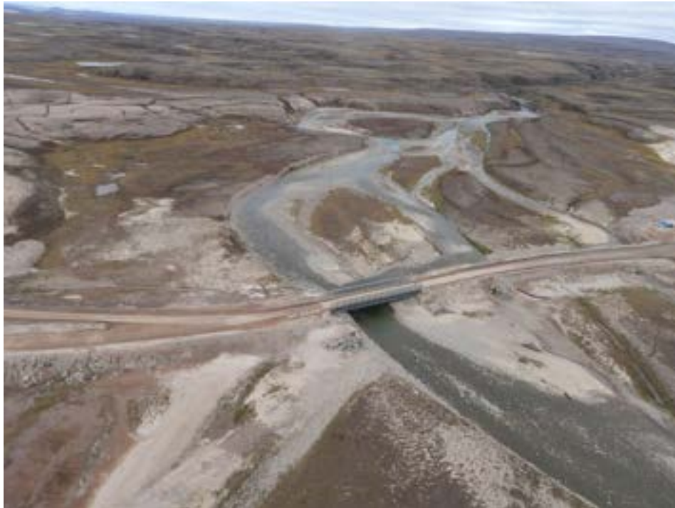
Aerial view of KM97 Bridge Crossing (August 2023)
