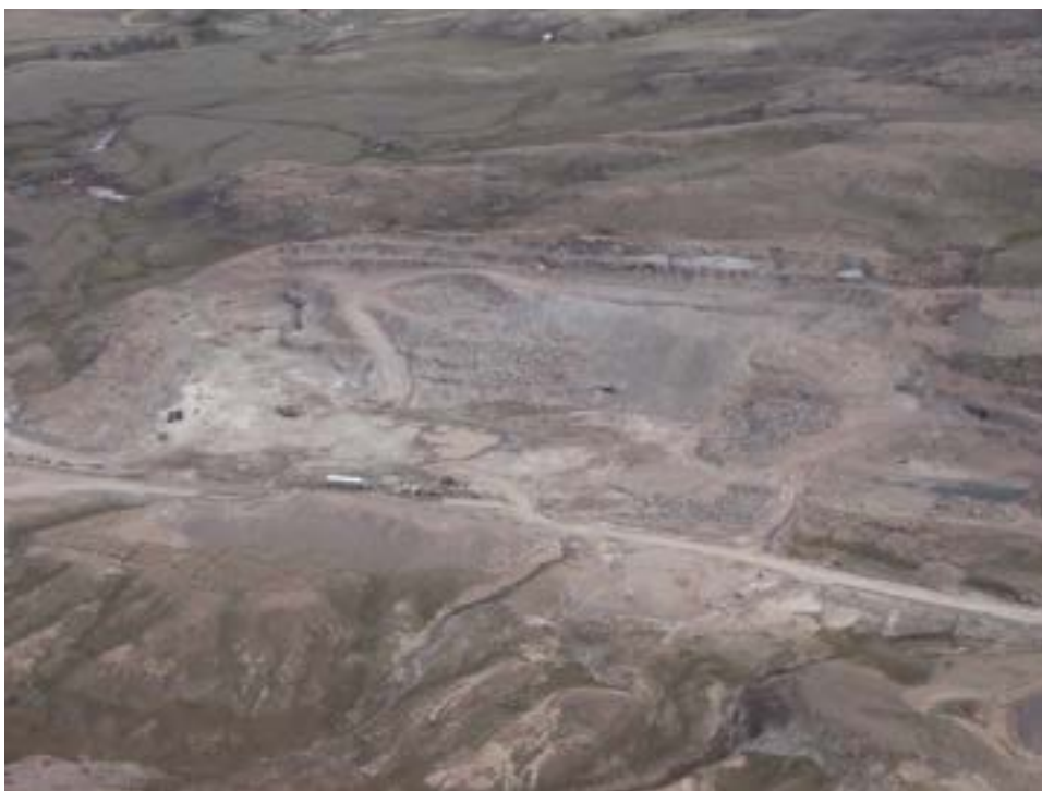
Aerial View of Quarry (Q1) (July 2023)
