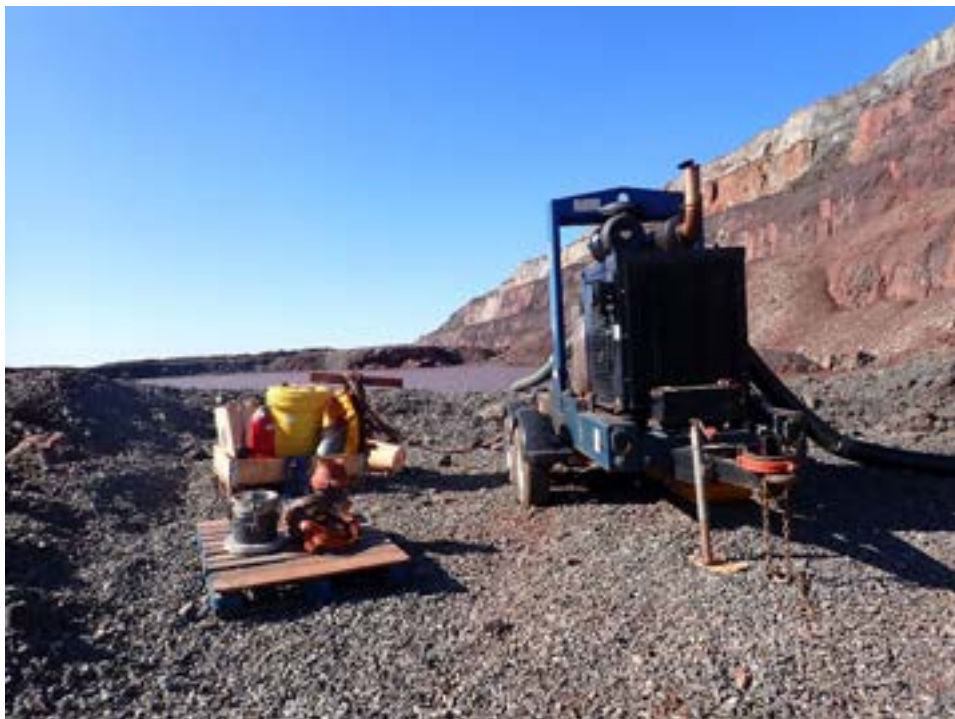
Water management at 570 Bench Laydown) (June 2023)
