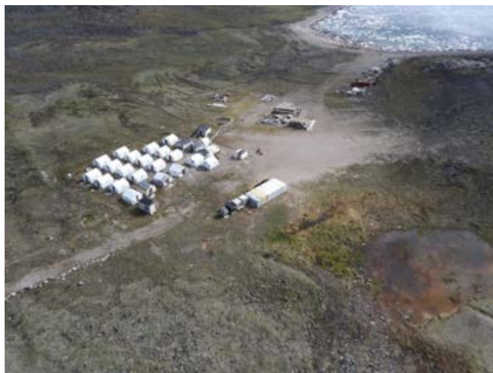
Aerial view of Steensby Camp – unoccupied (July 2023)
