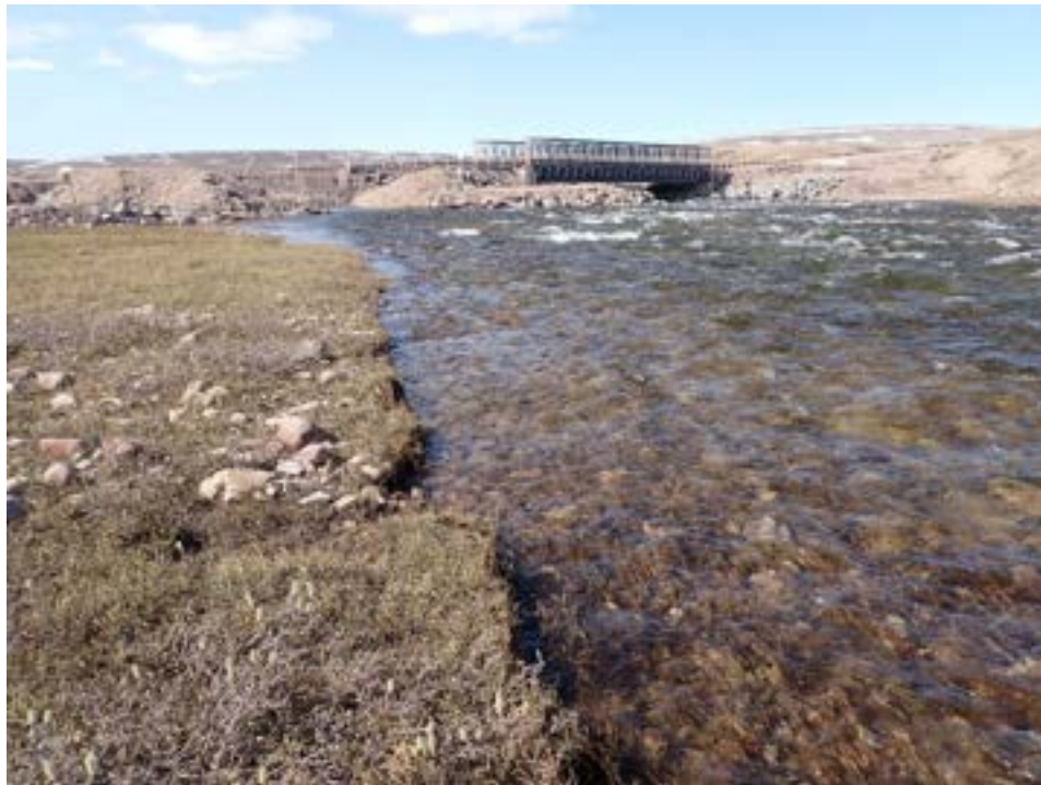
KM63 Bridge Crossing (July 2023)
