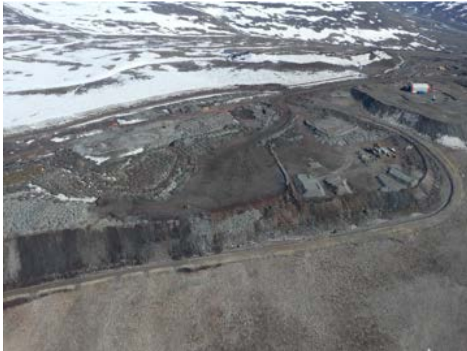
Aerial View of Waste Rock Facility (July 2023)
