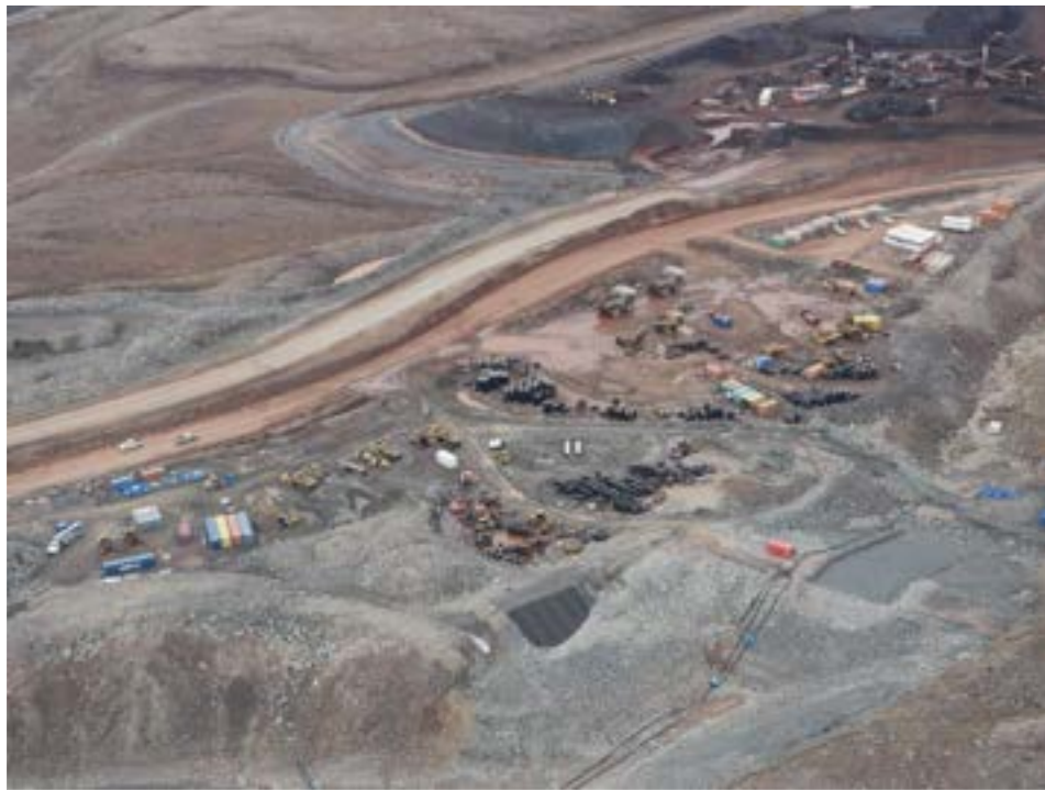
Aerial View of KM 104 Laydown (June 2023)
