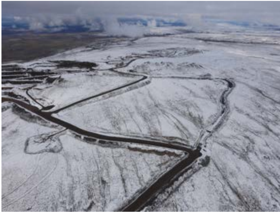
Aerial View of By-Pass Road (September 2023)
