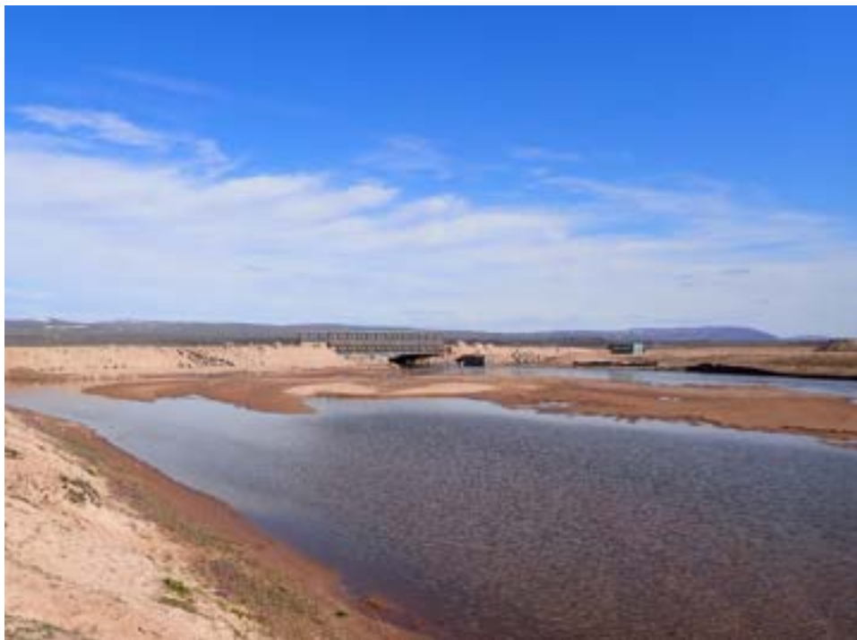
KM80 Bridge Crossing (July 2023)
