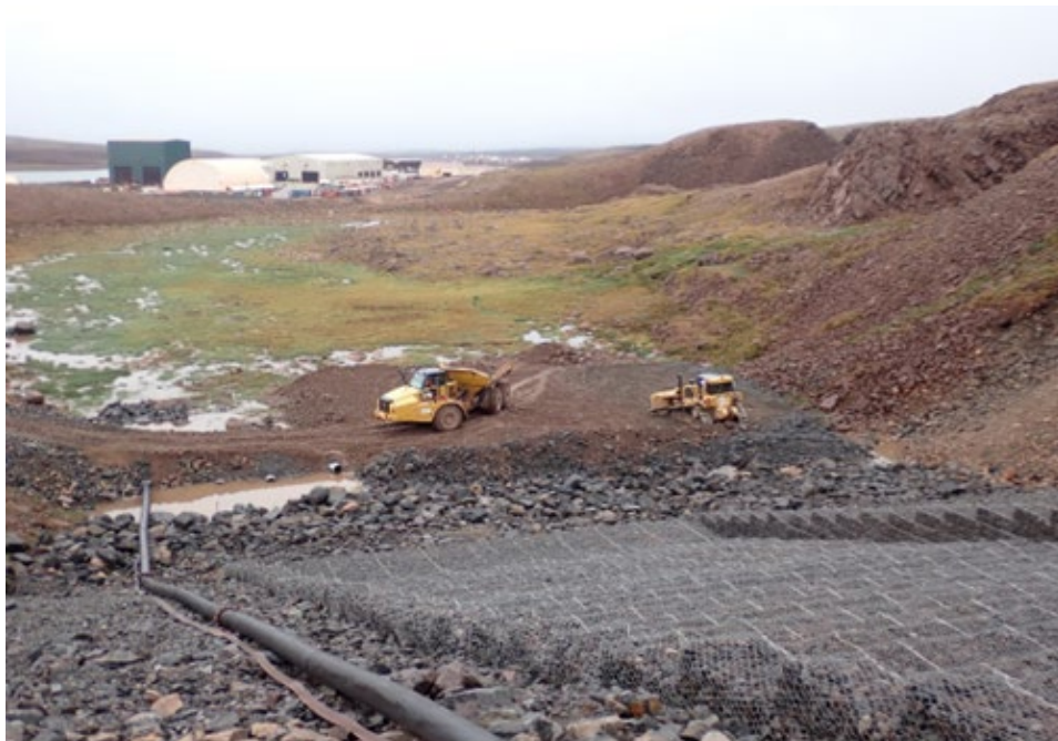
Construction of Geotube Pad at Mine Site KM105 Surface Water Management Pond (MS-11)) (August 2023)
