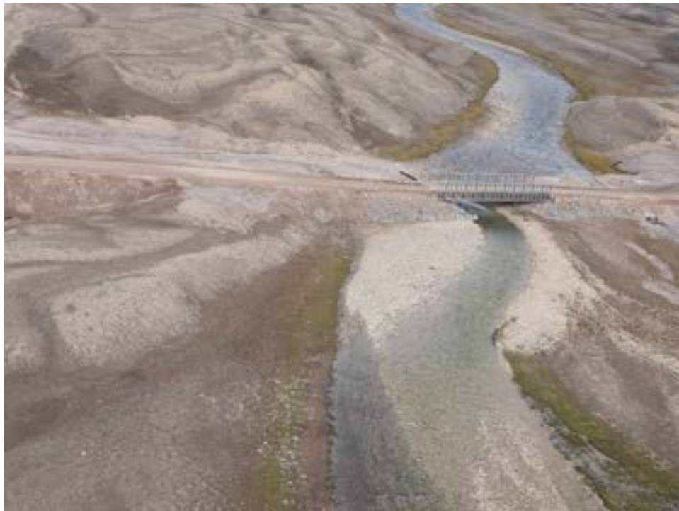
Aerial View of KM 63 Bridge (September 2023)
