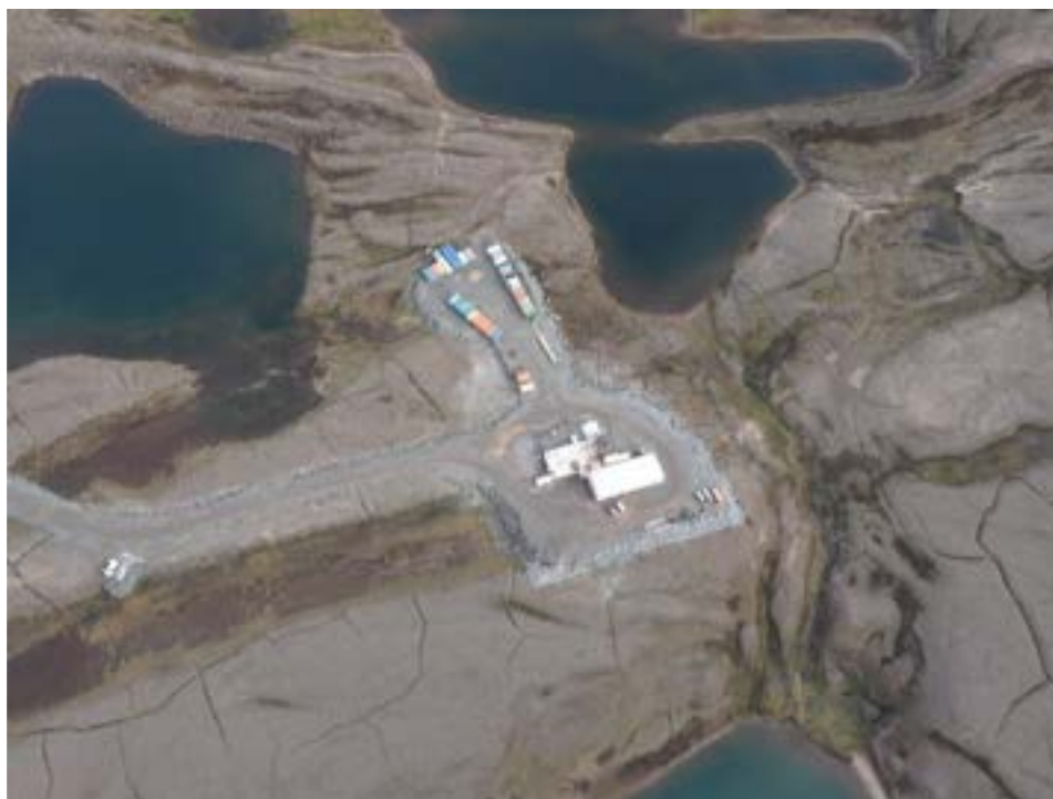
Aerial view of Emulsion Plant (September 2023)
