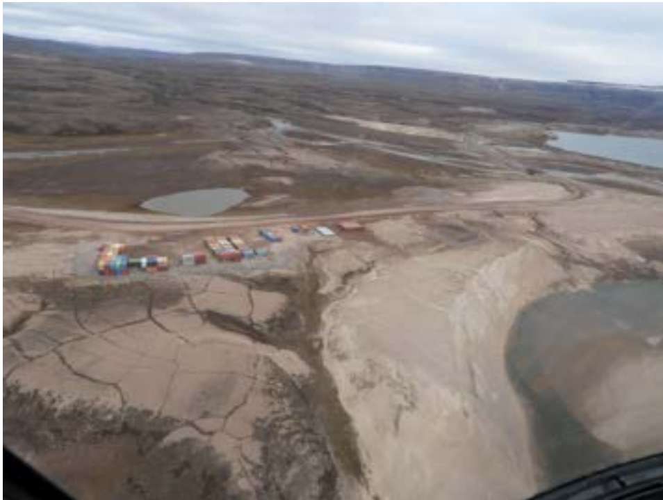
Aerial View of KM97 Laydown (September 2023)
