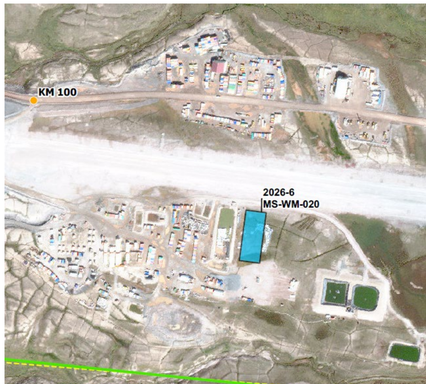
Figure 3. Mine Site Water Treatment Pond
