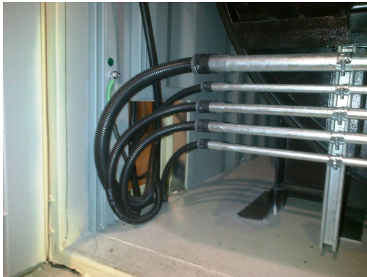
Flexible conduit in Container 2 (secondary chamber)
