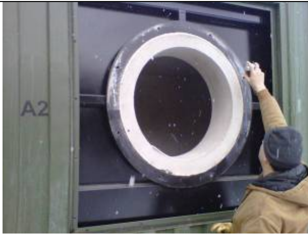
Gasket adhesive spray being applied
