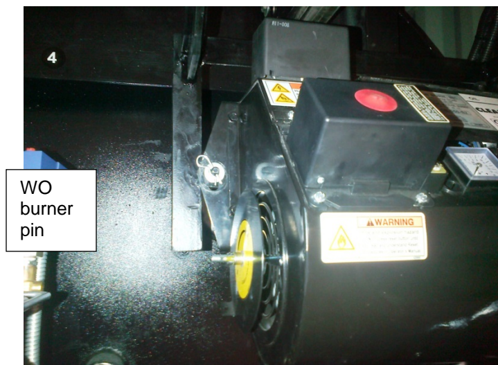
Waste oil burner secured with pin
