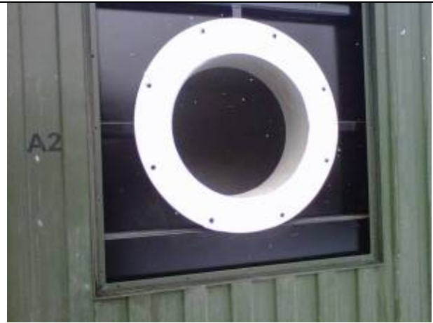
Correctly Installed Gasket
