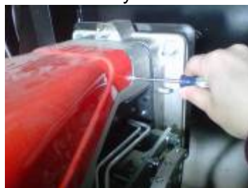
Secondary Burner has 4 screws (2 on each side)
