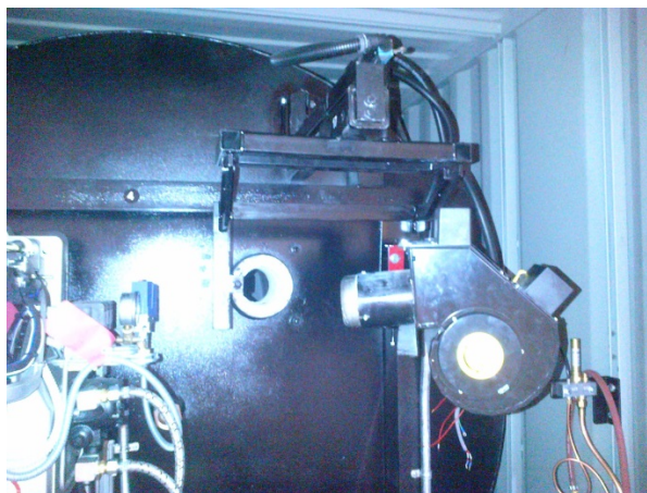
Swing the burner open
