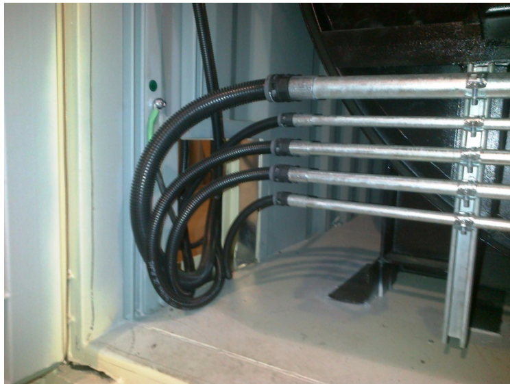
Flexible conduit in Container 2 (secondary chamber)
