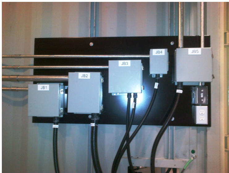
Junction Boxes in container 3 (control container)
