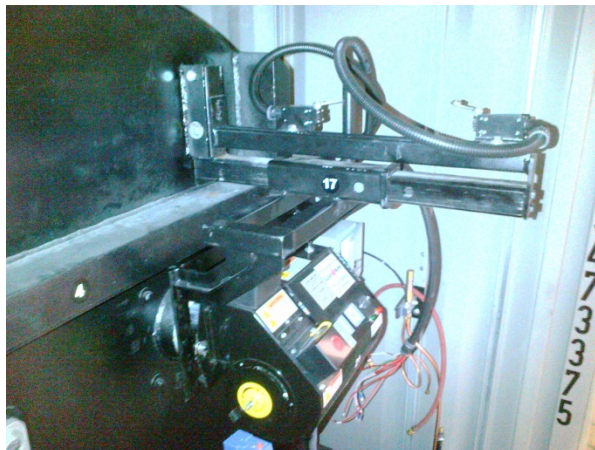
Swing the burner close, secure with pin and push all the way in until front limit switch is made
