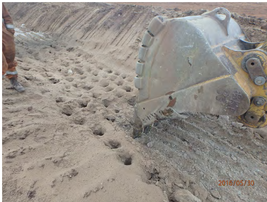
Figure 7: Excavator Bucket Ripping Pre Drilled Permafrost
