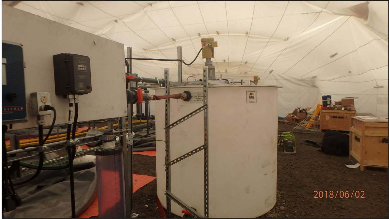
Figure 13 - Installation of Lime Mixing Station and controls
