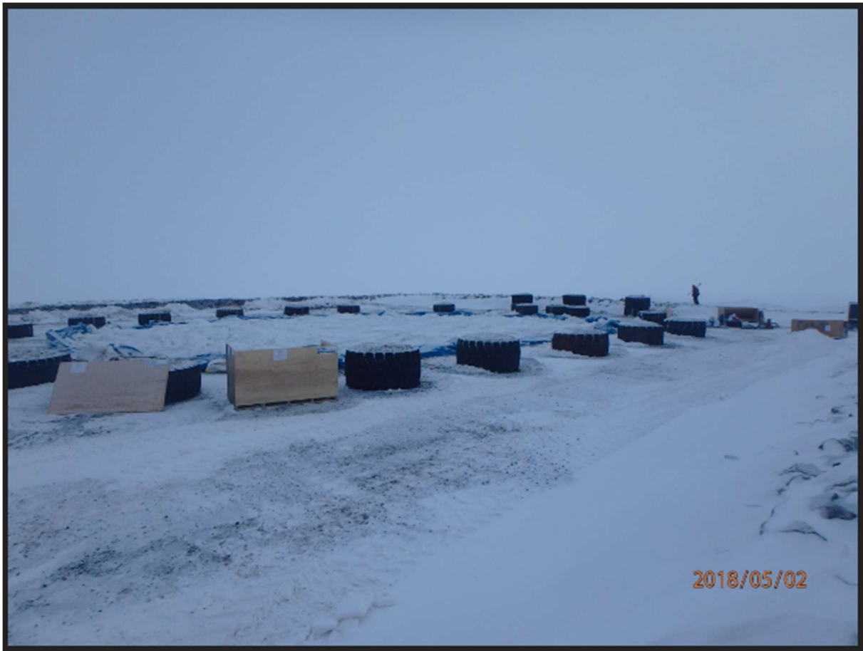
Figure 5 - Outside tire anchors for WTP building construction
