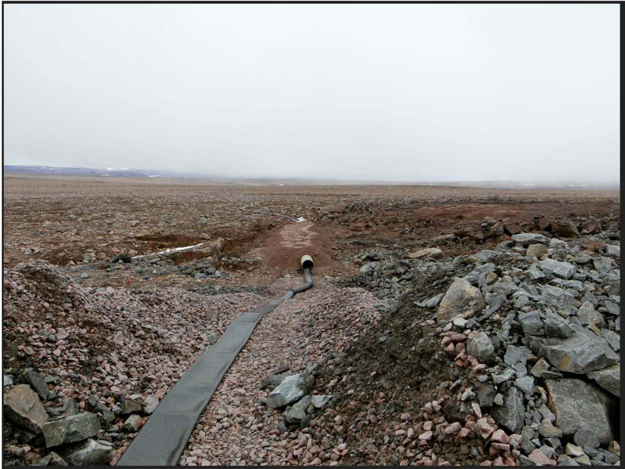
Figure 19 – WTP Discharge line out of discharge pump behind WTP, entering the tundra
