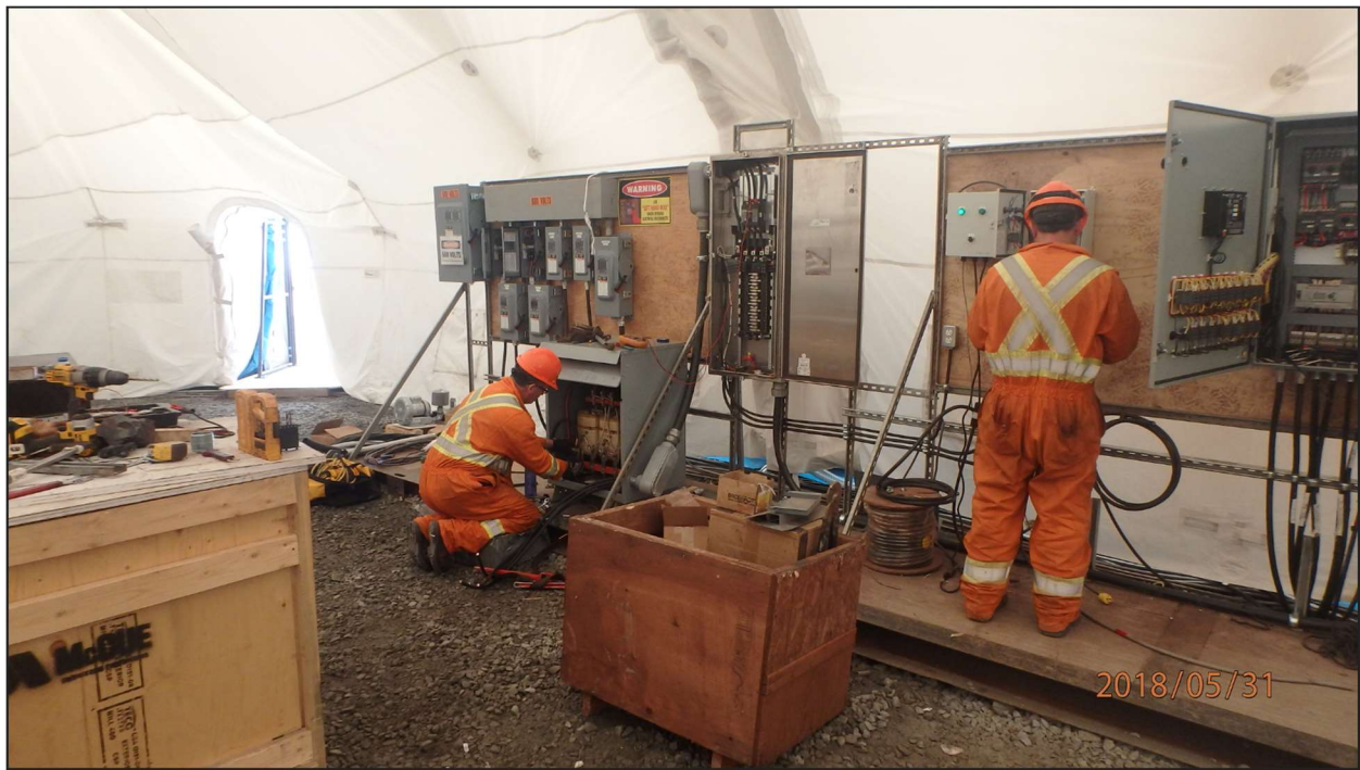
Figure 11 – Assembling power distribution and control panels.
