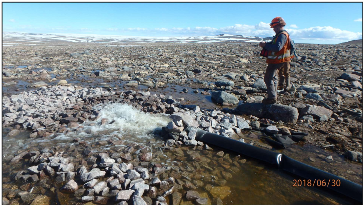
Figure 21 - WTP Discharge line end of pipe
