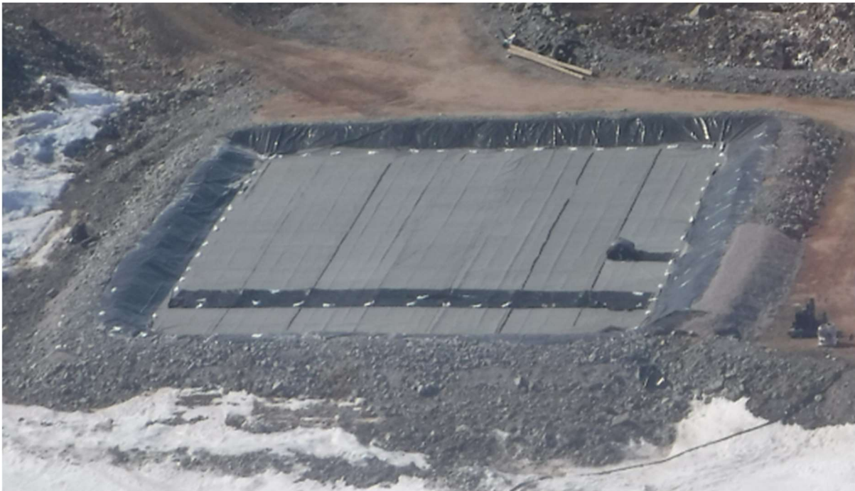
Figure 17 –Placement of geotubes in Geotube pond
