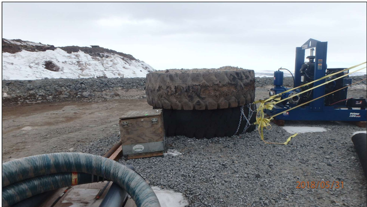
Figure 9 - WTP building outside tire anchors
