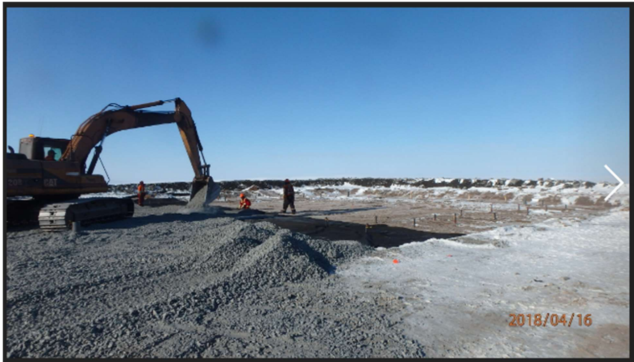
Figure 3 – Placement of geotextile material at the bottom of WTP and covering with \frac{3}{4} " minus rockfill
