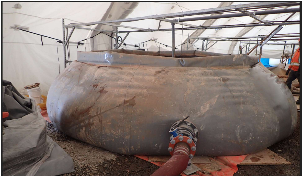
Figure 22 – Ferric Process Tank under construction
