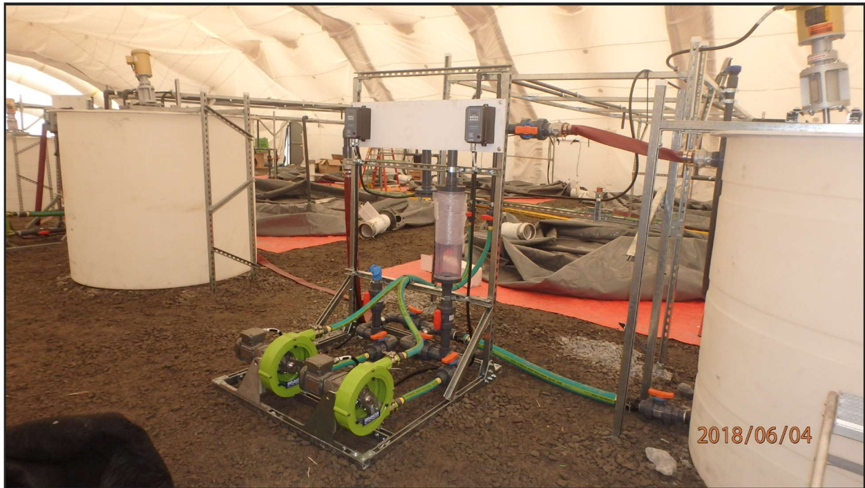
Figure 15 - Installation of Lime and Polymer Mixing Stations and controls
