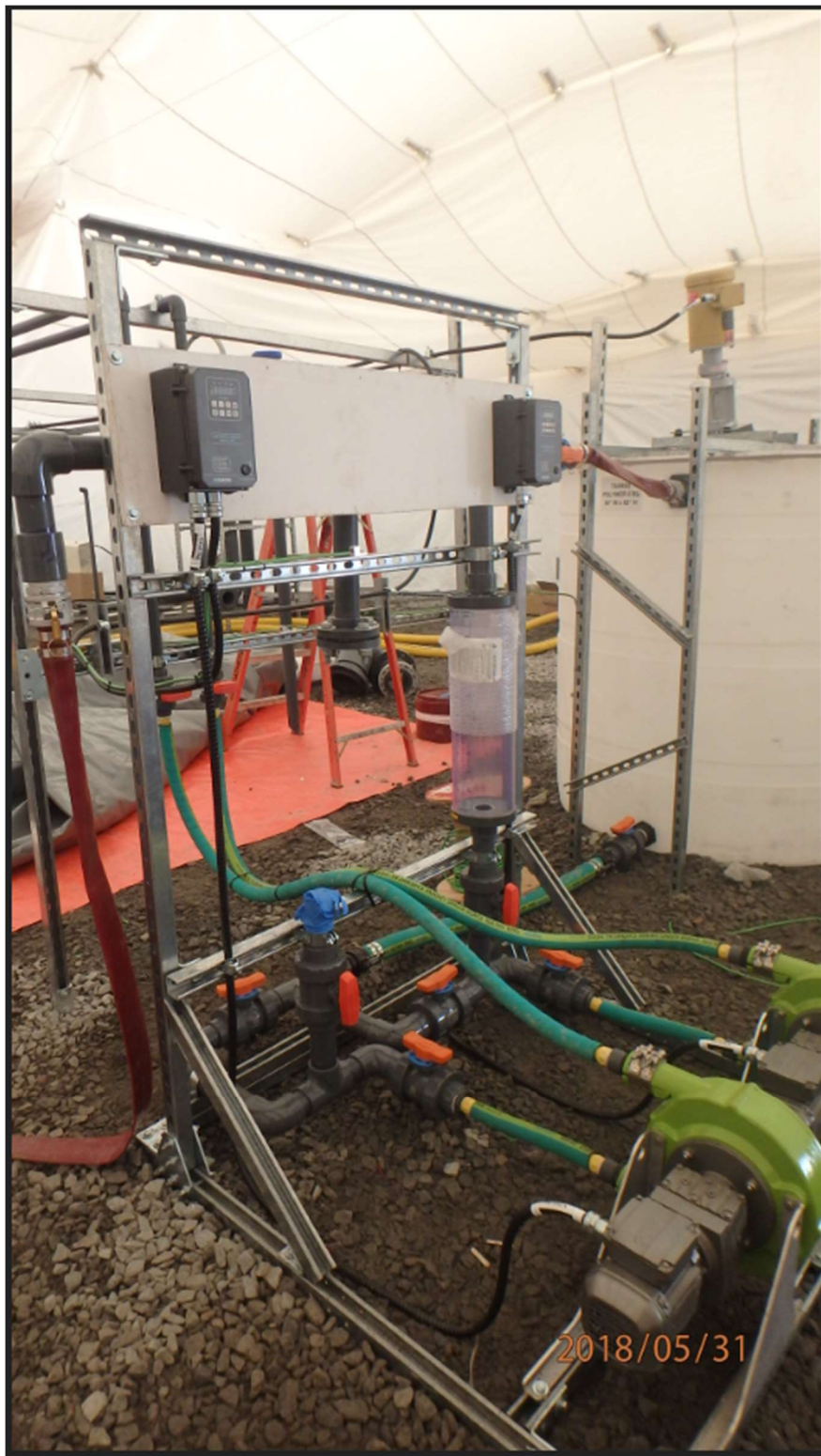
Figure 14 - Installation of Polymer Mixing Station and controls
