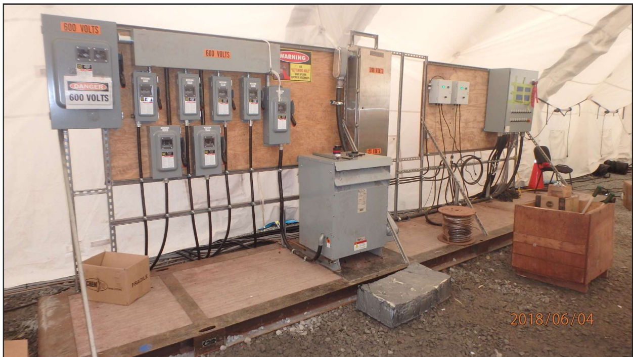
Figure 12 – Power distribution and control panels assembled.
