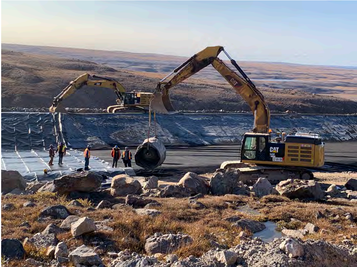
Deploying 2 nd Liner Panel - 6Sep20
