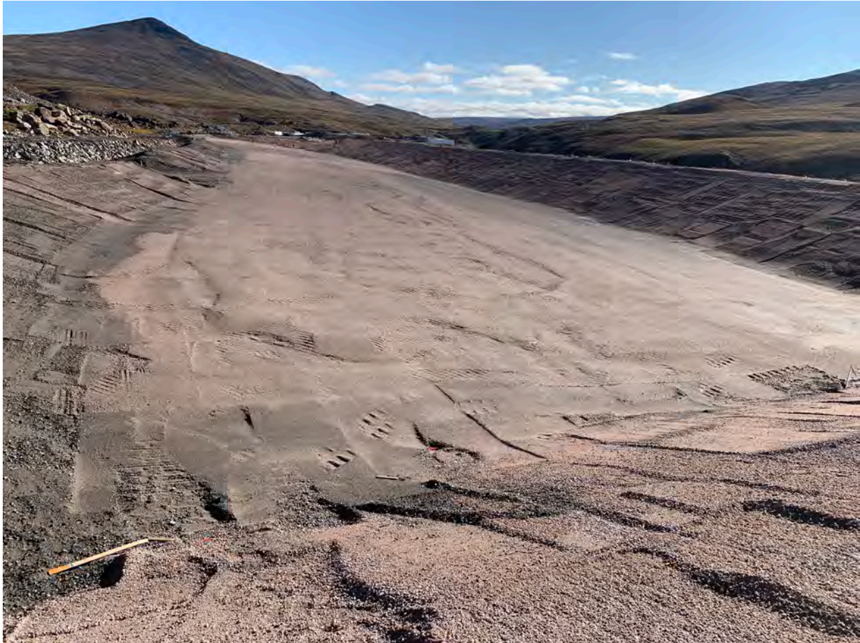
Placement of Intermediate Bedding - 20Aug20
