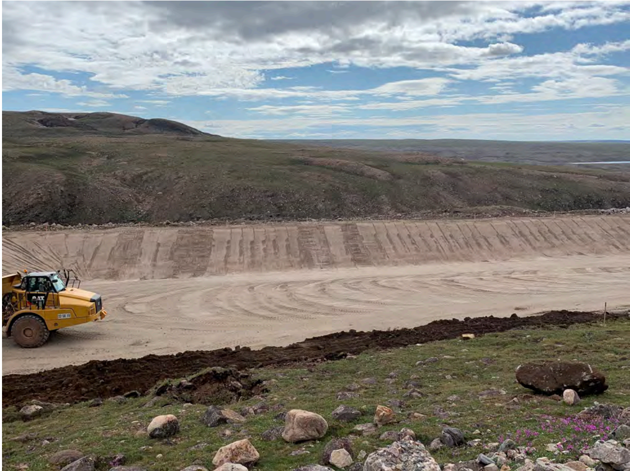
Preparing North Liner Anchoring - 21Jul20
