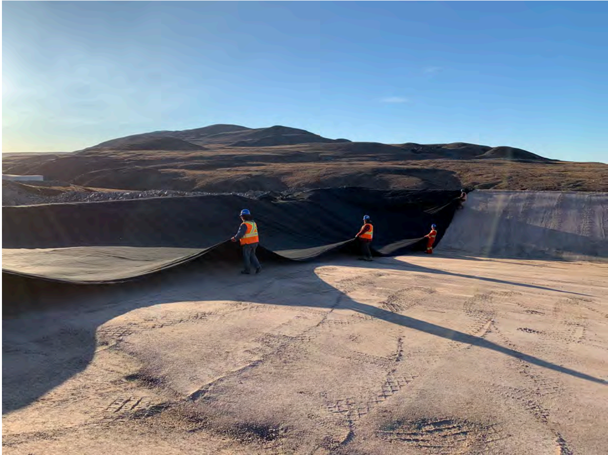
Deploying Geotextile Fabric - 5Sep20
