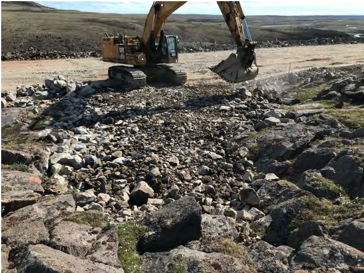
Filling in a Crevice with ROQ and 150mm minus – 7Jul20
