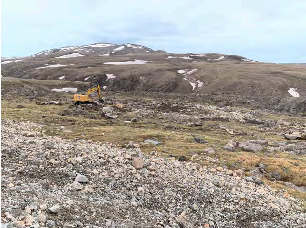
Prepare Foundation – Removal of Large Boulders - 27Jun20
