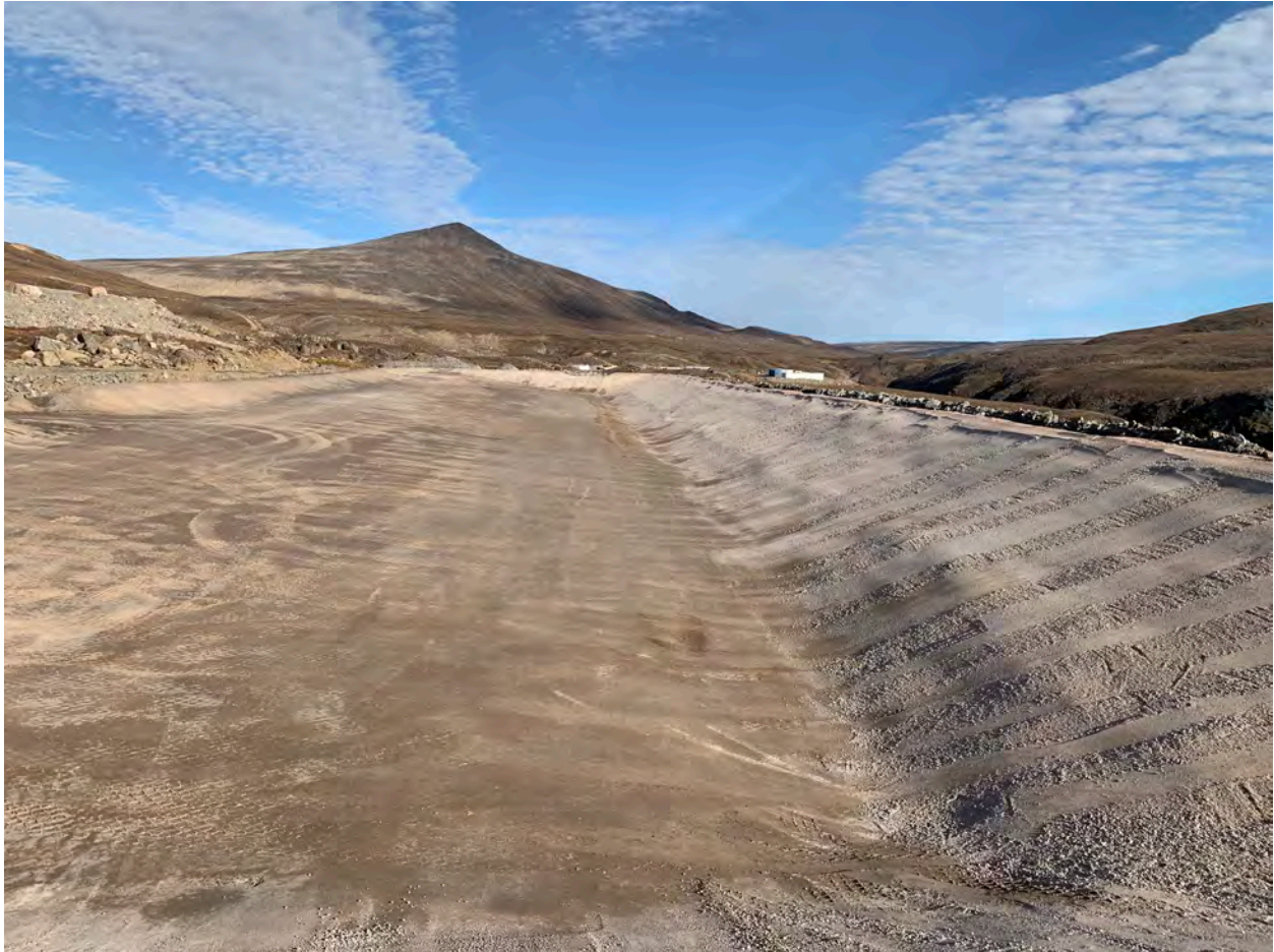
Completed Intermediate Bedding on Pond Bottom - 2Sep20
