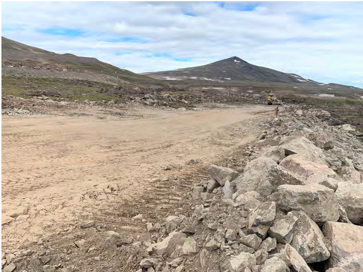
Top of 4 th Layer of ROQ on Berm - 5Jul20
