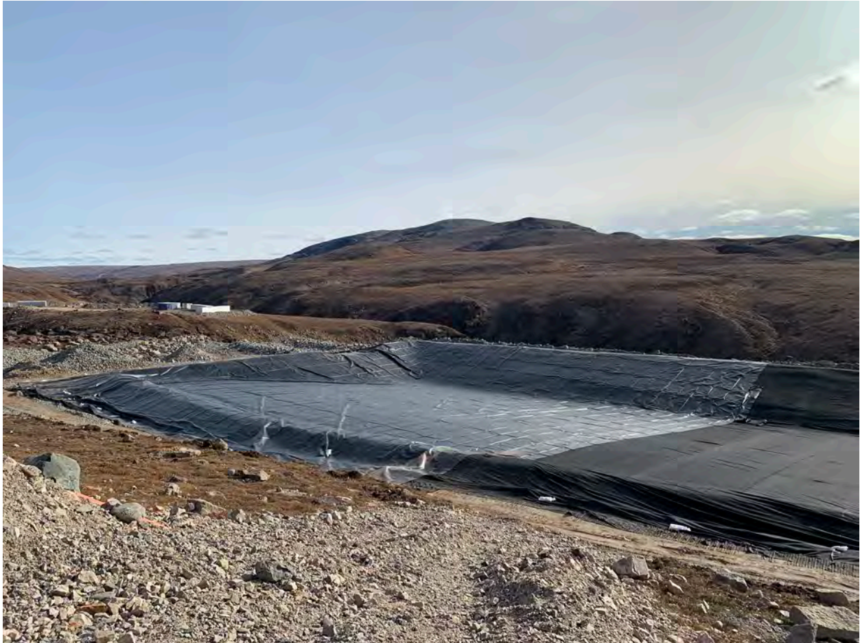
Deploying 1 st Liner Panel - 5Sep20
