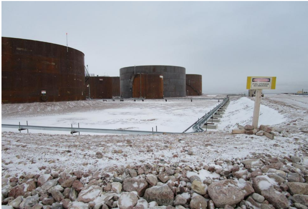
Fuel tank farm containment
