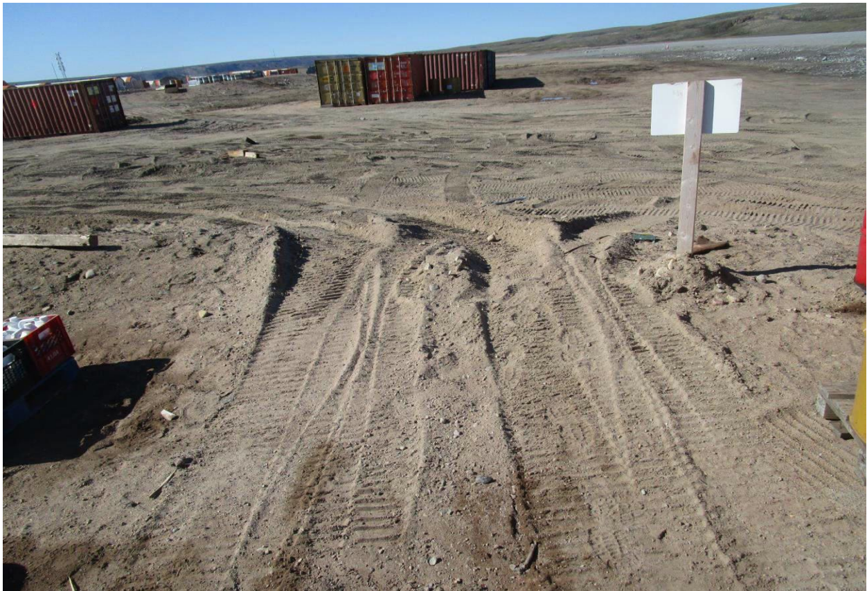
Barrel Fuel Containment – Shows travel over side dyke of cell. (Now MP-HWB-3)
