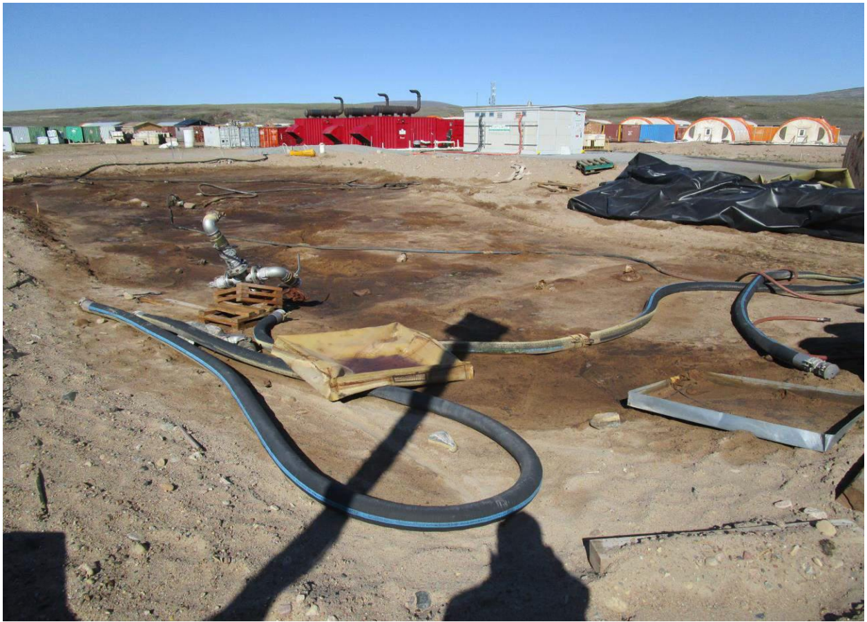
Generator Fuel Containment in process of decommissioning.
