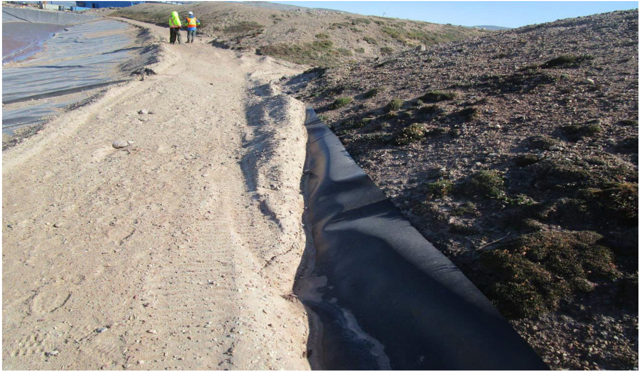
West Settling Pond – “Tuck-in” liner this location.
