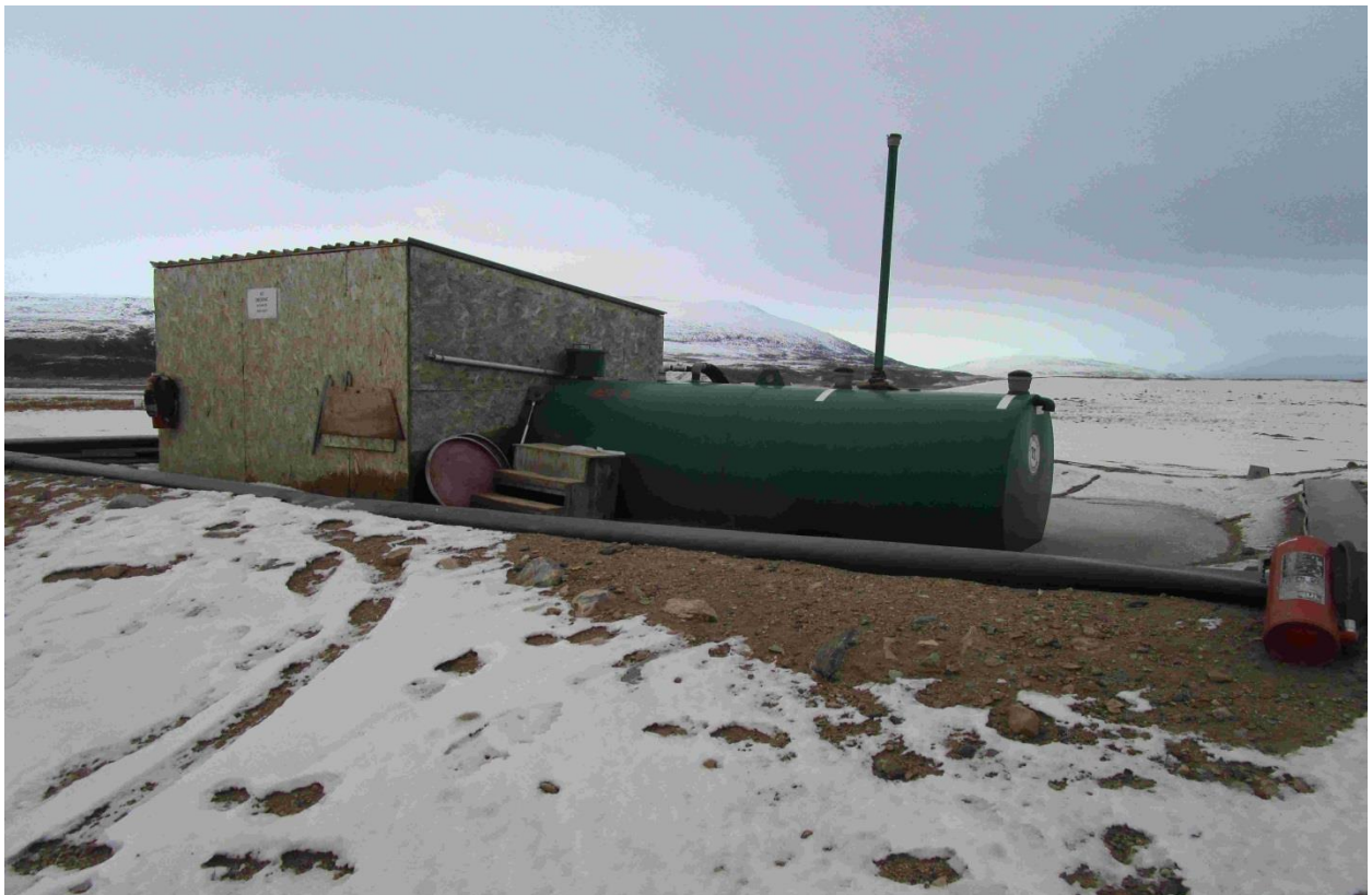
Helicopter Fuel Tank Containment
