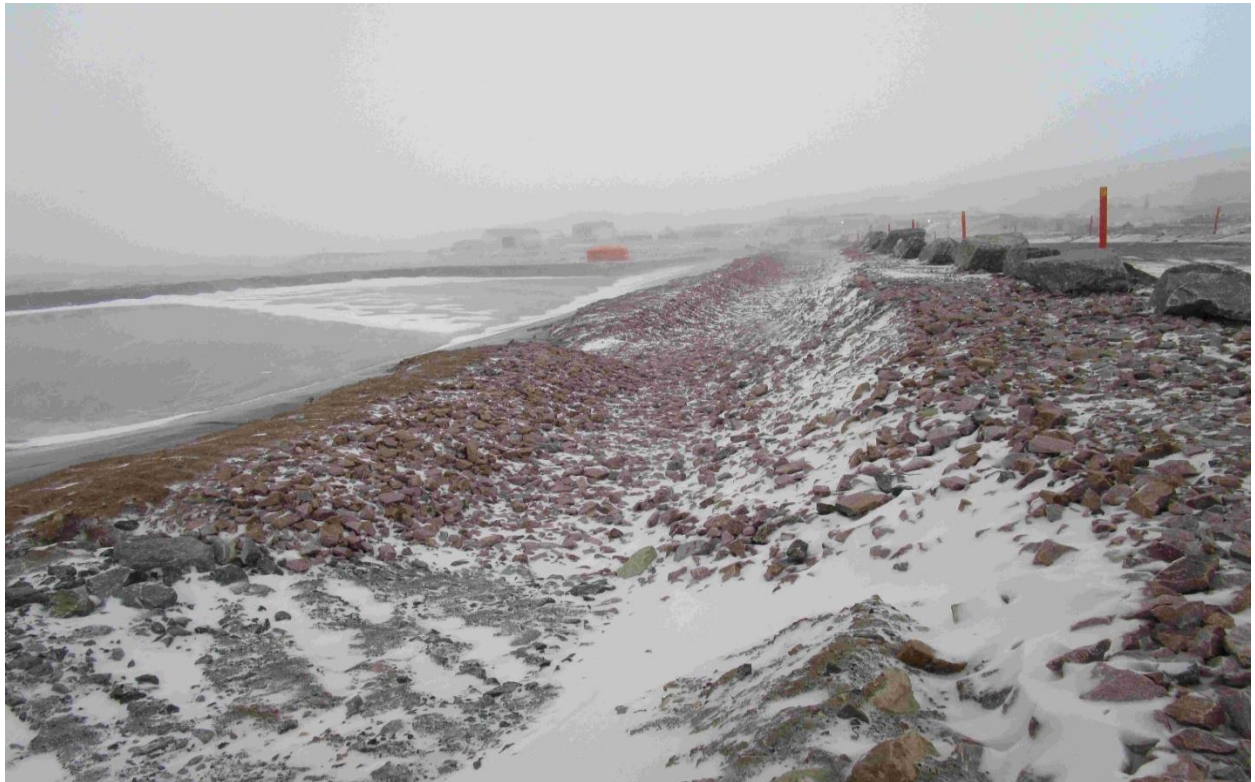
Crusher Pad Drainage Pond and Swale
