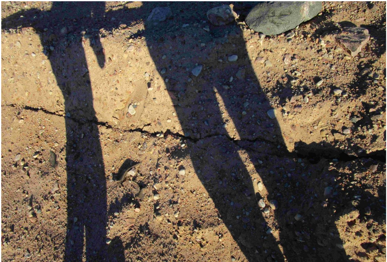
Indicates Movement in Anchorage at Sediment Pond East
