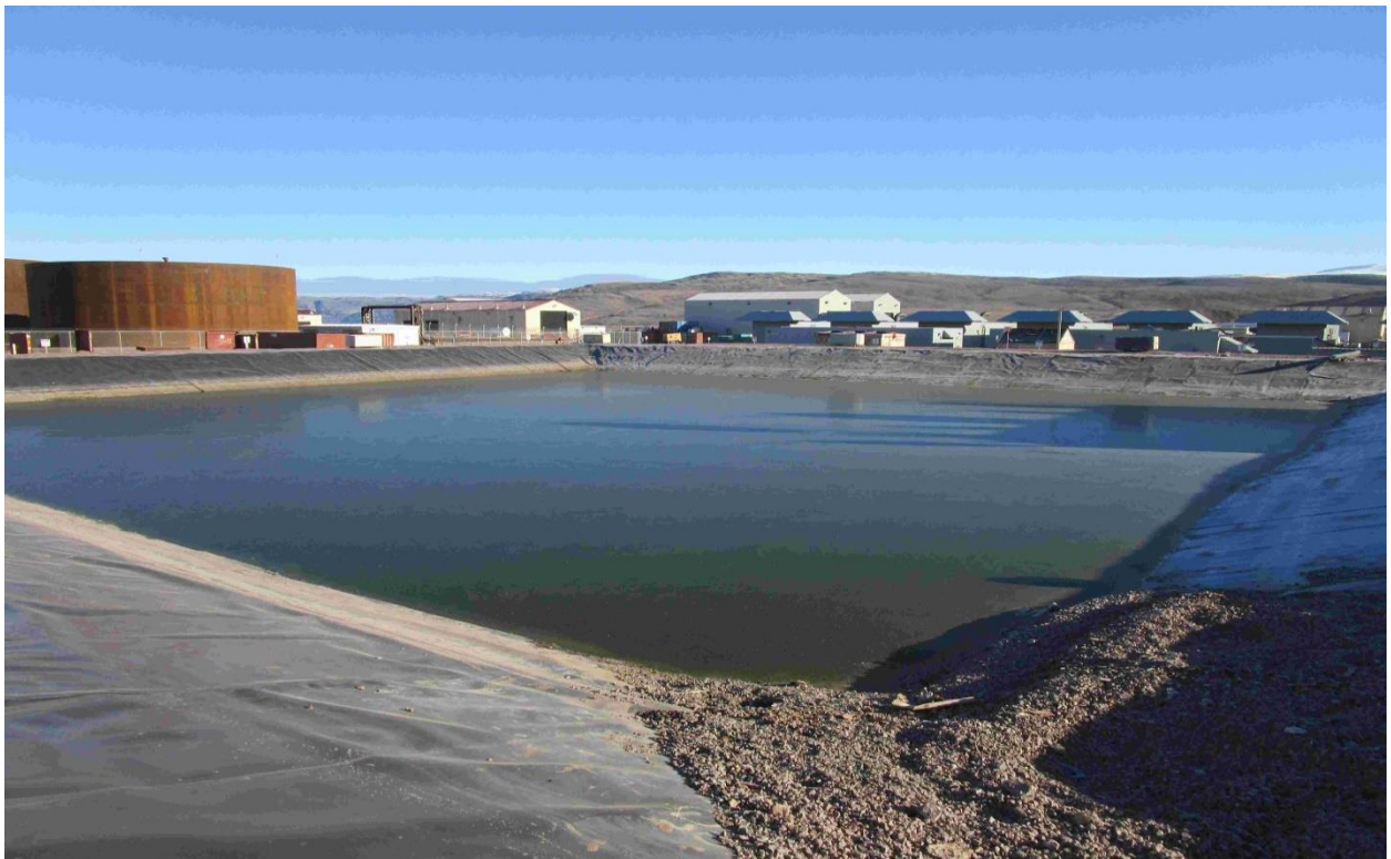
Polishing Waste Stabilization Pond
