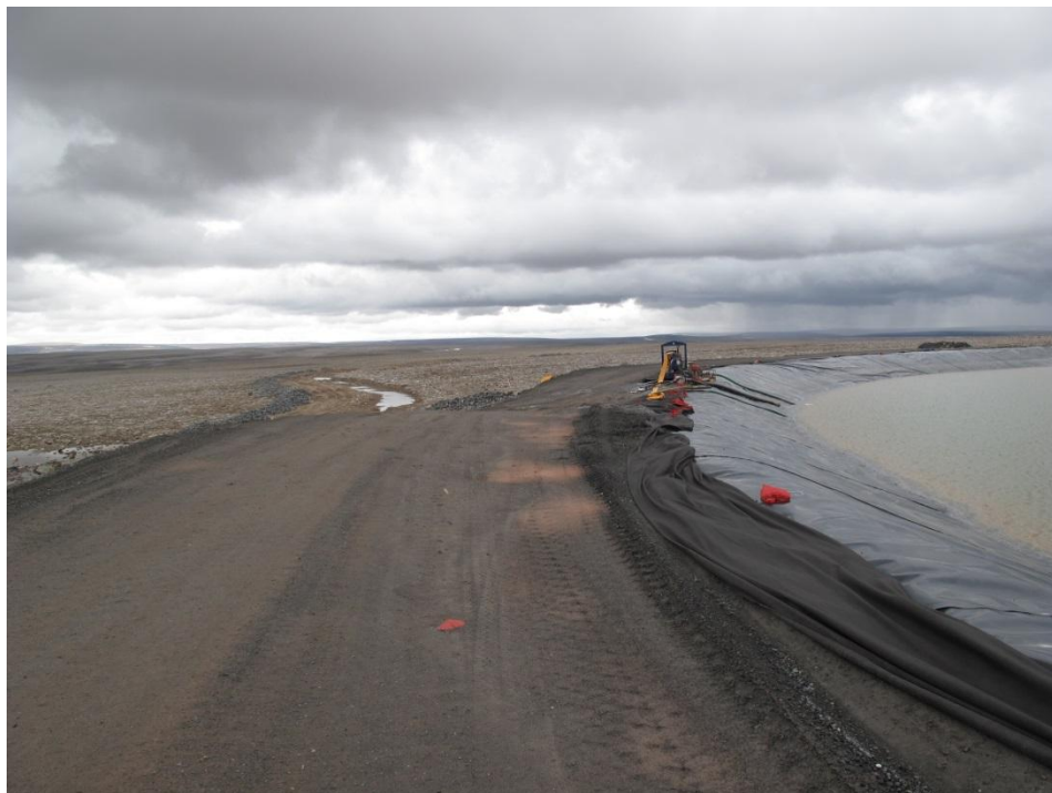
Photo 23: Mine Waste Rock Settling Pond – Dike and Pumping System for Discharge
