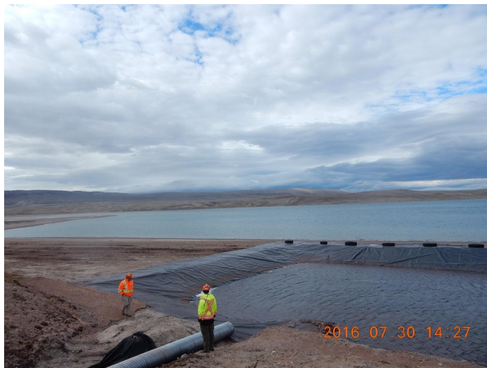
Photo 21: A close-up of Inlet to Sedimentation Pond (West) Port Area
