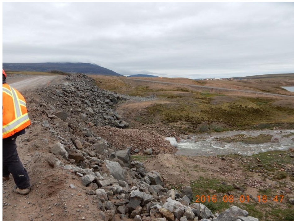
Photo 41: Tote Road Typical Drainage Crossing Culvert – During Rainfall Event
