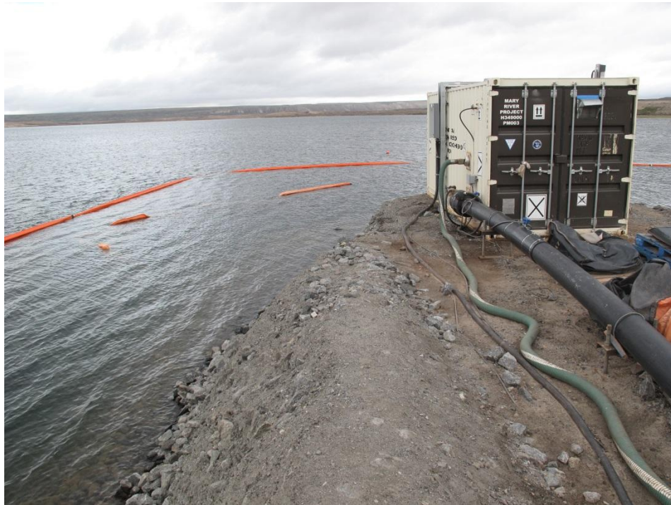
Photo 42: Raw Water Intake Jetty Head Requires Upgrade for Wave/Erosion Protection
