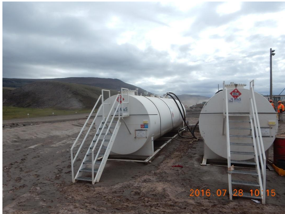
Photo 3: Mine Site Jet Fuel Storage Tank Farm Secondary Containment
