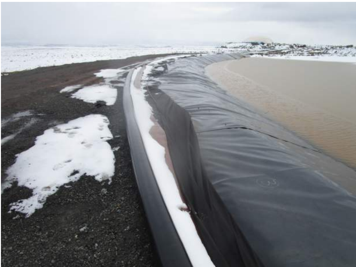
16. Waste Pile Drainage Containment
