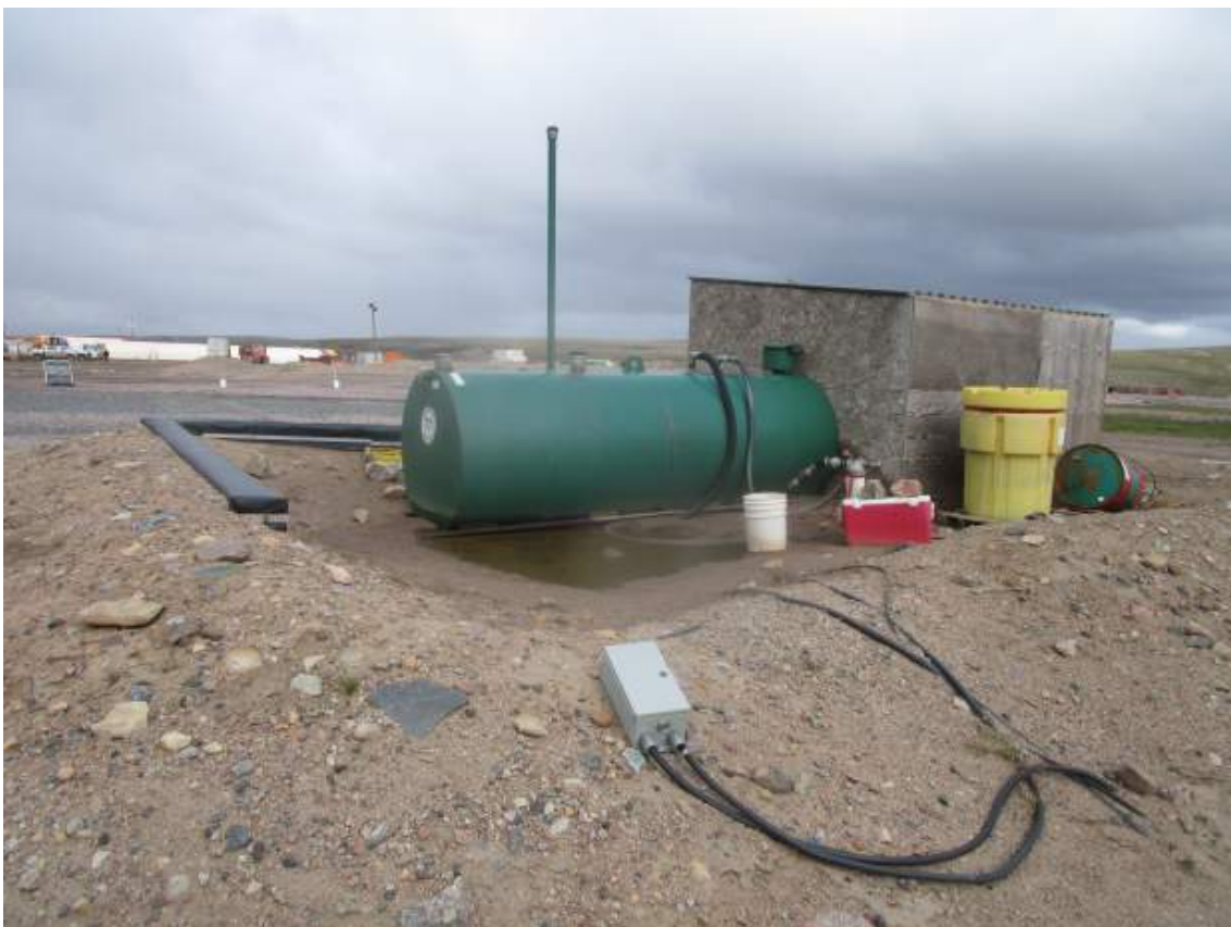
6. Helicopter Fuel Cell Containment
