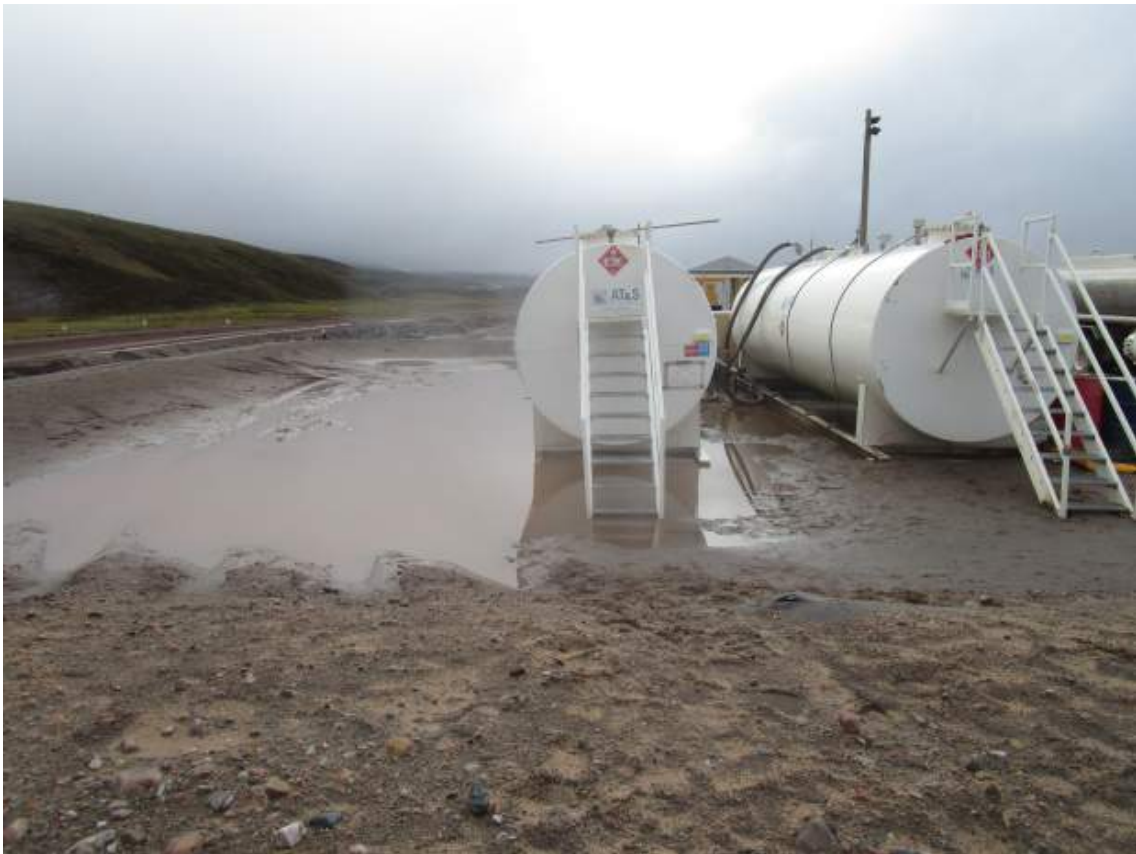
11. Jet Fuel Pump and Tank Containment
