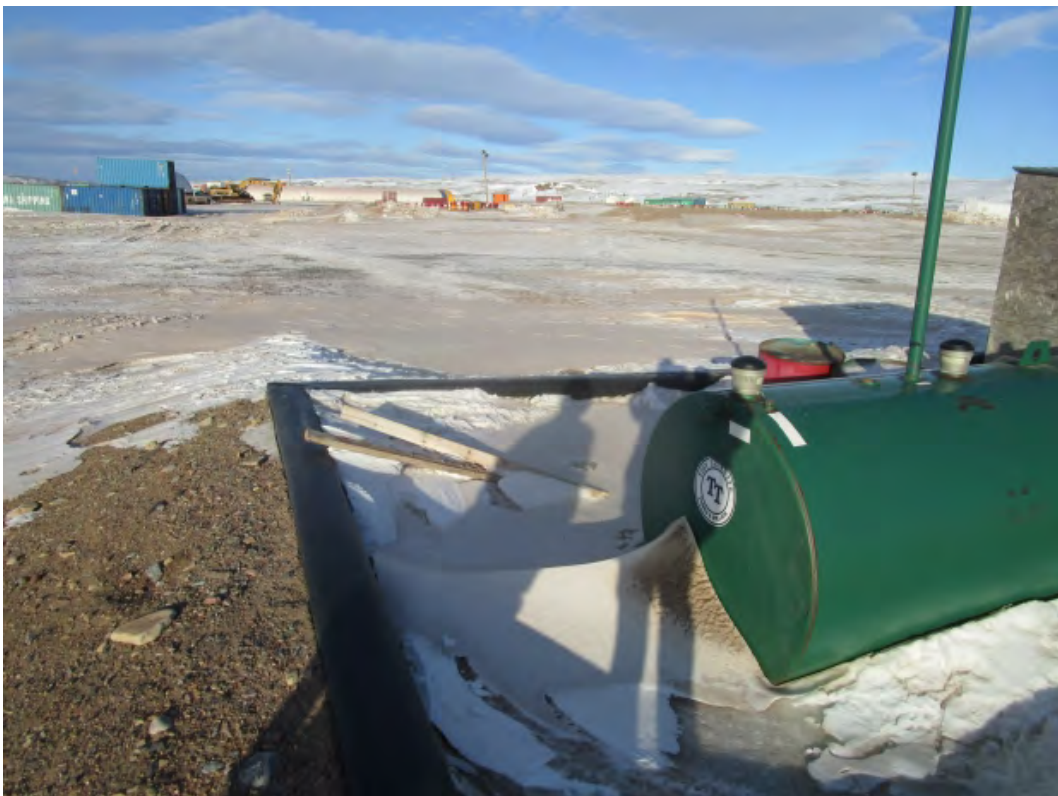
F. Helicopter Fuel Cell Containment
