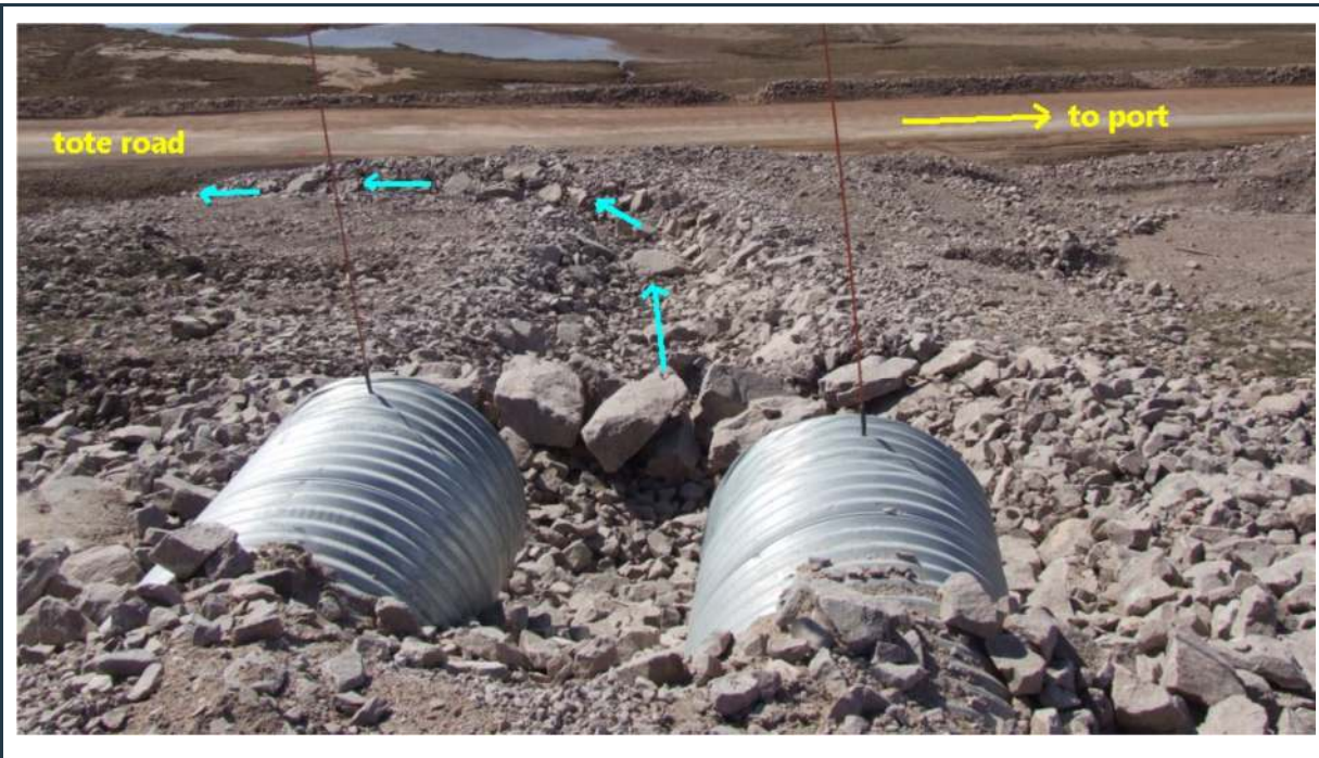
Figure 68: Culverts and drainage ditch, conveying surface water from higher elevation toward the road
