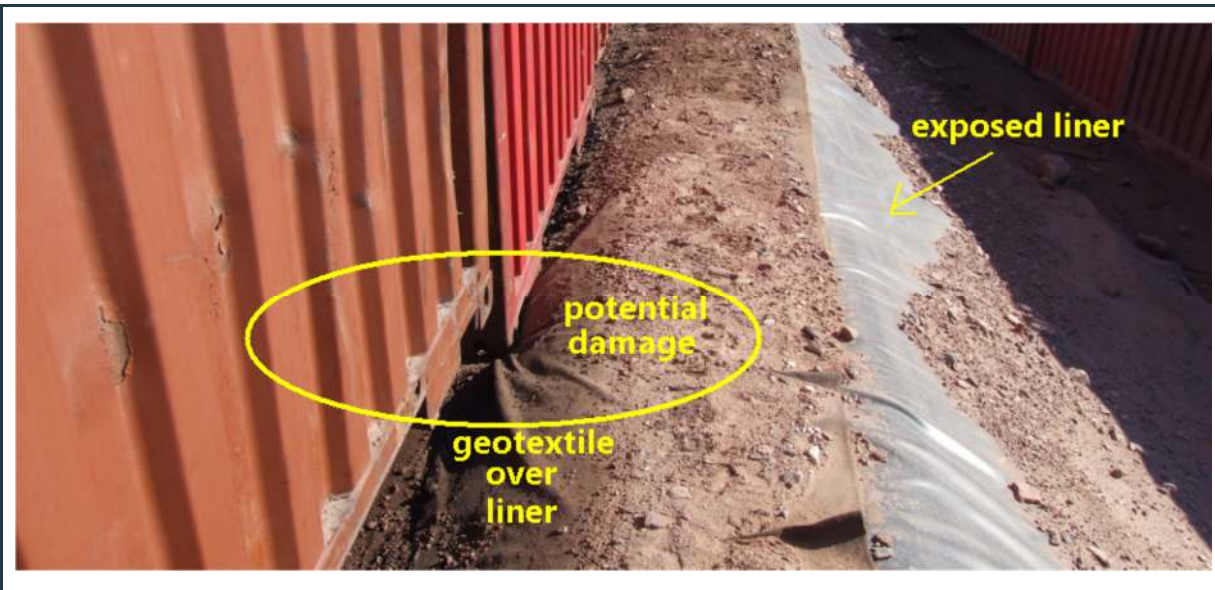
Figure 48: Exposed geotextile and liner at the HWB-4 pond, with location of potential damage to liner
