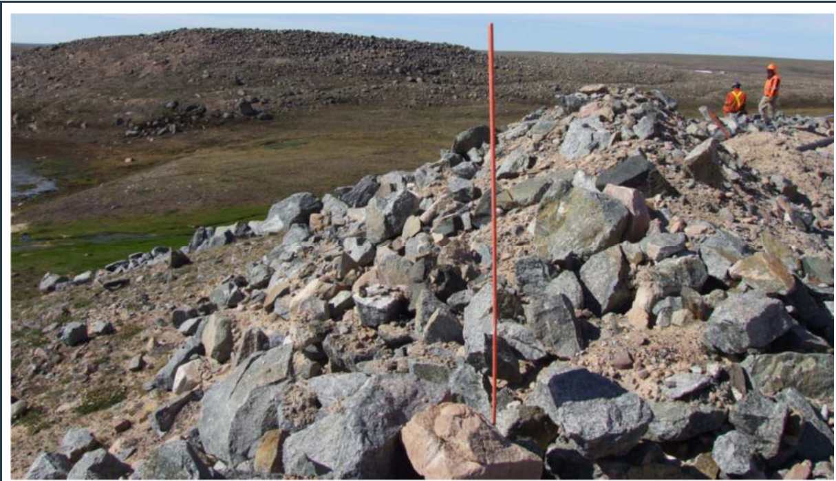
Figure 40: Water discharge area. Stable slope, comprising a mix of crushed rock and soils.
