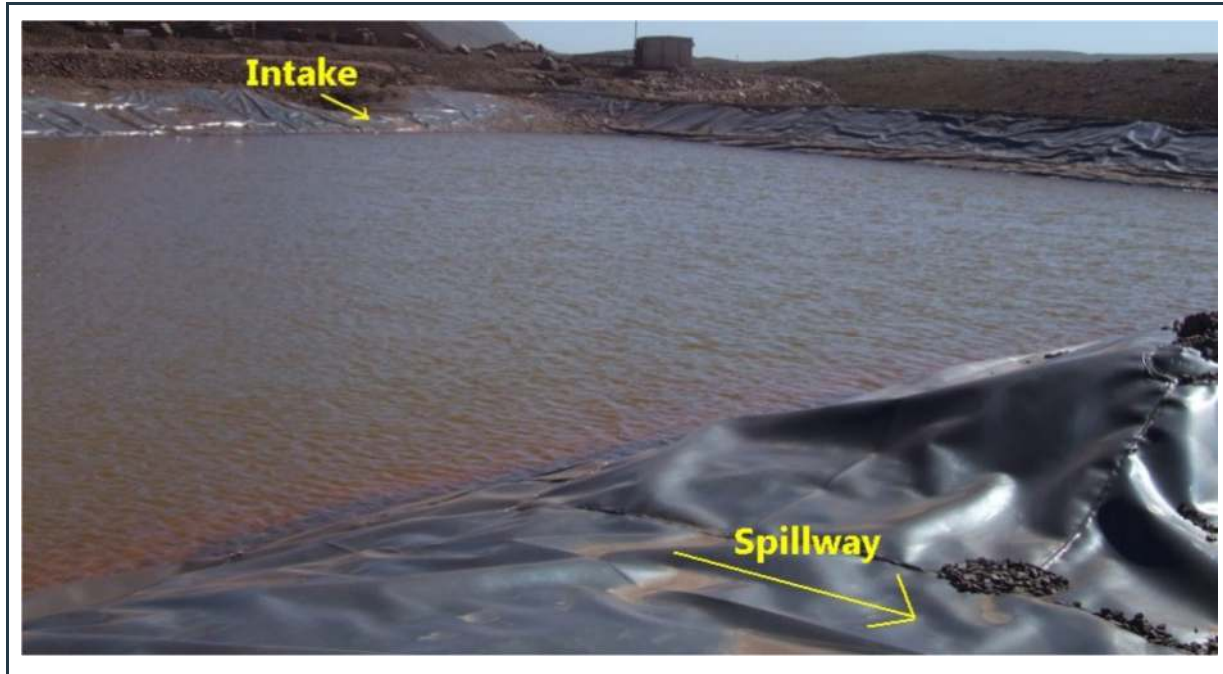
Figure 20: MS-06 surface water collection pond
