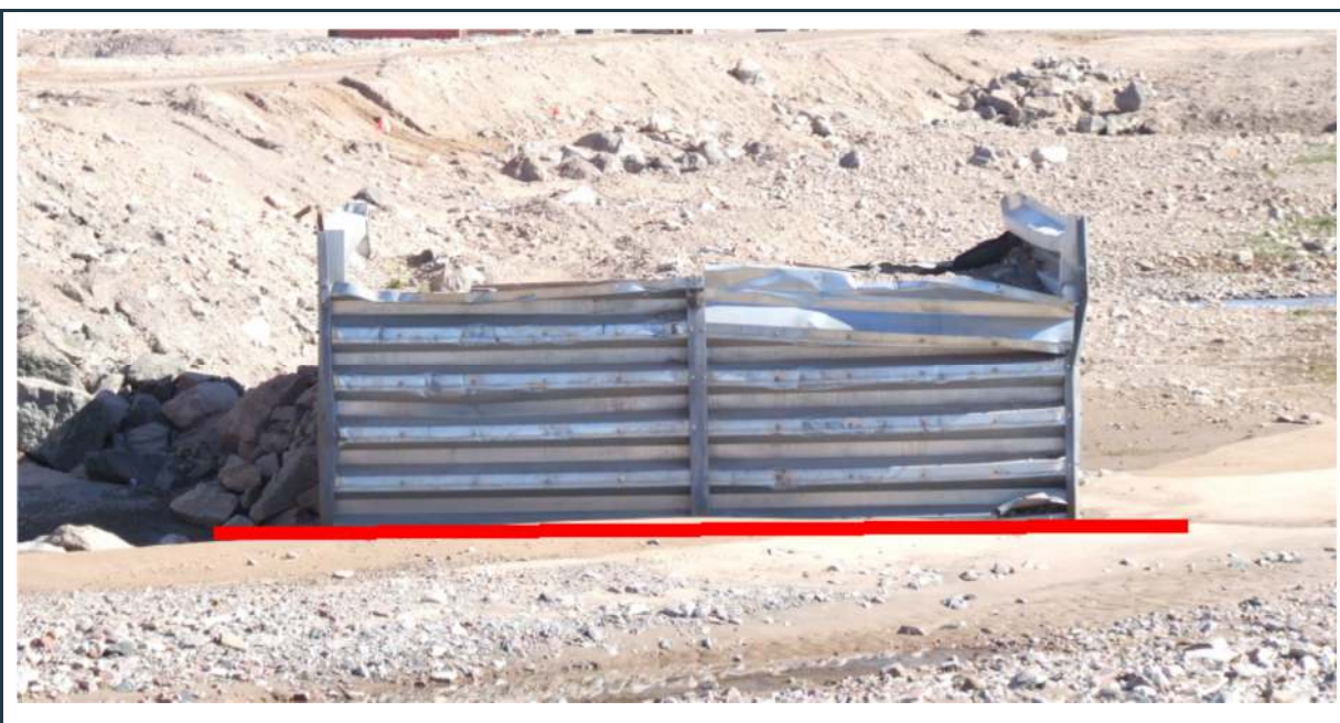
Figure 81: One of the “old” abutments at bridge 97. The section above the red-line may be removed, but the removal is not necessary.
