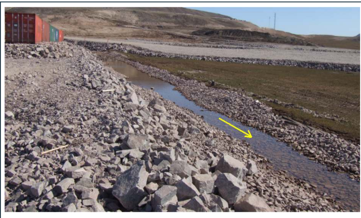
Figure 67: 380 M surface water collection ditch (under construction)
