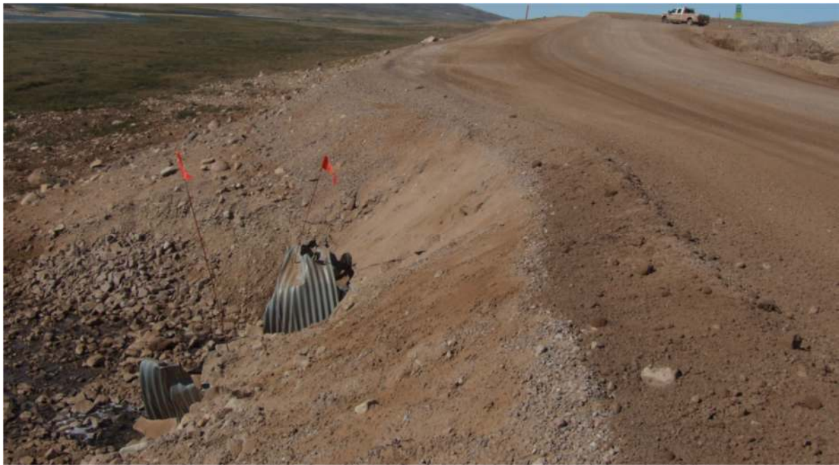
Figure 100: View of culvert(s) 114D (somewhat damaged outlet). Repair and extension is required.
