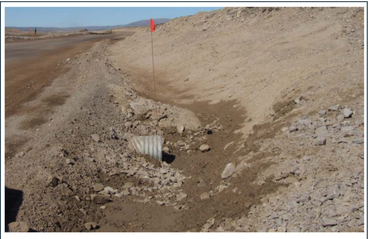
Figure 95: View of culvert 110A (inlet) in good condition
