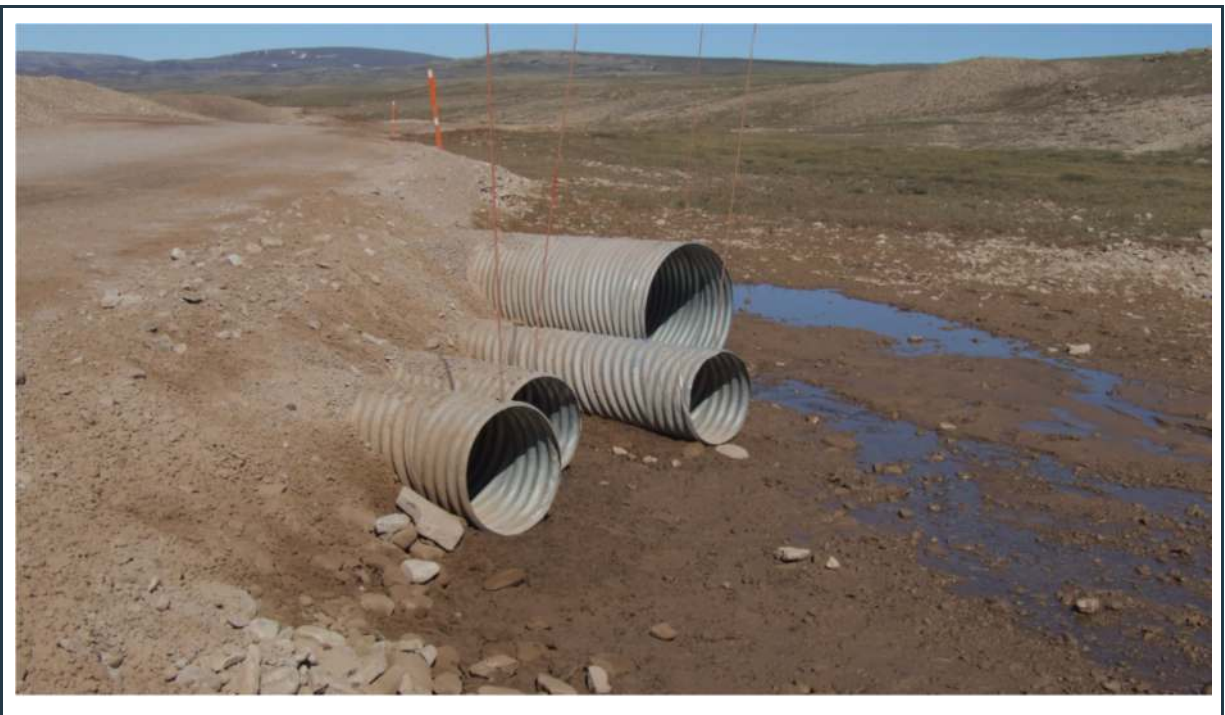
Figure 91: View of culvert(s) 102 (inlet) in excellent conditions
