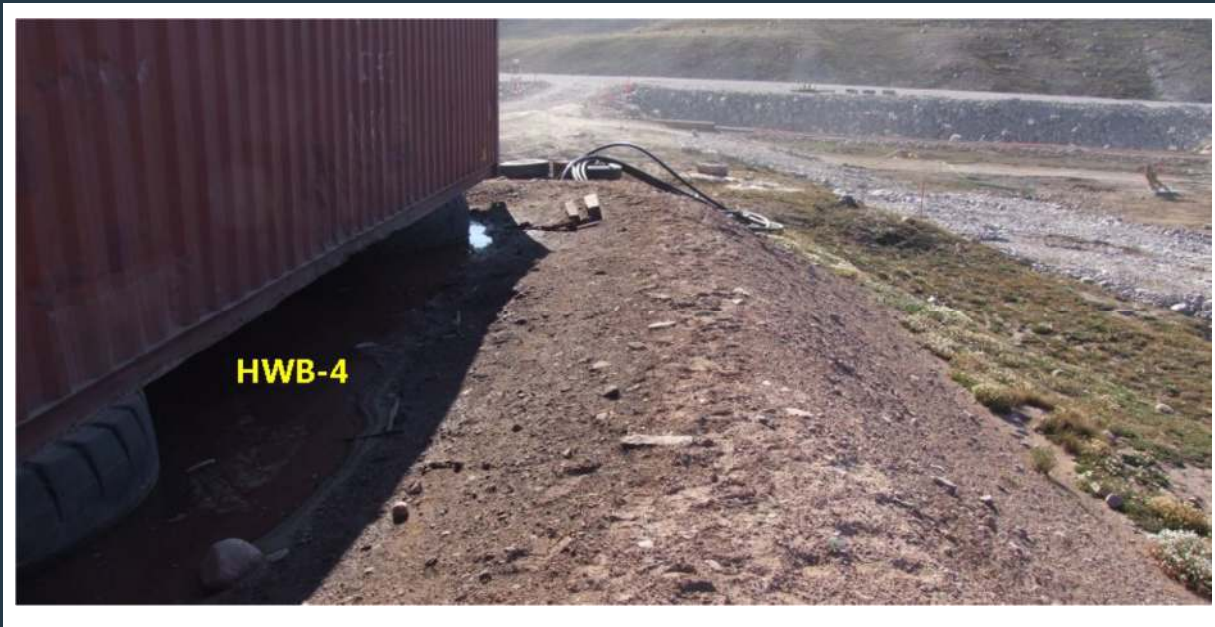
Figure 46: Stable berm at the HWB-4 pond
