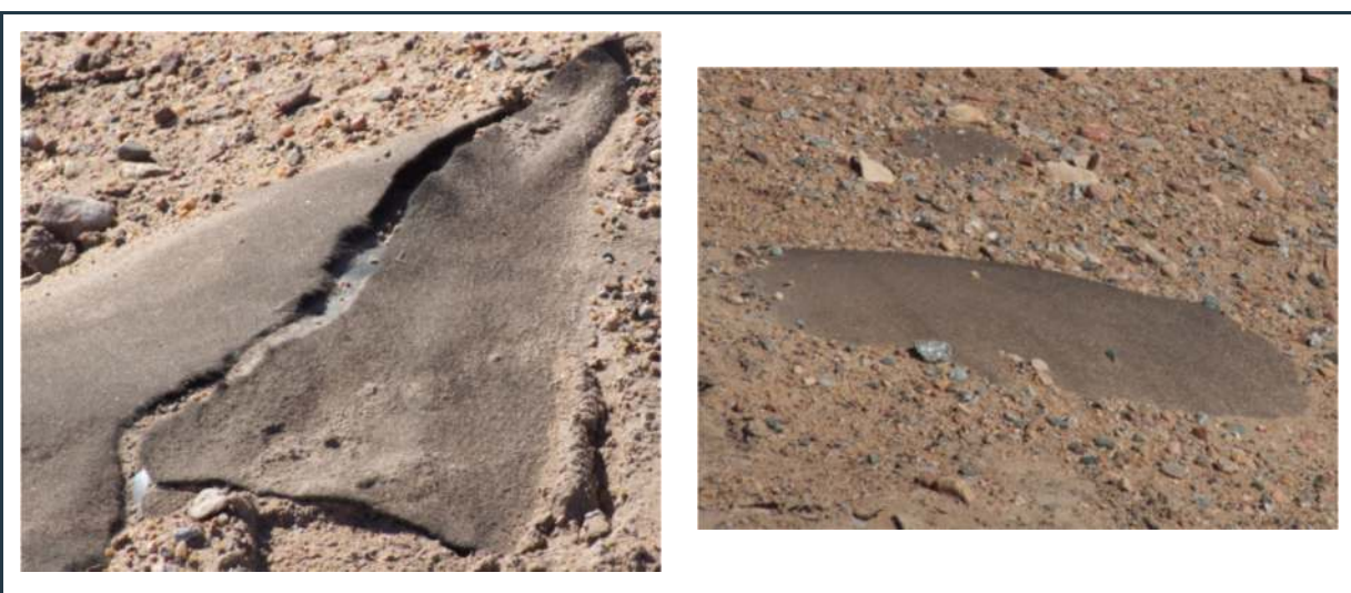
Figure 33: Exposed and ripped geotextile fabric on the berm of the jetfuel farm
