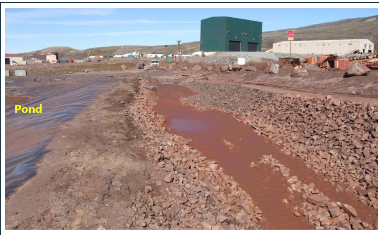
Figure 23: MS-06 surface water collection pond and side-ditch
