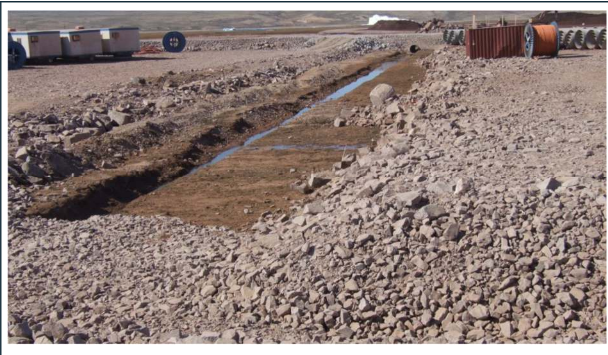
Figure 66: W13-W14 surface water collection ditch (under construction)
