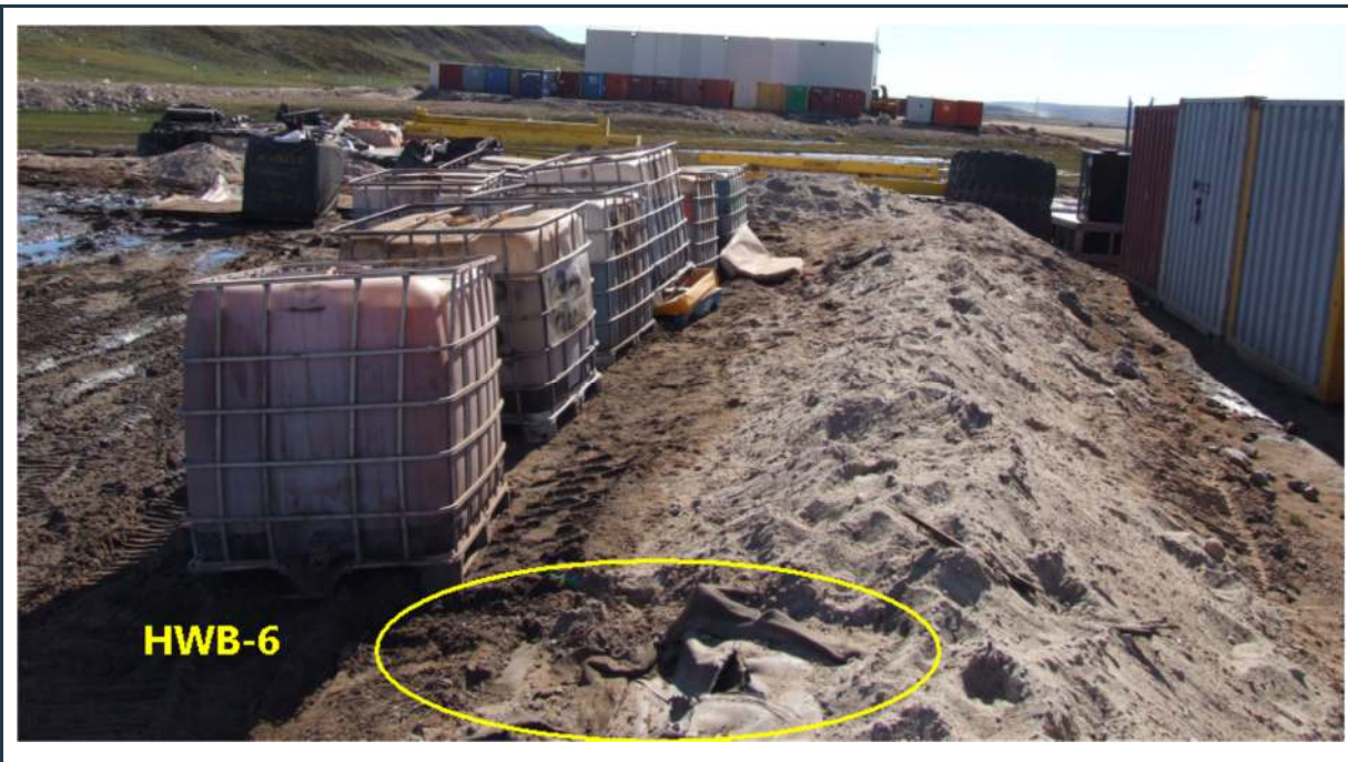
Figure 16: View of HWB-6. Note the damaged liner at the yellow circle.
