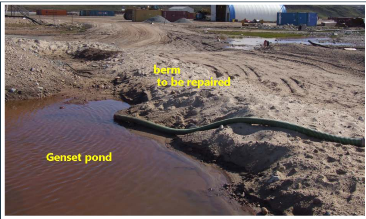
Figure 31: View of the south section of the berm that needs to be repaired (raised and regraded)
