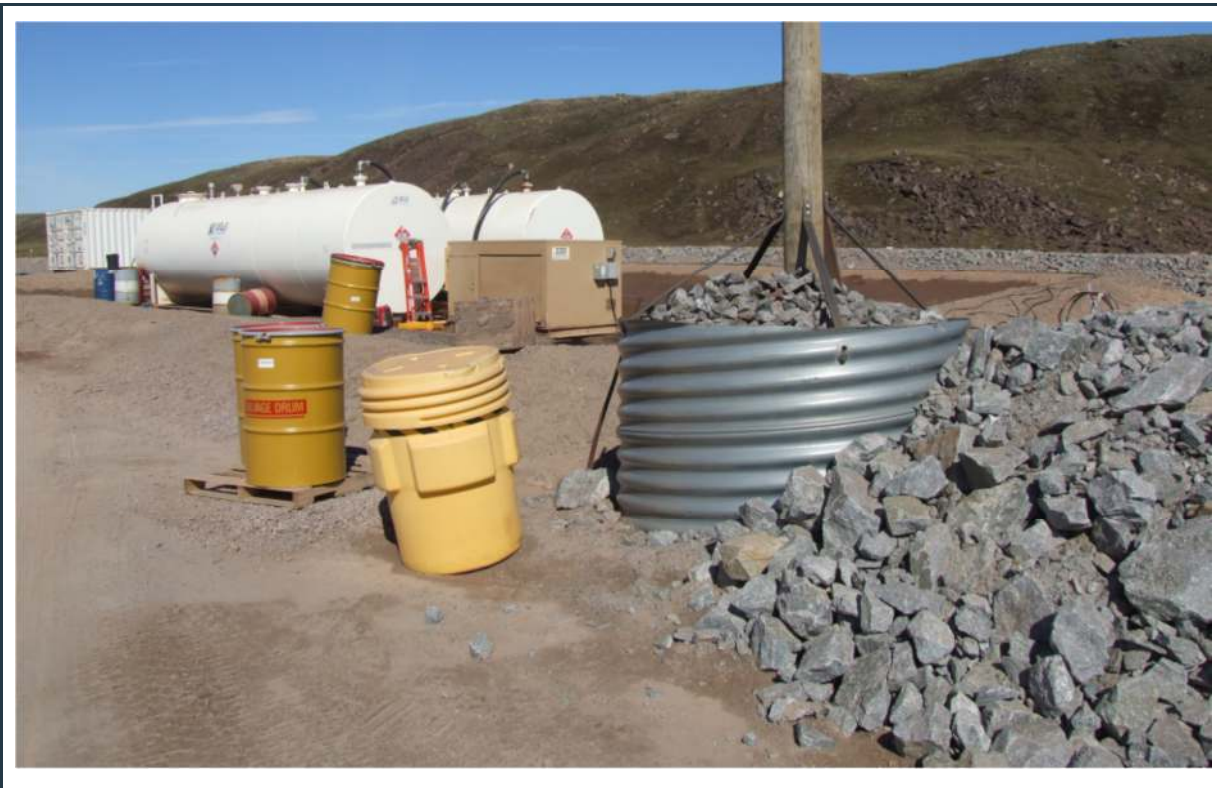
Figure 32: View of the jetfuel farm's double berm system (note the additional crushed rock berm)
