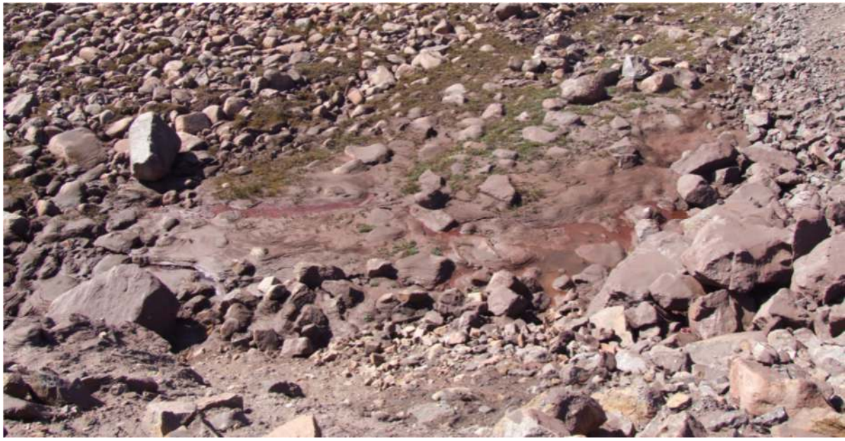
Figure 24: Water seepage at the toe of the tote road embankment near the crusher pad
