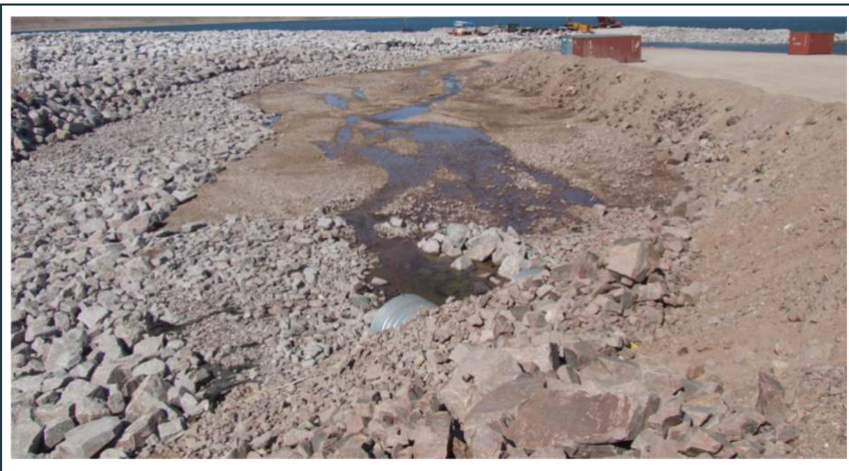
Figure 65: P-SWD-7 surface water collection ditch adjacent to the new freight dock (under construction)
