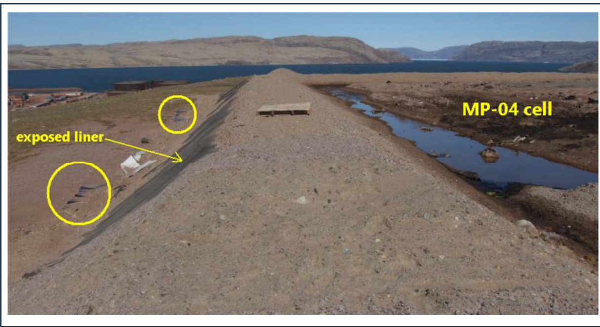
Figure 53: Stable berm at the MP-04 landfarm with exposed liner on the downstream face of the berm
