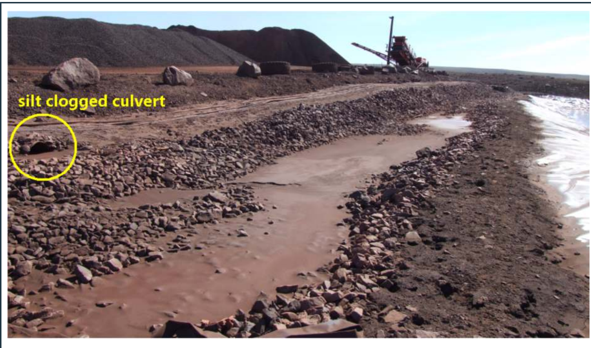
Figure 22: Surface water collection ditch with clogged culvert
