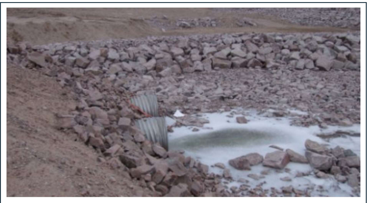
Figure 56: View of the P-SWD-7 surface water collection ditch and culverts, adjacent to the new freight dock (under construction).
