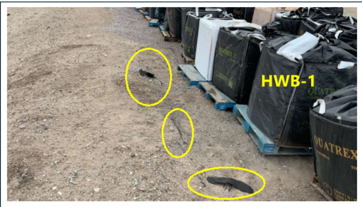
Figure 40: Ripped geotextile and exposed liner at the stable northern berm of the HWB-1 cell.
