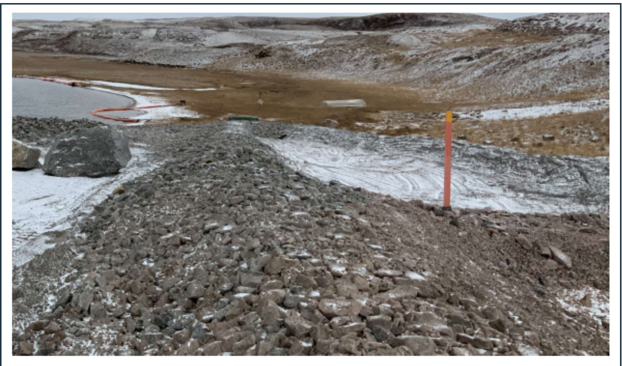
Figure 36: Use of floating silt curtains in the vicinity of the CLSP check berms.
