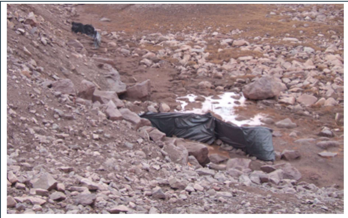
Figure 20: Minor water seepage as ice mount at the toe of the embankment where the crusher pad ditch embankment fill meets the tundra.
