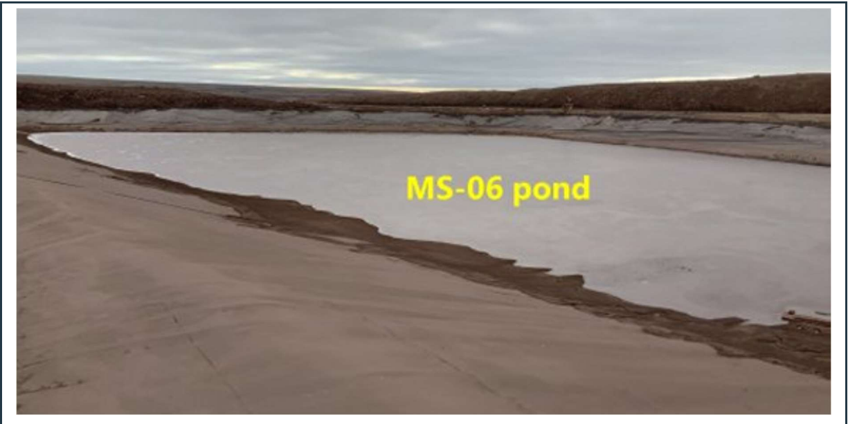
Figure 17: MS-06 surface water collection pond (low water level with frozen surface).
