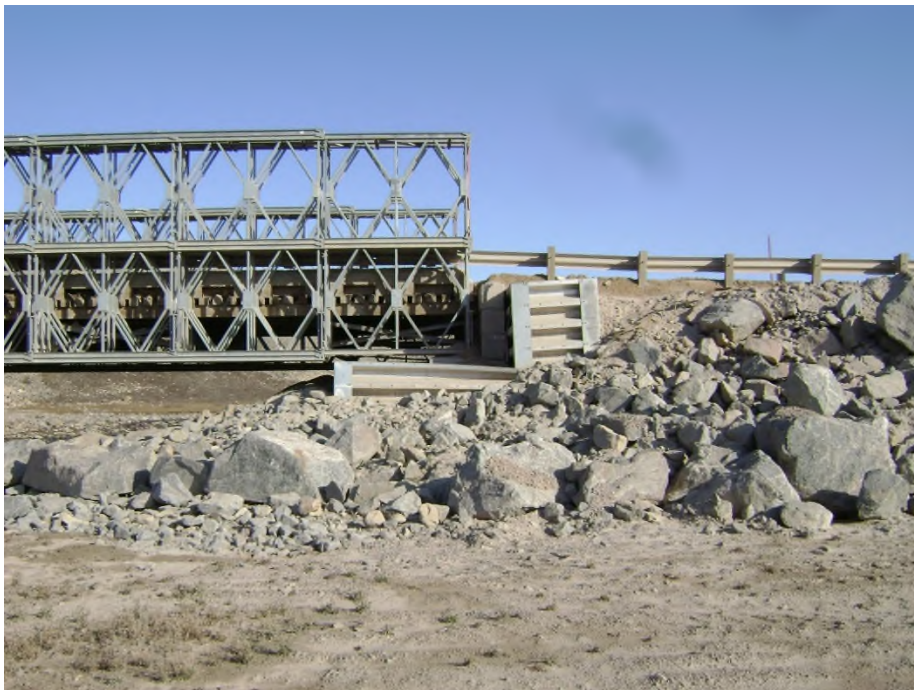
Photo 31 (2708): KM 64 Bridge, south abutment. Note tilting of upper bin wall.
