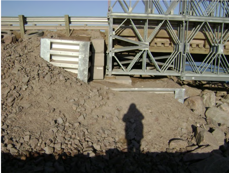
Photo 28 (2678): KM 17 Bridge, west abutment. Note tilting of upper bin wall.
