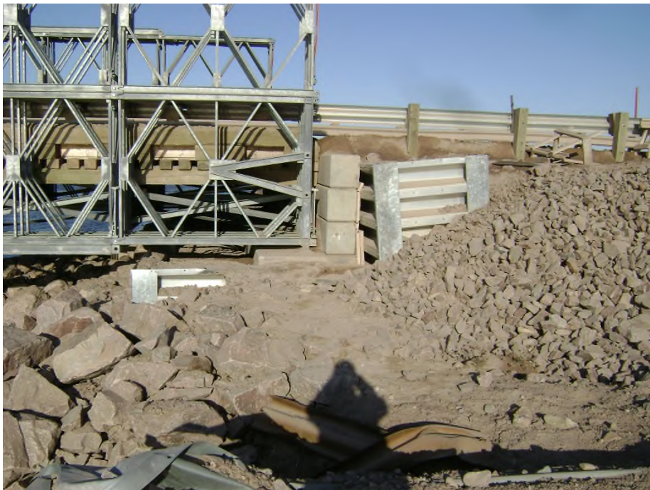
Photo 29 (2683): KM 17 Bridge, east abutment. Note tilting of upper bin wall.
