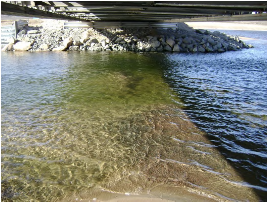
Photo 34 (2718): KM 80 Bridge, road surfacing gravel that has fallen through the centerline joint in the bridge deck and is visible in the river.
