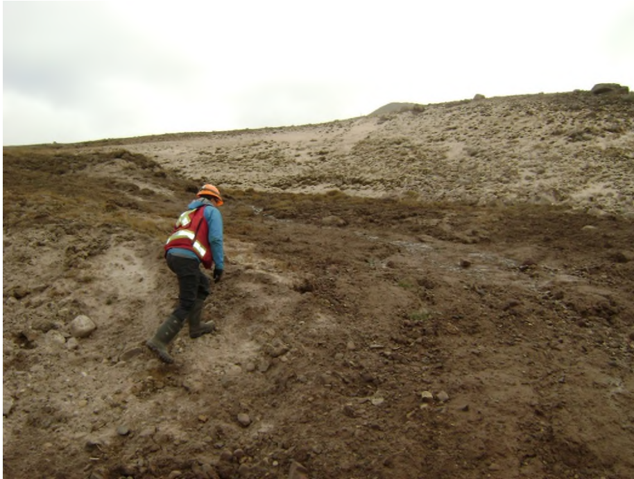
Photo 36 (2523): KM 2.5 slope instability and mud slide adjacent to the Tote Road.
