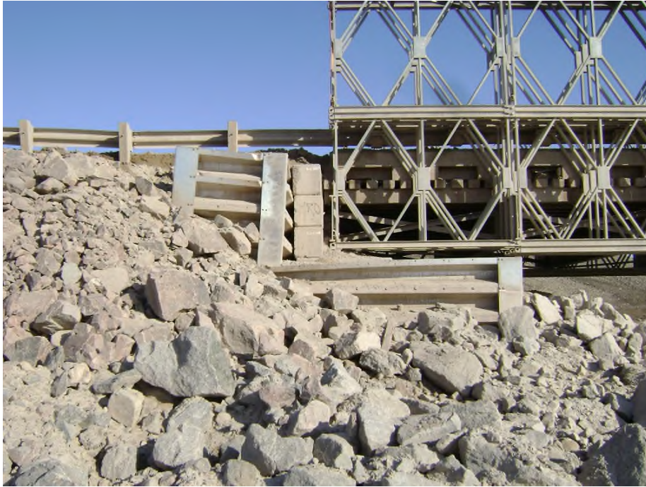
Photo 30 (2683): KM 63 Bridge, north abutment. Note tilting of upper bin wall.
