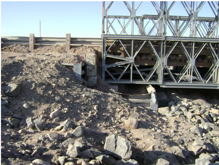
Photo 35 (2719): KM 97 Bridge, north abutment. Shorter upper bin wall has not tilted as much as other bridges. Lower chord of the bridge truss appears to be in contact with the lower bin wall.
