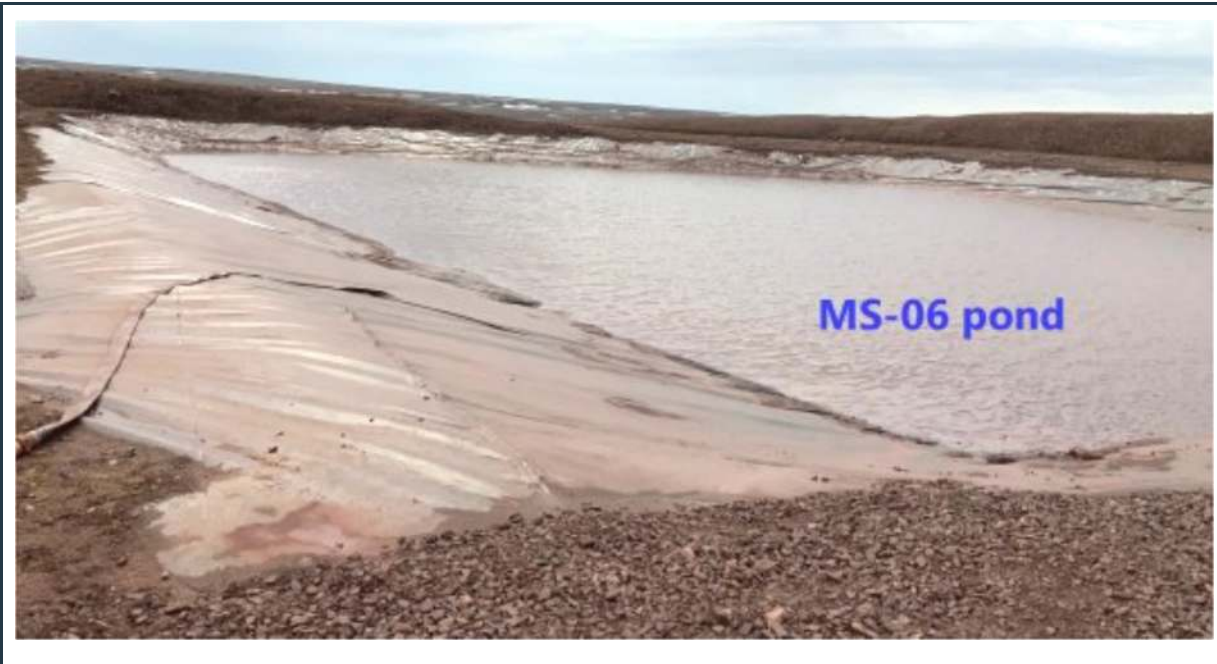
Figure 21: MS-06 surface-water collection pond with stable berms and intact liner.
