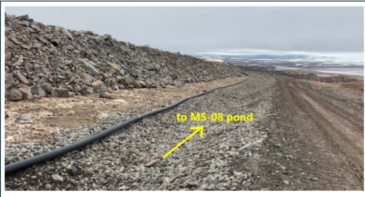
Figure 29: Well-maintained drainage ditch along the east side of the waste rock facility
