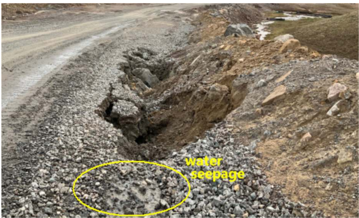
Figure 48: Surface water flowing from the quarry area along the road resulted in a failure of the edge of the access road leading to the quarry. Immediate repair was requested to prevent accidents.
