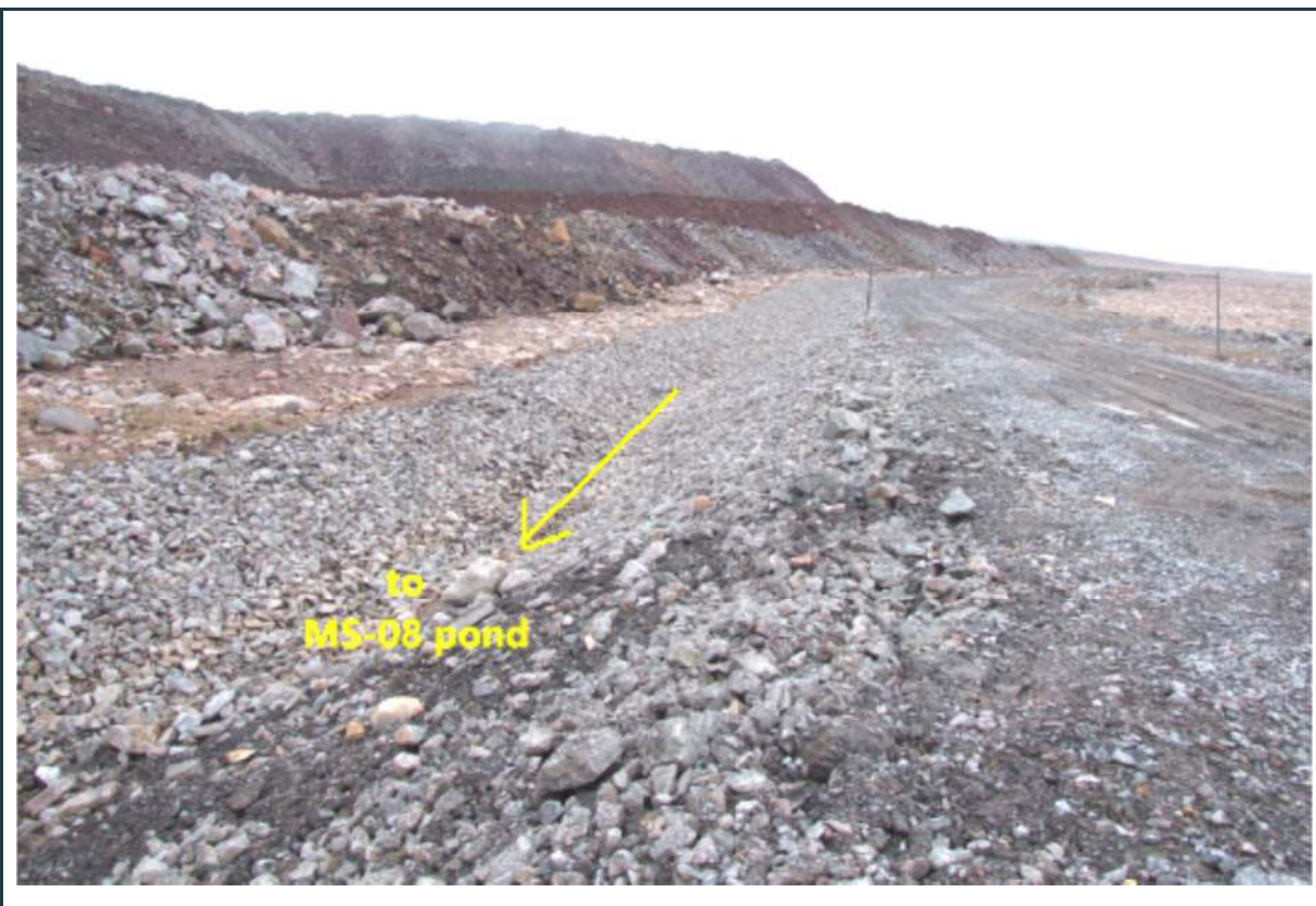
Figure 30: Well-maintained drainage ditch along the west side of the waste rock dump
