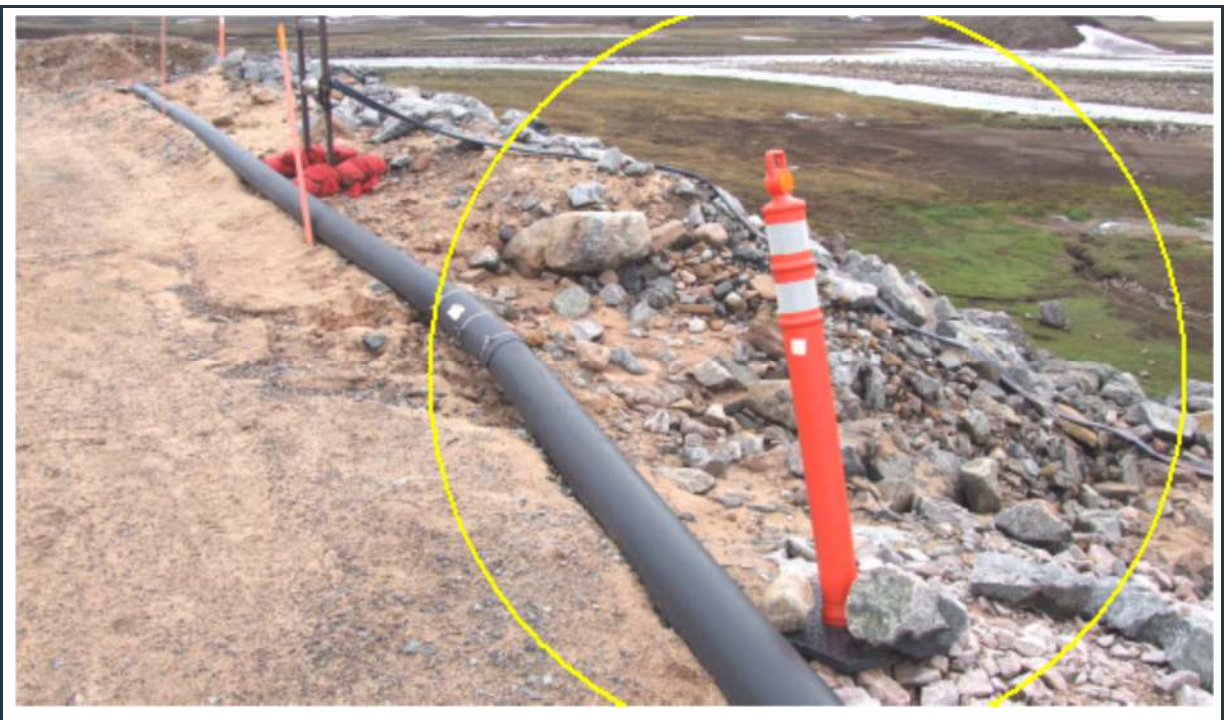
Figure 42: Minor crest/slope erosion (cobbles and boulders rolling down the slope) at the water discharge area. Placement of rock fill is required here to improve slope integrity and prevent erosion.
