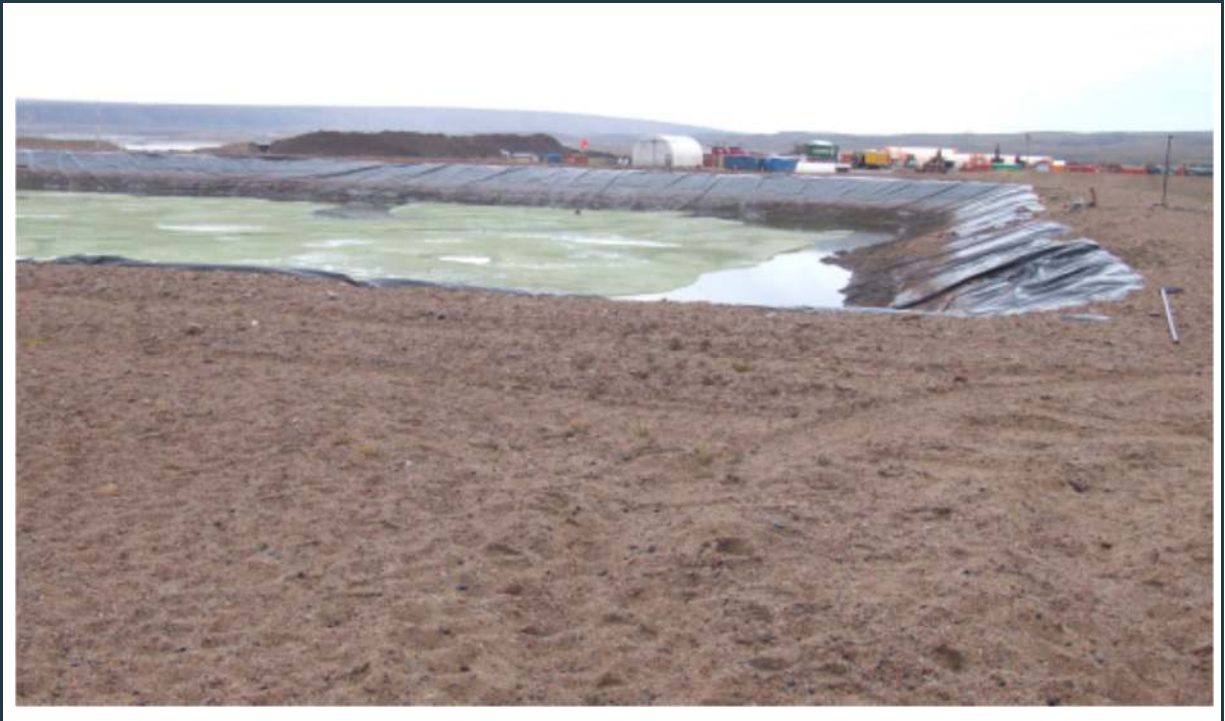
Figure 9: PWS pond #2 – Berm and liner in good condition. The water was recently lowered, and ice still visible in the pond.
