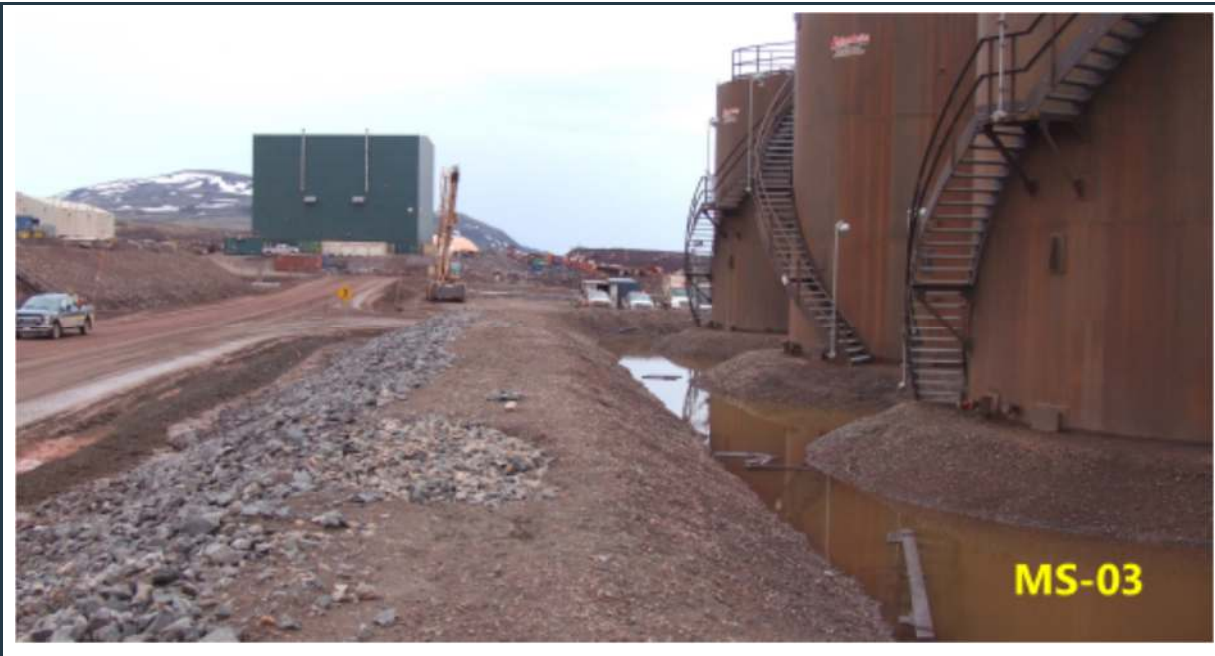
Figure 37: View of the MS-03 diesel fuel tank farm. Note some floating debris that should be removed.
