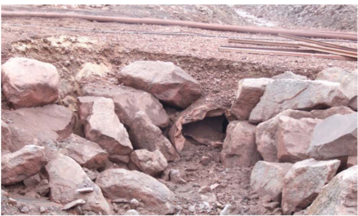
Figure 23: Damaged and clogged (silted) culvert in the ditch shown in Figure 22, near the MS-06 pond.
