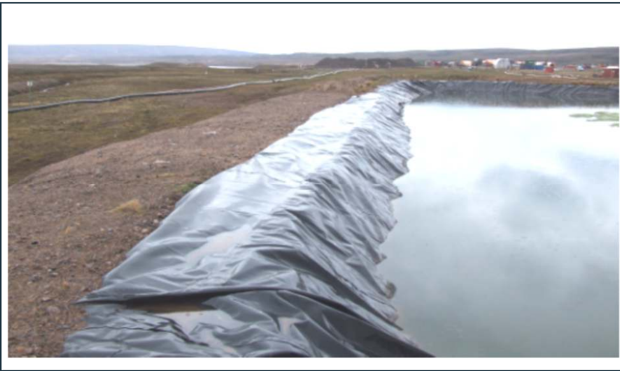
Figure 8: PWS pond #1. Well maintained perimeter berm and liner (note some floating ice in the pond).
