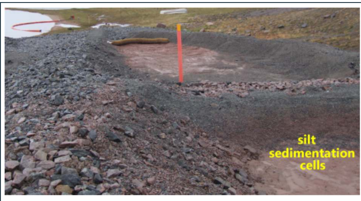
Figure 40: CLSP check dams and berms, forming efficient silt sedimentation cells
