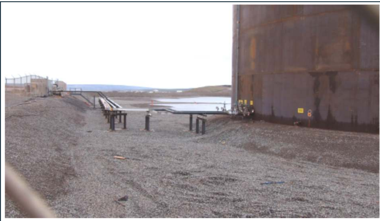
Figure 38: View of the recently completed fuel tank farm with well-constructed stable perimeter berms.
