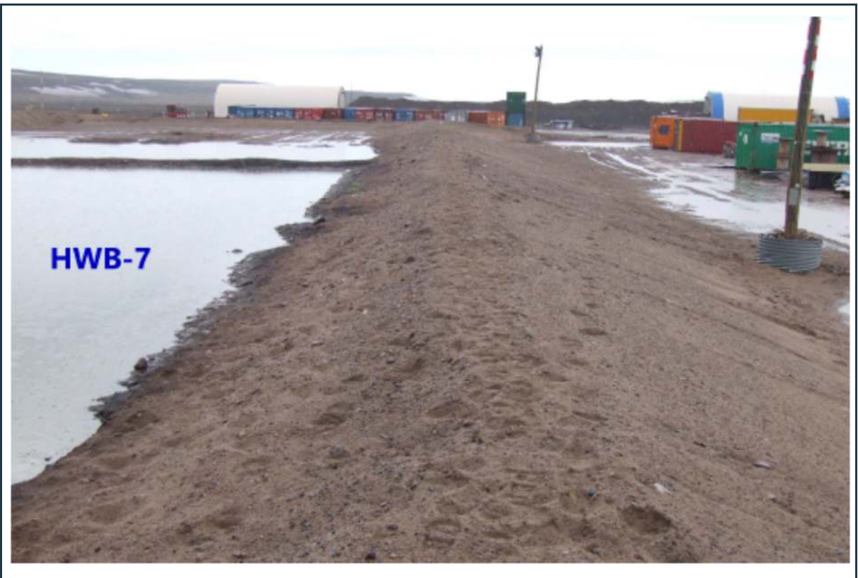
Figure 20: View of the stable berm around the HWB-7 cell.
