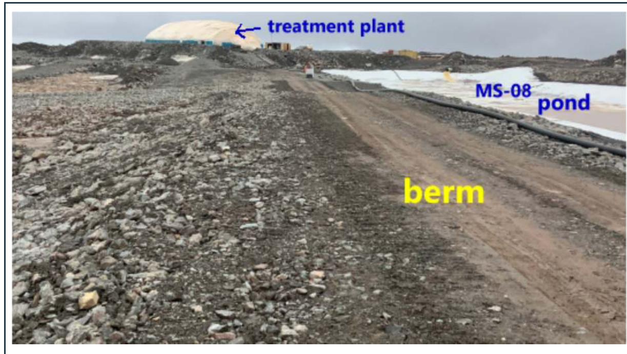
Figure 27: View of the new, robust berm with shallow side-slopes around the MS-08 pond
