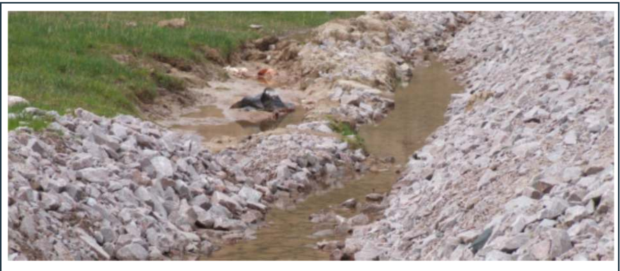
Figure 76: View of the “P-SWD-3 surface water collection ditch with failing side slope. The sloughing is caused by the uncontrolled water flow into the ditch along its alignment (see the next image).
