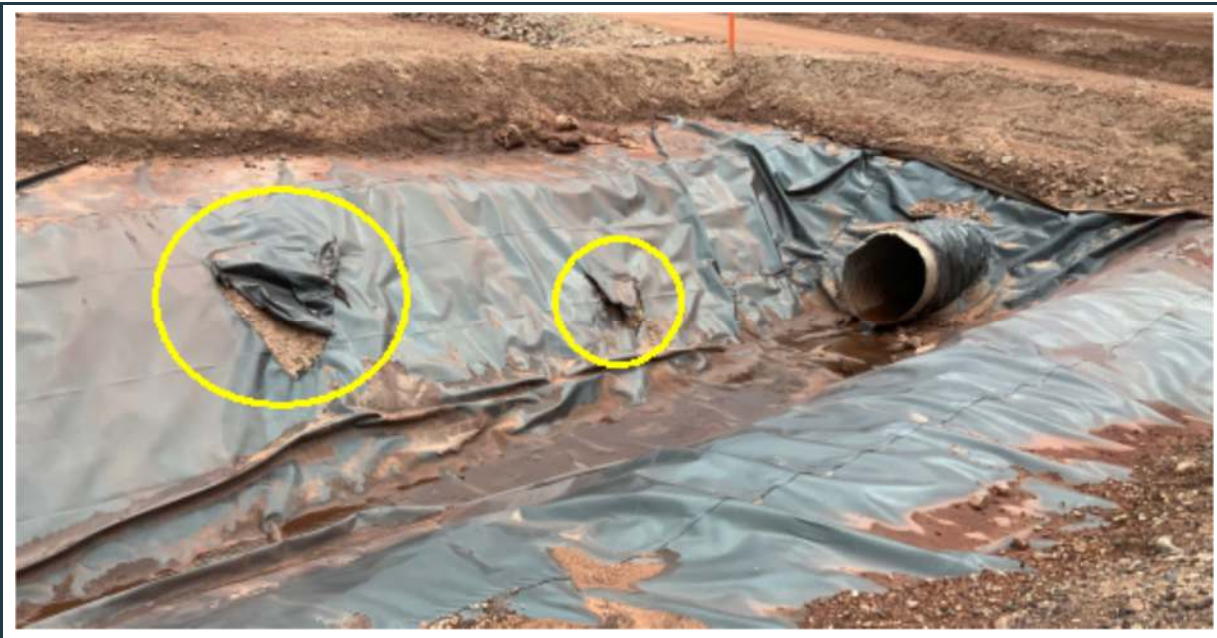
Figure 68: Some liner damage on the slope of the southern intake channel to the MP-05 settling pond.
