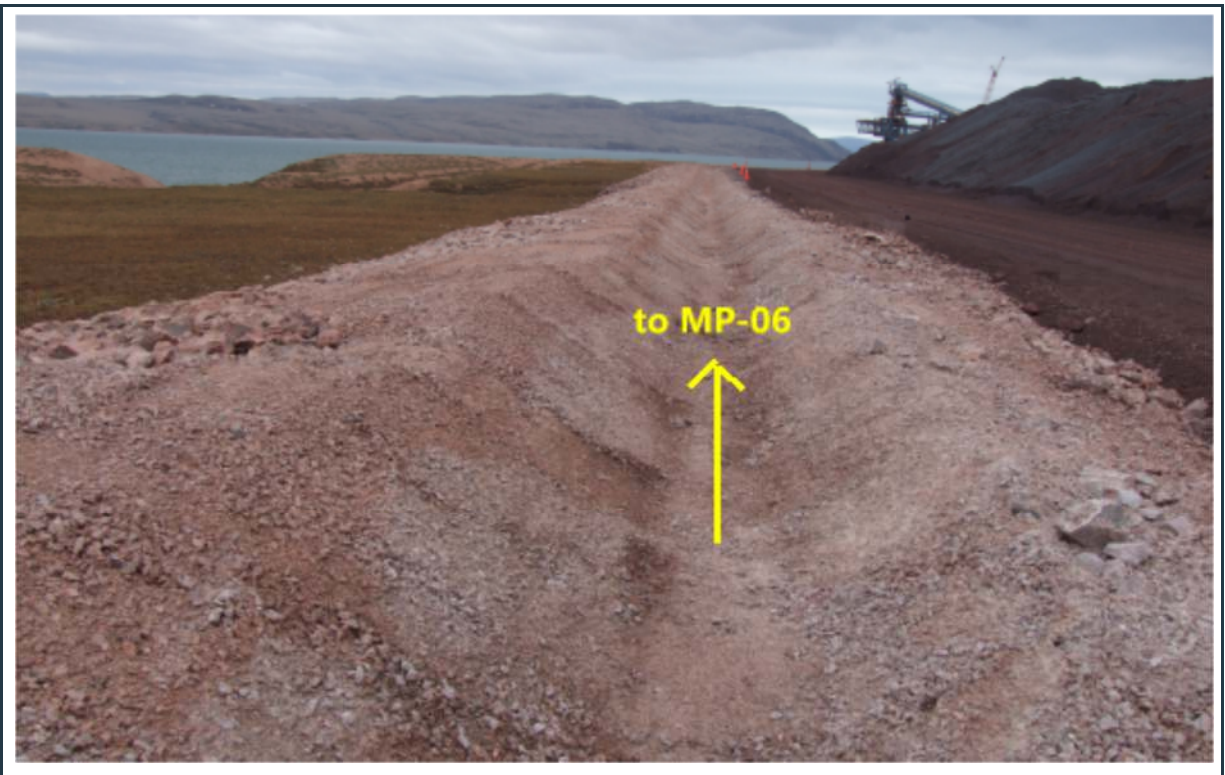
Figure 72: Surface water collection ditch adjacent to the crushed ore storage, draining to MP-06 pond.
