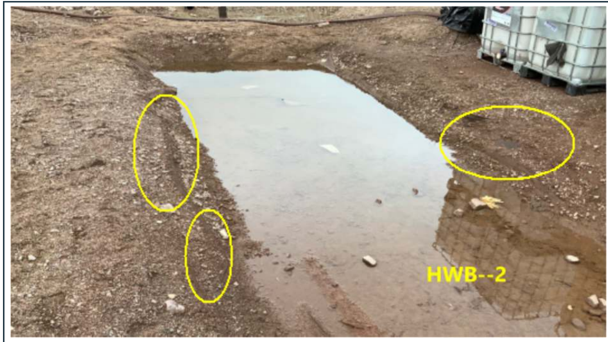
Figure 55: Ponding water in the empty HWB-2 cell with locally exposed geotextile and liner. Empty containers stored immediately adjacent to the cell.
