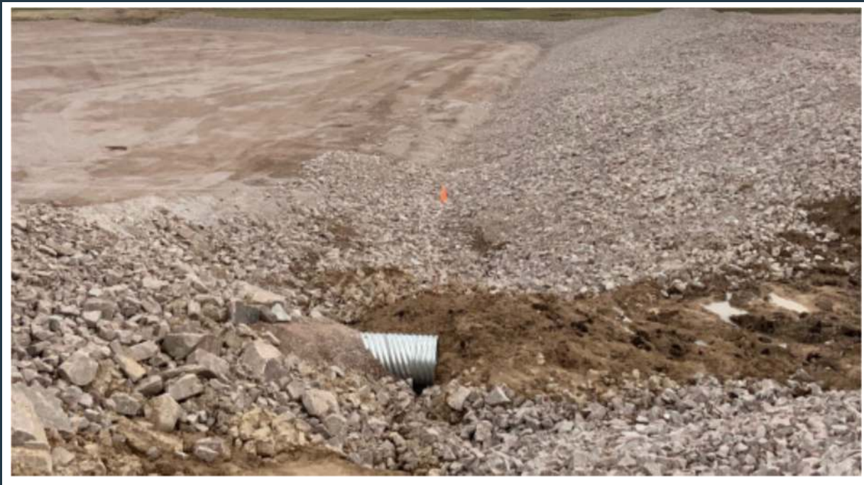
Figure 85: View of the P-SC surface water collection ditch and culvert (still under construction).
