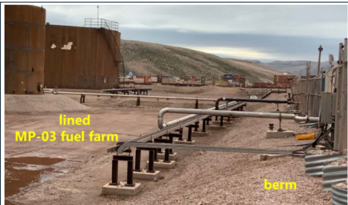
Figure 62: View of stable, well maintained berms around the MP-03 fuel tank farm.
