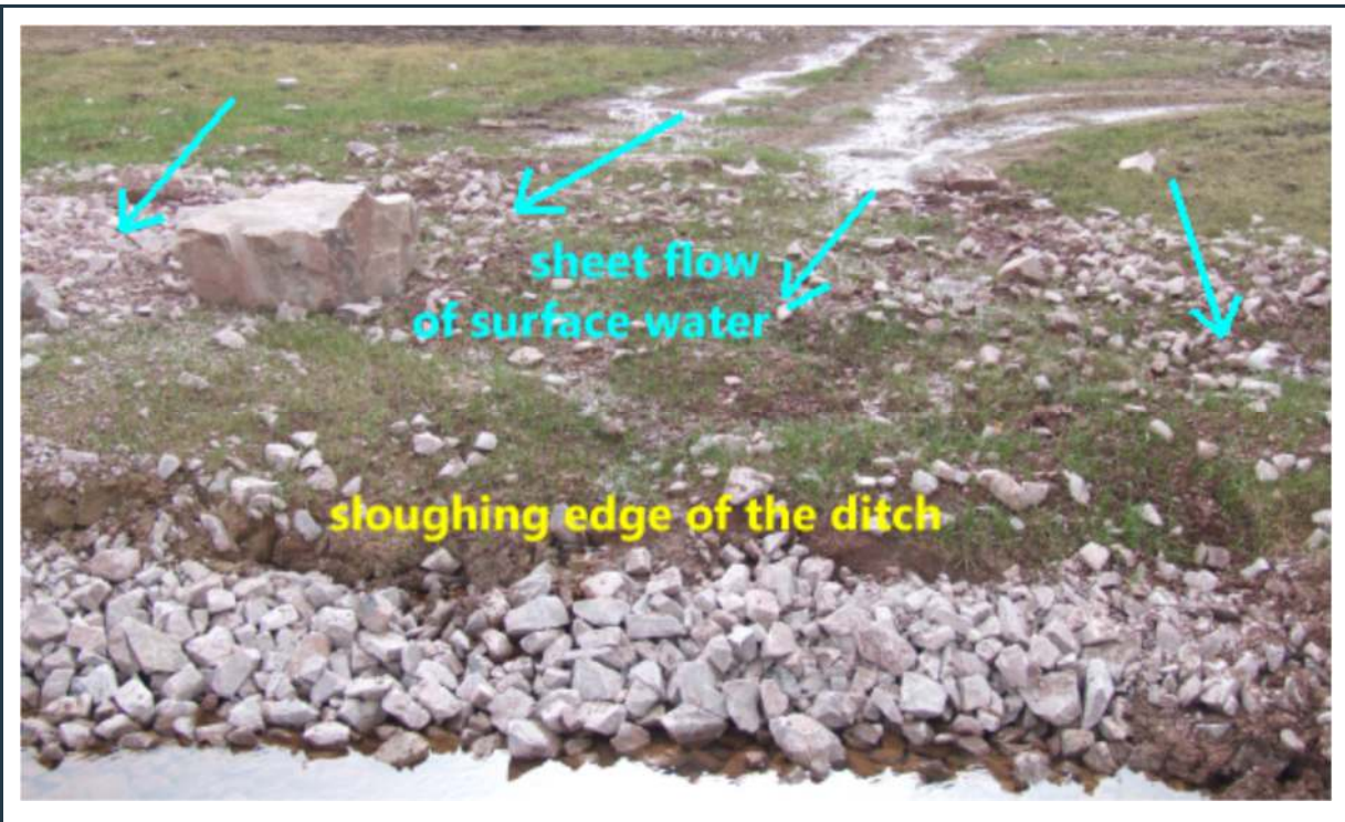
Figure 77: Sheet flow of surface water resulting in sloughing of one side of the P-SWD-3 ditch.
