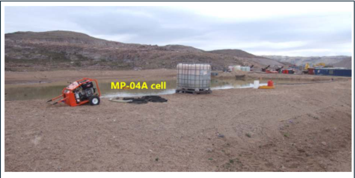
Figure 65: View of the MP-04A contaminated snow dump cell with stable berms.
