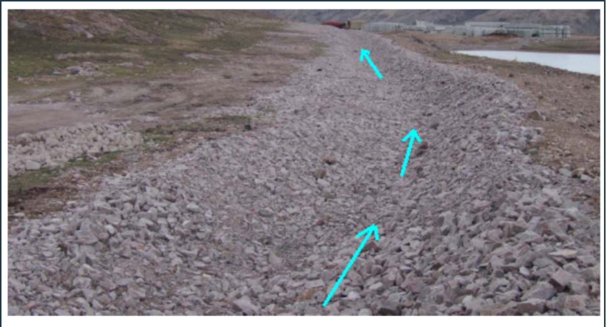
Figure 79: View of the well maintained P-SWD-6 - "Q01 South" surface water collection ditch.
