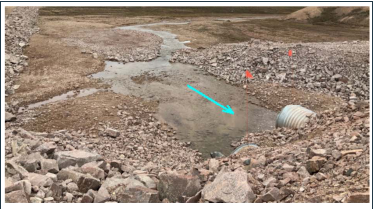
Figure 80: View of the P-SWD-7 surface water collection ditch and culverts (inlet).
