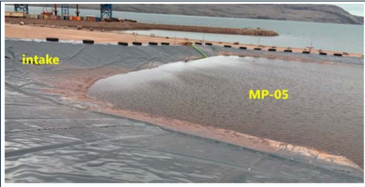
Figure 67: View of stable berms at the MP-05 settling pond (north-east corner of the ore stockpile).
