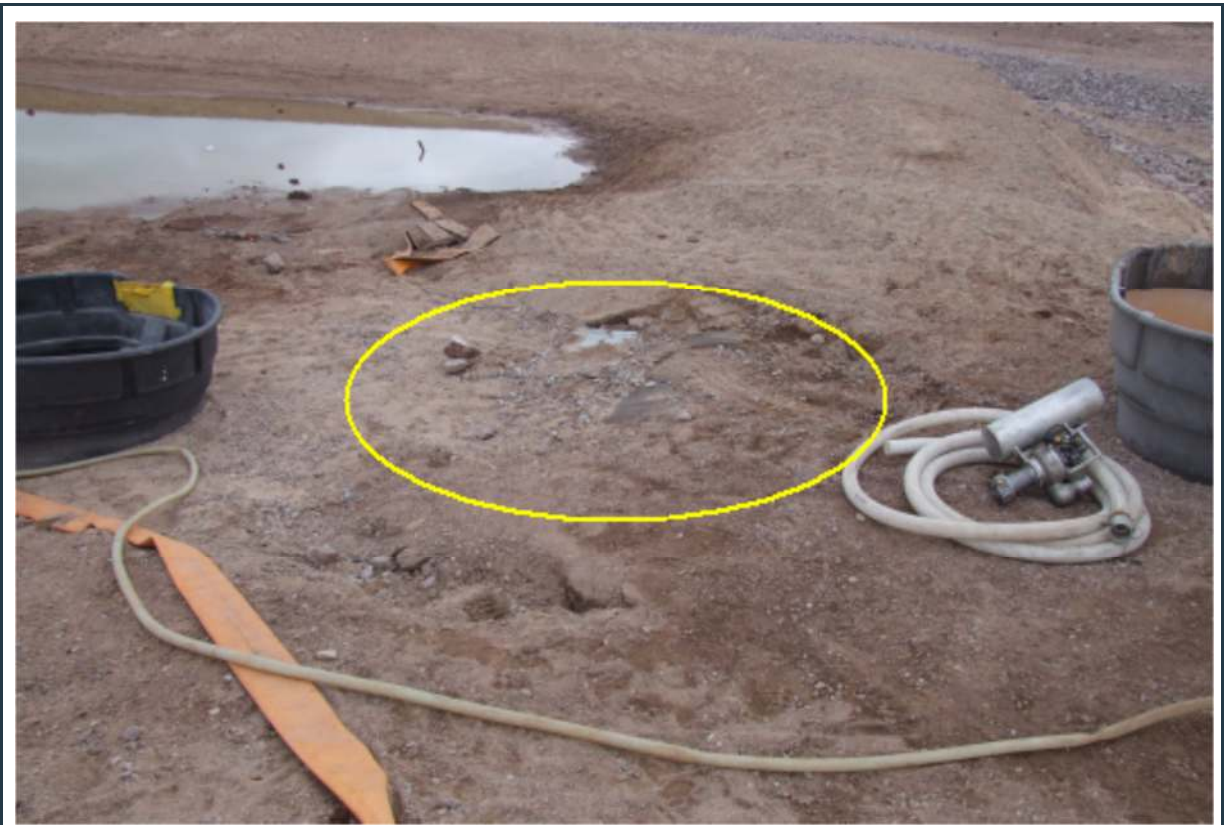
Figure 66: Condition of the ramp to the MP-04A snow dump, with exposed liner (yellow circle).
