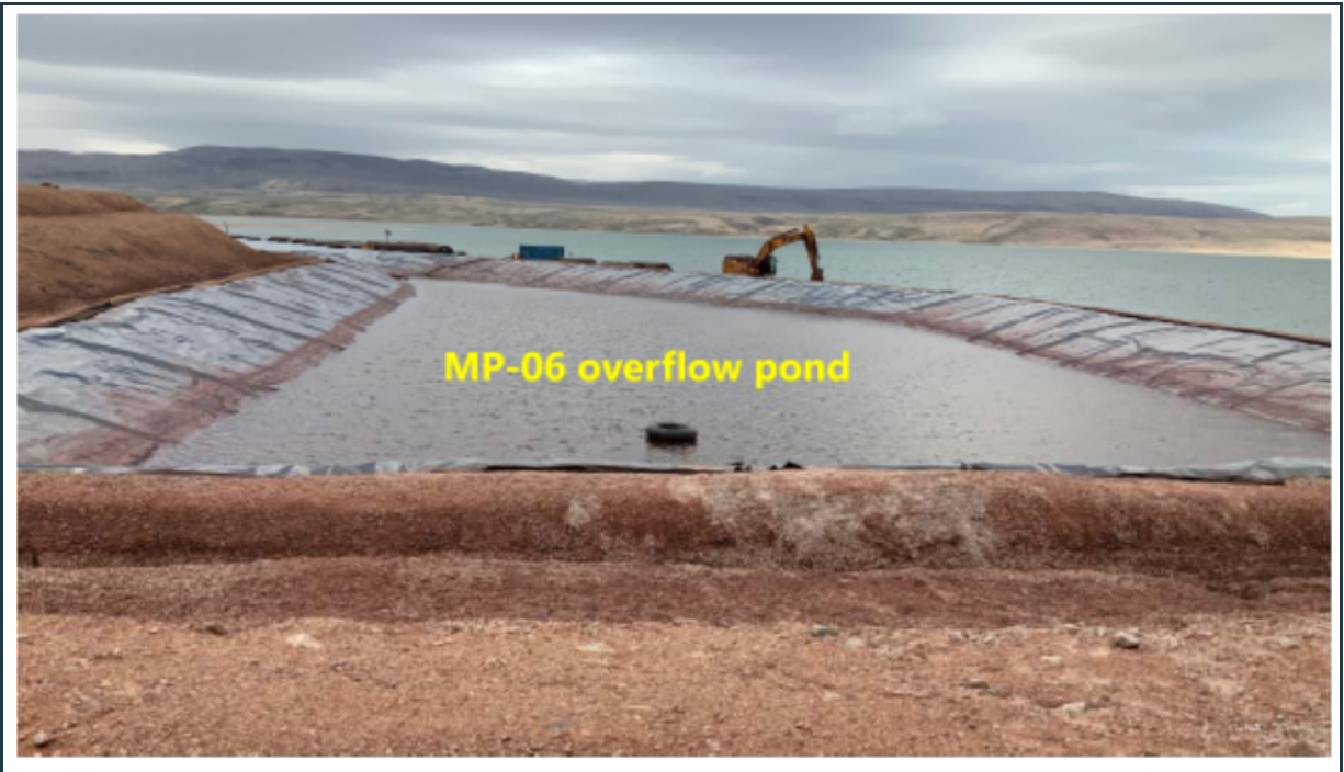
Figure 71: View of the lined MP-06 overflow pond, with stable berms.
