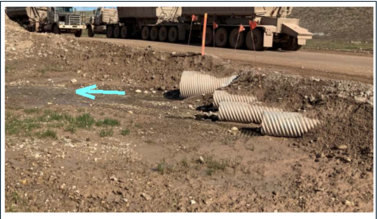
Figure 106: View of culvert(s) 102 (outlet) in good conditions.
