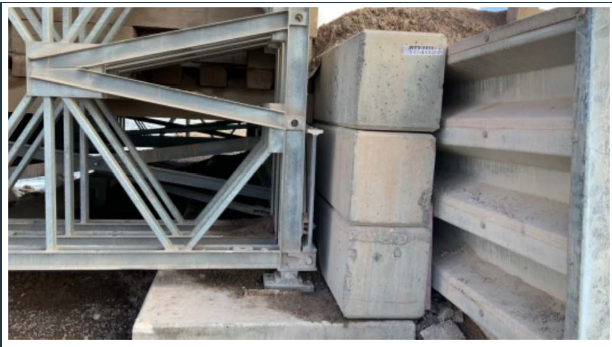
Figure 90: Foundation and abutment conditions at the south-west abutment of bridge 17.
