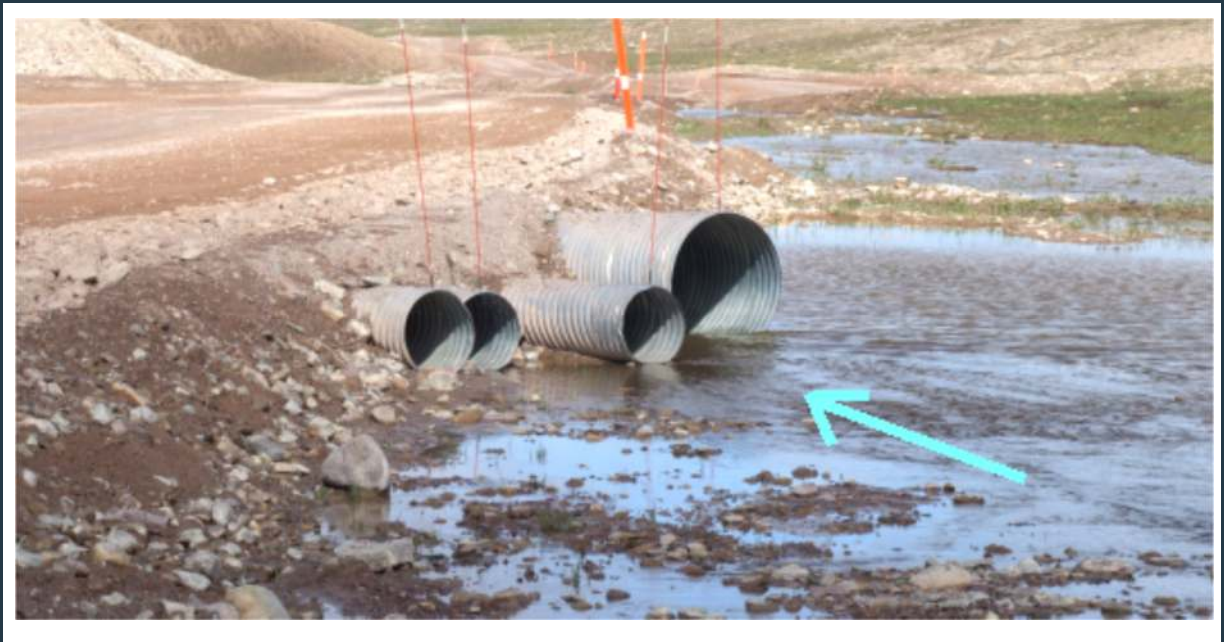
Figure 105: View of culvert(s) 102 (inlet) in good conditions.
