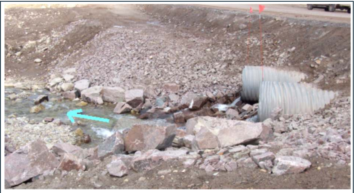
Figure 104: View of culvert(s) 094 (outlet) in good condition.
