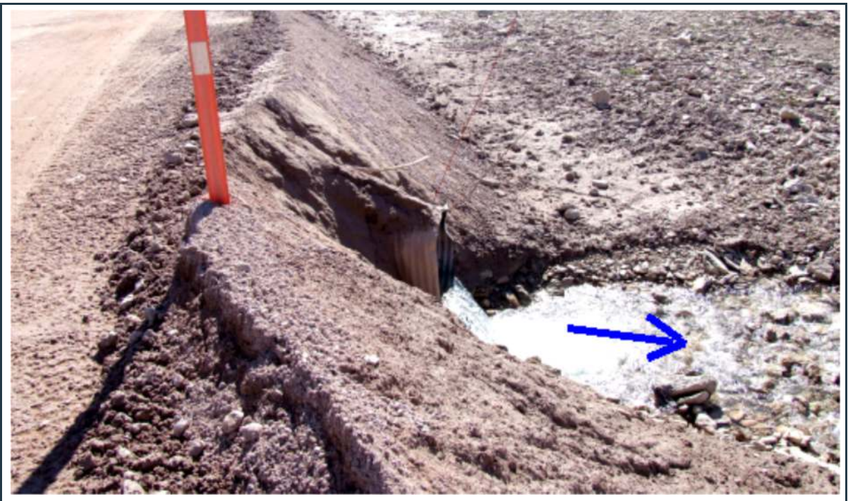
Figure 102: View of culvert 083 (outlet), with some slope erosion around the culvert.
