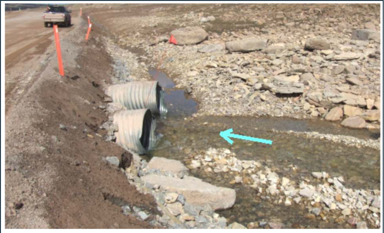
Figure 103: View of culvert(s) 094 (inlet) in good condition.
