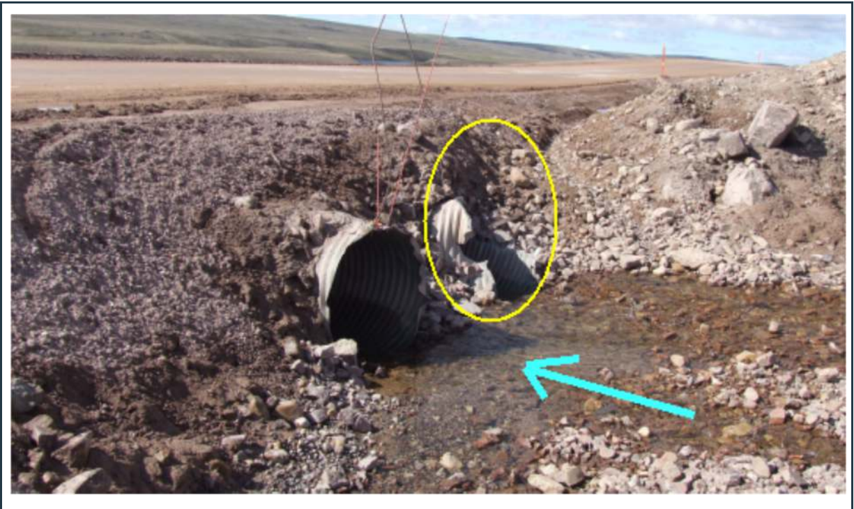
Figure 115: View of culvert(s) 114D inlet. Repair of the northern pipe is required (yellow circle).
