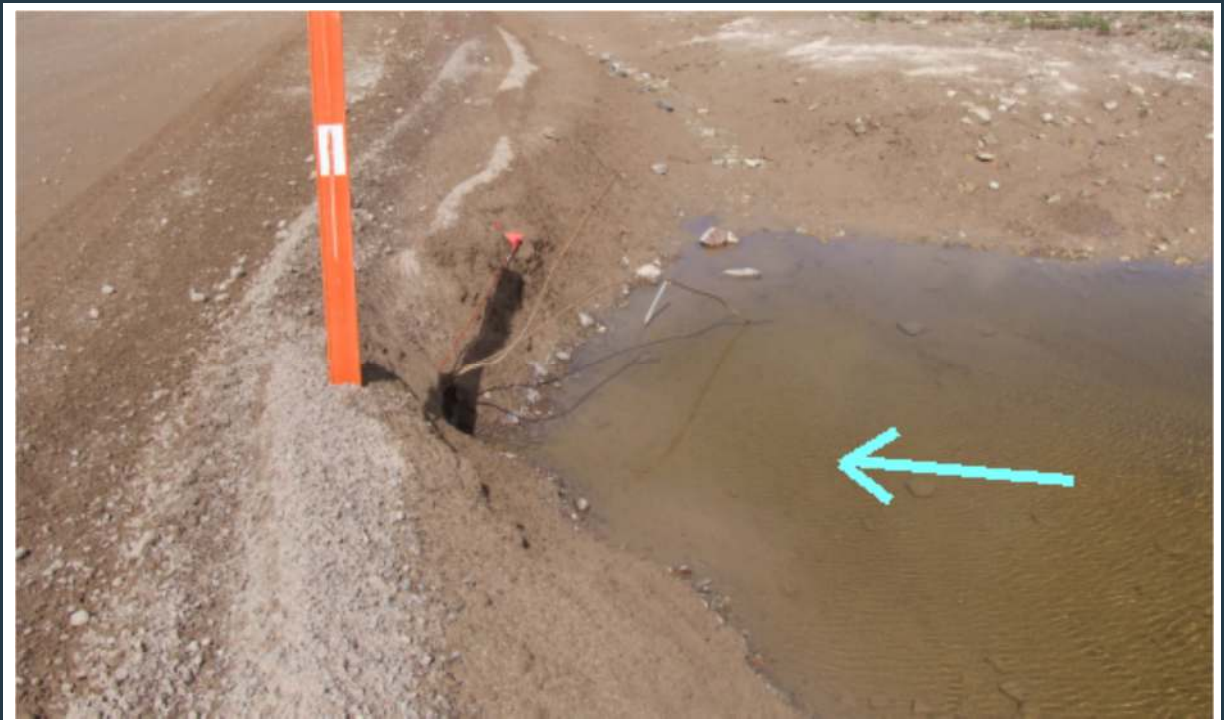
Figure 107: View of culvert 107 (inlet). Extension of the culvert and placement of riprap are required.
