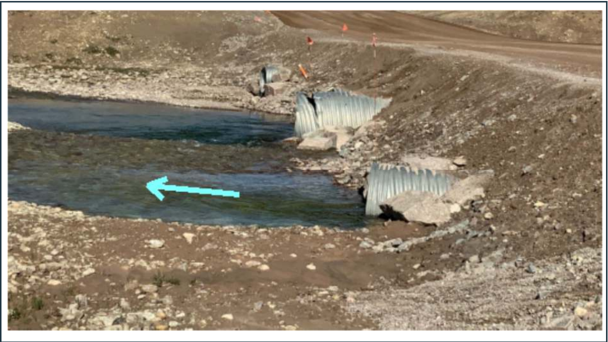
Figure 100: View of culvert(s) 078 (outlet). Minor damage visible on one pipe.
