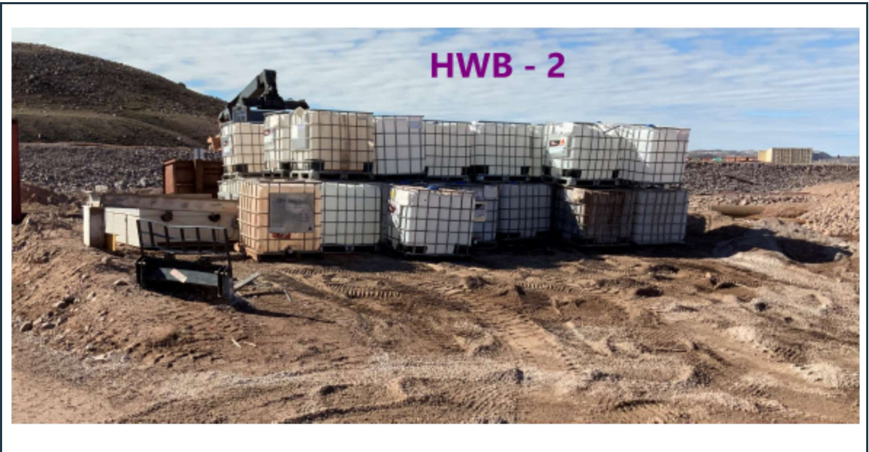
Figure 43: View of the former HWB-2 cell, with only empty containers stored on the top of clean sand and gravel fill pad. No hazardous waste is stored in this cell.
