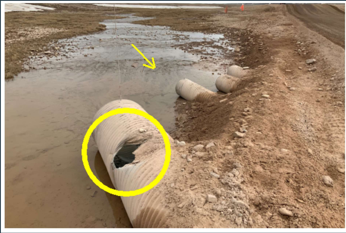
Figure 93: View of culvert(s) 102 inlets. Note the minor damage on one of the pipes (yellow circle).
