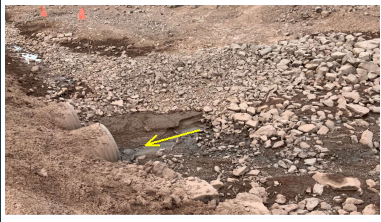
Figure 69: View of twin culverts, draining surface water from the quarry area under the tote road (inlet).
