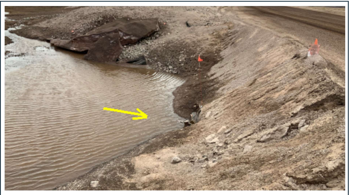
Figure 83: View of the inlet of culvert BG-038, with minor erosion on the slope of the road embankment.
