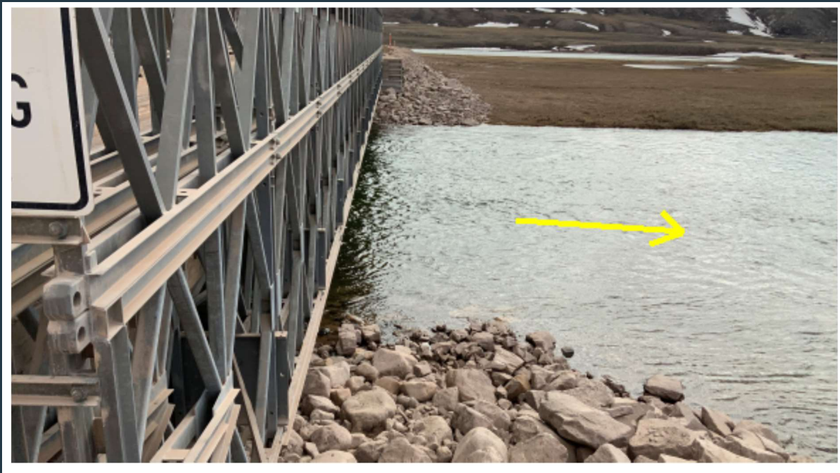
Figure 71: View of the north side of "bridge 17". Note the rip-rap scour protection at the abutments.
