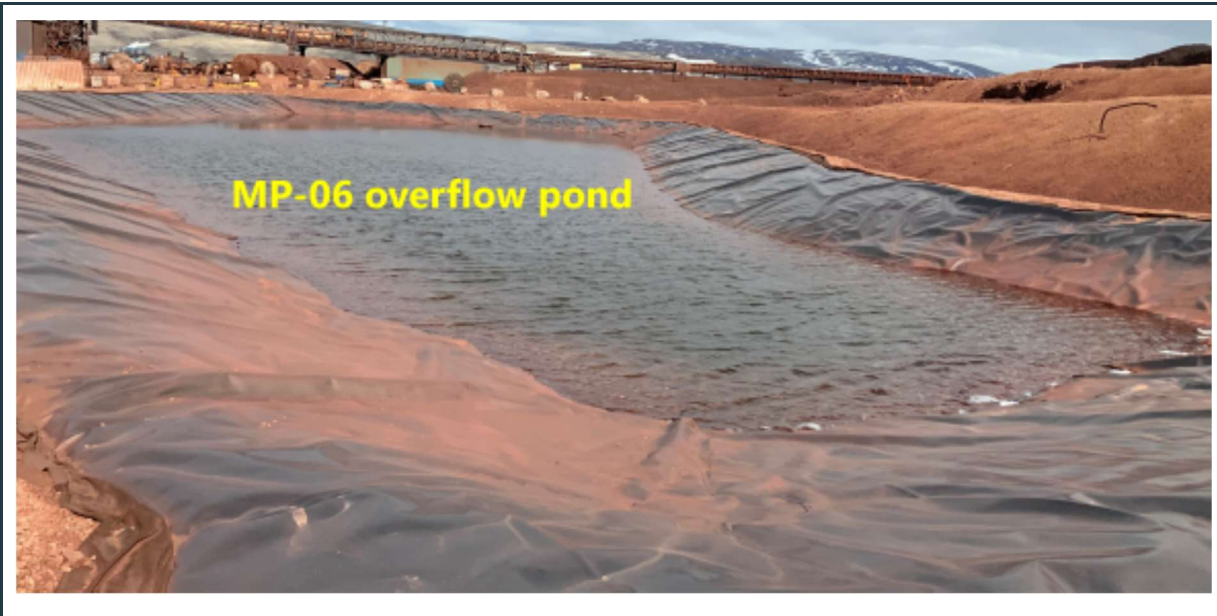
Figure 57: View of the lined MP-06 overflow pond, with stable berms.
