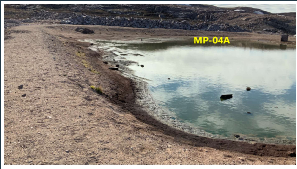
Figure 49: View of the MP-04A cell with stable berms and ponding melted snow.
