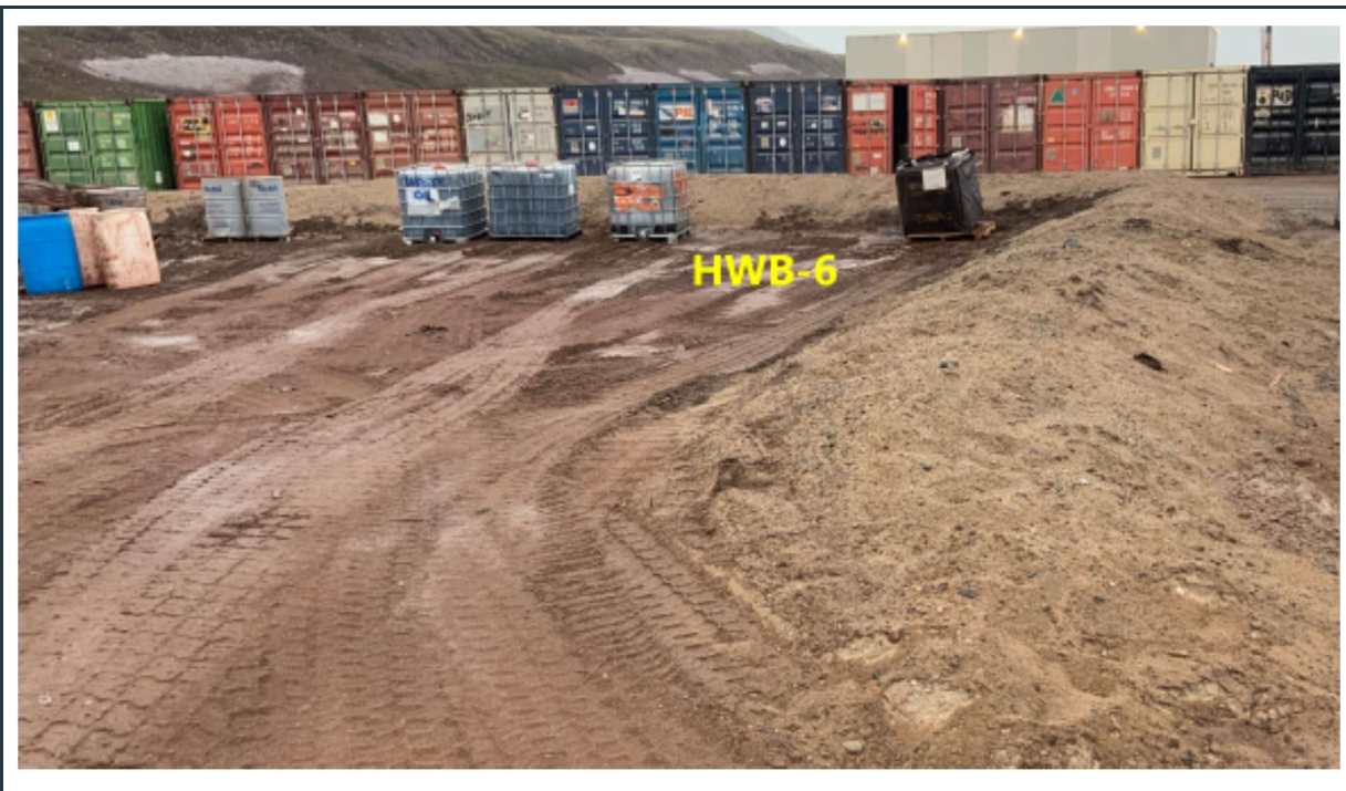
Figure 18: View of the recently upgraded stable berm and interior granular fill protecting the liner at the HWB-6 cell.
