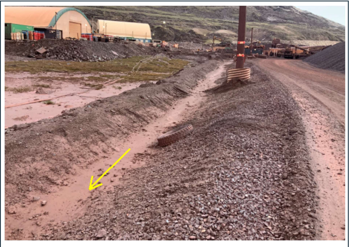
Figure 21: Well-maintained drainage ditch next to the crusher plant, leading to the MS-06 pond.
