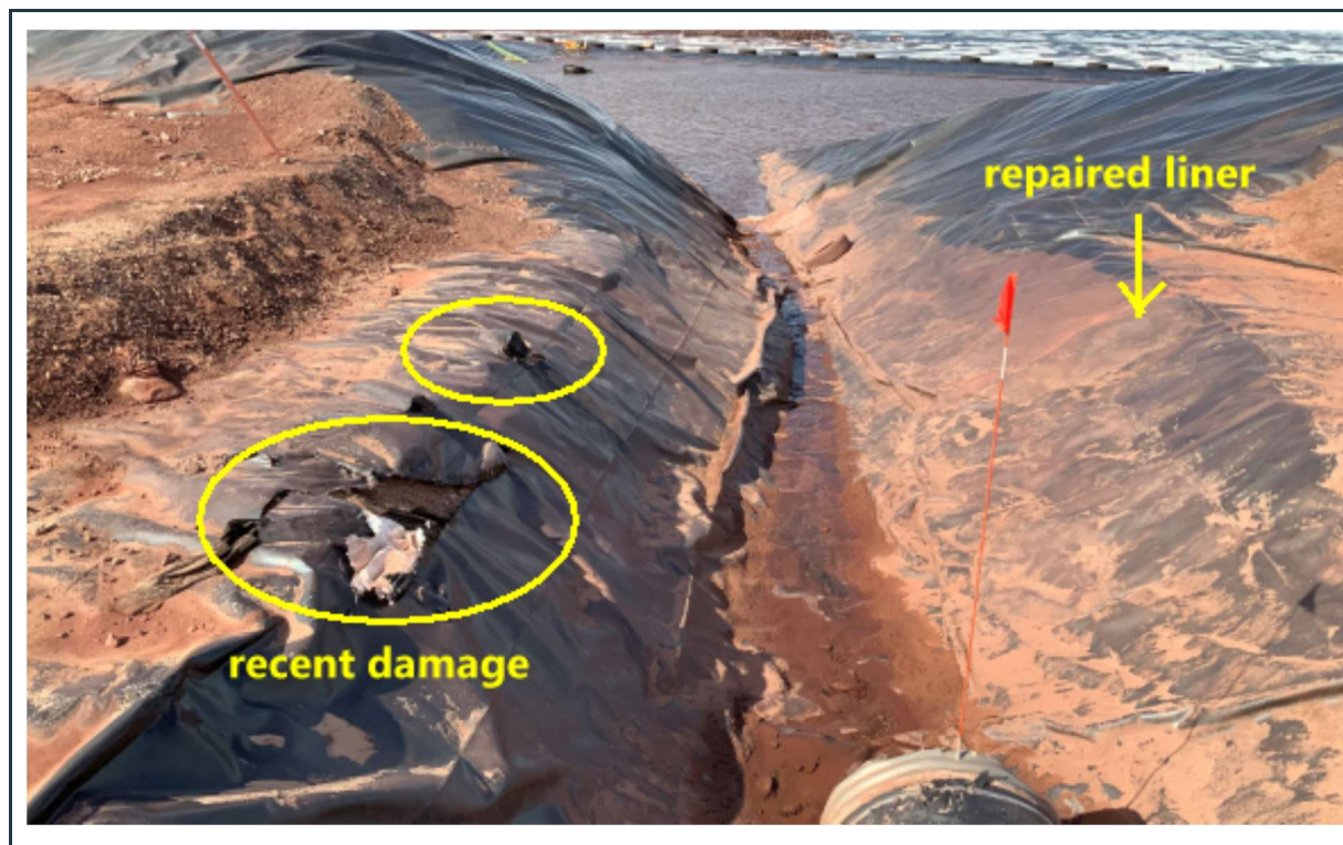
Figure 53: Some recent liner damage on the west slope of the southern intake channel.
