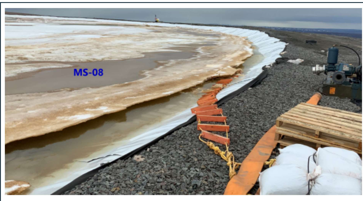
Figure 24: View of stable berm and intact liner at the MS-08 pond. Ice is still present at the end of June.
