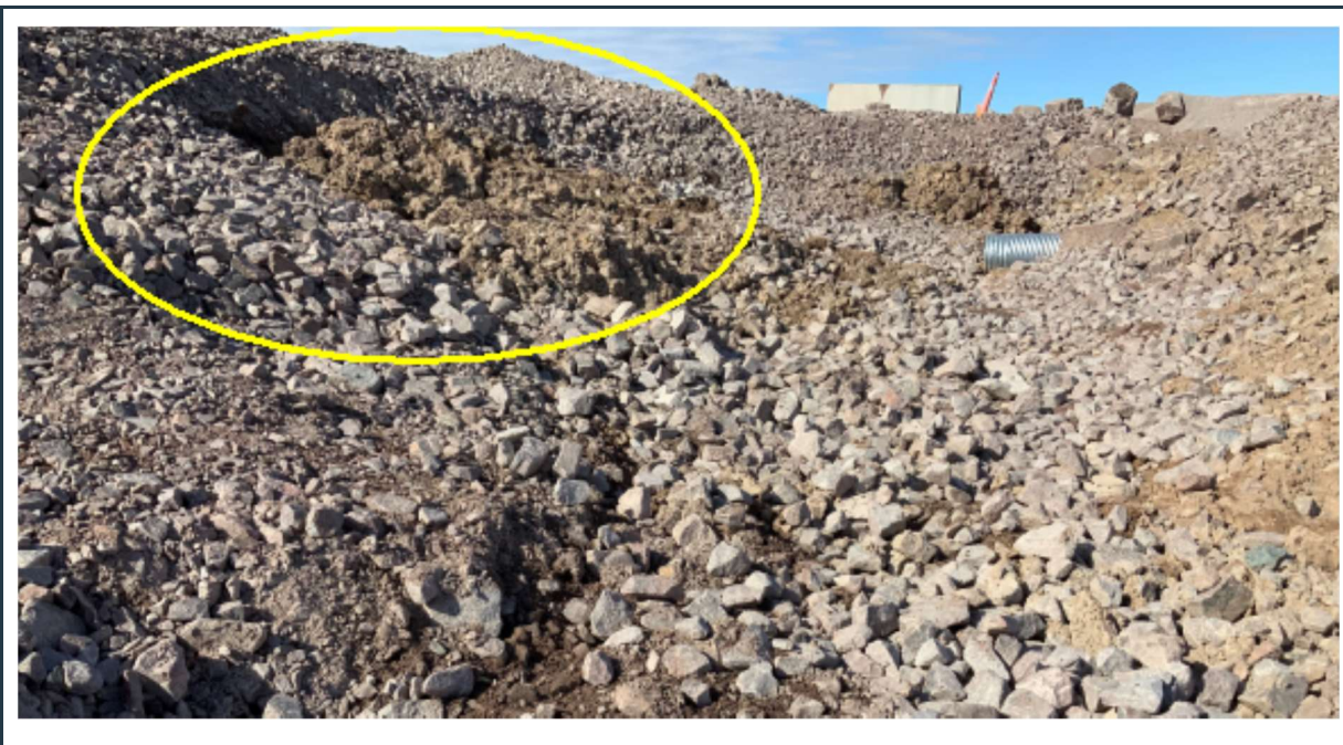
Figure 68: View of the PSC surface water collection ditch and culvert (still under construction). Note the localized slope failure on the left side of the image (yellow circle), which section will require slope rehabilitation with riprap placement.
