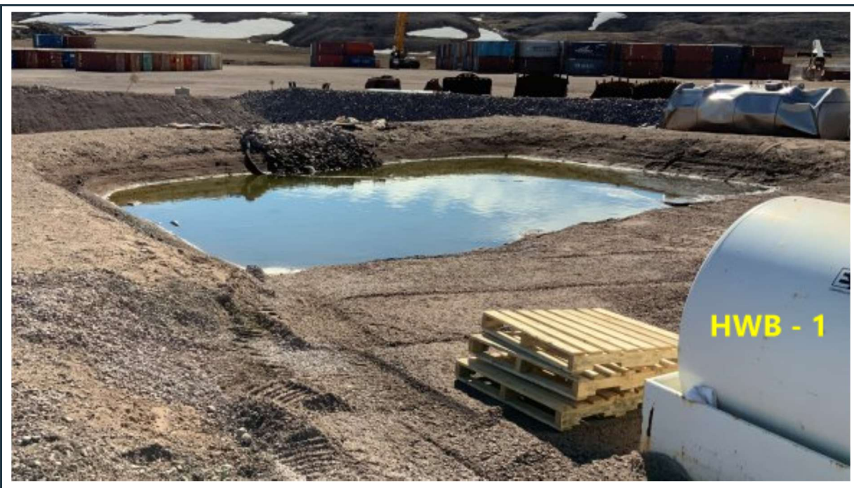
Figure 42: View of the back of the HWB-1 cell, with ponding water and upgraded (regraded) cell floor.
