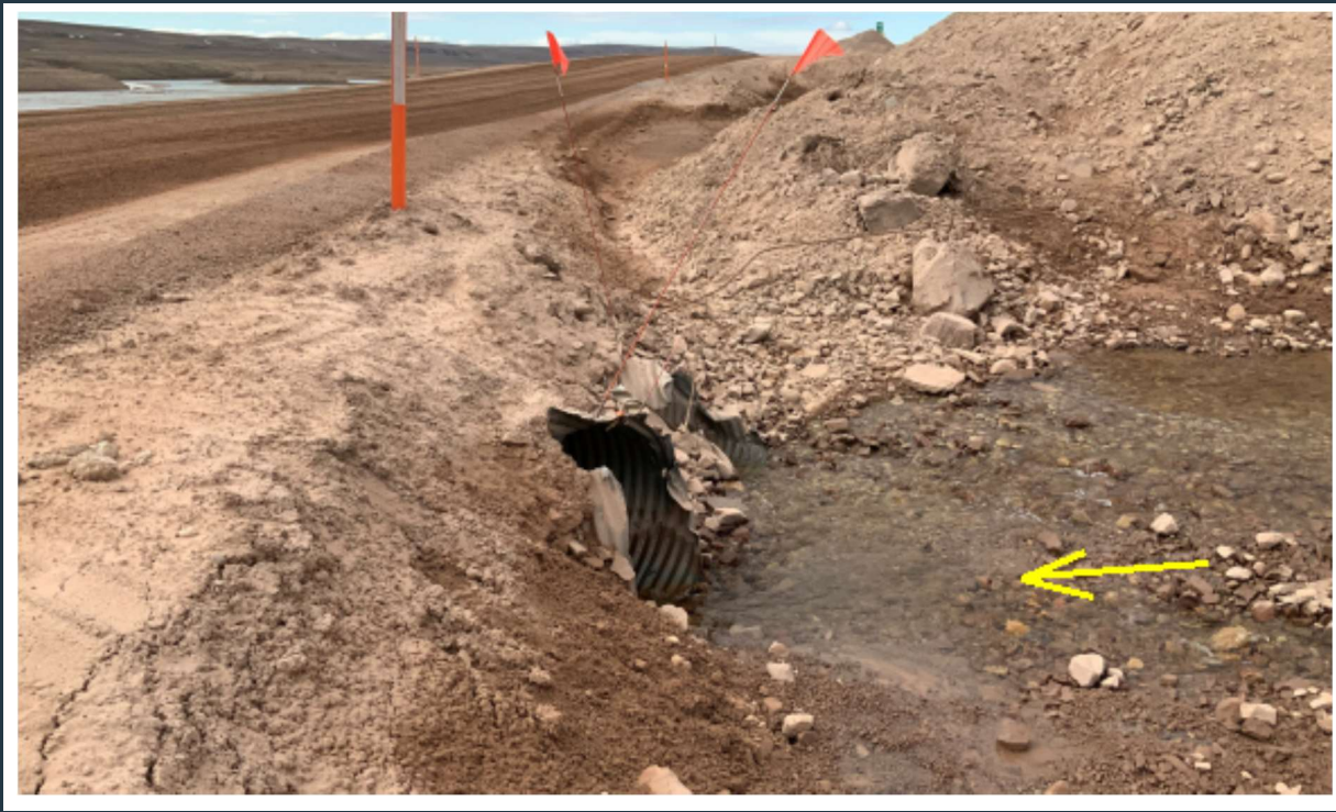
Figure 103: View of culvert(s) 114D inlets. Repair of both pipes is required.
