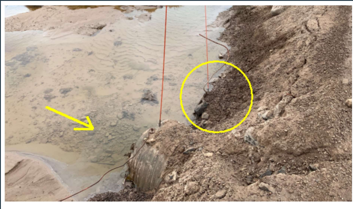
Figure 81: View of the inlet to culverts 030A and B. Note that one of the pipes is clogged (yellow circle).
