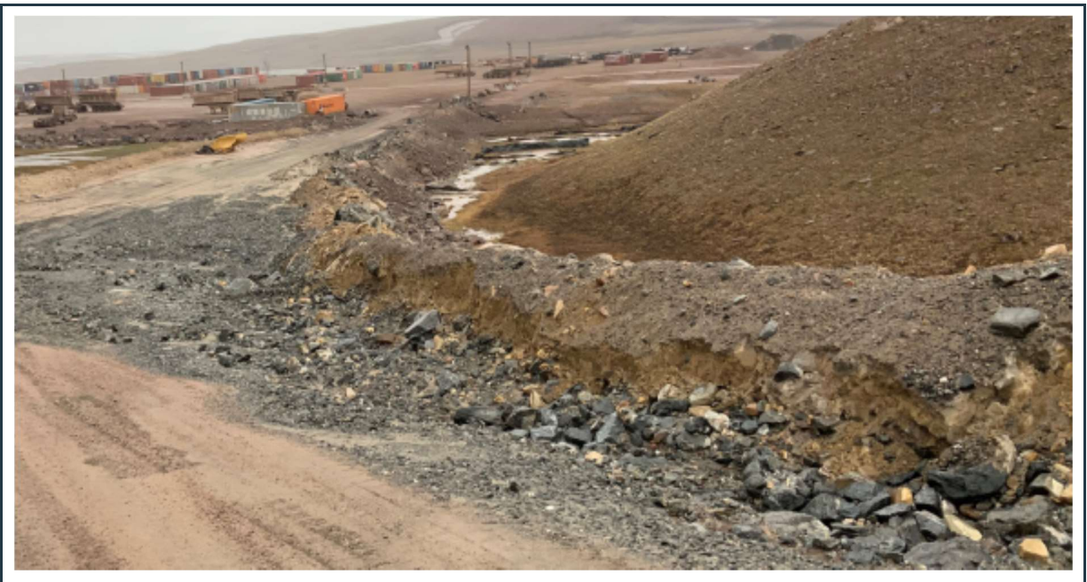
Figure 38: Erosion and stability problem along the access road to the quarry.
