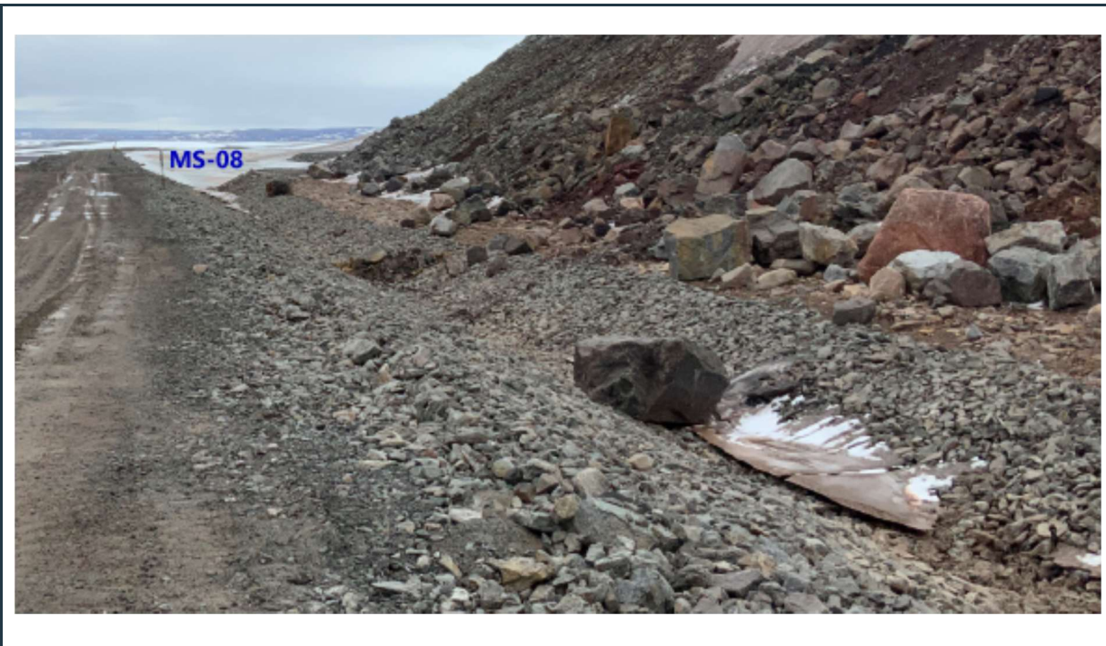
Figure 25: Drainage ditch around the west side of the waste rock facility. Boulders should be removed.
