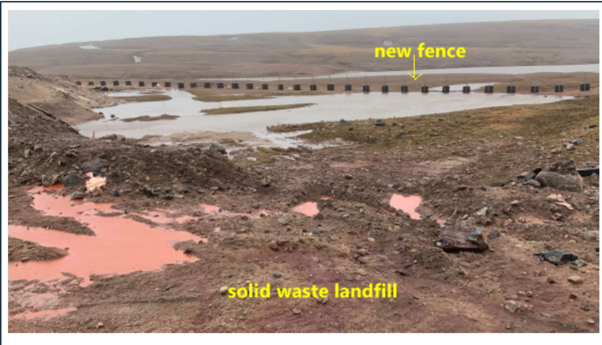
Figure 33: Solid waste landfill facility with ponding water along a section of the new perimeter fence.
