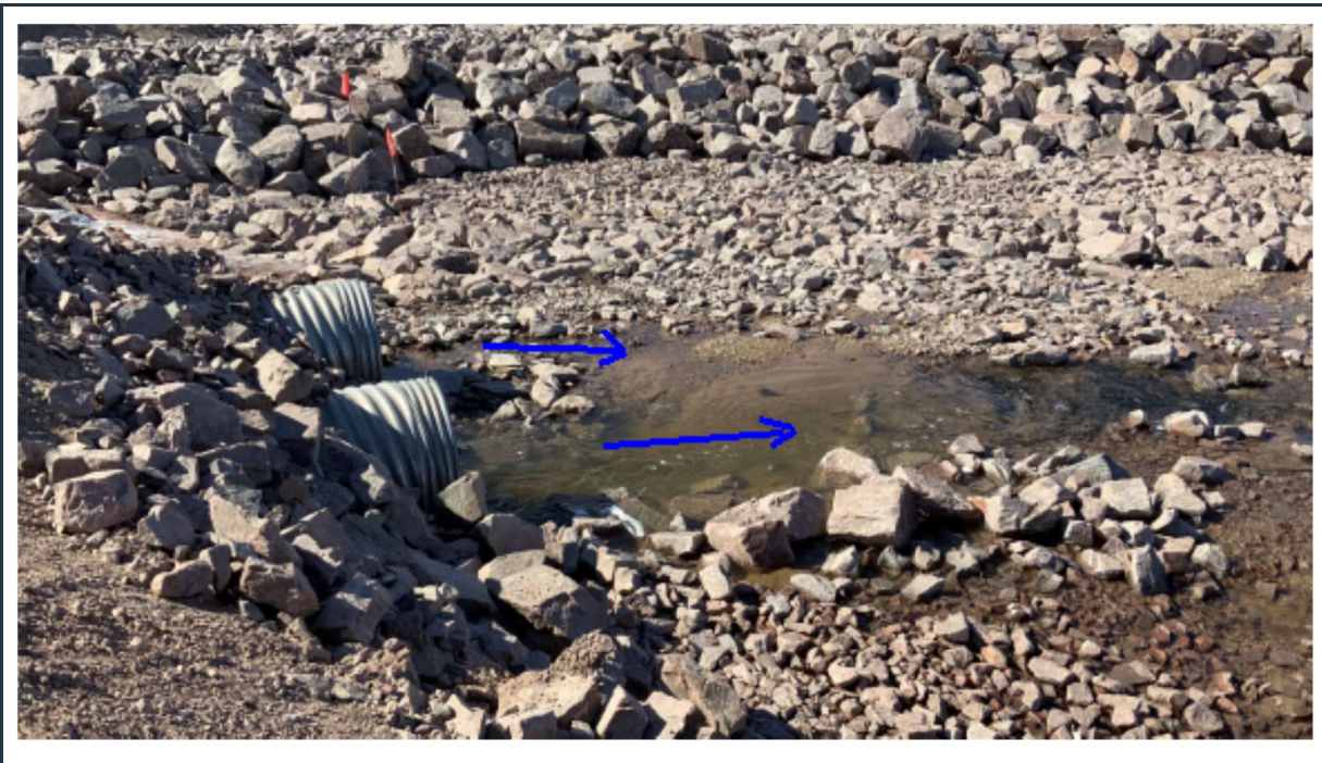
Figure 64: View of the P-SWD-7 surface water collection ditch and culverts (outlet).
