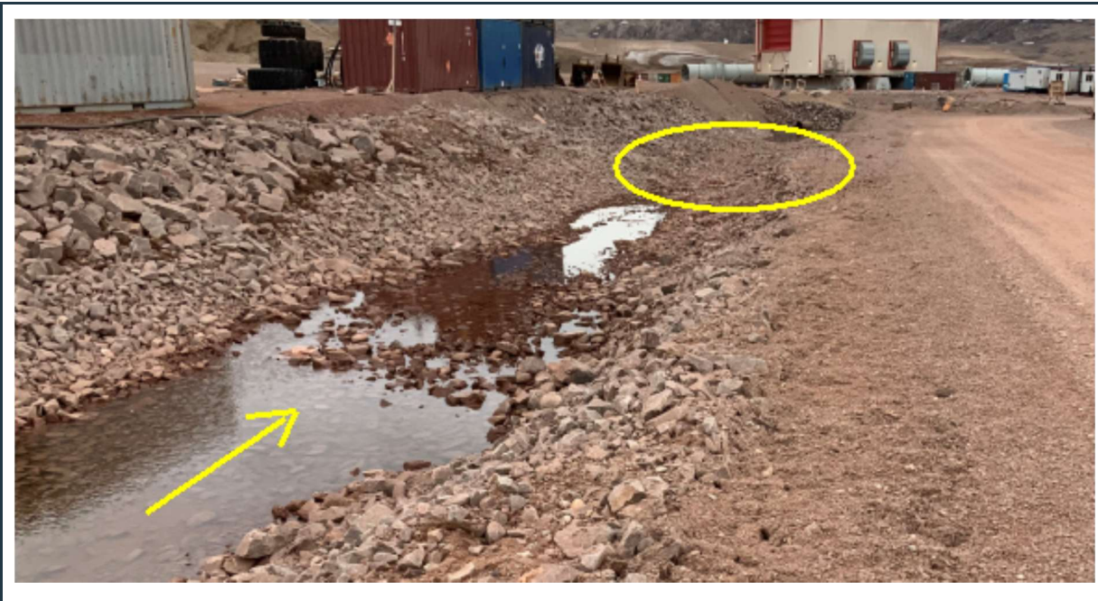
Figure 67: View of the east section of the 380 M surface water collection ditch.
