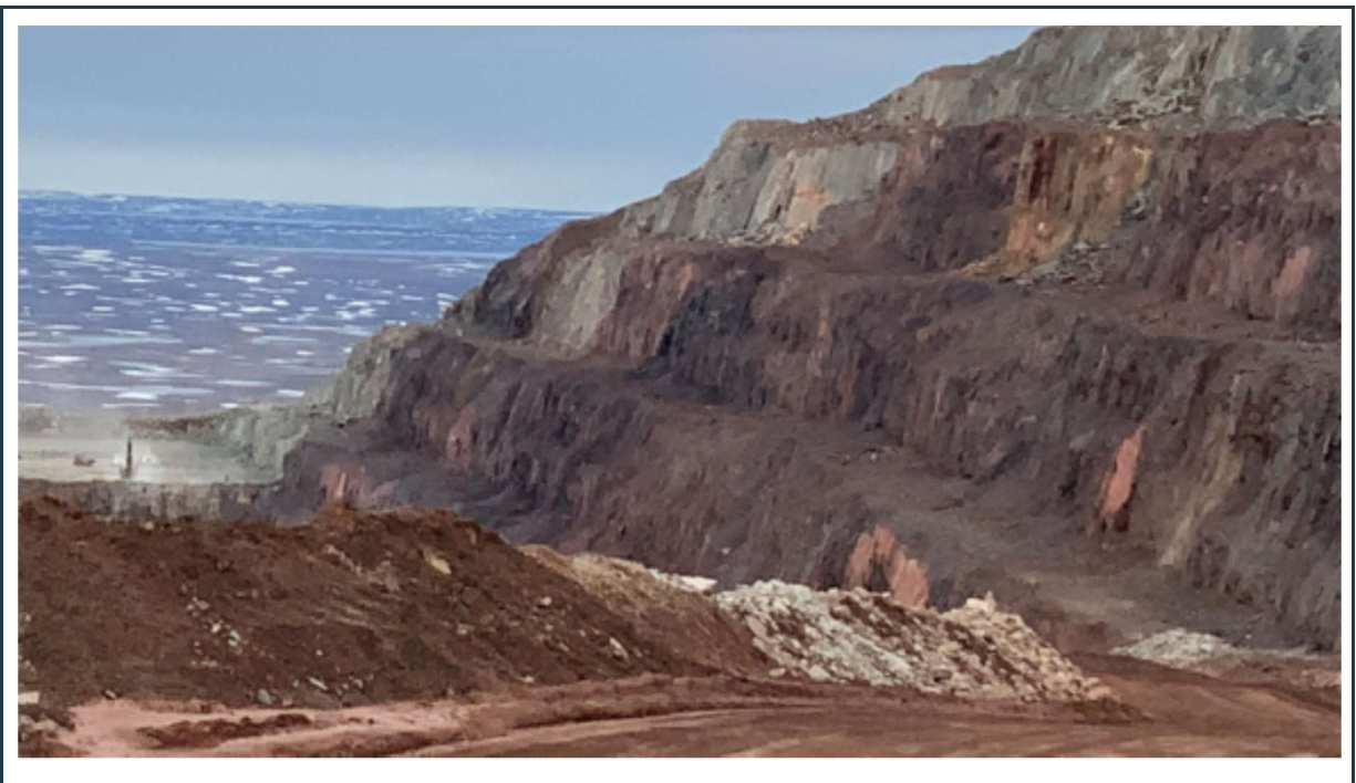
Figure 36: Stable pit-walls with minor rock weathering and pit-wall erosion.
