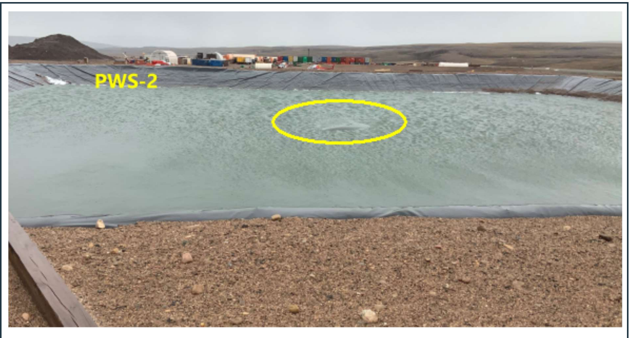
Figure 11: PWS pond #2 – Stable, well-maintained berm around the pond. – A small “floating” section of the liner is visible in the center of the pond (yellow circle).
