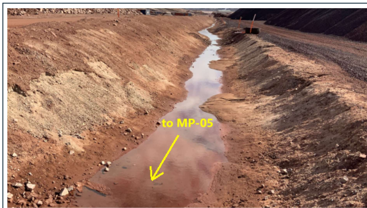
Figure 54: Surface water collection ditch adjacent (east) to the ore storage, draining to the MP-05 pond.
