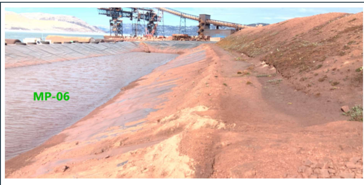
Figure 56: View of the east slope of the lined MP-06, with increased soil erosion from the adjacent berm.
