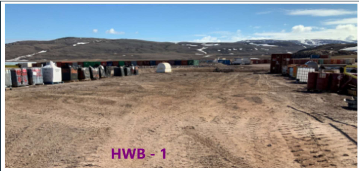
Figure 41: View of the practically empty HWB-1 cell with upgraded (regraded) cell floor.
