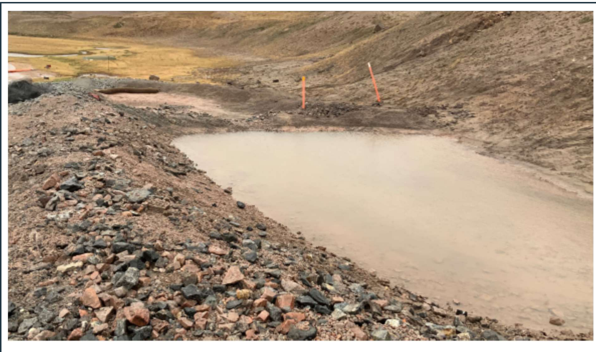
Figure 34: Camp Lake check dams and berms, constructed around the silt sedimentation cells.
