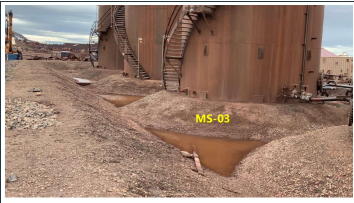
Figure 31: Well-maintained, stable berms around the MS-03 diesel fuel farm, with some ponding water.
