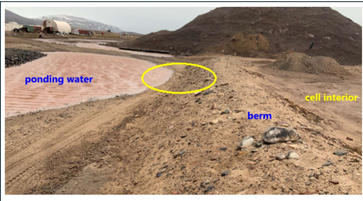
Figure 29: View of ponding water adjacent to the north-east berm of the “fuel bladder” cell. Trucks bypassing the ponding water on the road are “cutting” into the toe of the berm (yellow circle).
