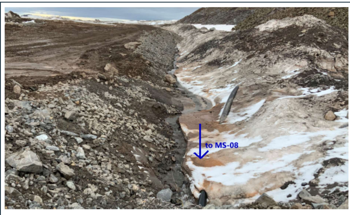
Figure 26: Snow-filled drainage ditch around the east side of the waste rock facility, leading to the MS-08 pond.
