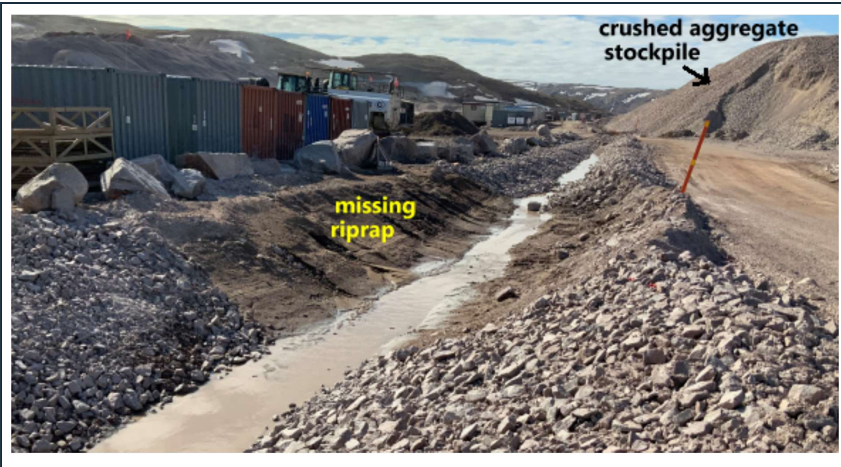
Figure 61: P-SWD-5 – “Q01-North” surface water collection ditch with missing riprap at a short section.
