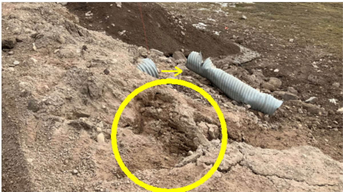
Figure 98: View of culvert 110A outlet. Note that a section of the pipe was cut off, and the erosion of the road embankment adjacent to the culvert (yellow circle).
