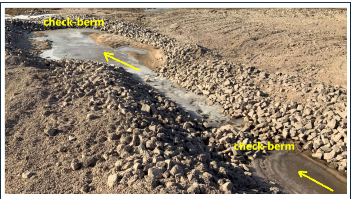
Figure 78: View of the check-dams downstream of the culvert at KM33, shown above.
