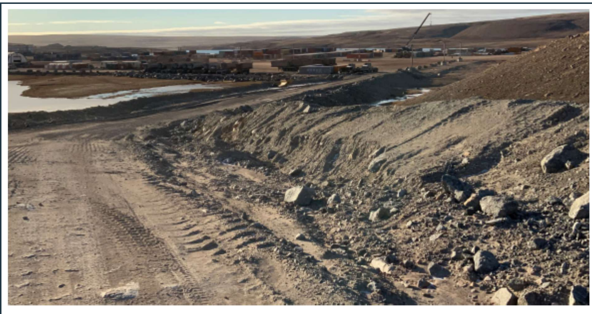
Figure 38: Erosion and stability problem along the access road to the quarry.
