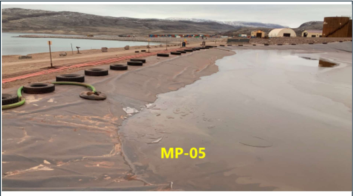
Figure 51: View of the stable berms and intact liner at the MP-05 settling pond.
