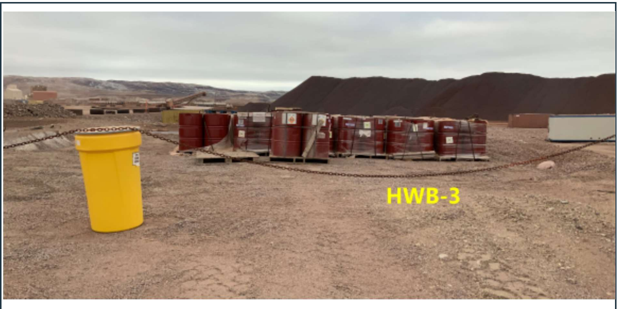
Figure 44: View of the HWB-3 cell with stable berms, containing fuel barrels.
