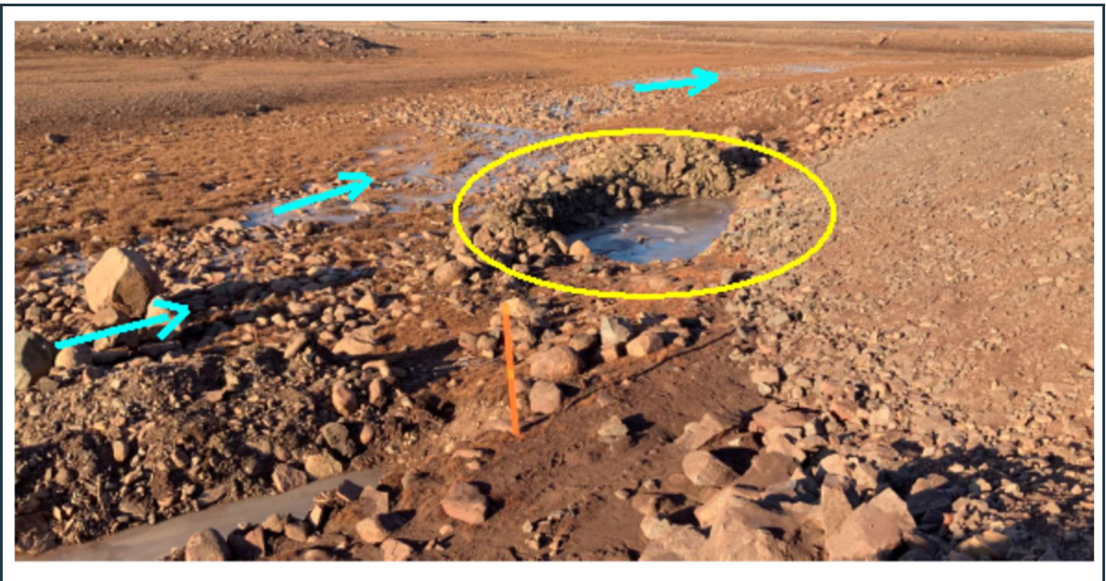
Figure 22: Seepage water within the relatively permeable, cobbly overburden adjacent to the area of the crusher pad and MS-06 pond. It appears to be surface water, percolating down into the ground and flowing from higher elevations within the valley adjacent to the crusher pad. The excavated hole (temporary sump) at the toe of the MS-06 berm must be filled (yellow circle).
