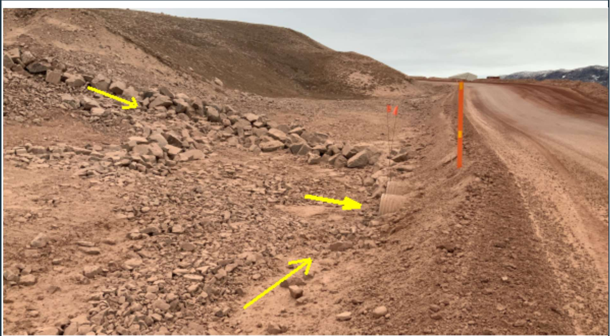
Figure 67: View of twin culverts, draining surface water from the quarry area under the tote road (inlet).
