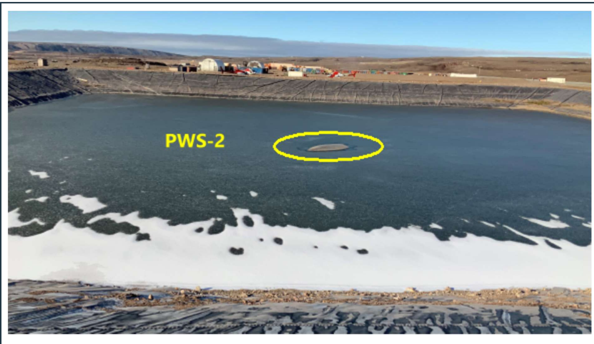
Figure 11: PWS pond #2 – Stable, well-maintained berm and liner. – A small section of the liner is visible in the center of the pond (yellow circle). Note the ice formation in the pond in September.
