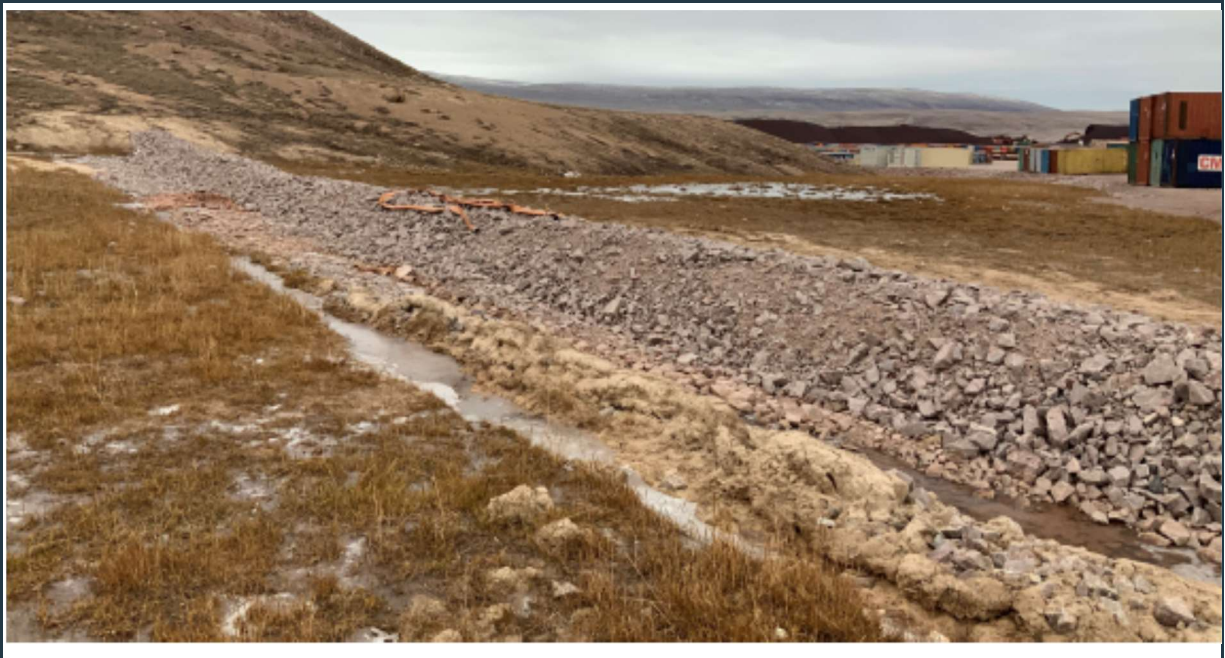
Figure 57: View of a section of the P-SWD-3 surface water collection ditch with failed side slope. The failure of the ditch was caused by the uncontrolled water flow from the adjacent snow pile.
