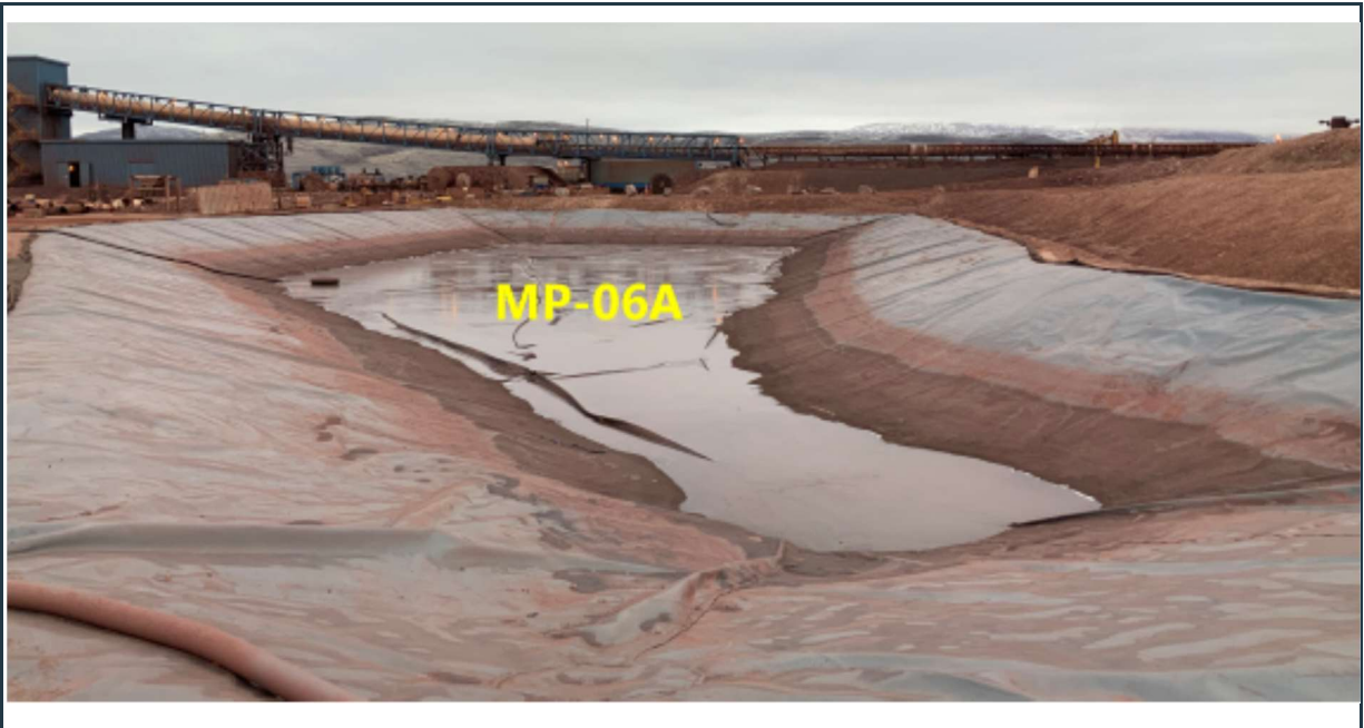
Figure 55: View of the lined MP-06A overflow pond, with stable berms.
