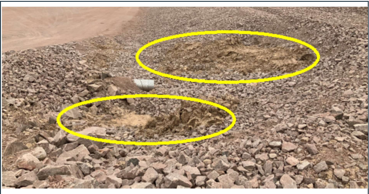
Figure 66: View of the PSC surface water collection ditch and culvert (still under construction). Note the localized slope failures (yellow circles), which sections will require slope rehabilitation with riprap placement.
