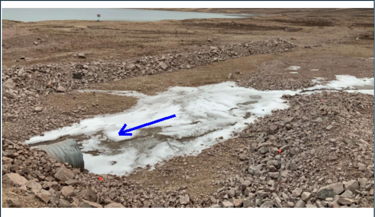
Figure 61: View of the P-SWD-7 surface water collection ditch and culverts (inlet).
