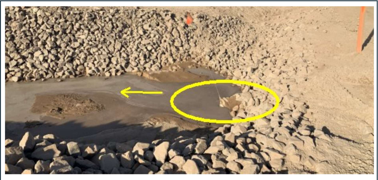
Figure 77: View of the outlet of a culvert at KM33 near the lake access check-dams. Note that the ditch and culvert are full with silt, they should be cleaned.
