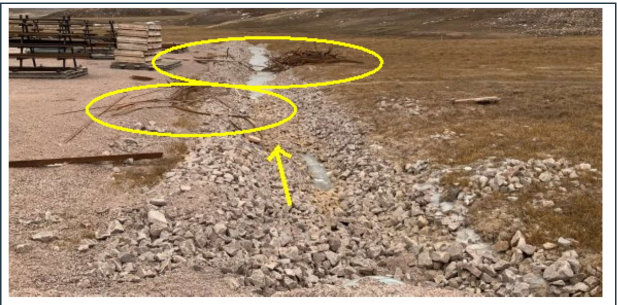
Figure 58: View of the north end of the P-SWD-3 surface water collection ditch. All debris should be removed from the ditch (yellow circles).
