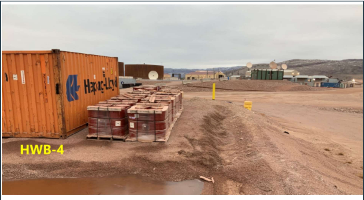
Figure 45: Stable berms around and ponding water within the HWB-4 cell, storing jetfuel and containers.
