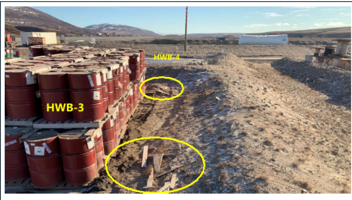
Figure 15: View of stable berms and stored fuel barrels in HWB-3. Wooden debris should be removed.
