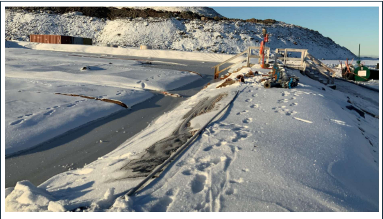
Figure 27: Stable berm and intact liner at the water treatment pond, adjacent to the waste rock facility.
