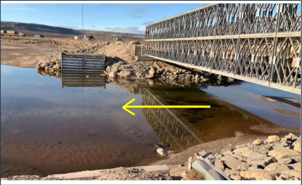
Figure 73: View of the west side of bridge 80, with the "old" abutment providing additional support.
