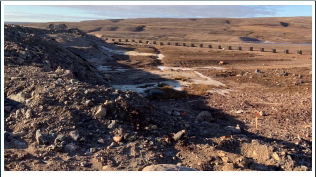
Figure 33: Solid waste landfill facility with some ponding water adjacent to the soil-covered waste.
