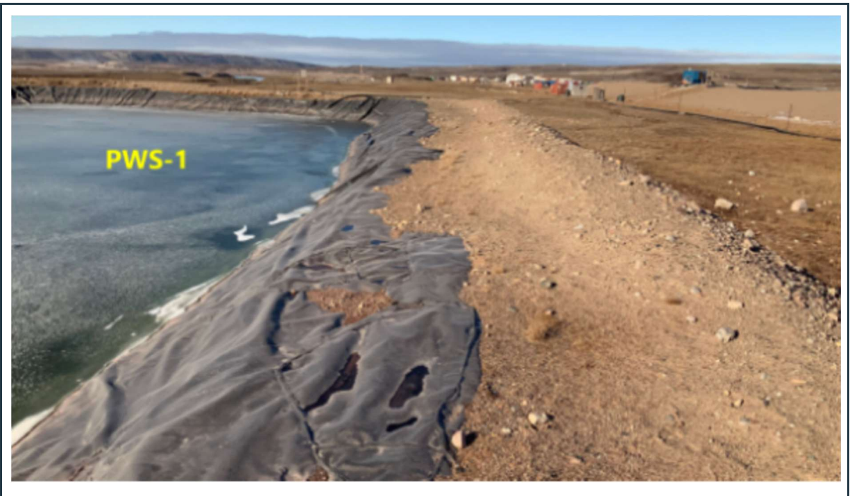
Figure 10: PWS pond #1. Well-maintained, stable perimeter berm and liner.
