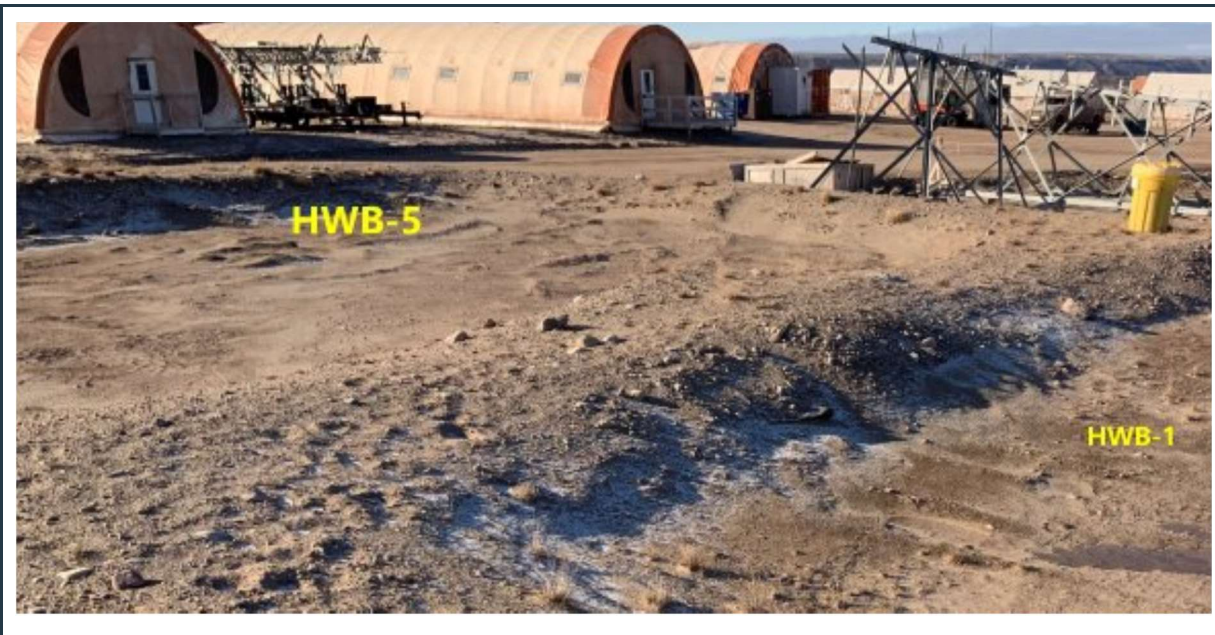
Figure 17: View of the berms around the currently empty HWB-5 cell, adjacent to the HWB-1 cell.
