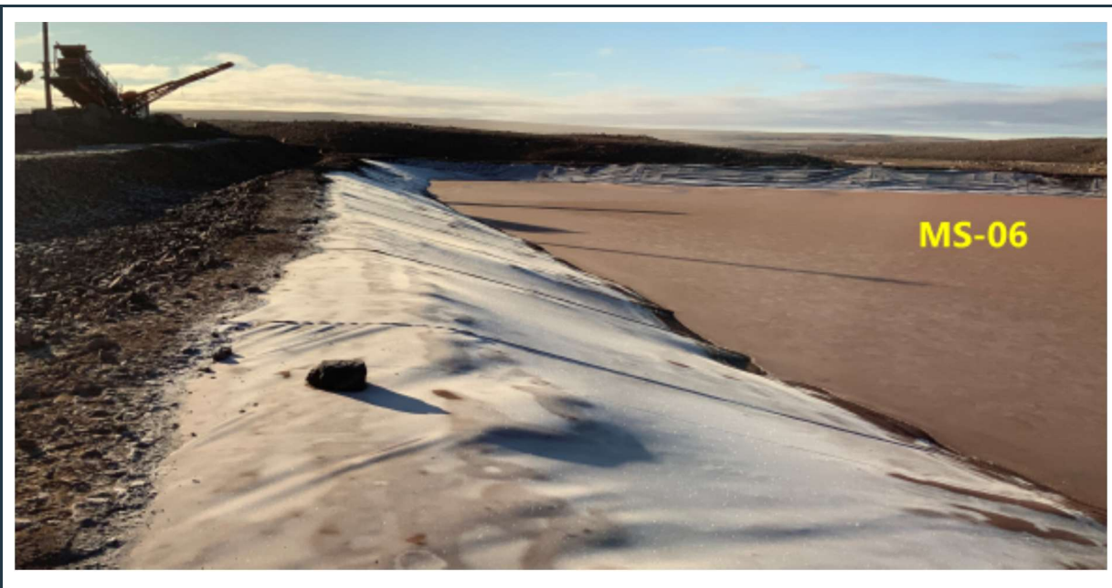
Figure 20: MS-06 settling pond with robust, stable berms and intact liner.
