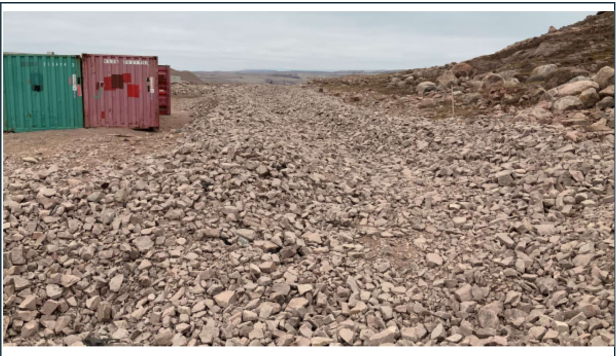
Figure 60: View of the rock fill lined P-SWD-6 surface water collection ditch.
