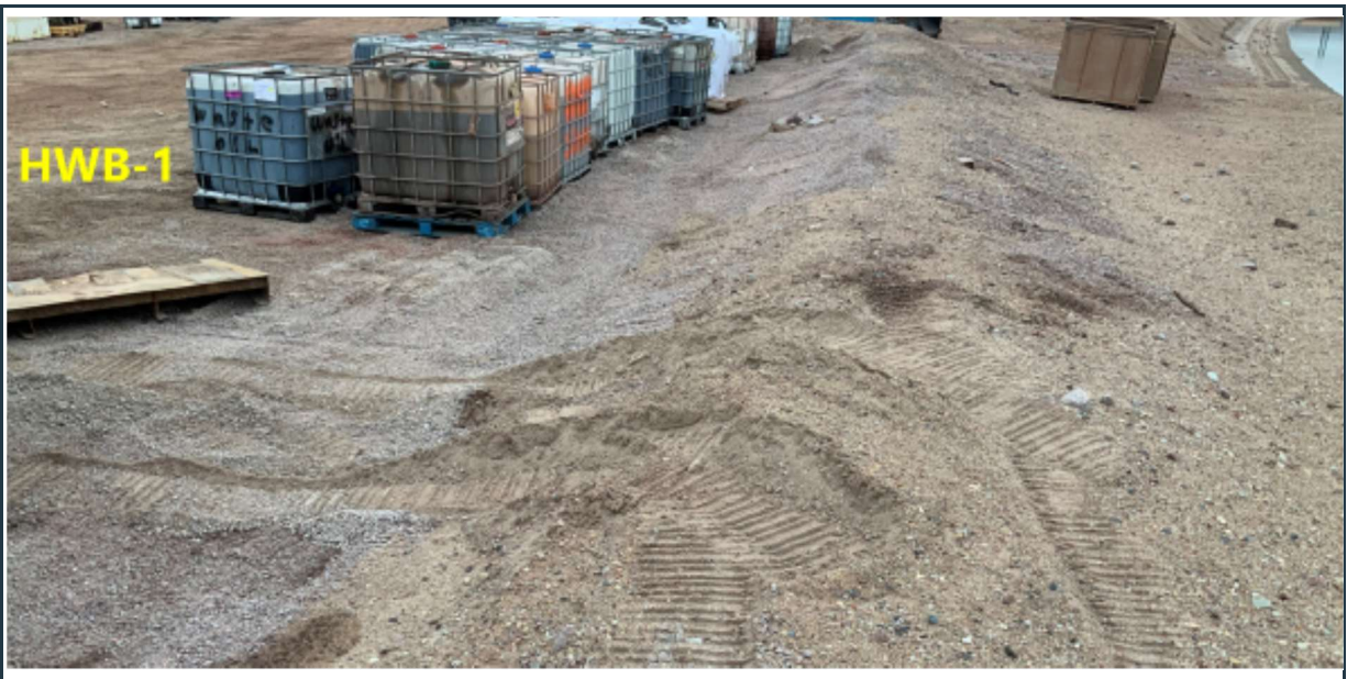
Figure 42: View of one of the berms with tire-tracks. Driving trucks on the berms should be avoided.
