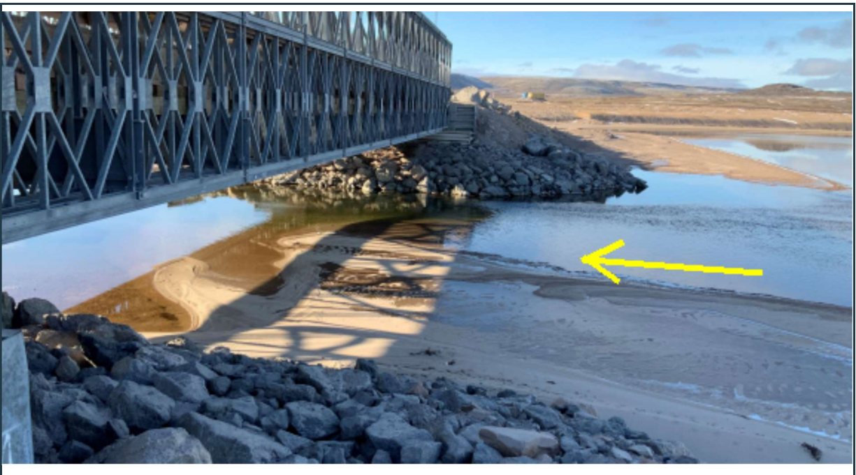
Figure 74: View of stable abutments at bridge 80. Note the low flow in September.
