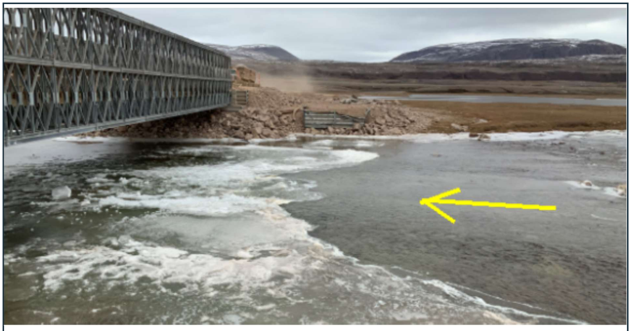
Figure 70: View of the south side of "bridge 17", with stable abutments.
