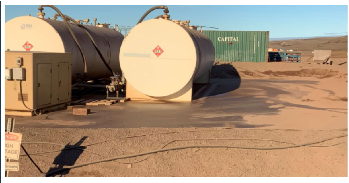
Figure 30: View of the well-maintained sand and gravel berm at the lined jet-fuel storage facility. The ponding water within the cell indicates good liner performance.
