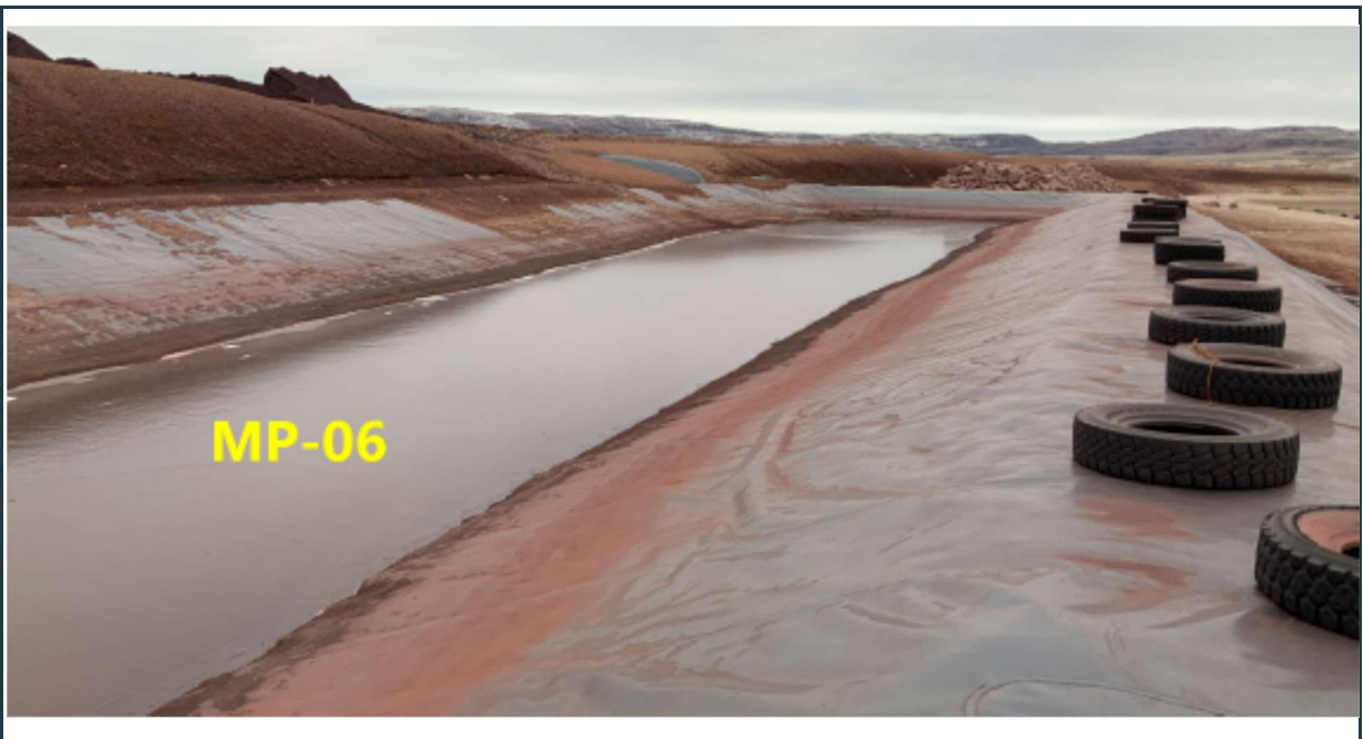
Figure 54: View of the lined MP-06 pond with robust, stable berms.
