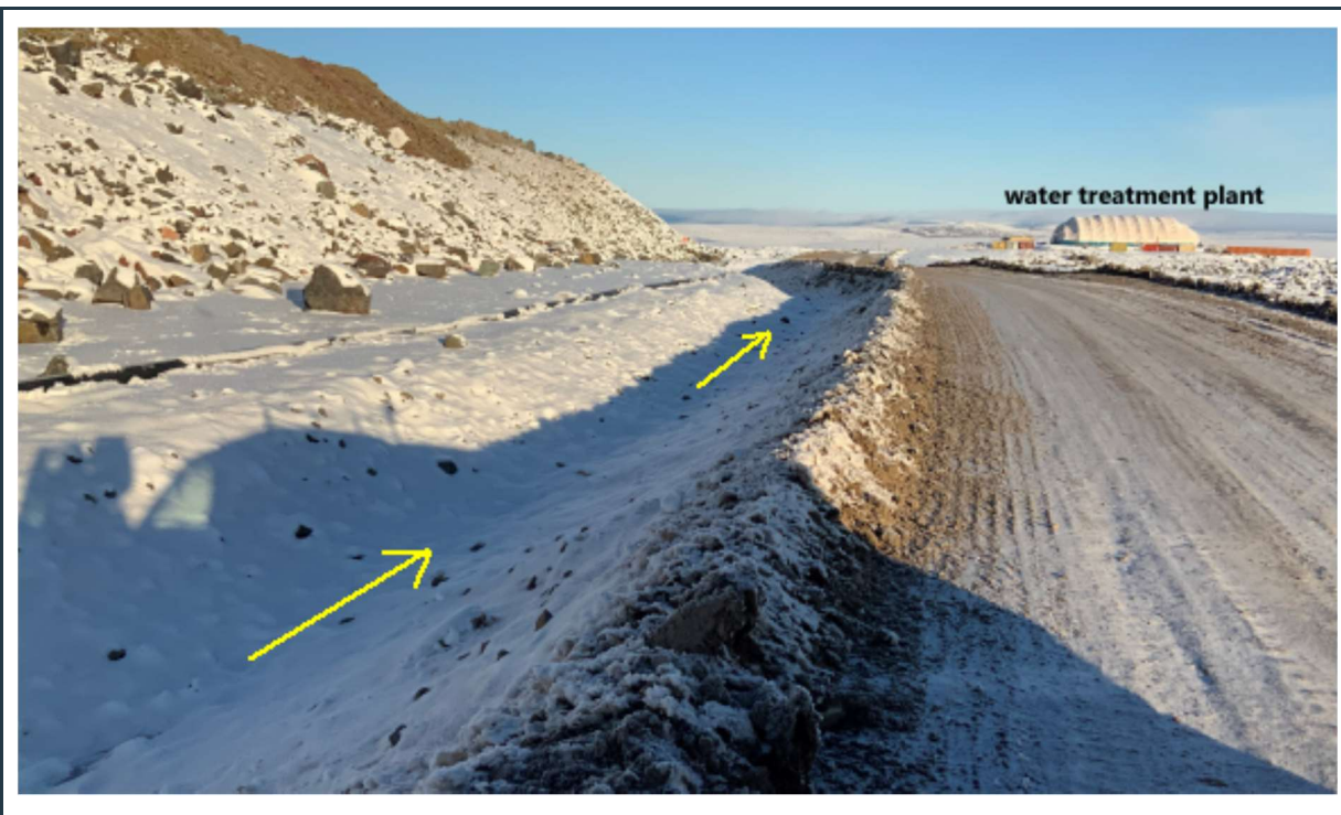
Figure 26: Snow visible in the drainage ditch around the east side of the waste rock facility, leading to the MS-08 pond. Note the water treatment plant at the site.
