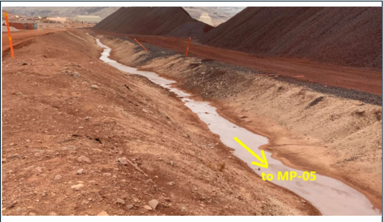
Figure 53: Surface water collection ditch adjacent (east) to the ore storage, draining to the MP-05 pond.
