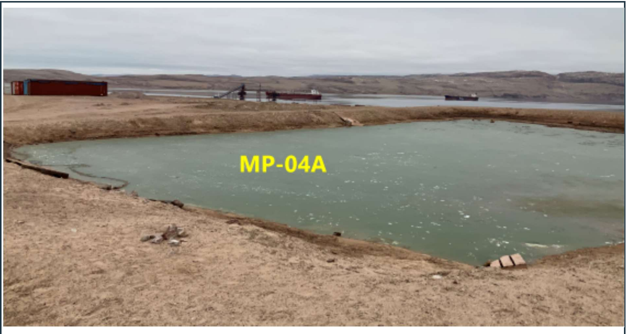
Figure 49: View of the MP-04A cell with stable berms. The ponding water indicates good liner performance.
