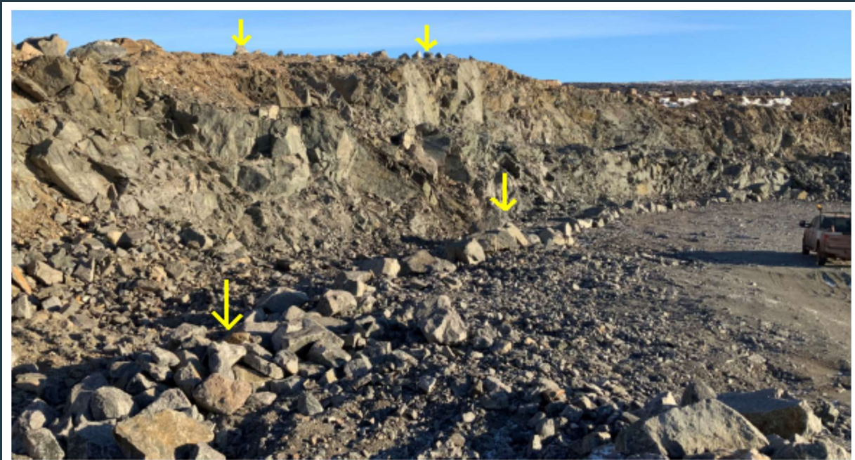
Figure 37: View of the rock face at the upper quarry level with some potential rolling rock hazard. Note the row of boulders placed on the crest and toe of the rock face to prevent unauthorized access to the wall. No activity is currently carried out in this quarry.
