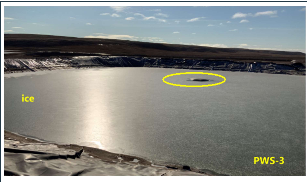
Figure 12: Stable perimeter berms around PWS pond #3 – A small section of the liner is visible in the shallow water of the pond (yellow circle).
