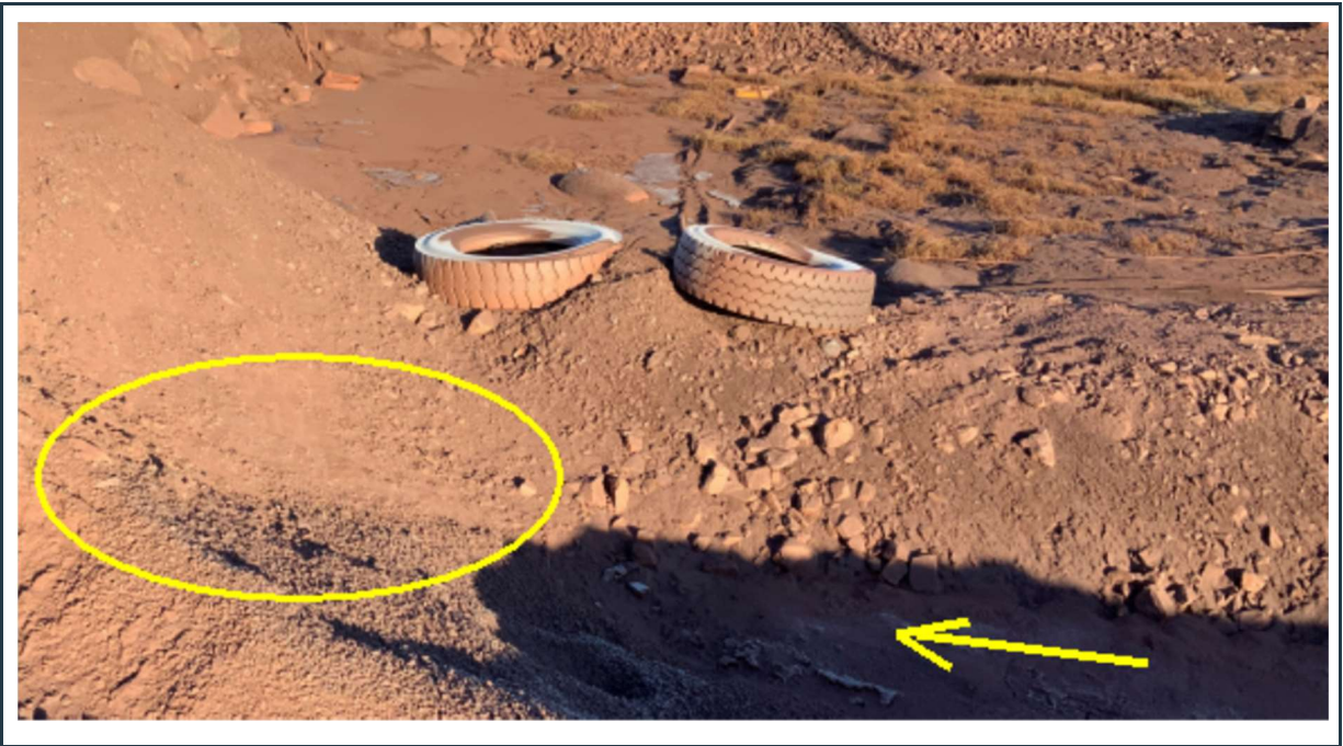
Figure 21: Drainage ditch next to the crusher plant leading to the MS-06 pond. The yellow circle indicates that the entry to the culvert that should drain the collected surface water from the ditch to the MS-06 pond is clogged, and it should be cleaned.
