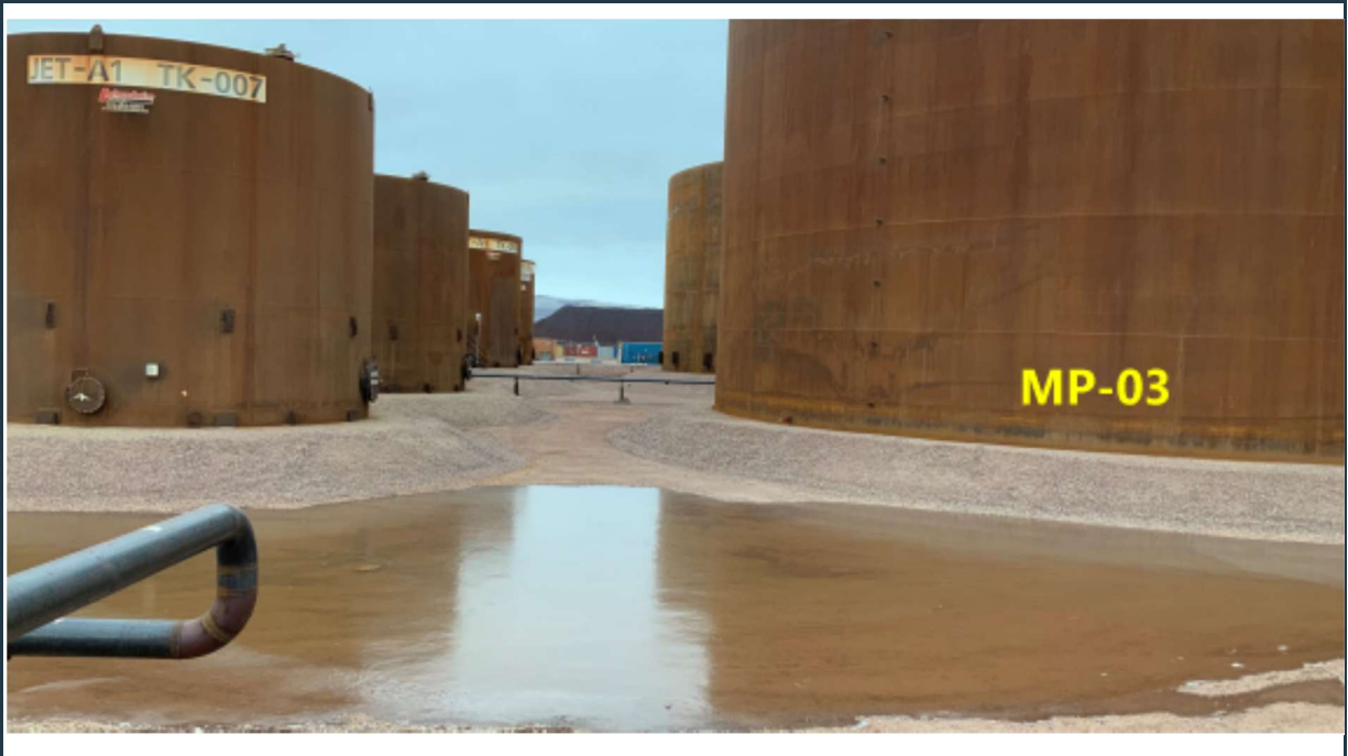
Figure 47: View of the well maintained MP-03 fuel tank farm. The ponding water indicates good liner performance.
