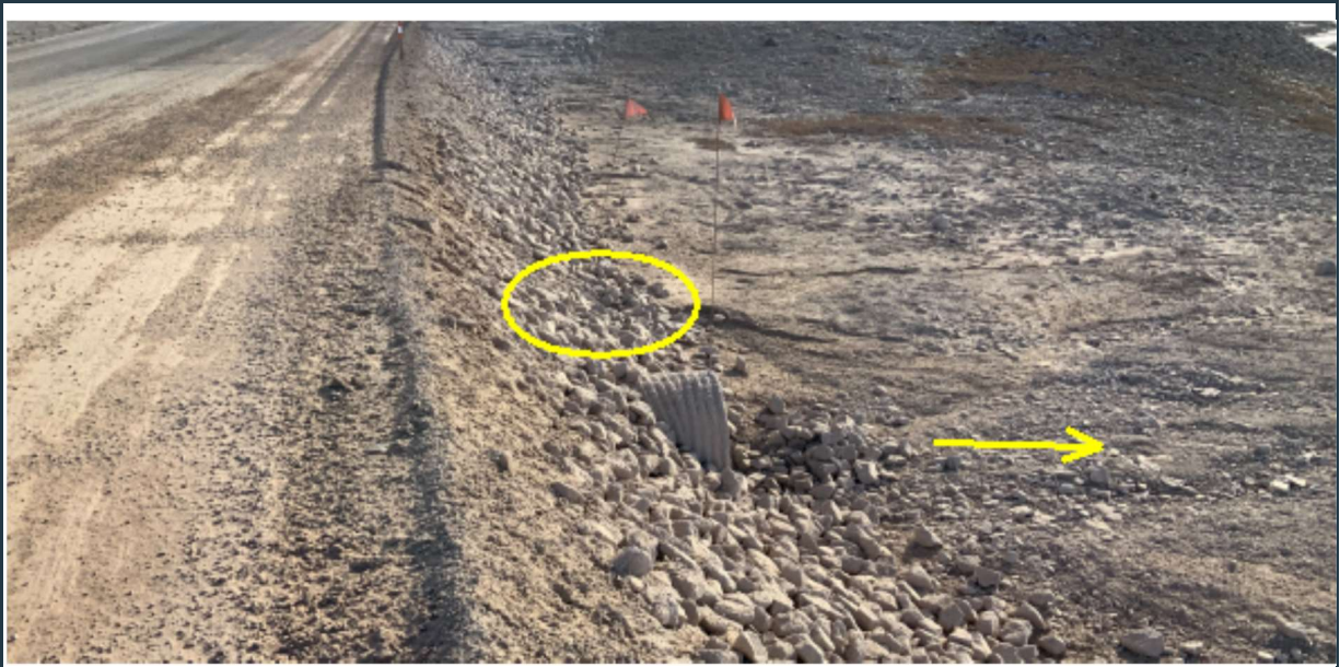
Figure 83: View of the outlet of the culverts. The end of one of the culverts is partially blocked by rock fill that should be removed from the front of the pipe and spread around the outlet (yellow circle).
