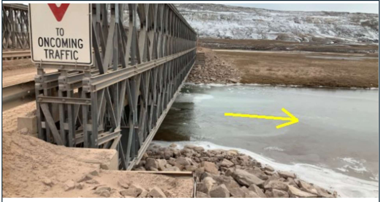
Figure 69: View of the north side of "bridge 17", with stable rip-rap scour protection at the abutments.
