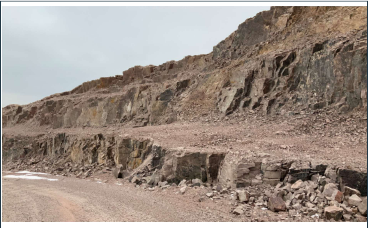
Figure 56: View of stable highwalls with minor weathering and bench erosion in the Q01 rock quarry.
