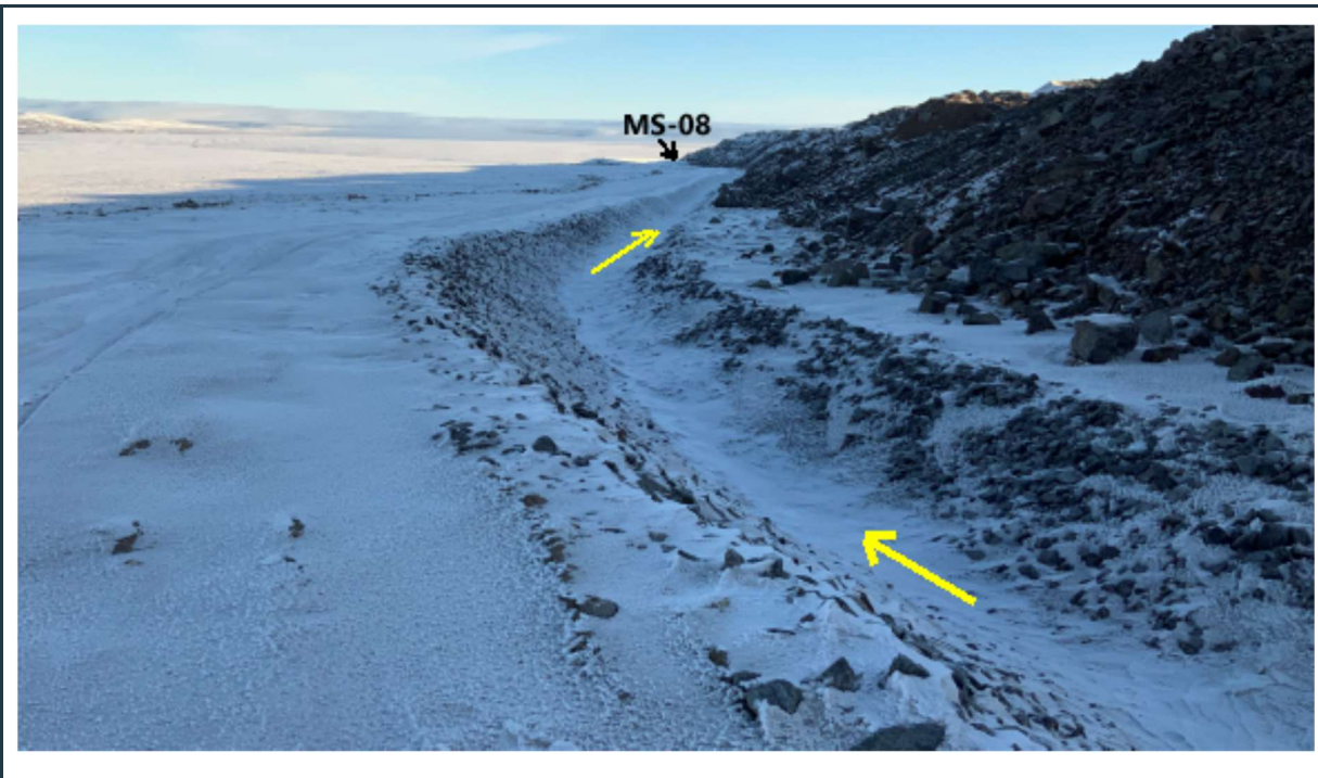
Figure 25: Drainage ditch around the west side of the waste rock facility.
