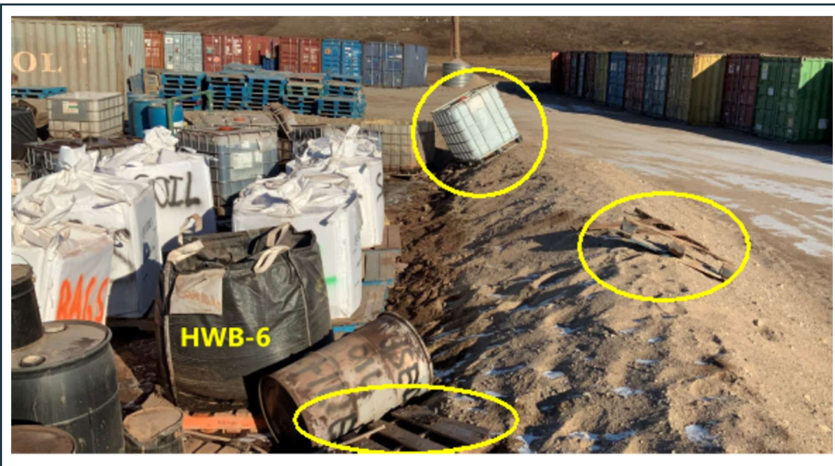
Figure 18: View of the now full HWB-6 cell. Note a container and some wooden debris placed on the berm instead of inside the cell. Those items should be placed inside the cell and the berm shall be regraded.
