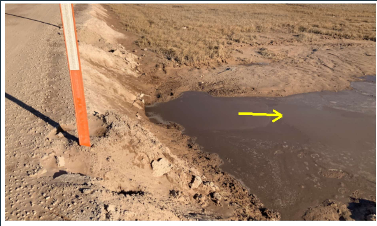
Figure 87: View of the outlet end of culverts 030A and B. Note that one of the pipes is clogged with soil.
