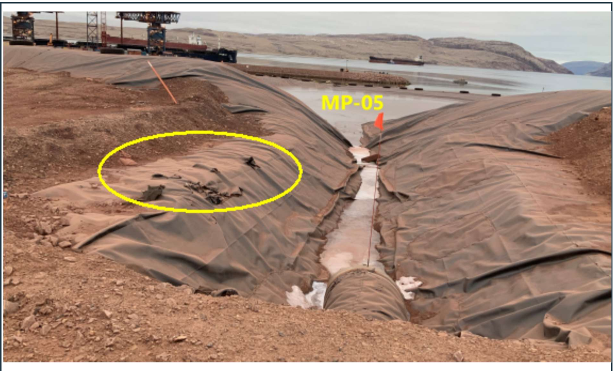
Figure 52: Damages to the liner still visible on the west slope of the southern inlet channel to MP-05.
