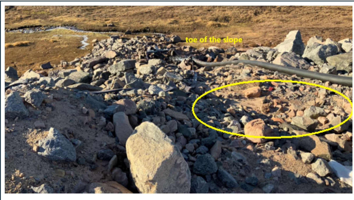
Figure 35: Rock fill riprap slope protection at the water discharge area. Note that some of the rock fill had “moved” to the toe of the slope. It is recommended to place new rock fill in the area marked with the yellow circle.
