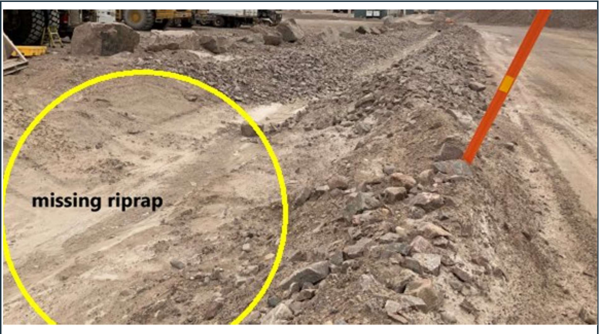
Figure 59: P-SWD-5 – “Q01-North” surface water collection ditch with missing riprap at a short section.
