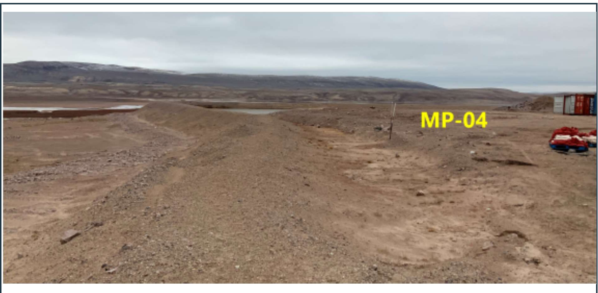
Figure 48: View of stable berm around the MP-04 landfarm, with soil covered waste and a few empty shipping containers within the cell.
