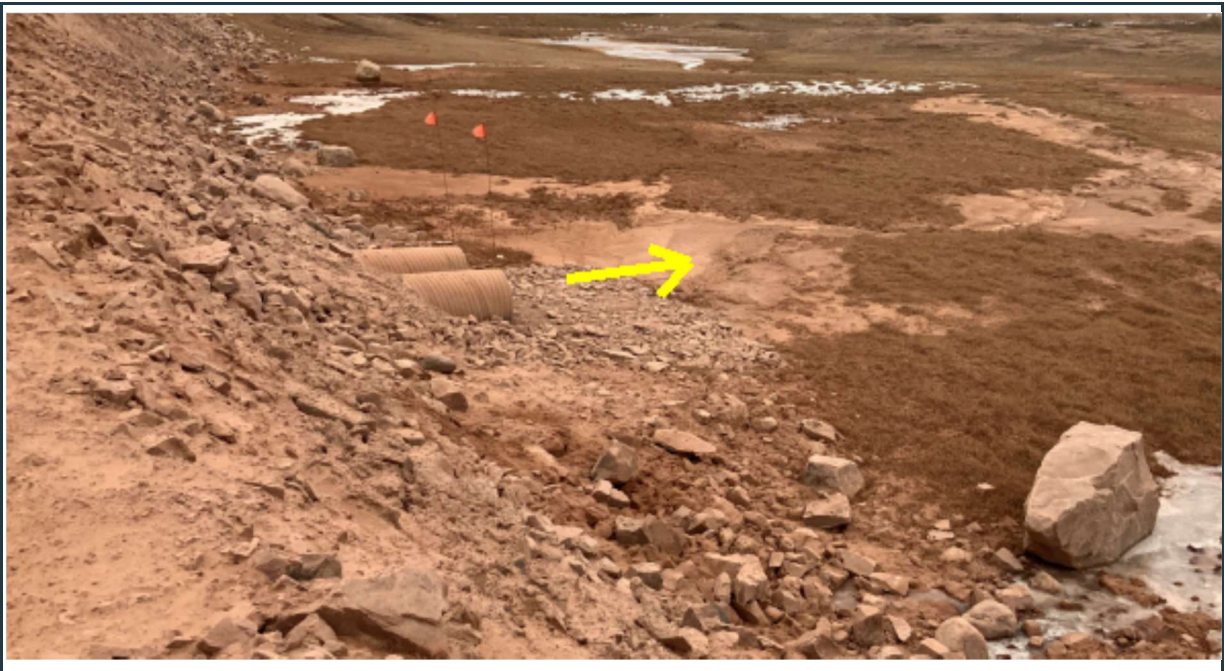
Figure 68: View of twin culverts, draining surface water from the quarry area (outlet).
