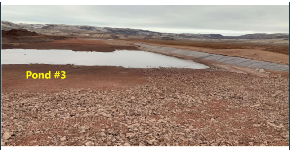
Figure 50: View of settling pond #3, with lined, stable berms along three sides of the pond.
