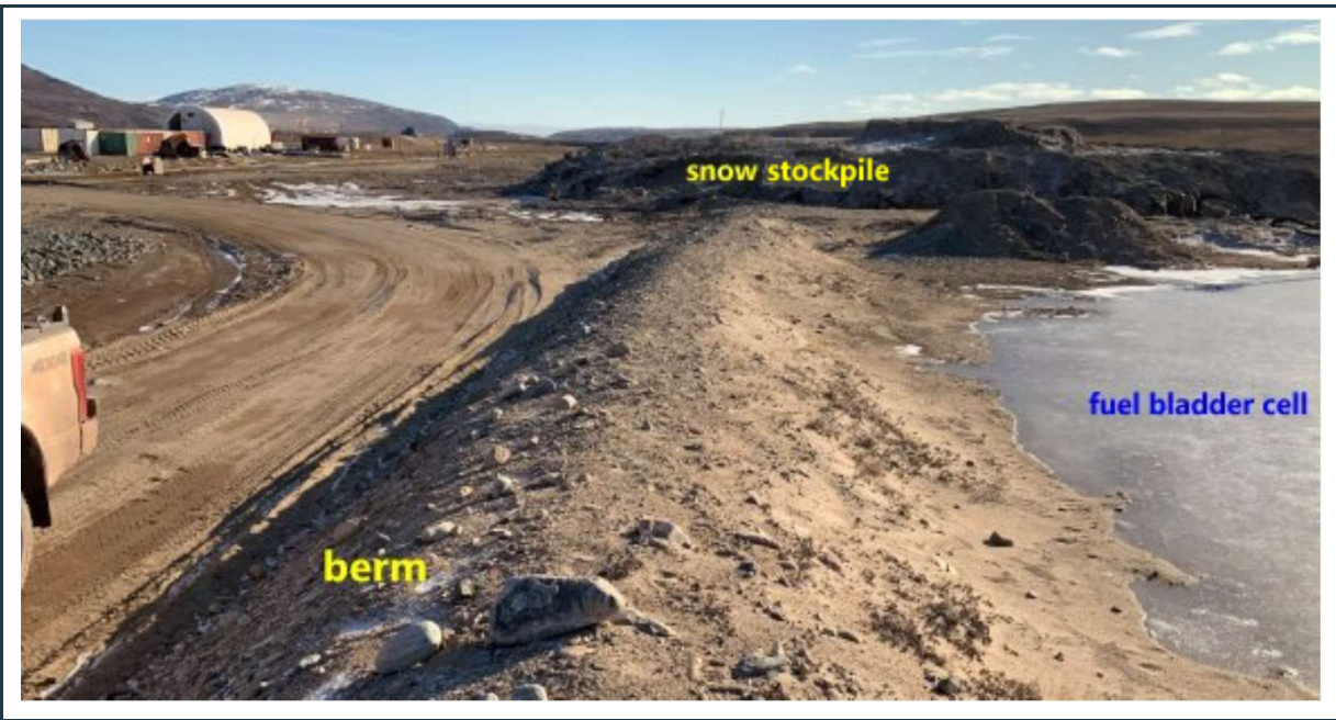
Figure 29: View of the snow stockpile adjacent to the “fuel bladder” cell. The melting snow has flooded the adjacent road next to the berm during the summer. It is recommended to excavate perimeter drainage ditches around the stockpile and prevent flooding of the road and berm.
