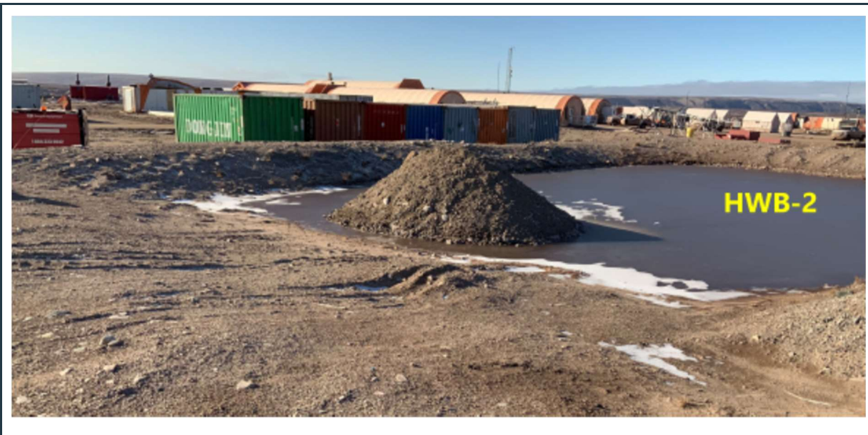
Figure 14: View of stable berms around HWB-2, and a pile of disposed soil that was dumped into the cell recently. The presence of water in the cell indicates good liner performance.
