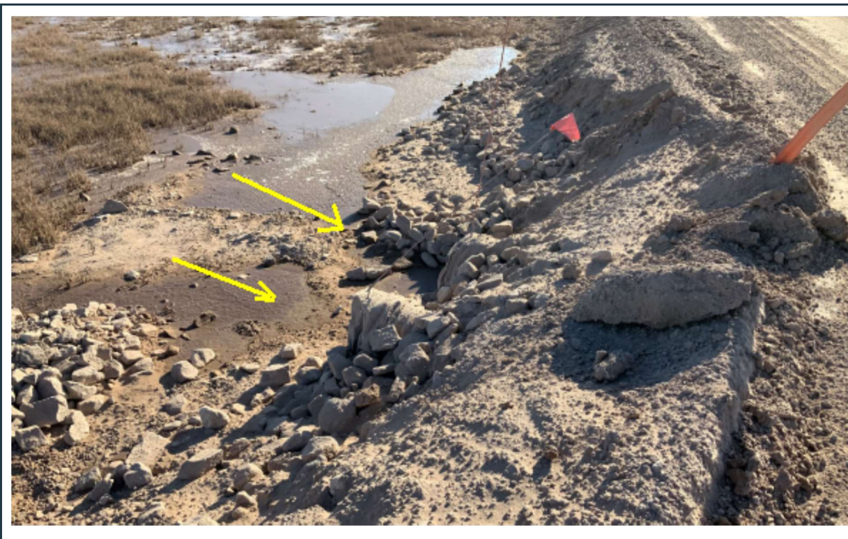
Figure 80: View of the inlet of the two culverts.
