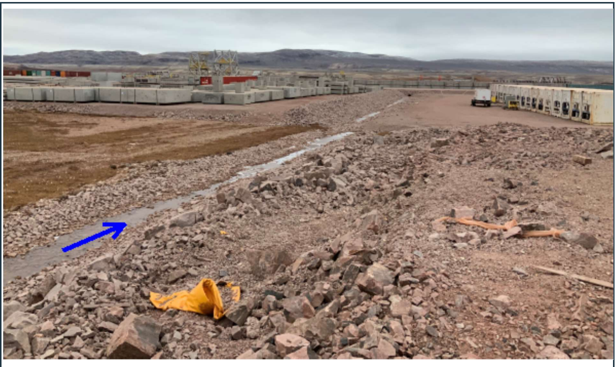
Figure 64: View of the south section of the 380 M surface water collection ditch.
