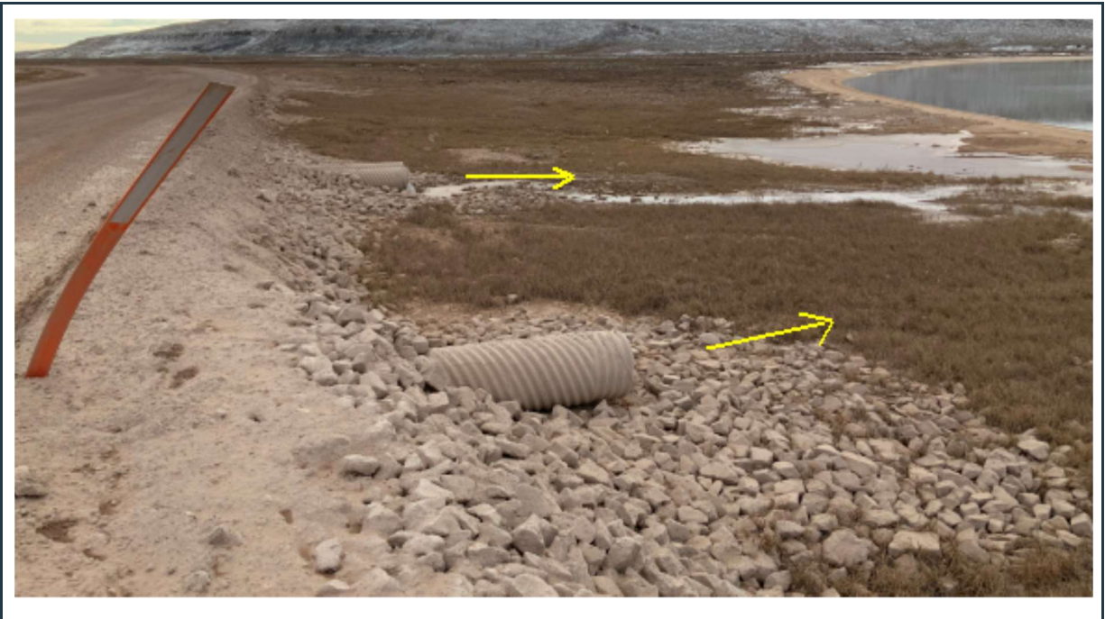
Figure 85: View of the outlet of the three culverts.
