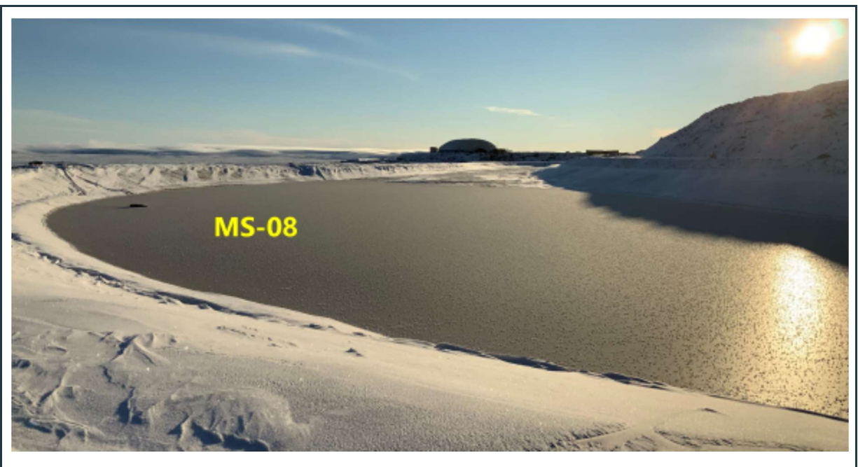
Figure 24: View of stable berm and intact liner at the MS-08 pond. Ice and snow were already present in the area in September.
