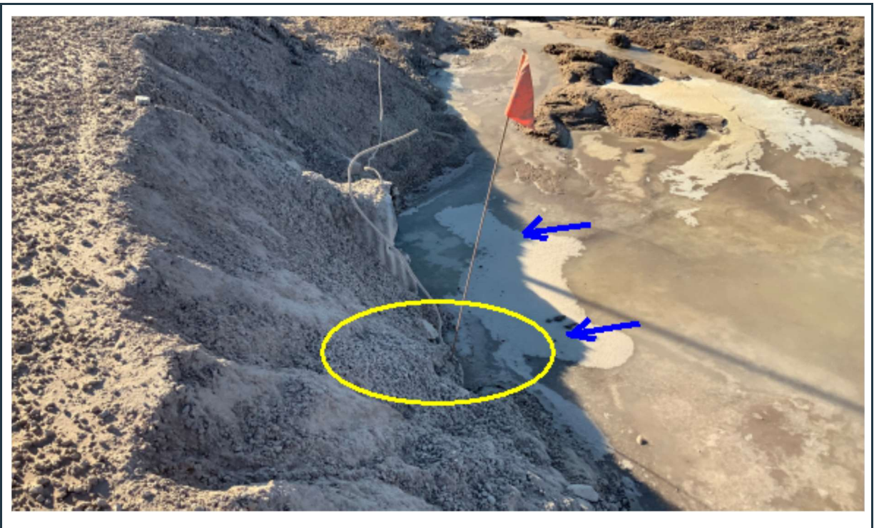
Figure 86: View of the inlet to culverts 030A and B. Note that one of the pipes is clogged (yellow circle).
