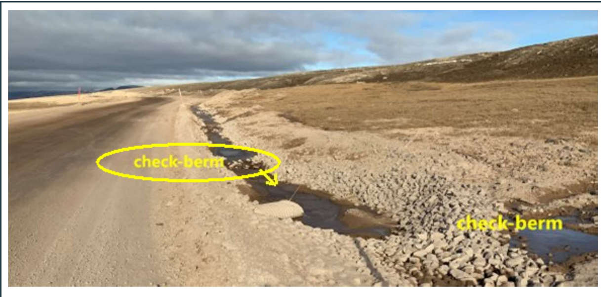
Figure 79: View of check-berms upstream of the culvert's inlet.
