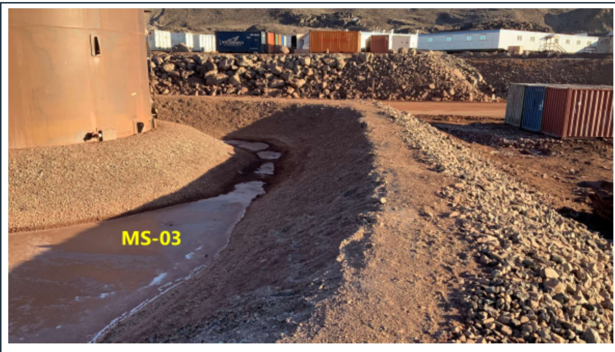
Figure 31: Well-maintained, stable berm around the MS-03 diesel fuel farm, with some ponding water.
