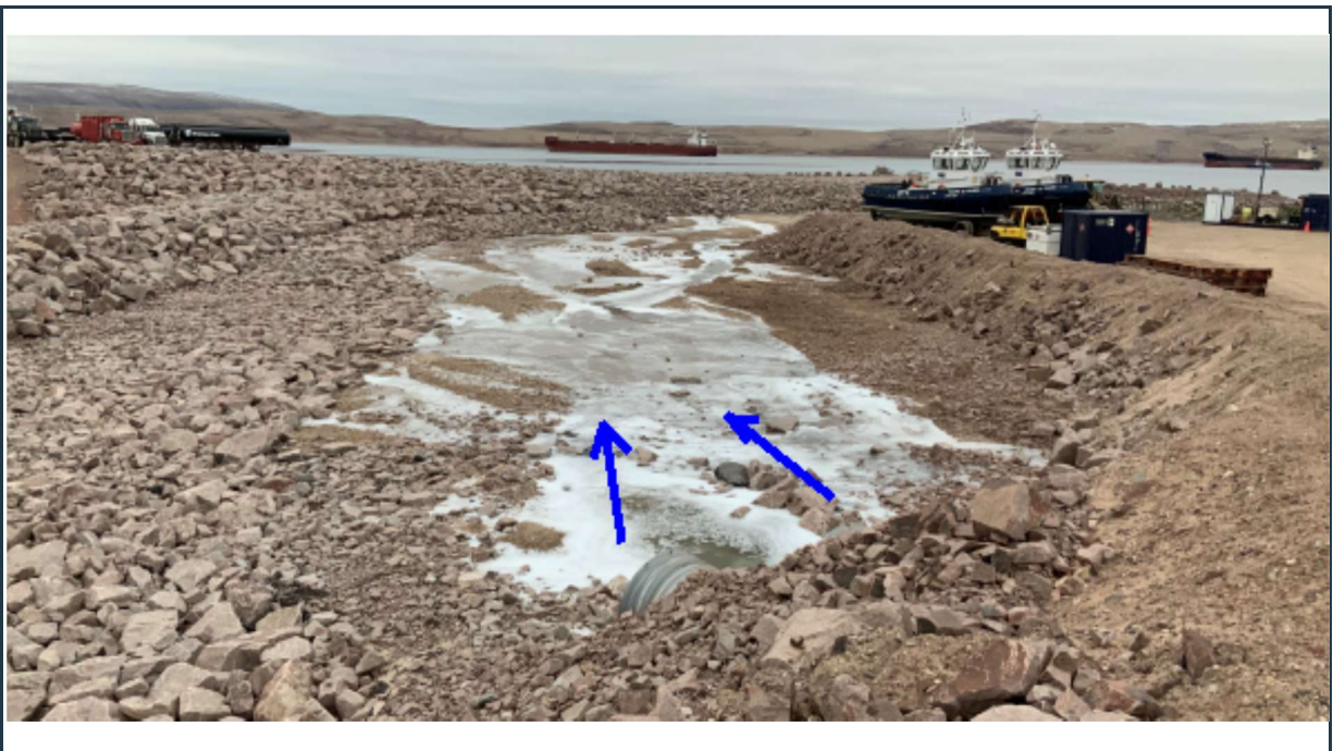
Figure 62: View of the well-maintained P-SWD-7 surface water collection ditch and culverts (outlet).
