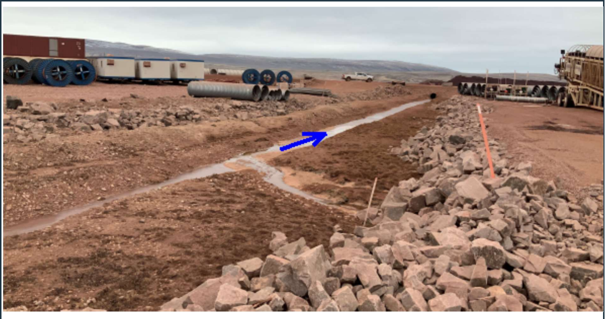
Figure 63: View of the W3/W14 uncompleted surface water collection ditch with some erosion.
