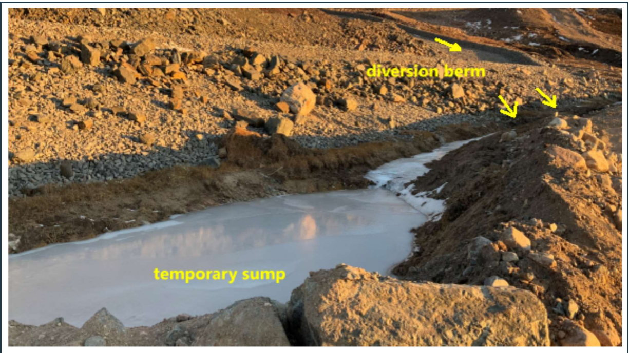
Figure 40: View of the surface water diversion berm at the new KM-106 ore stockpile area. Note the water seepage through the berm into a temporary sump, downstream from the diversion berm. The water from the sump is periodically pumped into the new nearby MS-07 pond.
