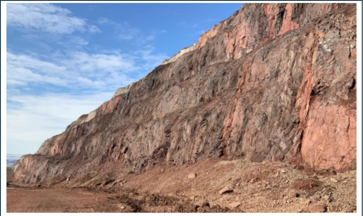
Figure 38: Stable pit-walls with minor rock weathering and pit-wall erosion.
