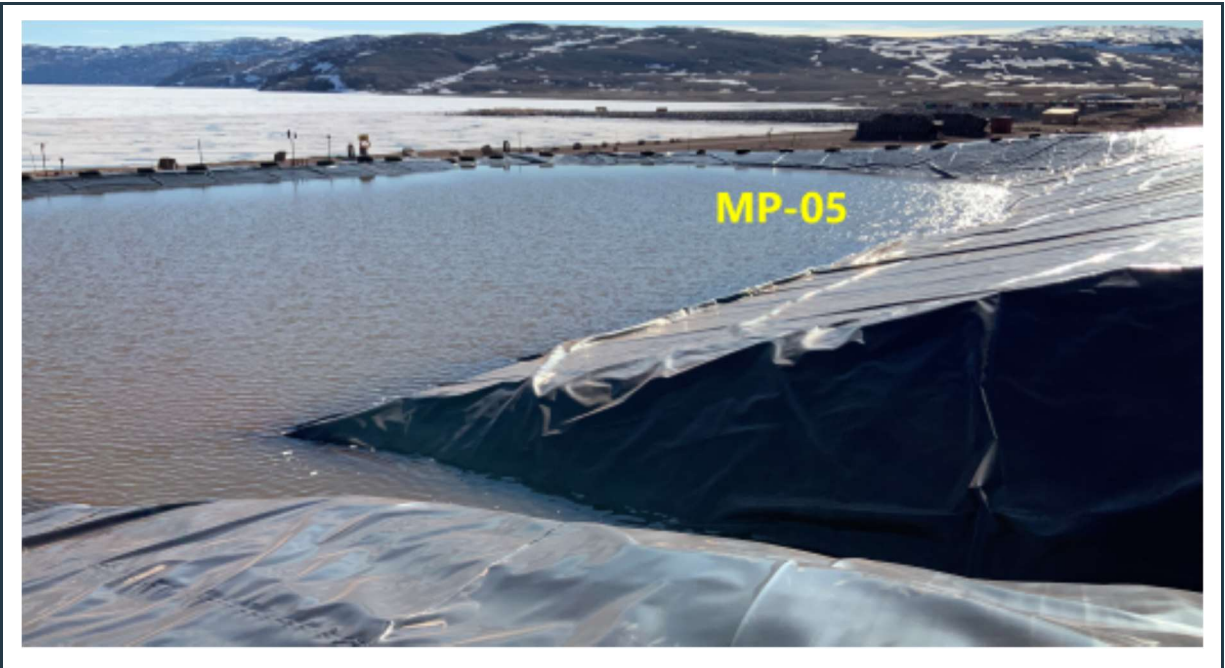
Figure 52: View of the stable berms and intact liner at the MP-05 settling pond (east of shiploader).
