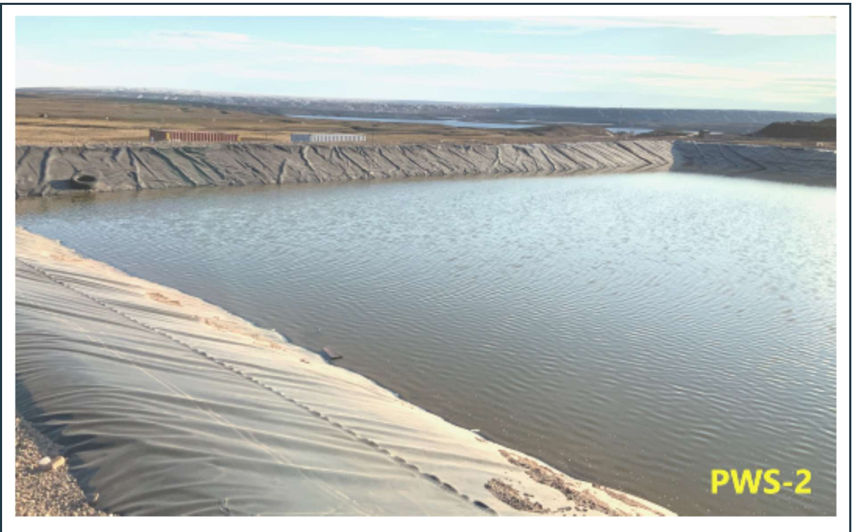
Figure 10: PWS pond #2 – Robust, stable, well-maintained berm and liner in and around the pond.
