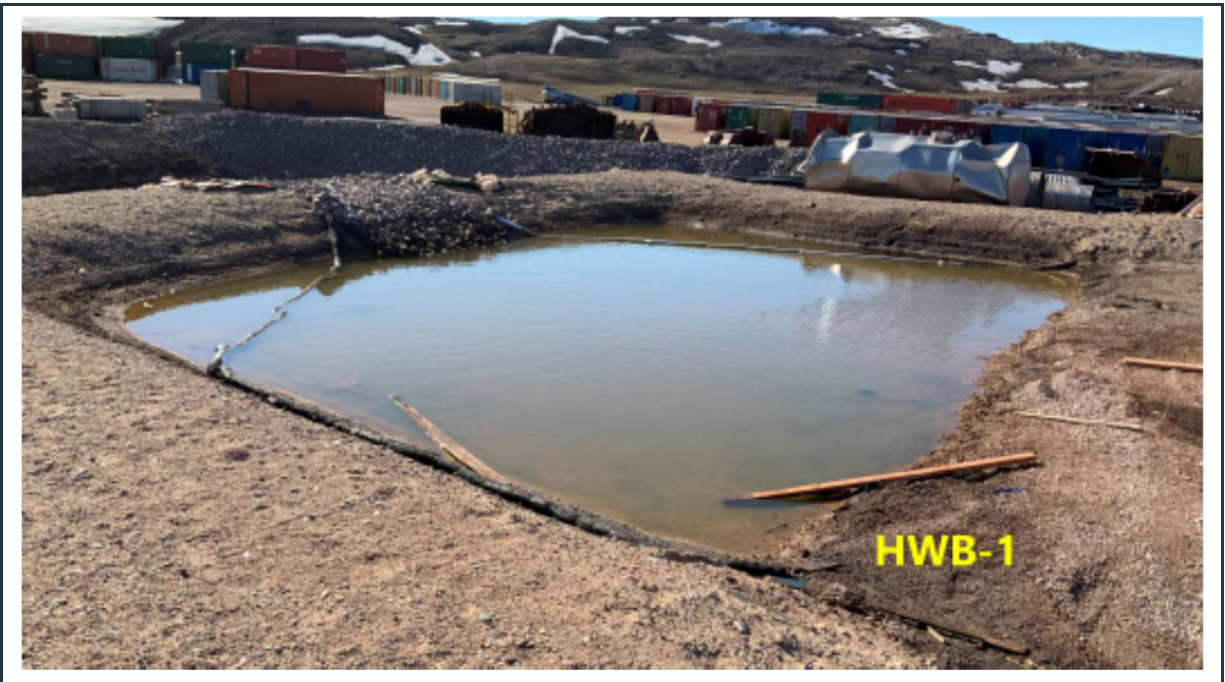
Figure 43: View of the back of the HWB-1 cell, with ponding water and stable spillway.
