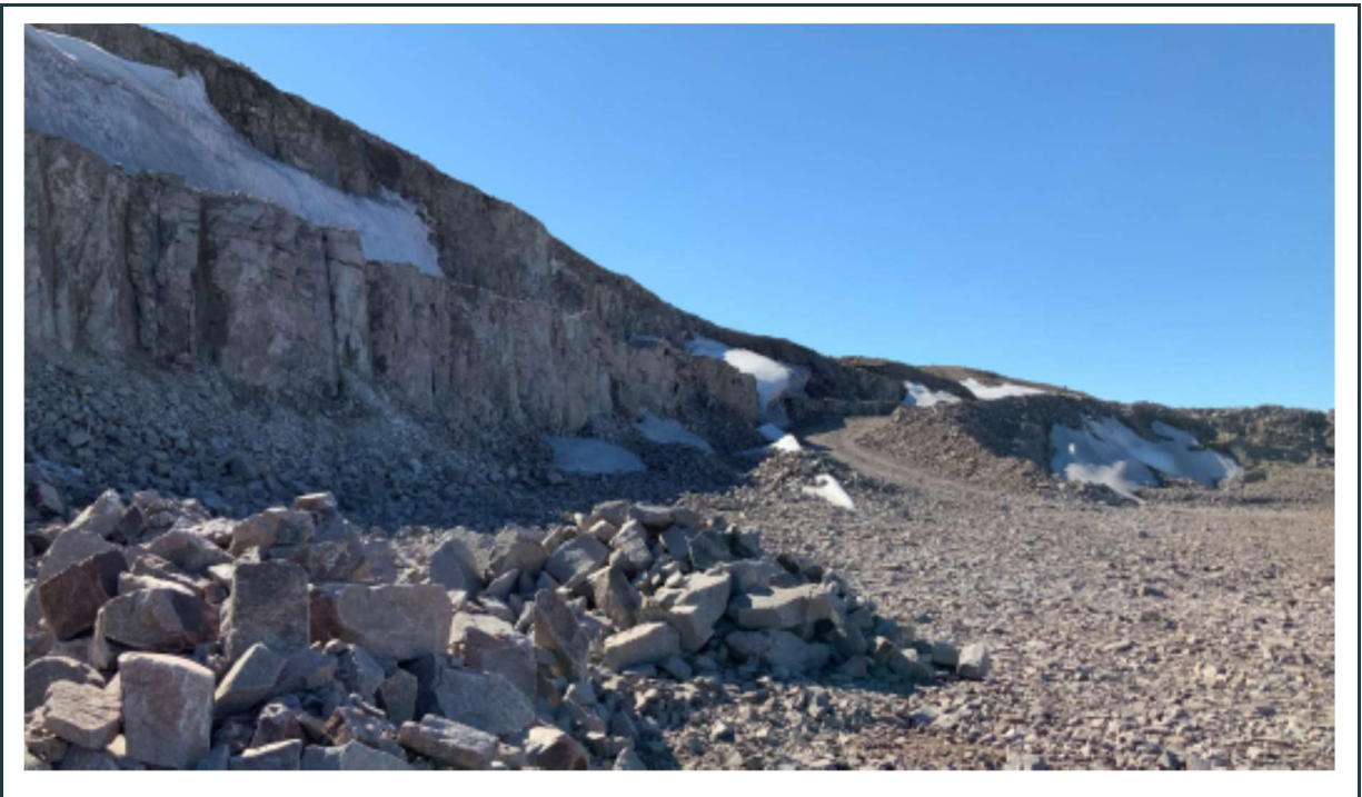
Figure 57: View of stable rock face with minor weathering and erosion in the Q01 rock quarry. The quarry is currently not in operation.
