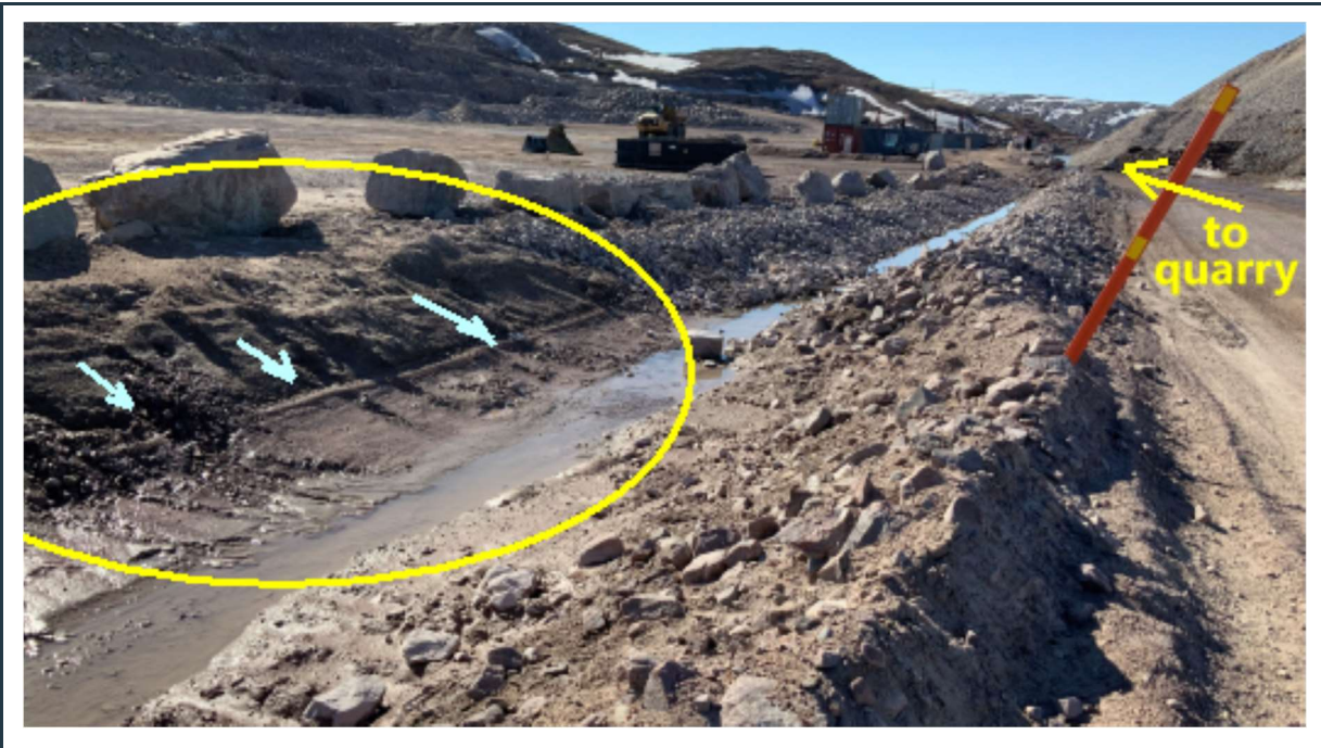
Figure 60: P-SWD-5 – “Q01-North” surface water collection ditch with missing riprap at a short section.
