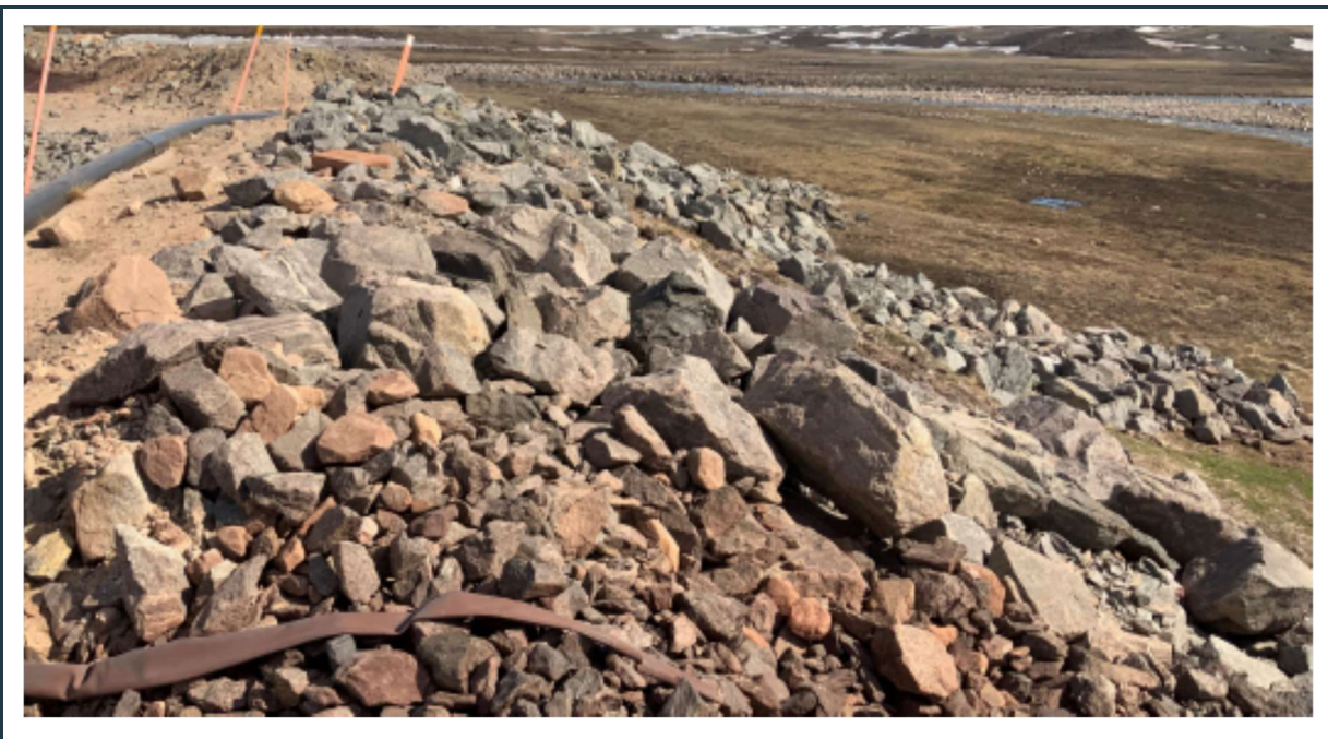
Figure 37: Stable rock fill riprap slope protection at the water discharge area.
