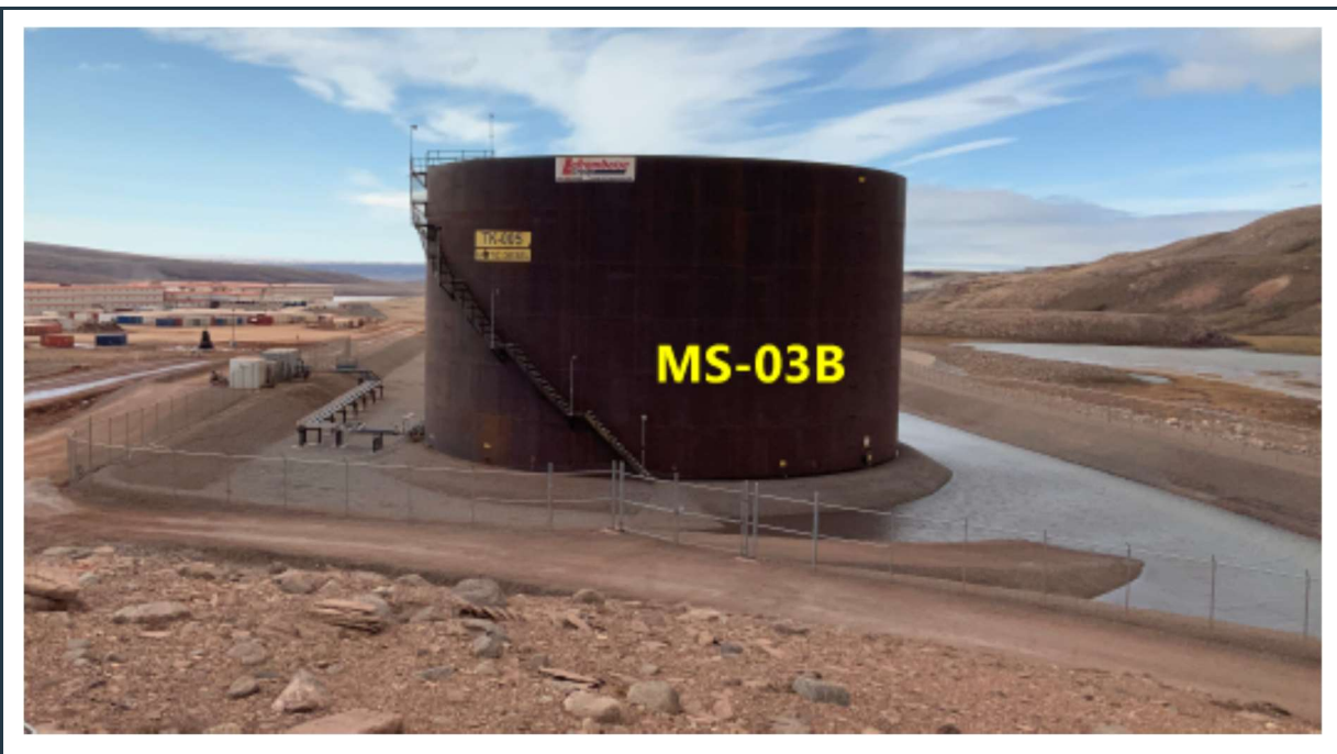
Figure 33: View of the well-maintained stable berms around the new lined fuel tank farm.
