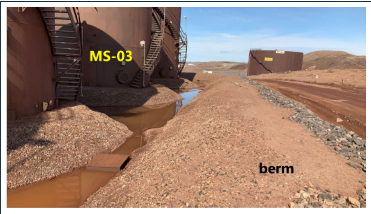
Figure 32: Well-maintained, stable berm around the MS-03 diesel fuel farm, with some ponding water.
