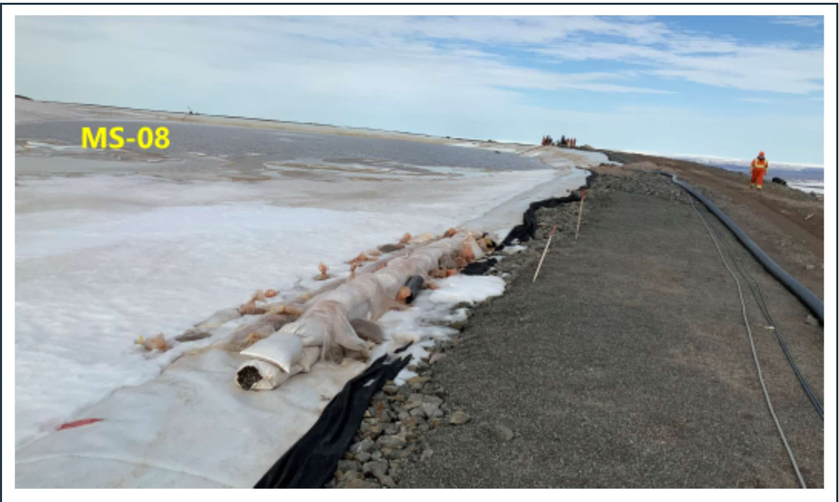
Figure 23: View of stable berm and intact liner at the MS-08 pond. Ice is still present at the end of June.
