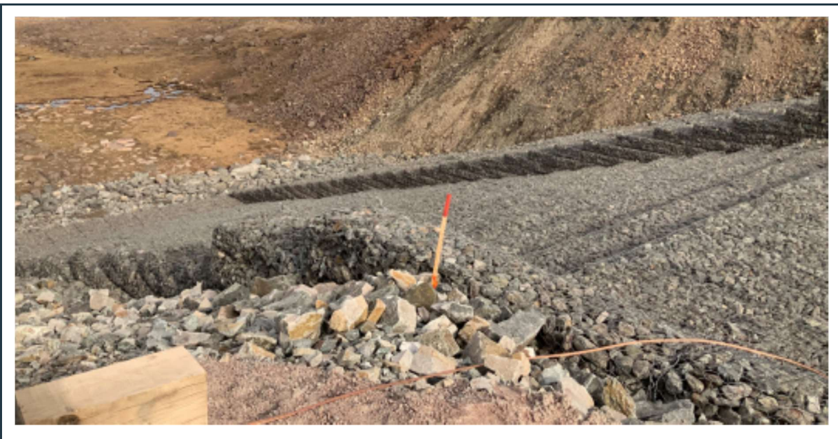
Figure 27: View of the recently completed stable emergency spillway (crushed rock filled gabion baskets and blankets) at KM105.
