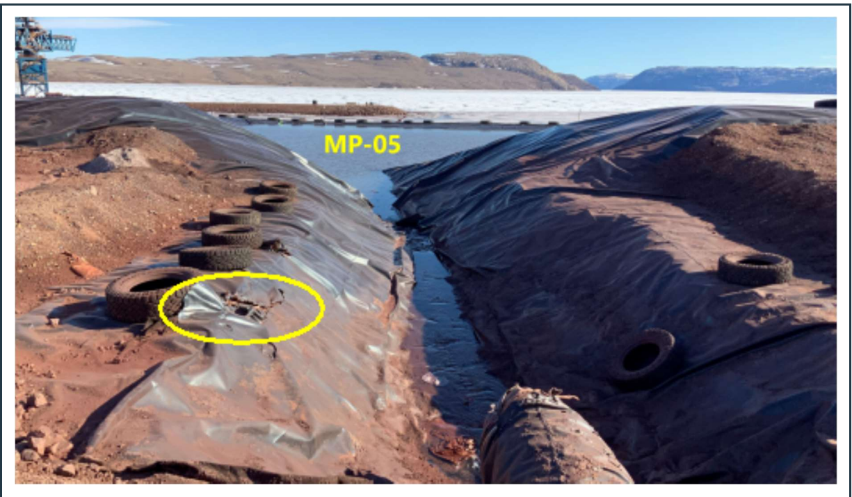
Figure 53: Minor liner damage on the west slope of the southern intake channel that should be repaired. Note the still frozen bay in the background.
