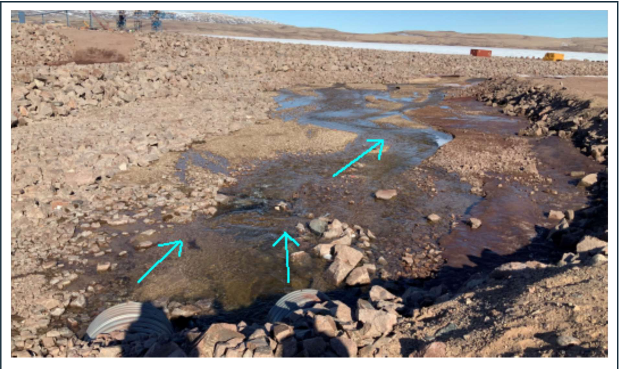
Figure 64: View of the P-SWD-7 surface water collection ditch and culverts (outlet).
