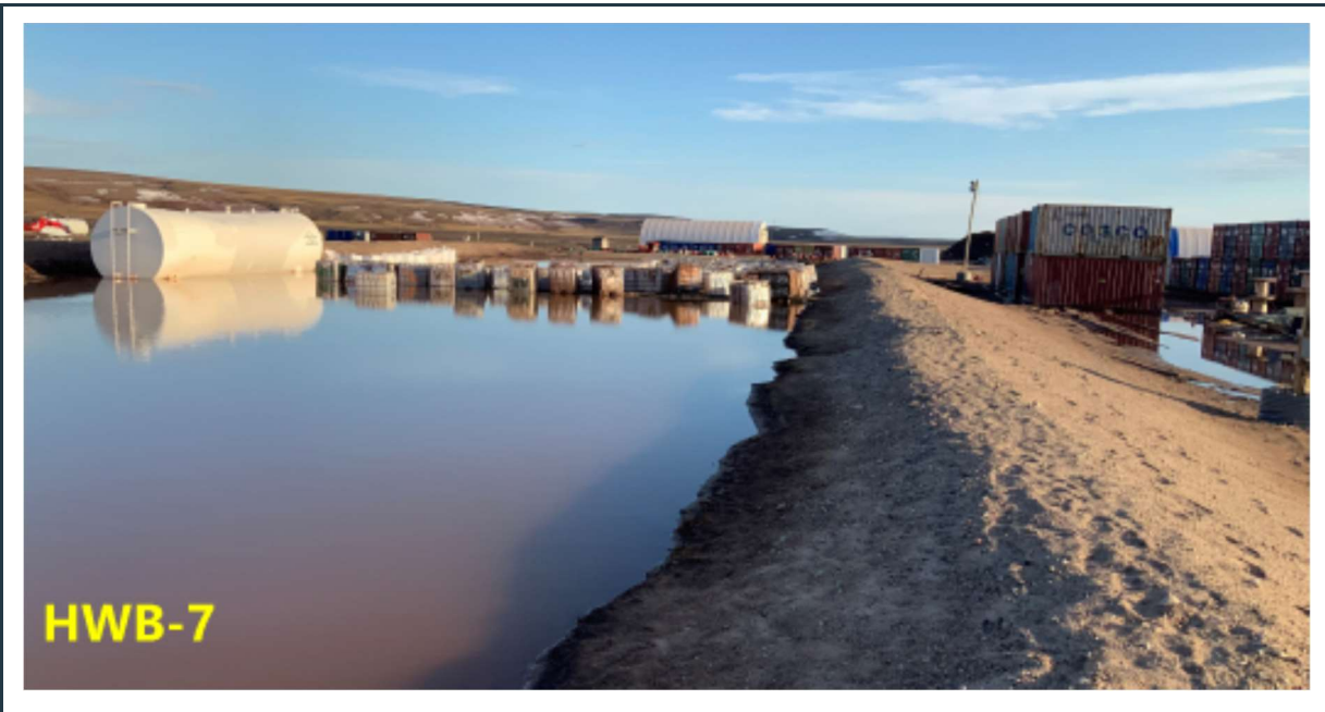
Figure 18: View of the large, flooded HWB-7 cell, with one large fuel tank and some containers stored.
