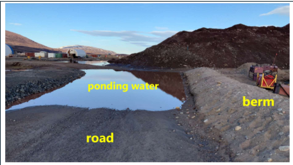
Figure 30: View of ponding water adjacent to the north-east berm of the “fuel bladder” cell. The low area of the road should be filled with sand and gravel, and the water diverted away from the cell.
