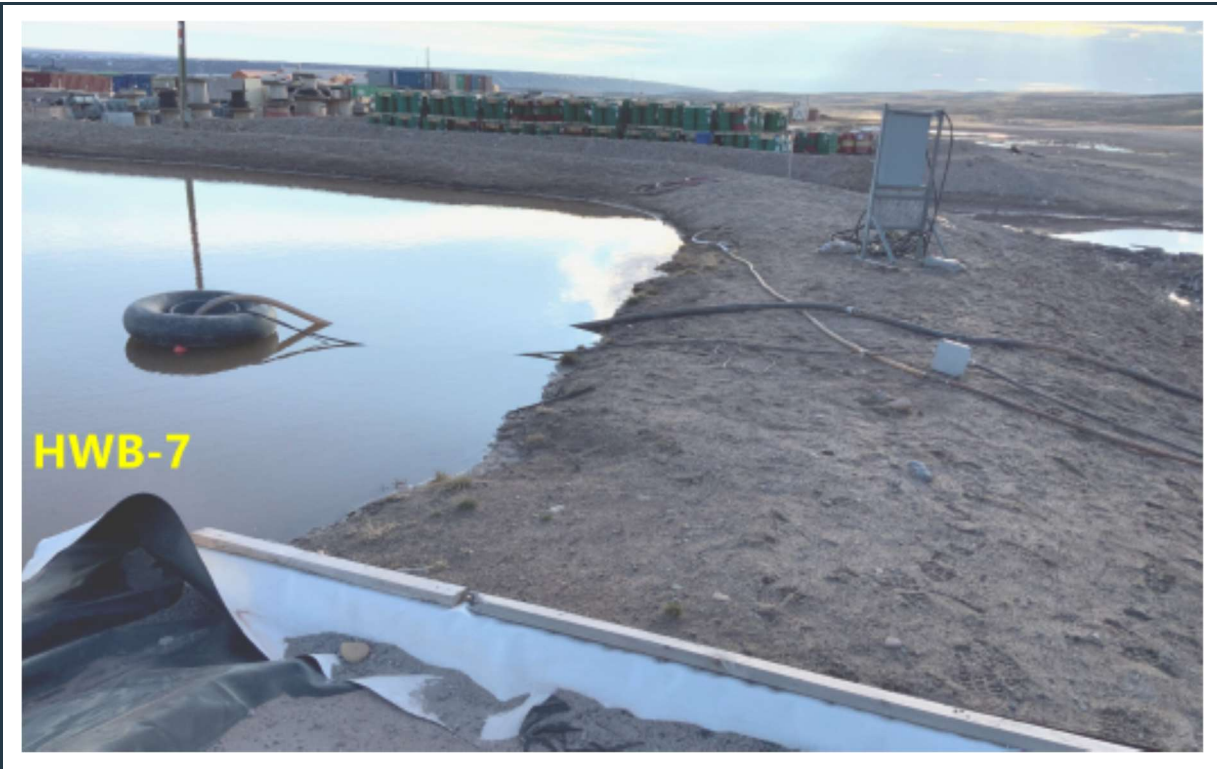
Figure 19: View of the somewhat lower crest of the east berm at the flooded HWB-7 cell.
