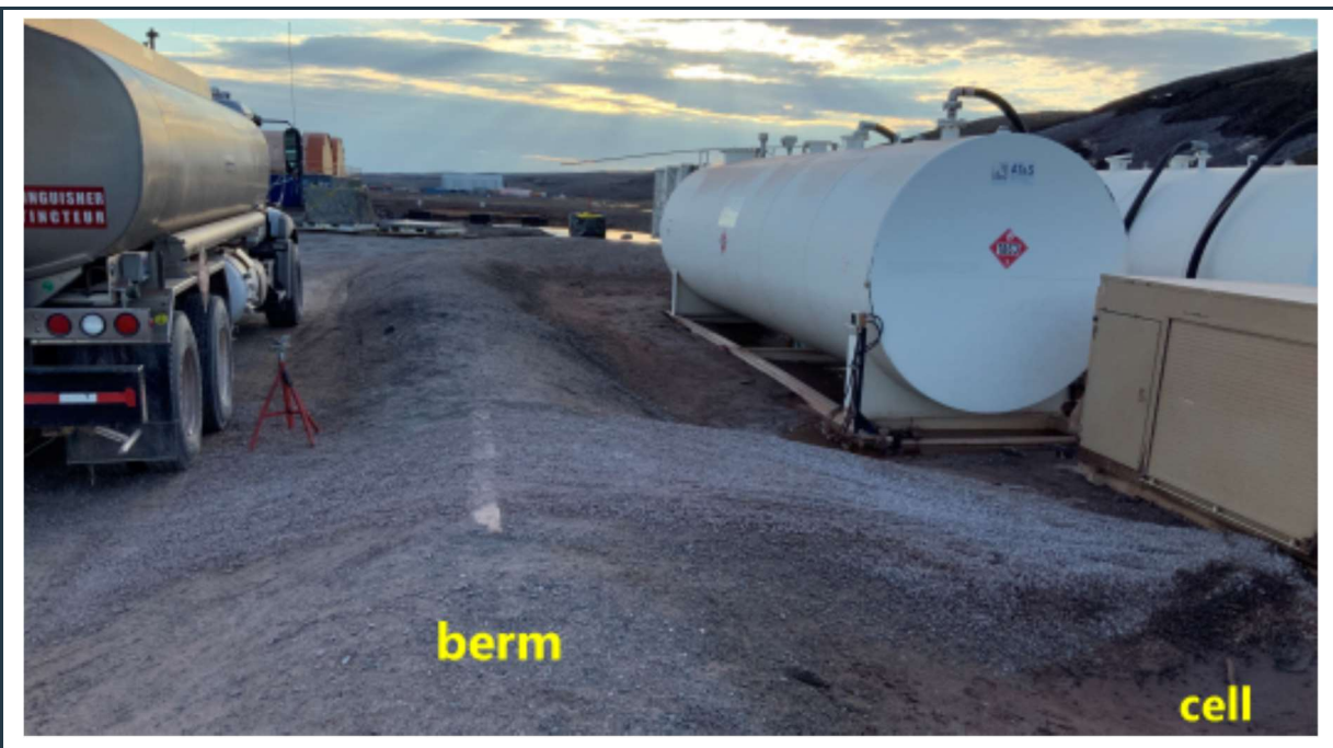
Figure 31: View of the well-maintained sand and gravel berm at the lined jet-fuel storage facility.
