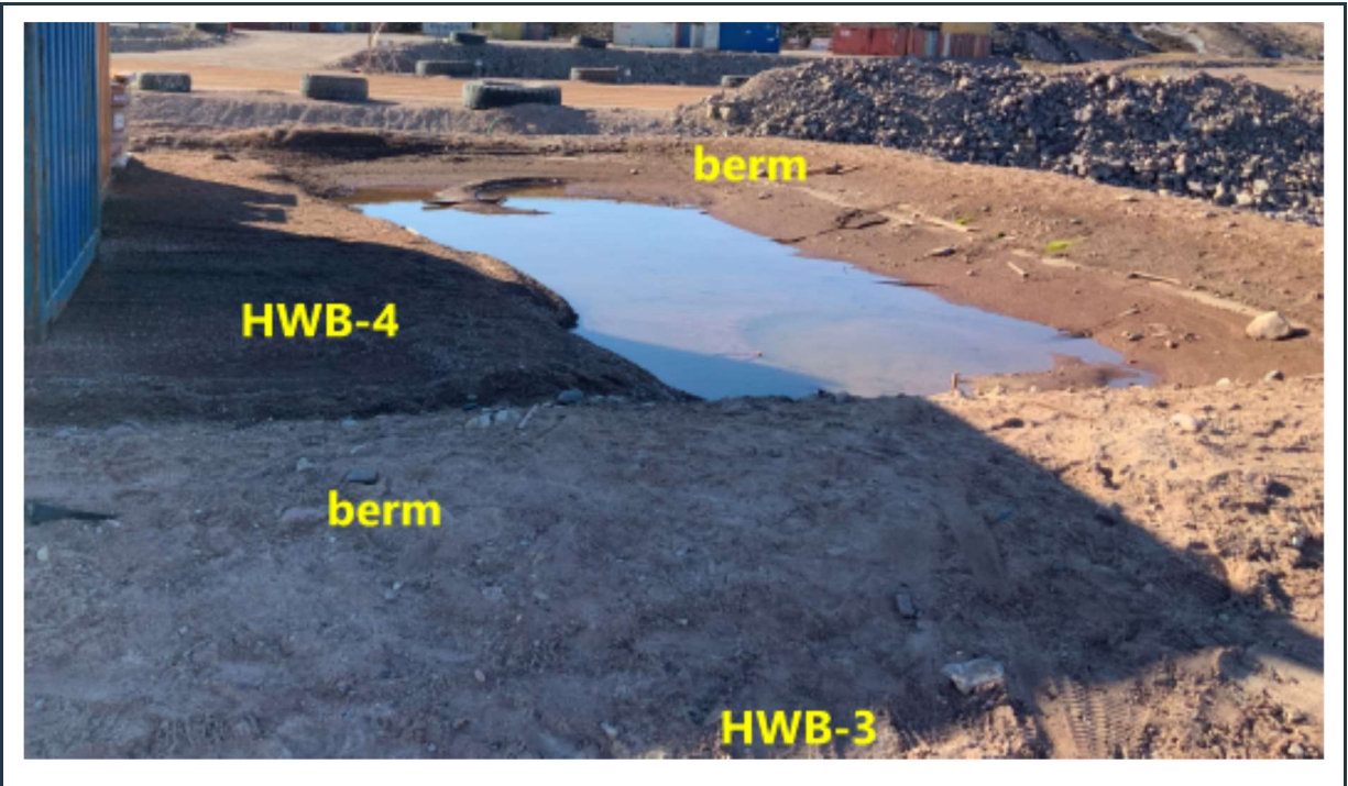
Figure 46: Stable berms around and ponding water within the HWB-3 and HWB-4 cells.
