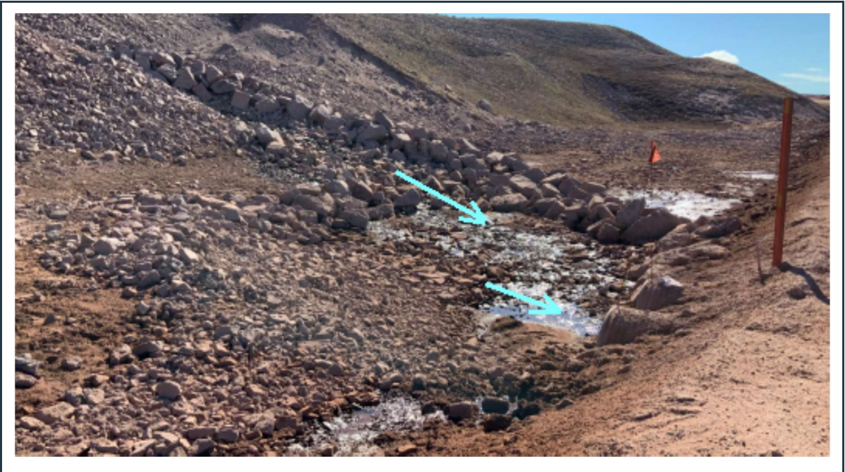
Figure 70: View of twin culverts' inlet, draining surface water from the P-SWD-6 - "Q01 South" surface water collection ditch.
