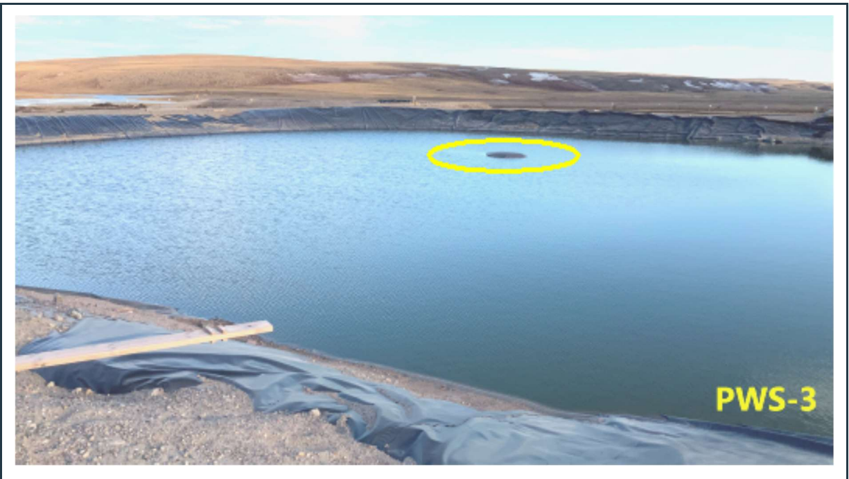
Figure 11: Stable perimeter berms and liner in PWS pond #3 – A small “floating” section of the liner is visible in the pond (yellow circle), which is quite common in shallow ponds.
