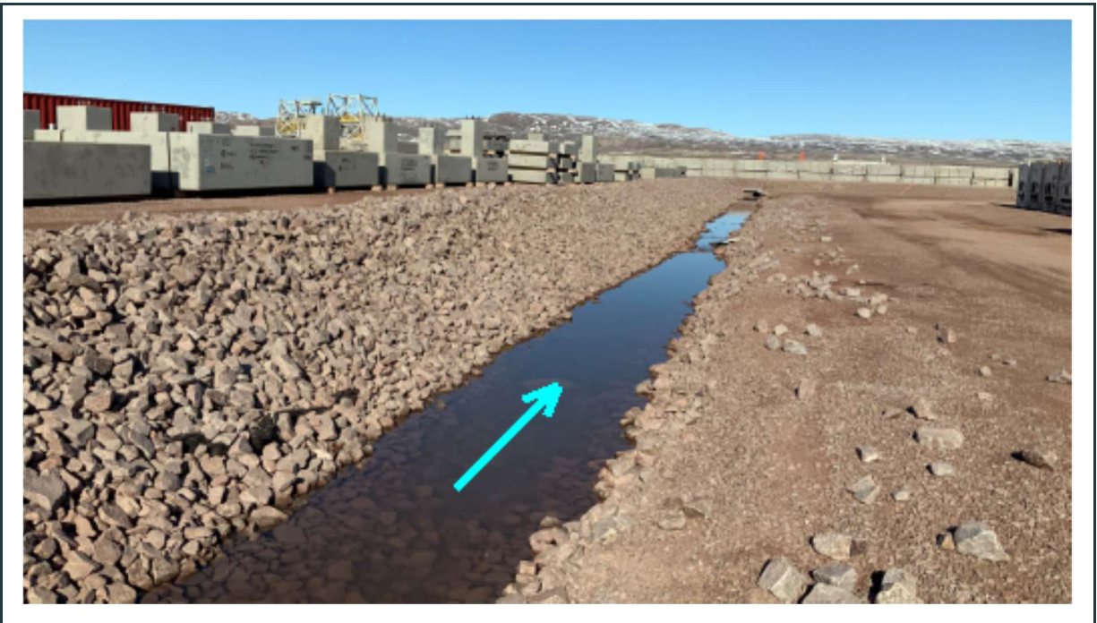
Figure 66: View of the south section of the 380 M surface water collection ditch in good condition.
