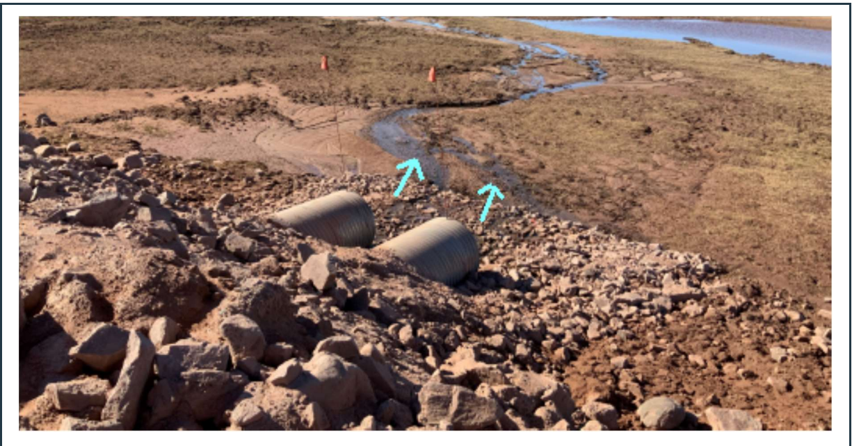
Figure 71: View of twin culverts installed under the tote road, draining surface water from the quarry area (outlet).
