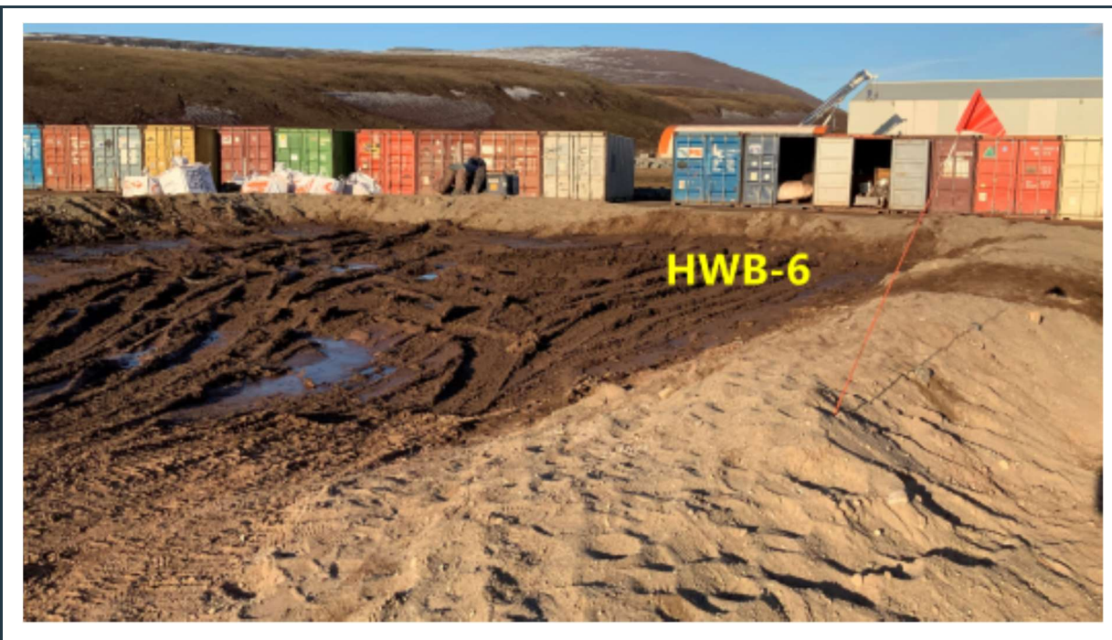
Figure 17: View of the somewhat disturbed but stable berm around the HWB-6 cell. The cell was recently emptied, and the internal subgrade disturbed, which needs to be leveled.
