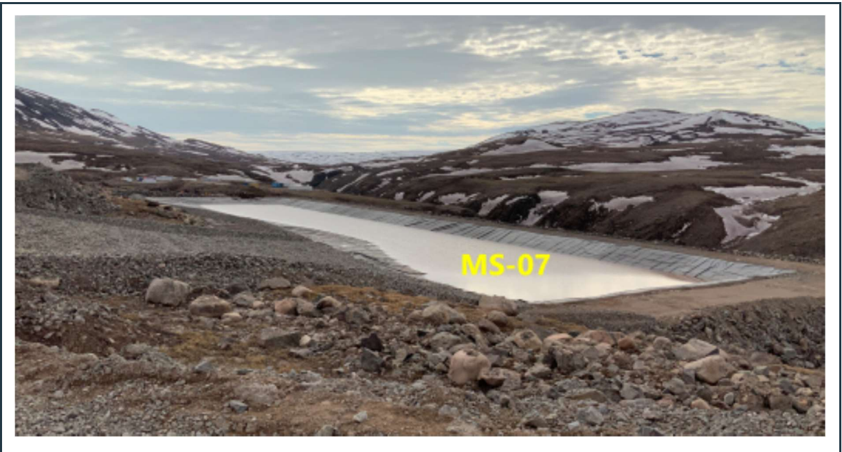
Figure 22: View of the MS-07 surface-water collection pond with robust, stable berms and intact liner.
