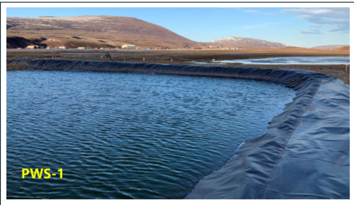
Figure 9: PWS pond #1. Well maintained stable perimeter berm and liner.
