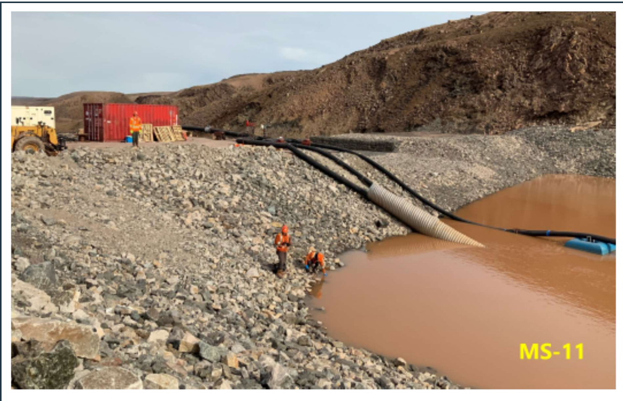
Figure 26: View of the recently completed robust, stable rock-fill dam at the MS-11 pond at KM105.
