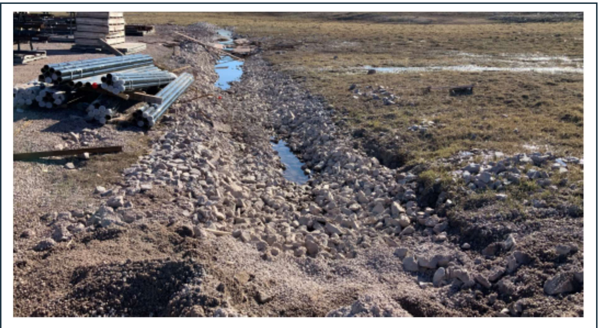
Figure 59: View of the northern part of the "P-SWD-3 surface water collection ditch with failed slopes and ponding water. The ditch should be redesigned and reconstructed.
