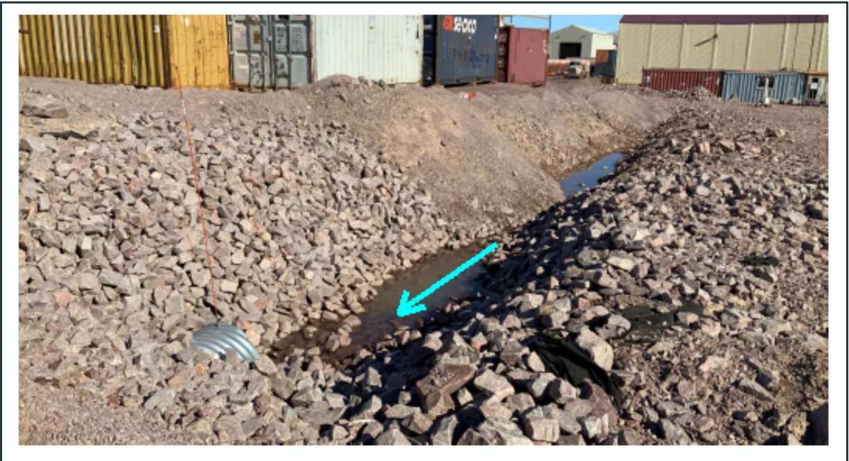
Figure 68: View of the west section of the PSC surface water collection ditch. Note the culvert with too high invert elevation, resulting in ponding water in this section of the ditch.
