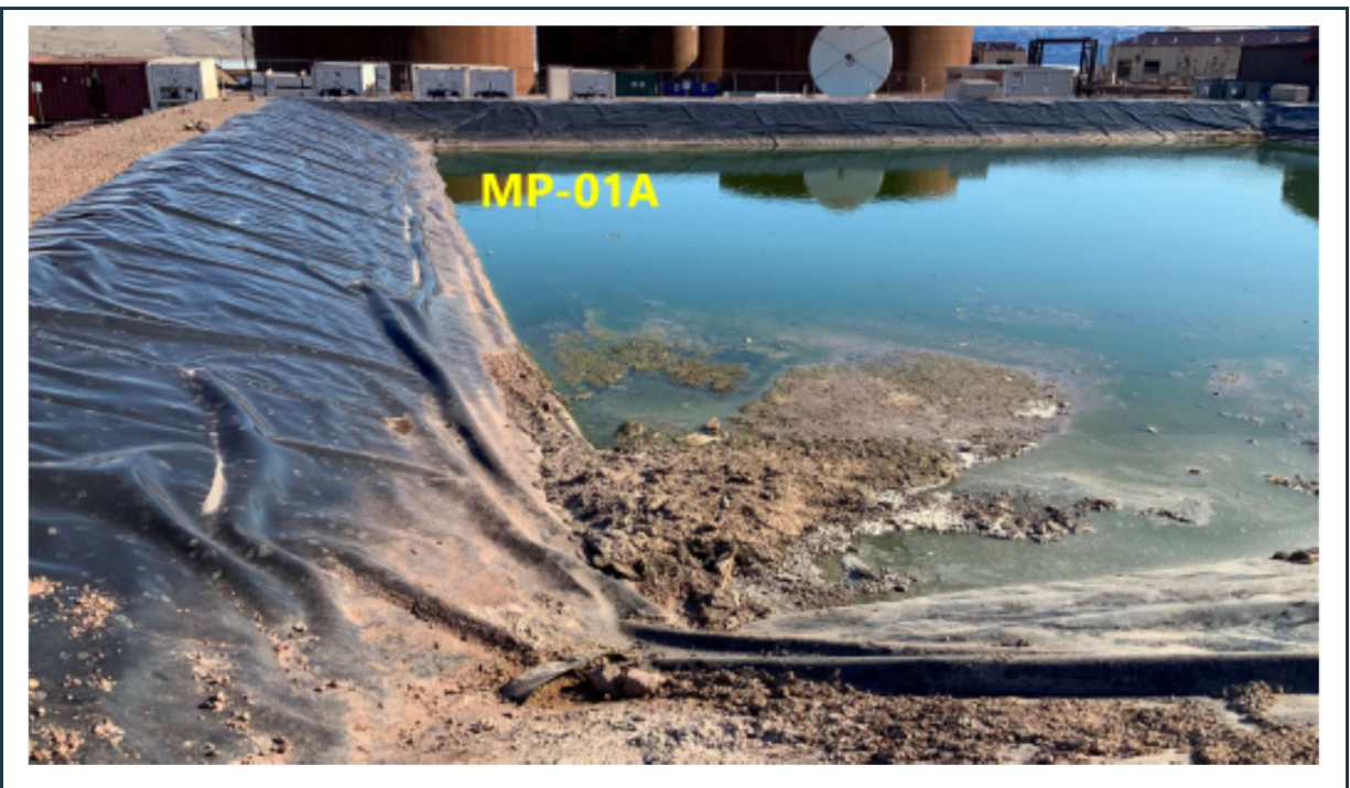
Figure 47: Berms and liner in good condition with stable slopes around the MP-01A pond.
