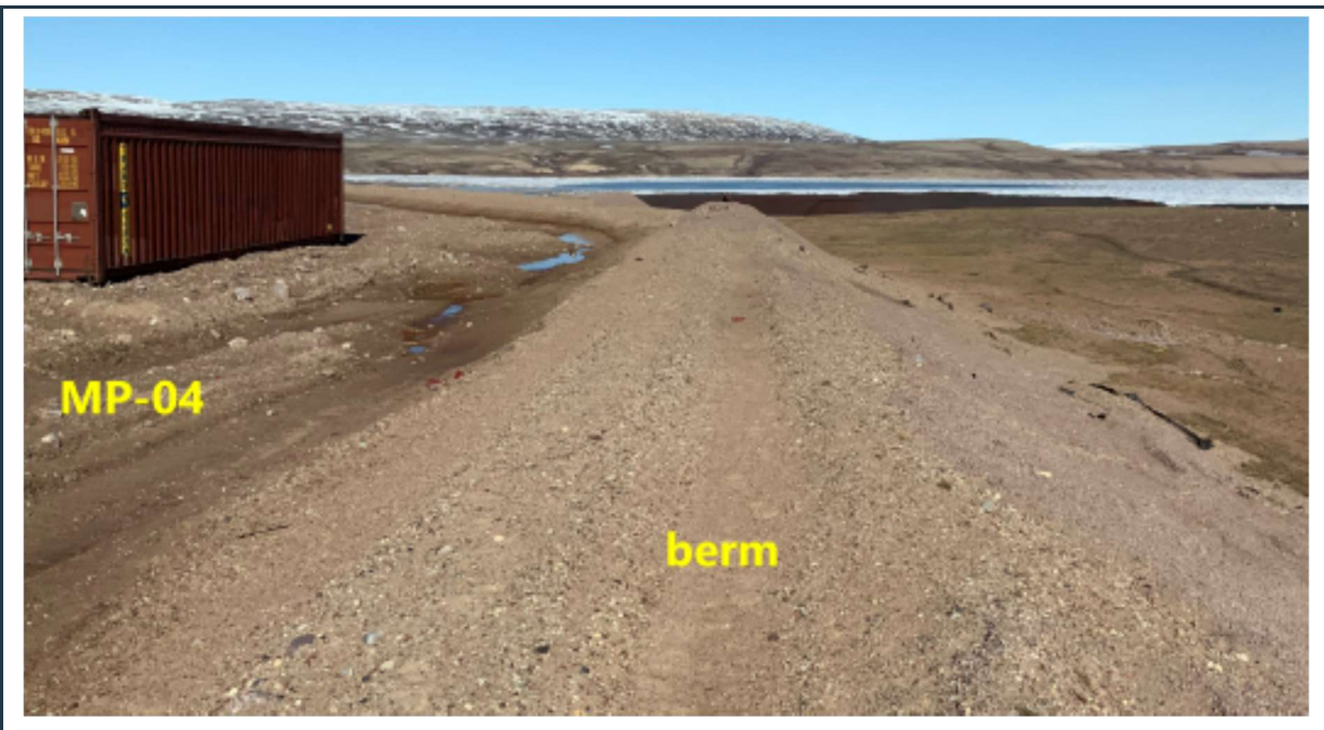
Figure 49: View of stable, robust berms around the MP-04 landfarm, with empty shipping containers stored within the cell.
