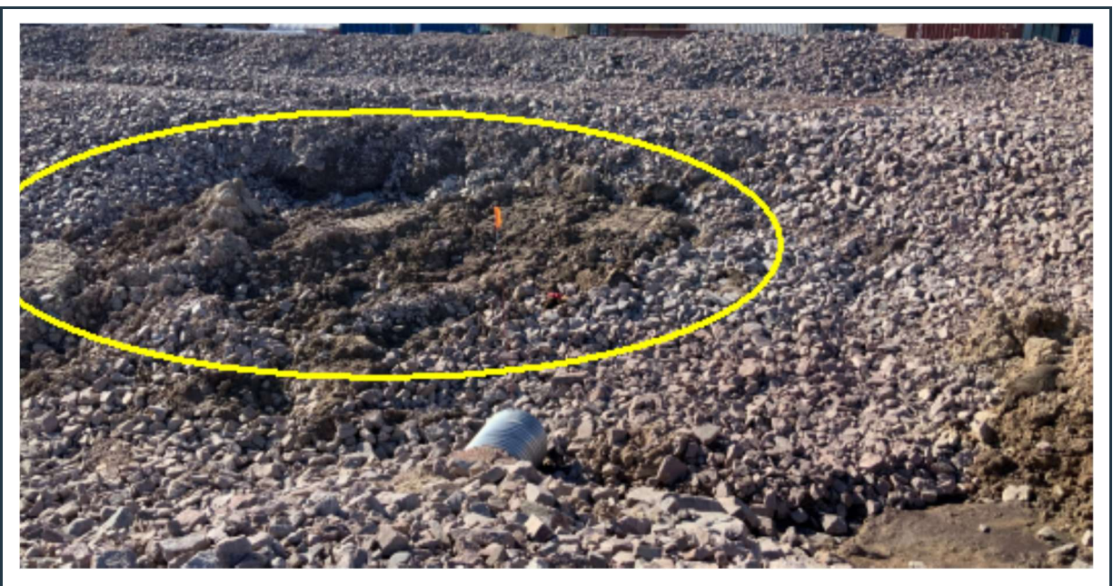
Figure 69: View of the south end of the same (Figure 67) culvert with too high invert elevation. Note the localized slope failure adjacent to the culvert, which should be repaired as soon as practically possible.
