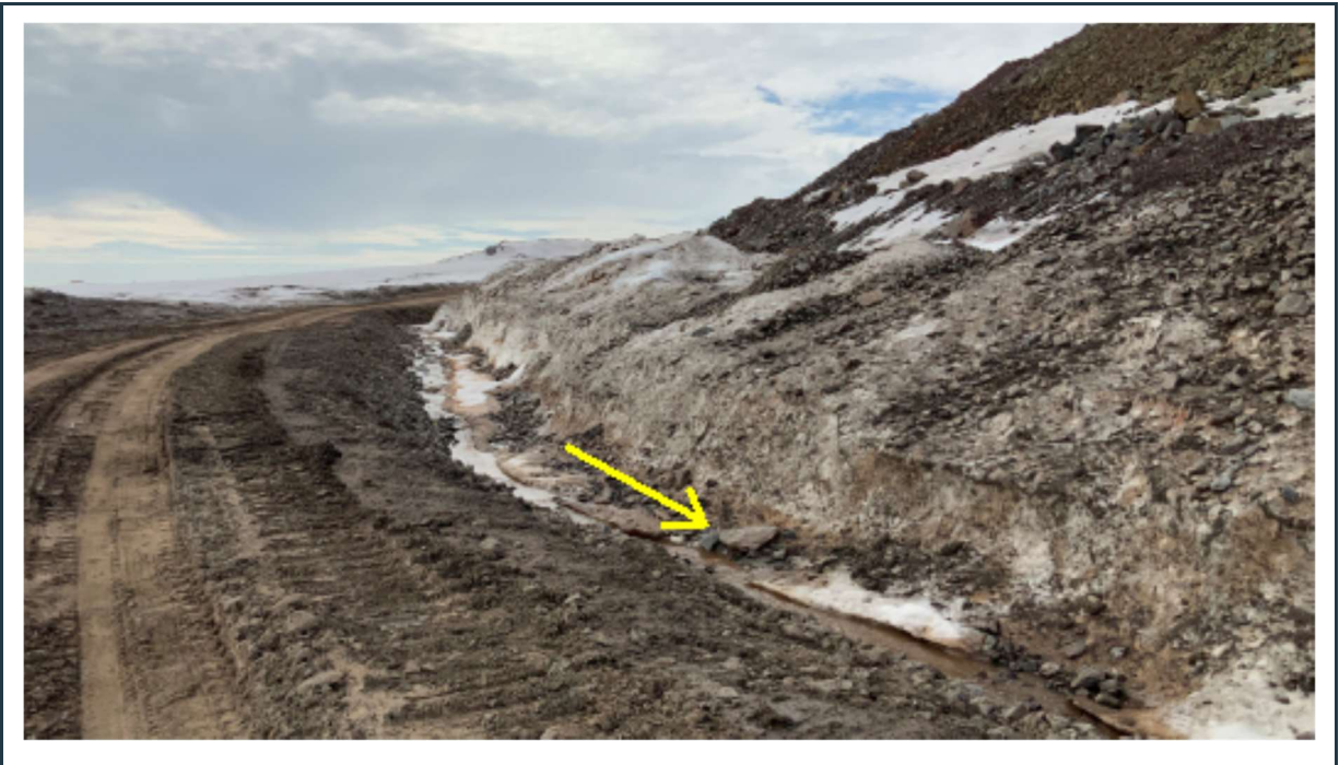
Figure 24: Snow-filled stable drainage ditch around the east side of the waste rock facility.
