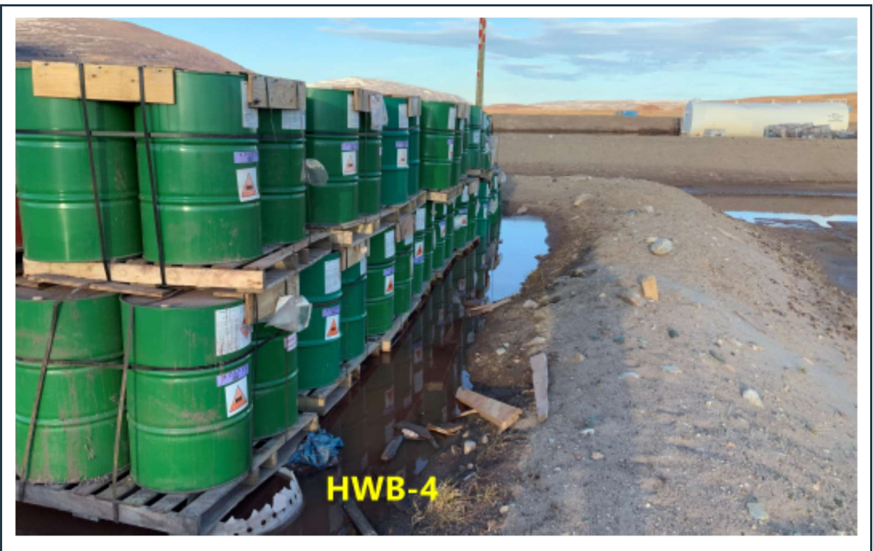
Figure 15: View of stable berms at HWB-4, with jet-fuel barrels stored on wooden pallets.
