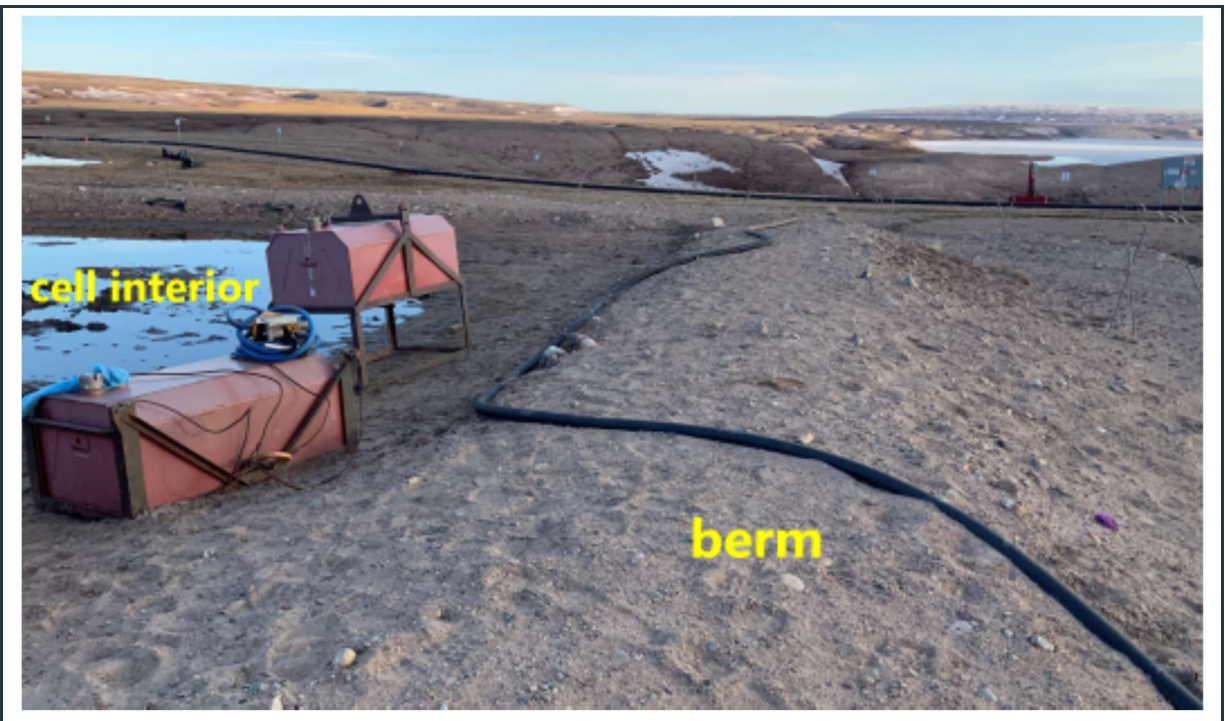
Figure 29: View of the stable berm around the "generator fuel bladder" cell.
