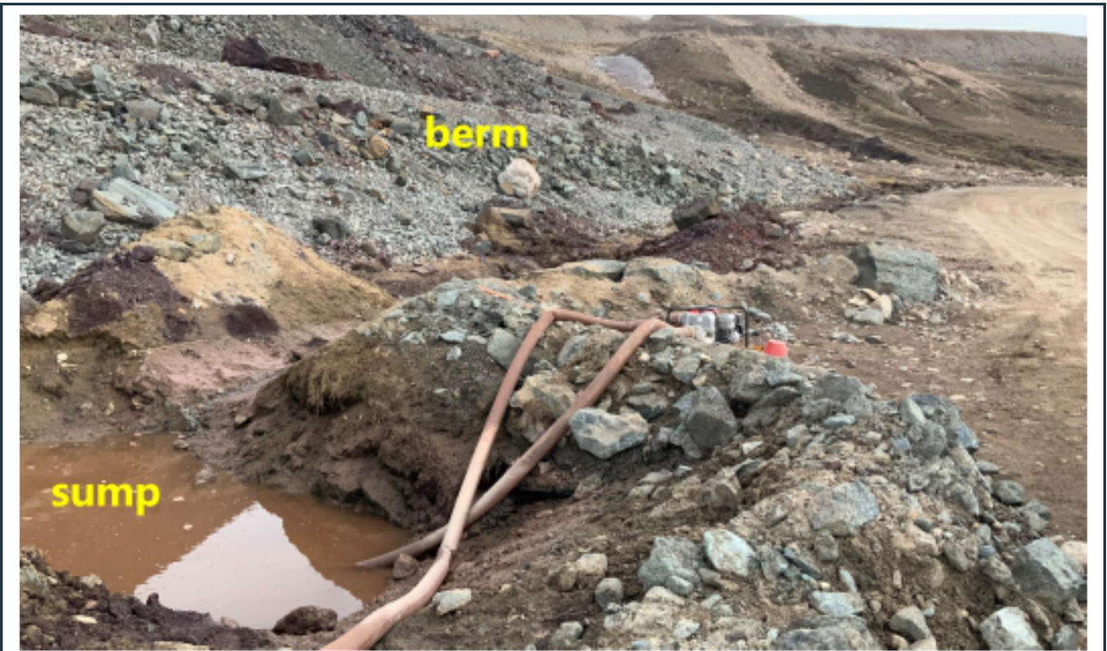
Figure 41: View of a temporary sump pit adjacent to the surface water diversion berm at the KM-106 ore stockpile area. The water from the sump is pumped to the nearby MS-07 pond.
