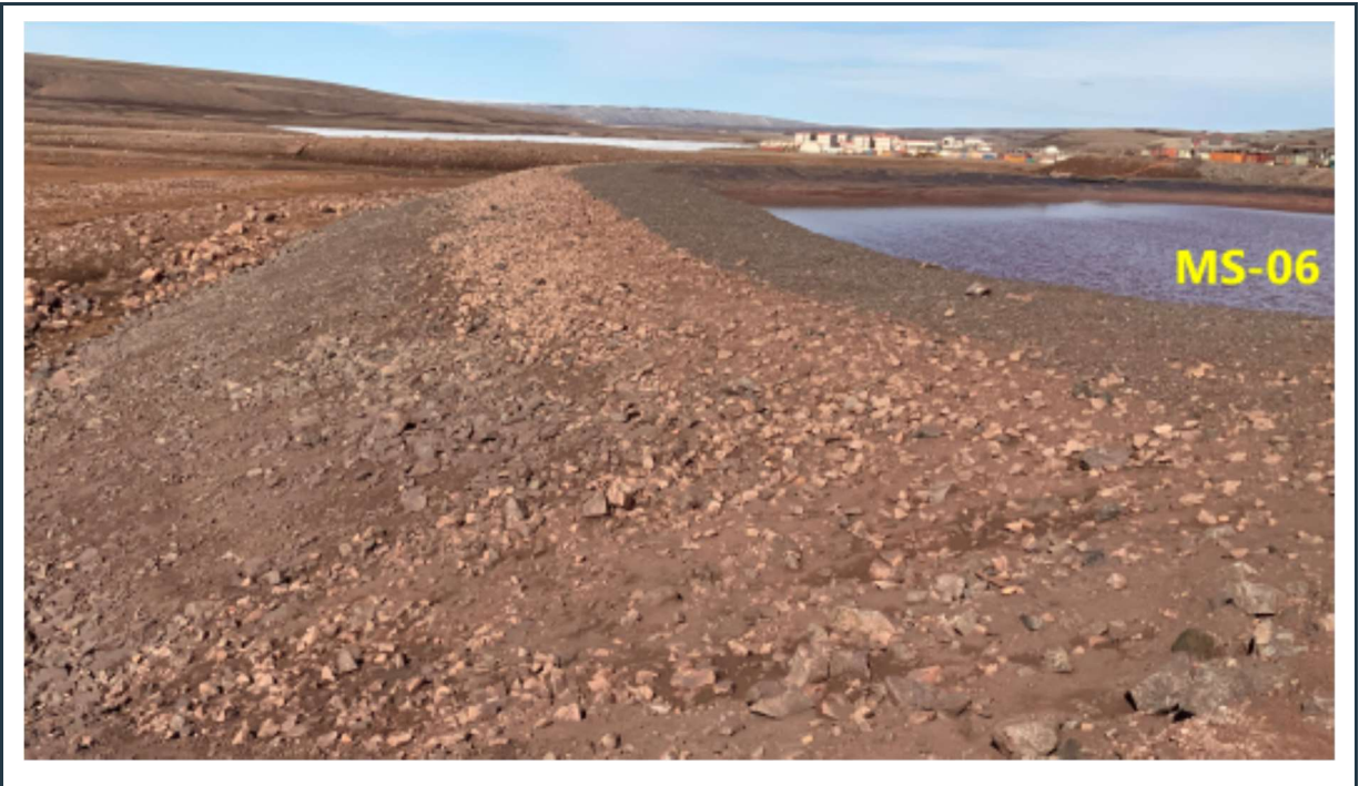
Figure 20: View of the MS-06 settling pond with robust, stable berms and intact liner.
