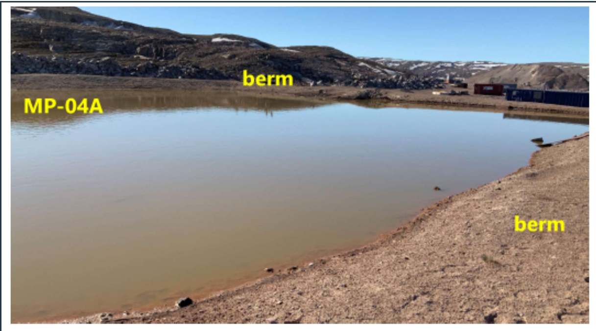
Figure 50: View of the MP-04A cell with stable berms and ponding melted snow.
