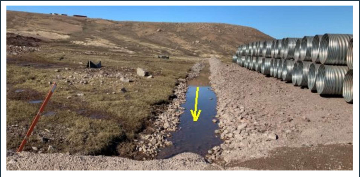
Figure 58: View of the "P-SWD-3 surface water collection ditch with ponding water and unstable slopes.
