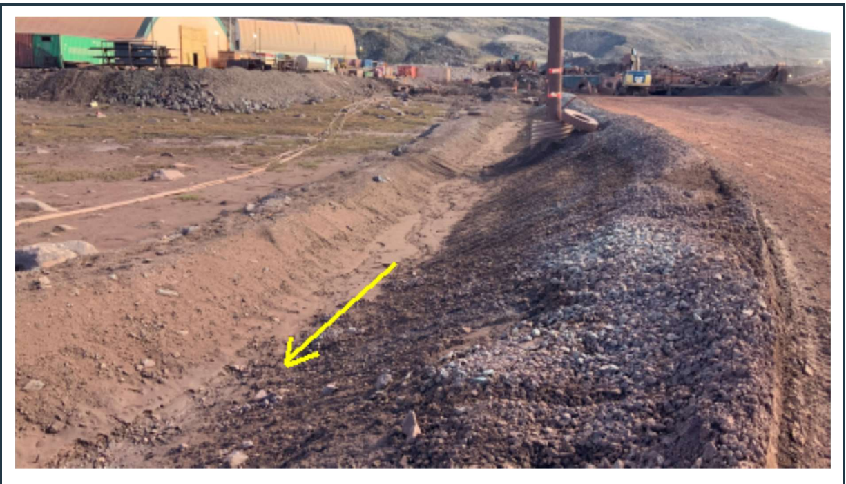
Figure 21: Well-maintained drainage ditch next to the crusher plant, leading to the MS-06 pond.
