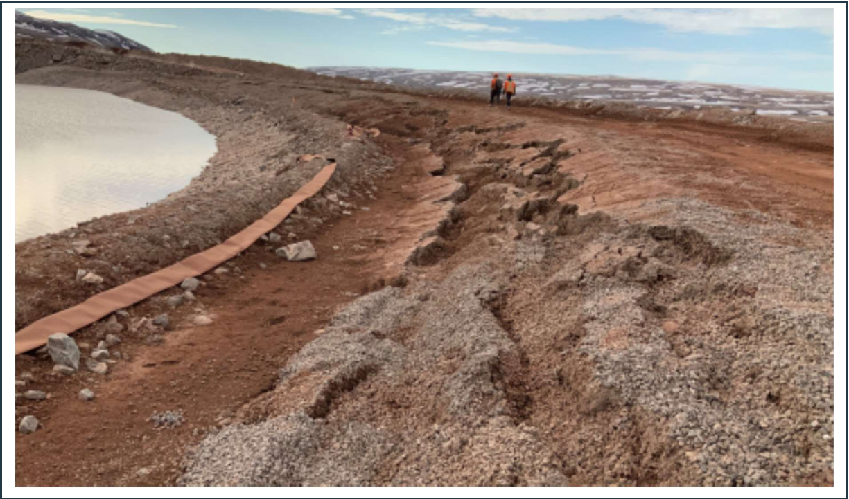
Figure 28: View of some frost related damages along the road next to the MS-11 pond (south pond) that must be repaired.
