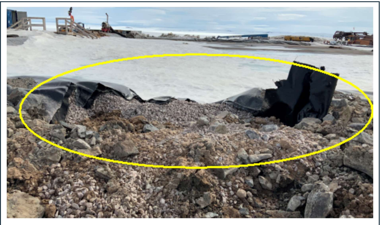
Figure 25: Damaged rock fill berm and liner at the south-west section of the berm at the water treatment pond, located adjacent to the waste rock disposal facility.
