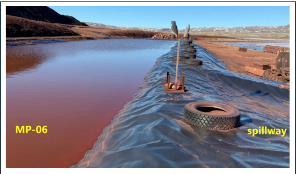
Figure 55: View of the lined MP-06 pond with robust, stable berms and spillway.
