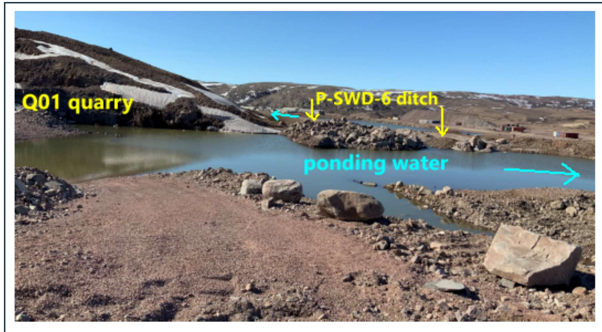
Figure 62: Ponding water next to the P-SWD-6 - "Q01 South" surface water collection ditch.
