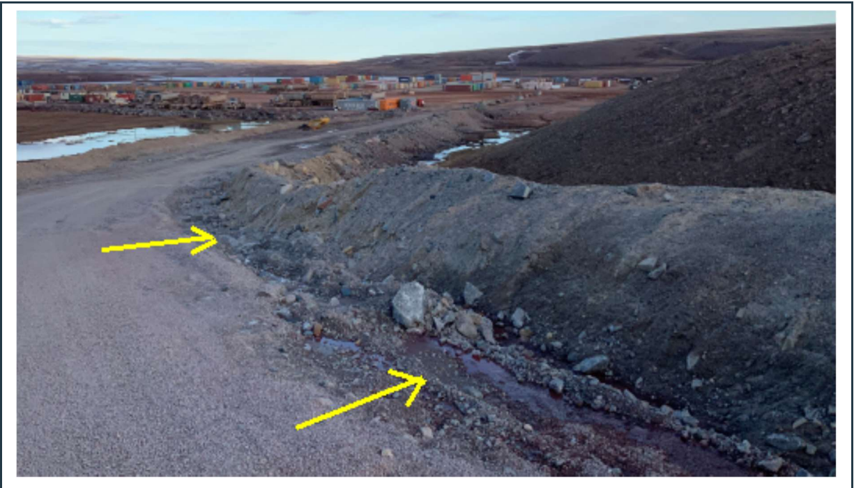
Figure 40: View of the access road to the quarry that requires additional maintenance work.
