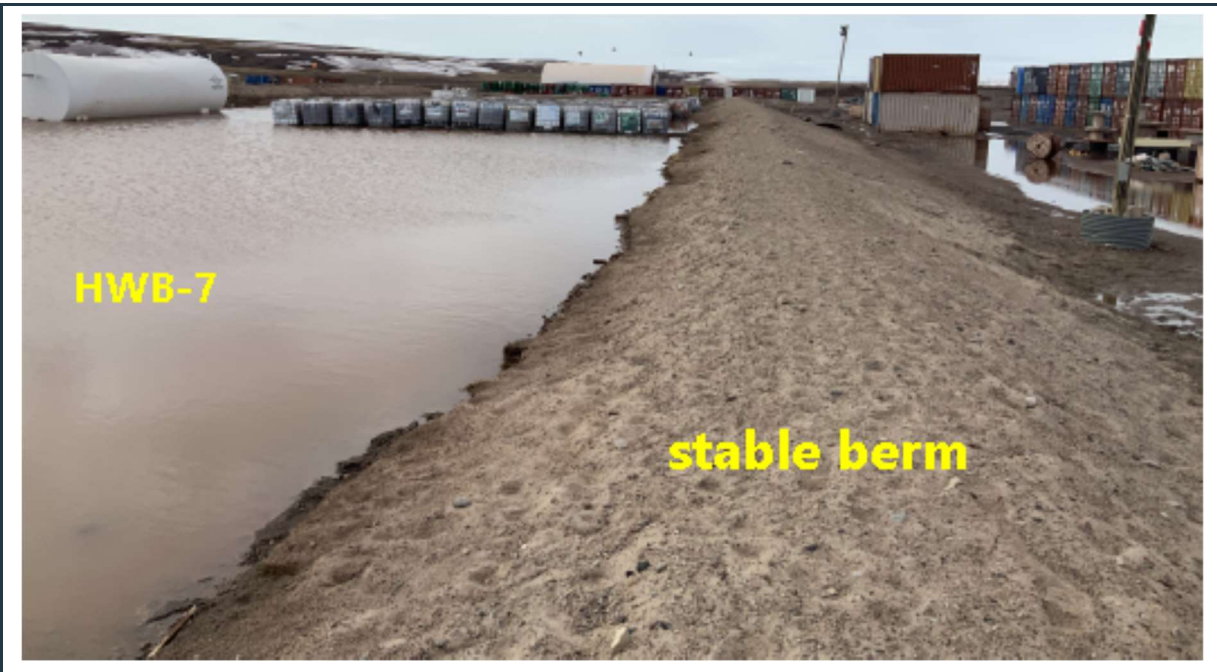
Figure 22: View of the stable berm around the HWB-7 cell, with an old fuel tank and oil filled plastic containers stored in the cell. The ponding water indicates good liner performance.
