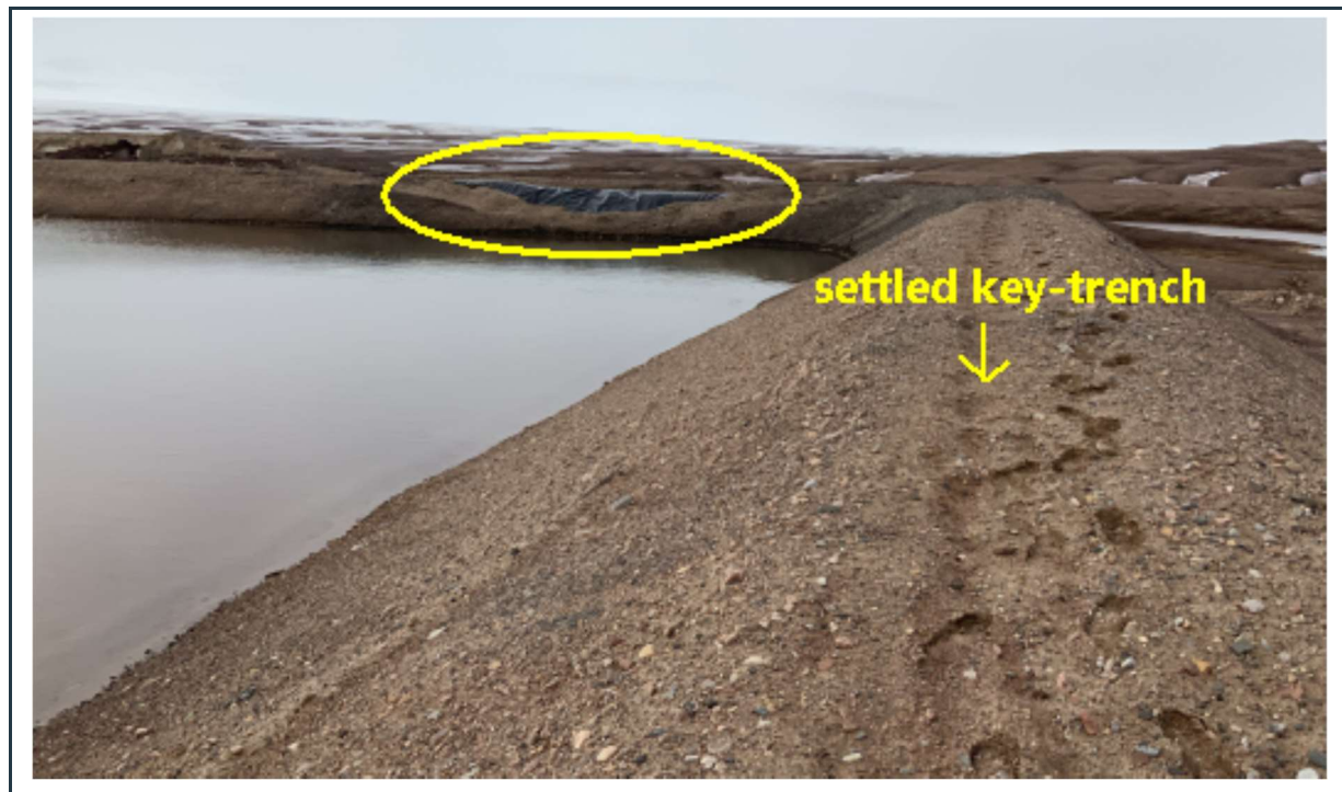
Figure 41: View of the currently empty Cell 2 at the landfarm. Note the exposed liner at one section of the berm, above the internal sump within the facility (see Figure 38).
