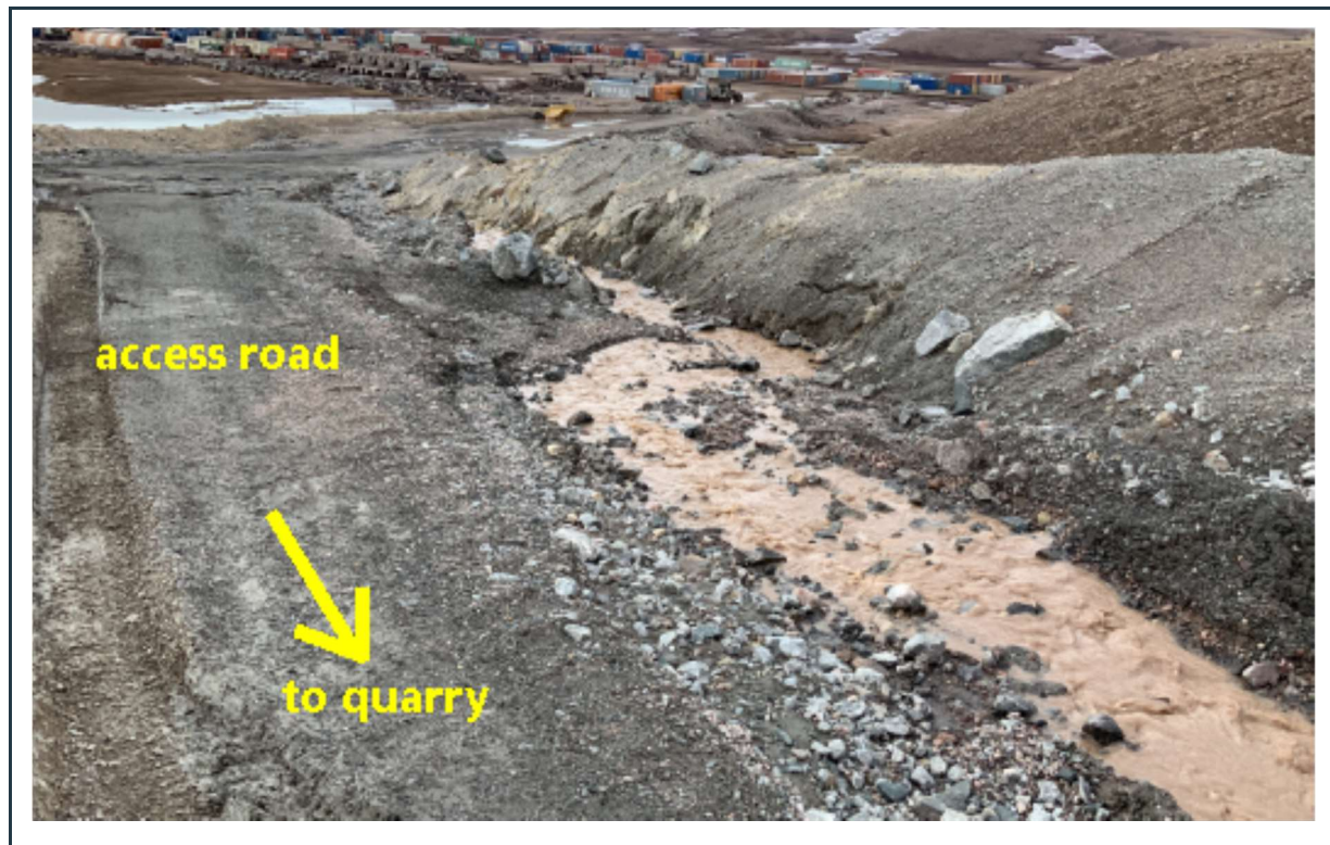
Figure 46: Erosion problem still exists along the edge of the access road to the quarry.
