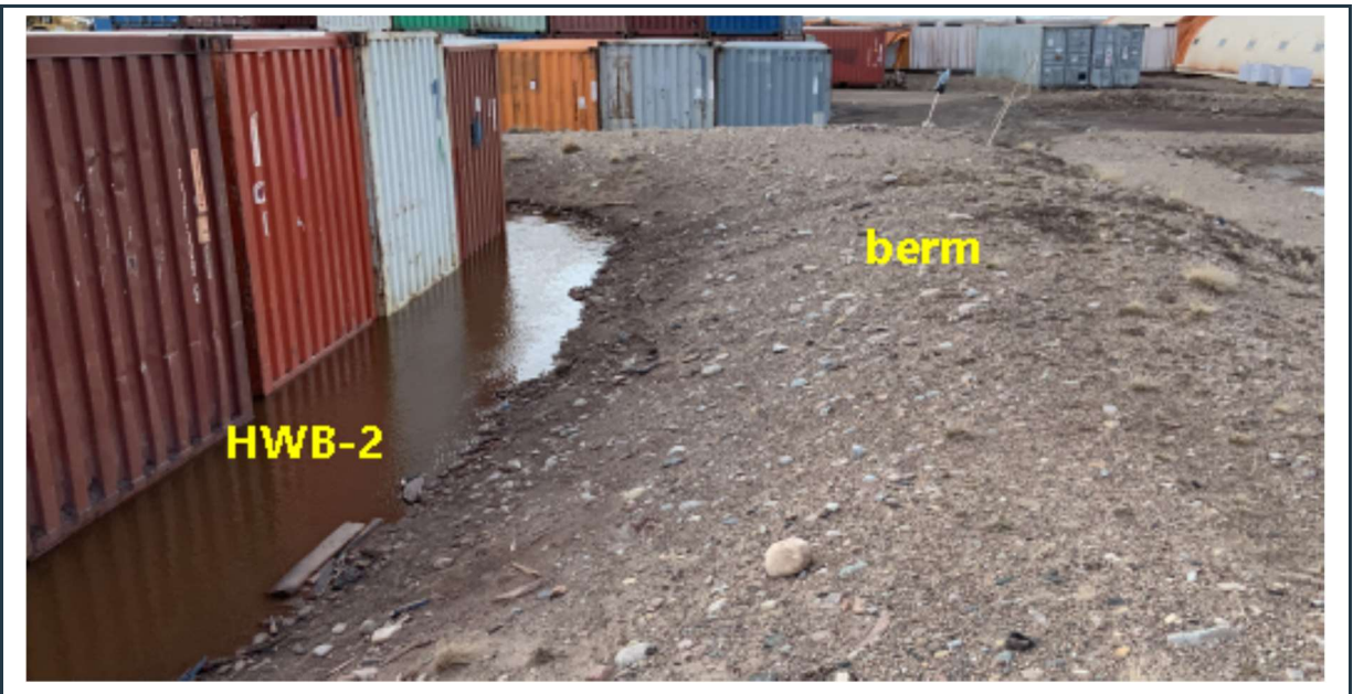
Figure 17: View of the robust, stable berms around HWB-2. The presence of water in the cell indicates good liner performance.
