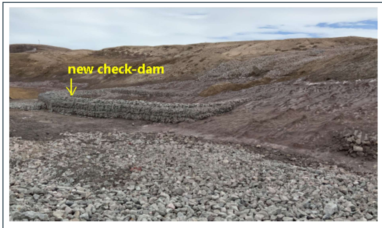
Figure 43: View of the new check-dam, adjacent to Camp Lake, to capture suspended solids potentially eroding from the airfield area and to prevent siltation in the lake.
