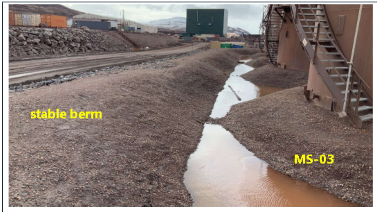
Figure 35: Well-maintained, stable berm around the MS-03 diesel fuel farm, with some ponding water.
