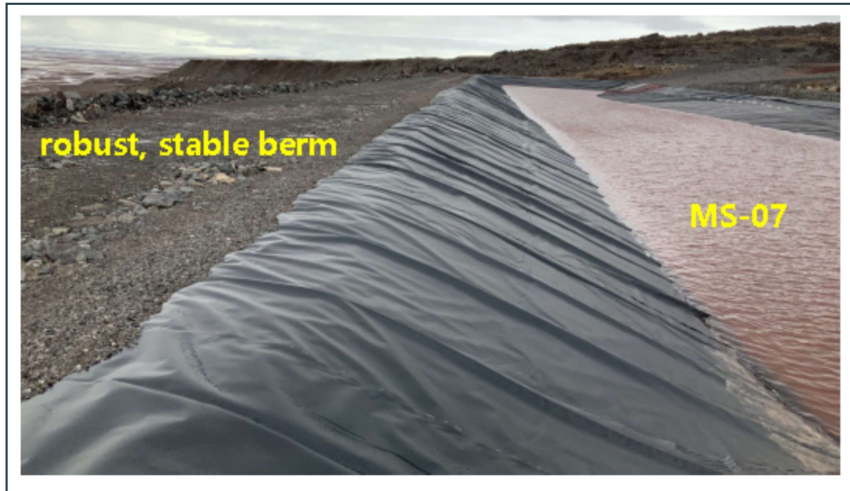
Figure 26: View of the robust, stable berms and intact liner at the MS-07 surface-water management pond.
