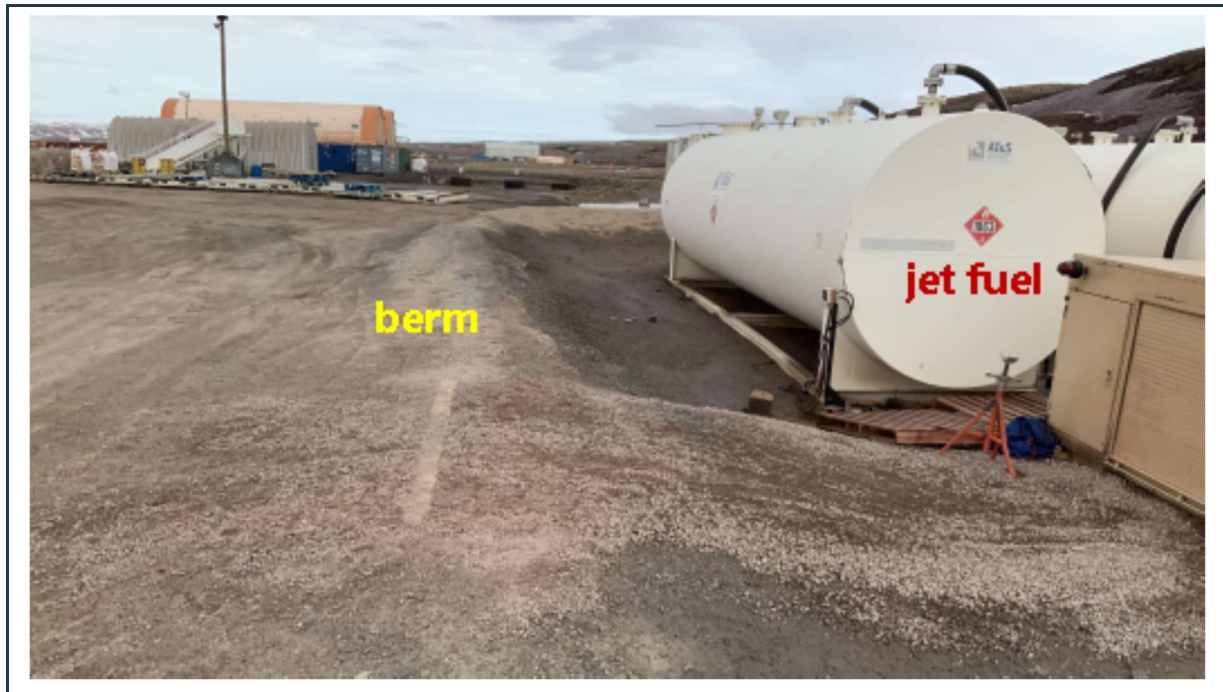
Figure 34: View of the well-maintained sand and gravel berm and access ramp at the lined jet-fuel storage facility.
