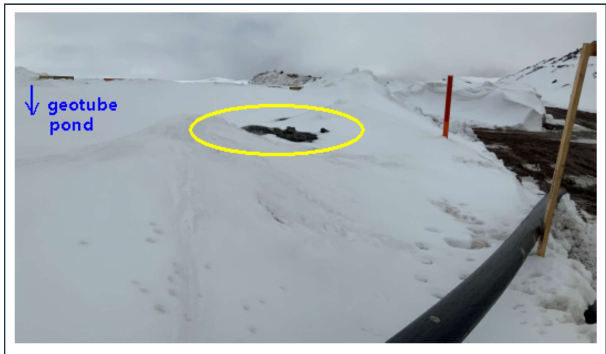
Figure 29: View of the snow- and ice-covered geotube pond. A small section of the liner at the south-west section of the berm (yellow circle) is still damaged and will require repair.
