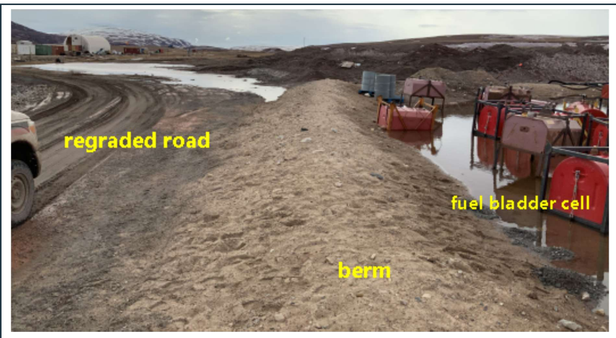
Figure 33: View of the stable berm around the "fuel bladder" cell. The adjacent road next to the east berm was recently regraded.
