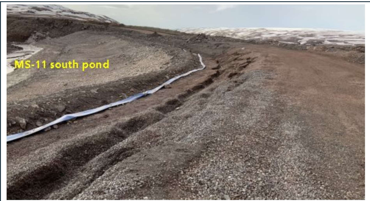
Figure 32: View of the loosely filled and cracked liner anchor trench along the road next to the south MS-11 pond's slope. The cracks should be backfilled with fine-grained soils, regraded, and compacted to minimize water infiltration into the ground next to the slope.
