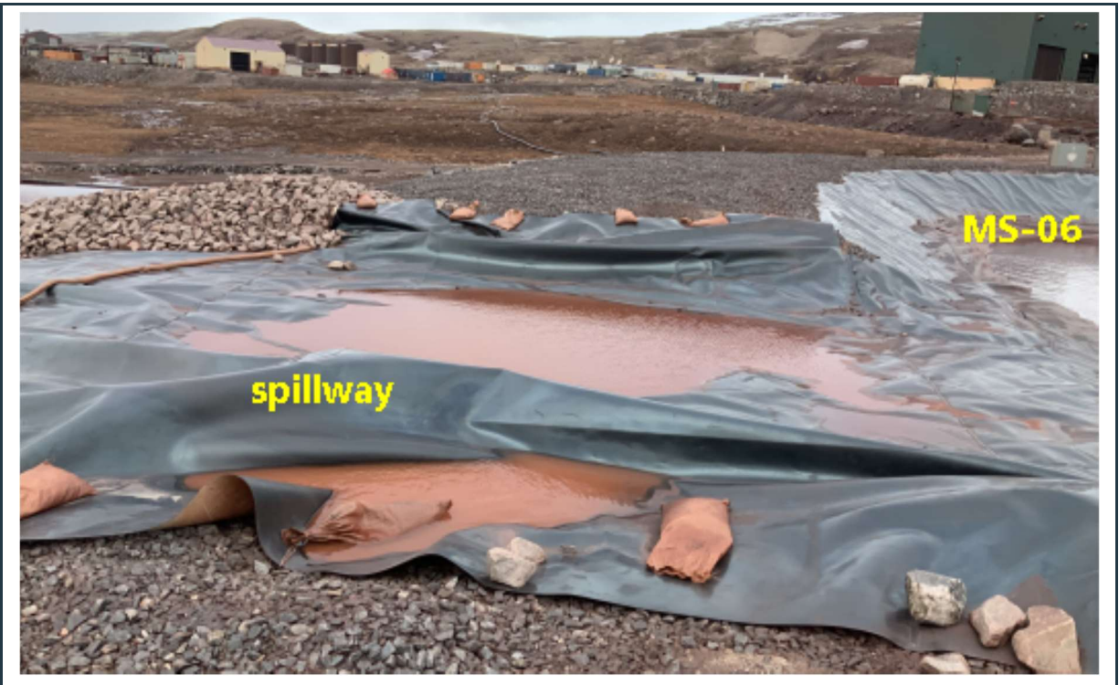
Figure 24: View of the robust, stable berm around the MS-06 pond, with temporary problem with the liner (lift-up by wind) at its spillway. Placement of more, heavier sandbags is recommended.
