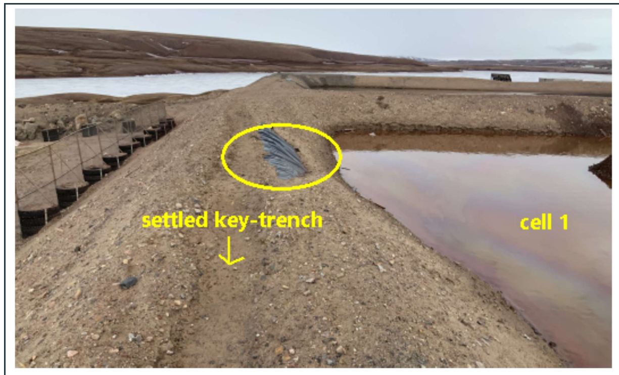
Figure 40: View of a section of the recently constructed berm at the landfarm's Cell 1. Note the exposed liner in one area of the berm and the settled anchor trench along the crest of the berm.
