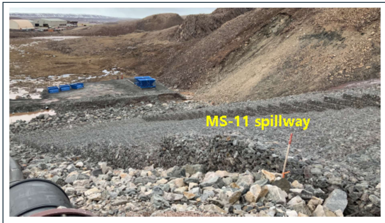
Figure 31: View of the robust and stable emergency spillway (gabion baskets and blankets filled with crushed rock) at KM105. Note the water seepage at the toe of the spillway.
