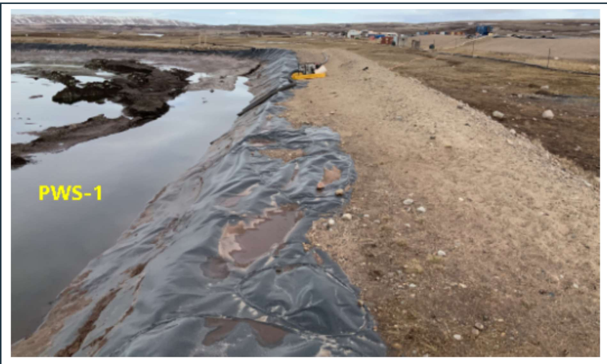
Figure 13: PWS pond #1. Well-maintained, stable perimeter berm and intact liner at the pond. Note the ice in the pond on June 22, 2023.
