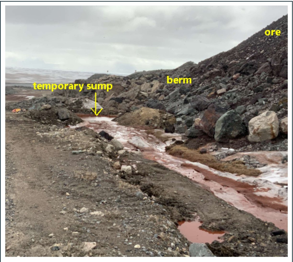
Figure 48: View of the edge of the stockpiled ore, and rockfill berm at the new KM-106 ore stockpile area and a temporary sump, downstream from the berm. The drainage ditch to the sump should be cleaned/graded and the water from the sump should be pumped into the nearby MS-07 pond (see Figure 26).
