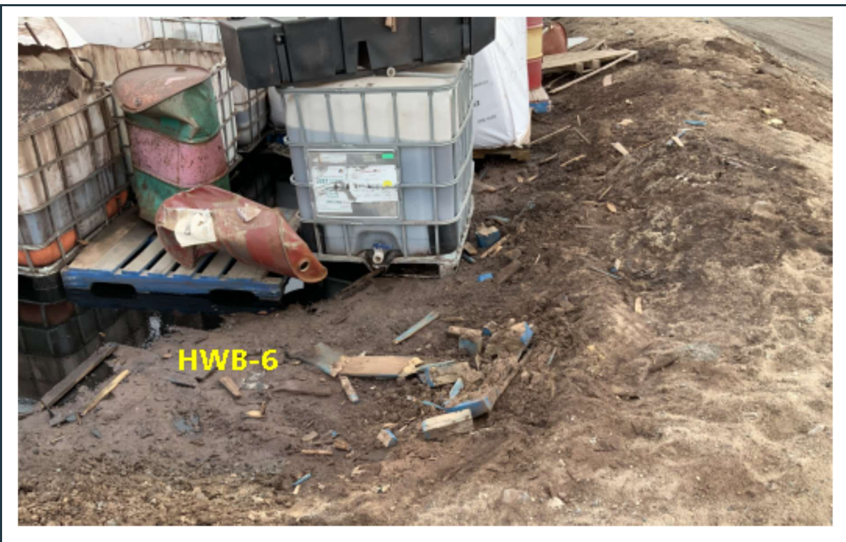
Figure 21: View of the completely full HWB-6 cell. The berm around the cell requires maintenance.
