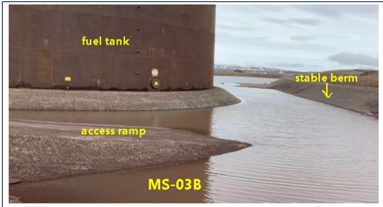
Figure 36: View of the well-maintained stable berm and access ramp to the interior of the new fuel tank farm. Note the ponding water, indicating good liner performance.
