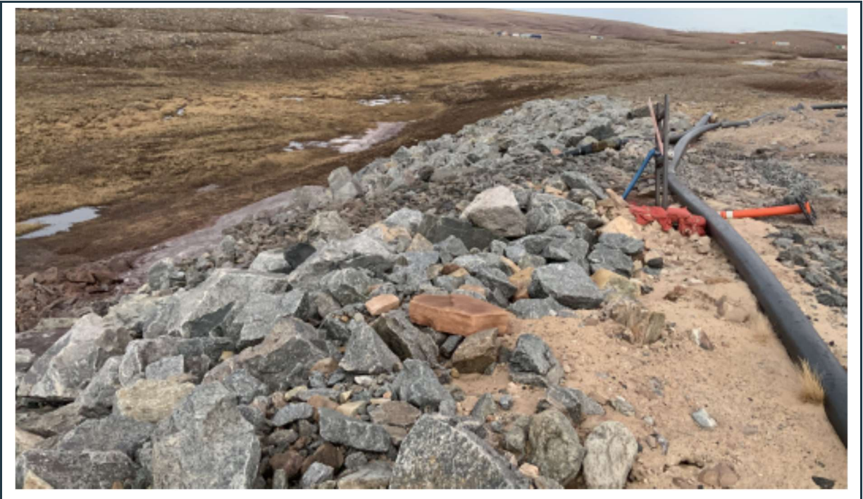
Figure 44: View of the stable rockfill riprap slope at the water discharge area.
