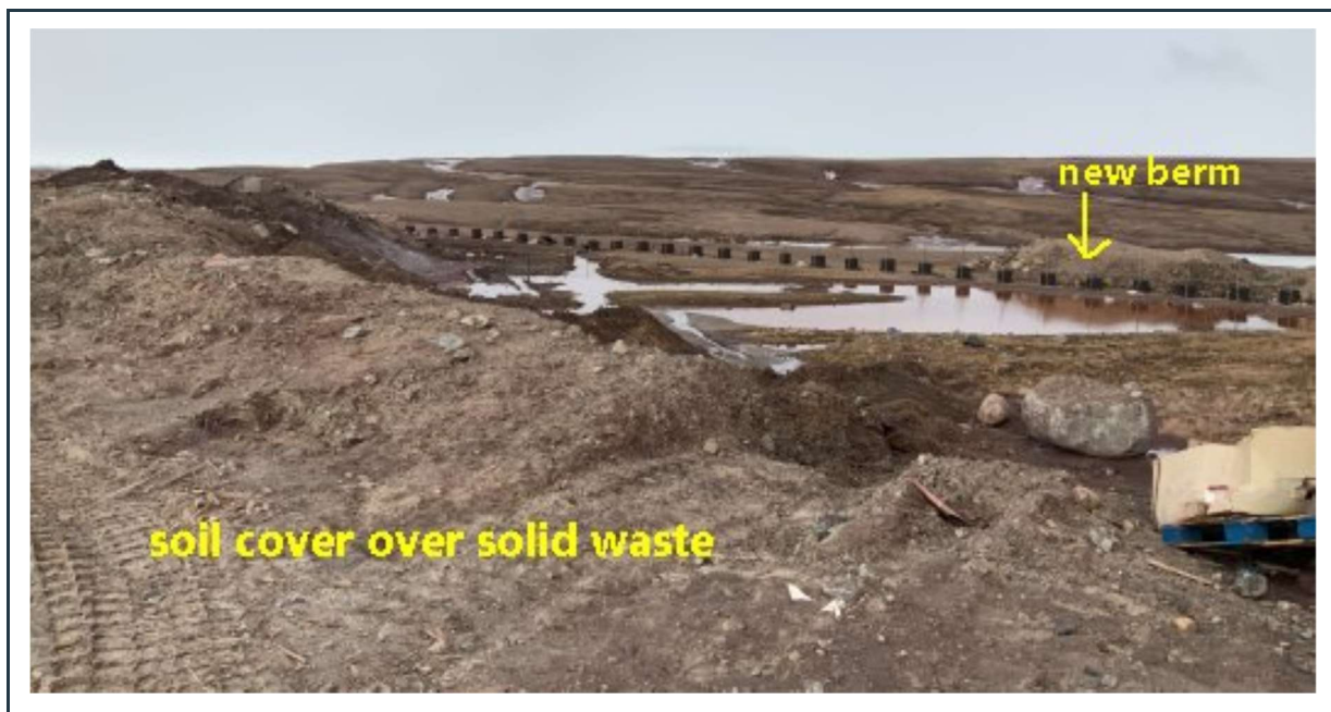
Figure 39: View of soil cover over non-hazardous solid waste in the landfill facility. Note the new berm under construction outside of the fence to prevent surface water leaving the landfill site.
