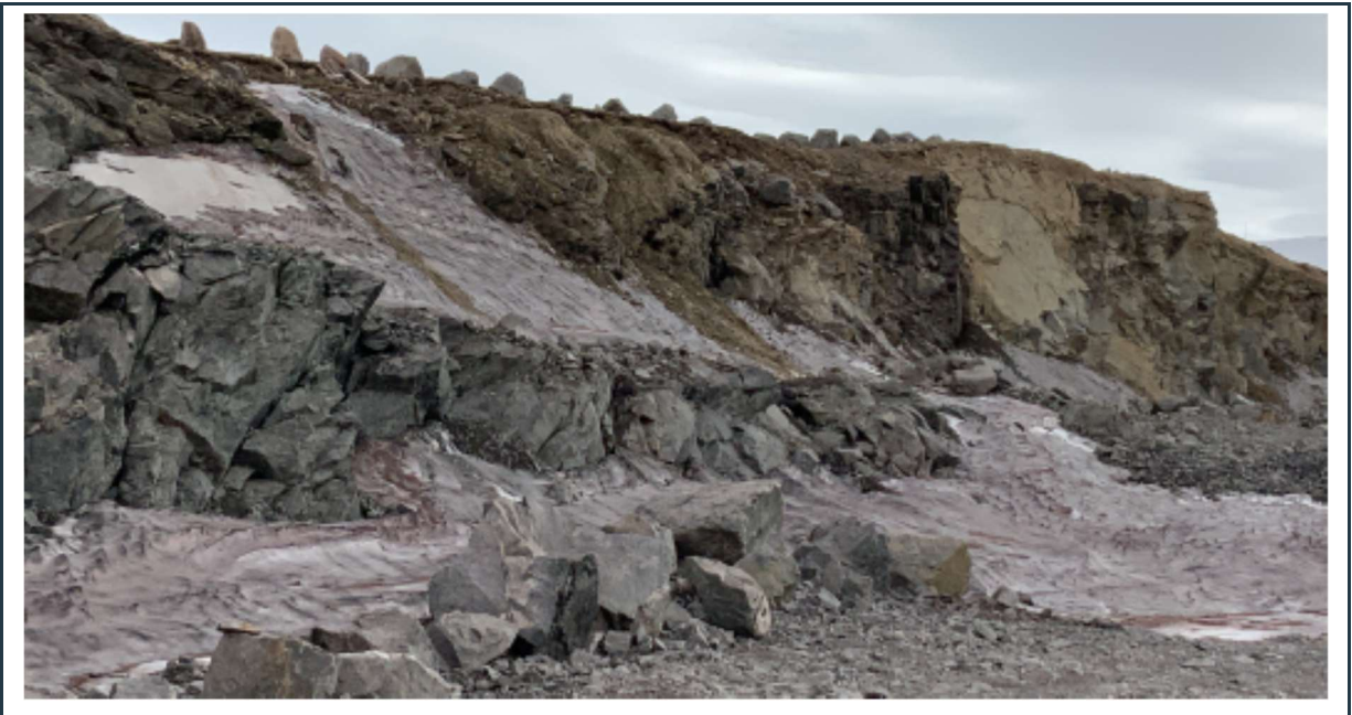
Figure 45: View of the snow-covered rock face at the upper quarry level with minor potential erosion and rolling rock hazard. No activity is currently carried out in this quarry.
