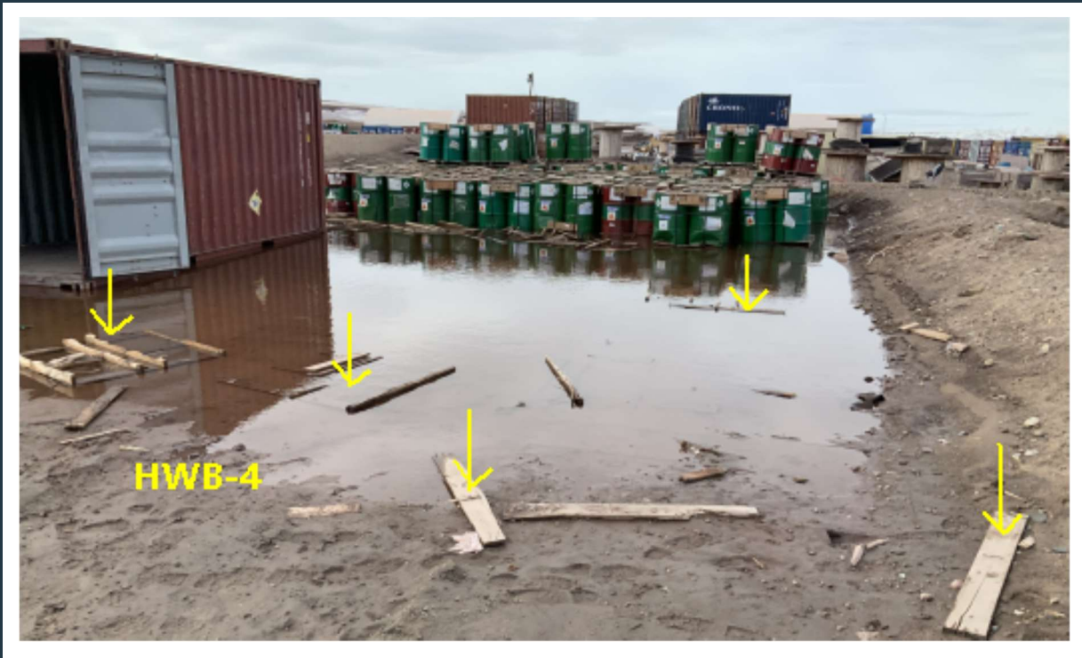
Figure 19: View of stable berms around the HWB-4 cell, with a shipping container and fuel barrels on wooden pallets stored in the cell. The broken pallets (yellow arrow) should be removed.
