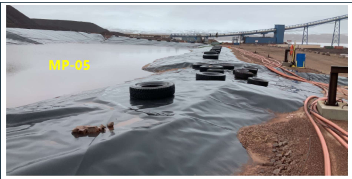
Figure 60: View of the robust, stable berms and intact liner at the MP-05 pond.
