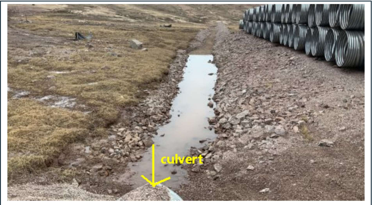
Figure 67: View of the southern part of the P-SWD-3 surface water collection ditch with failed slope sections, and ponding water due to inadequate longitudinal channel slope.
