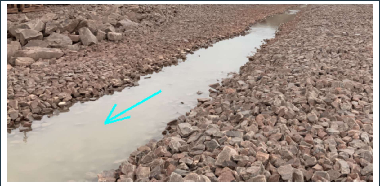
Figure 75: View of the recently completed W3/W14 surface water collection ditch with crushed rock riprap slope protection.
