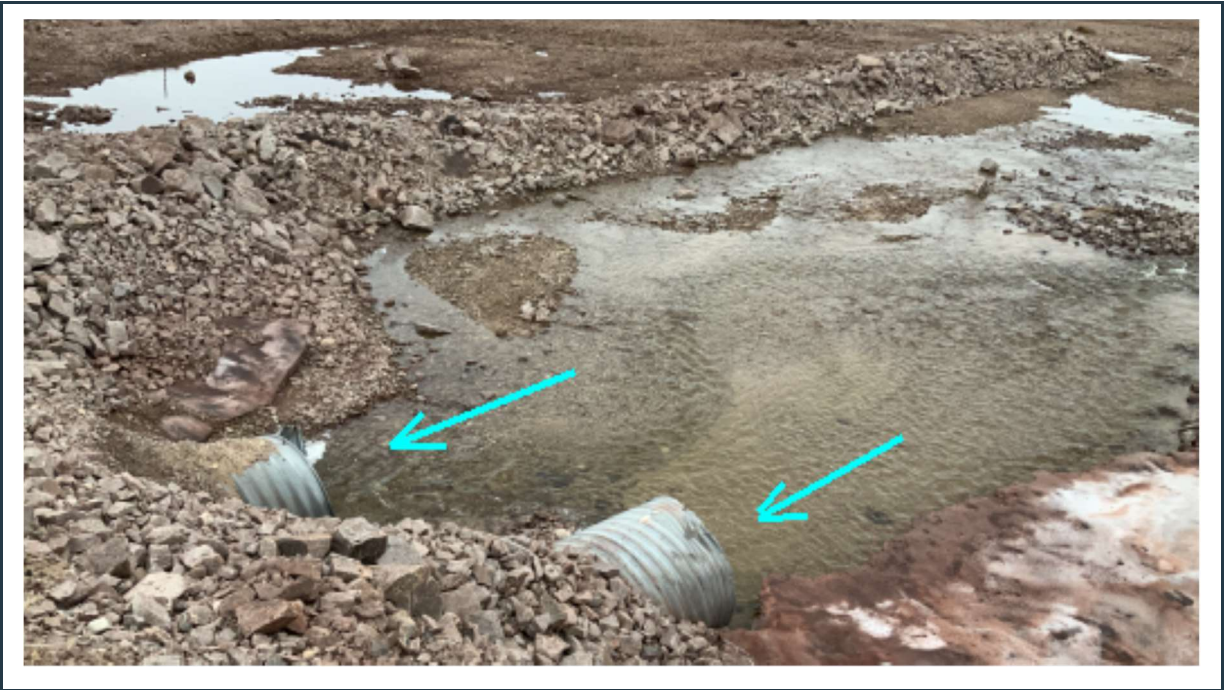
Figure 73: View of the P-SWD-7 surface water collection ditch and culverts (inlet).
