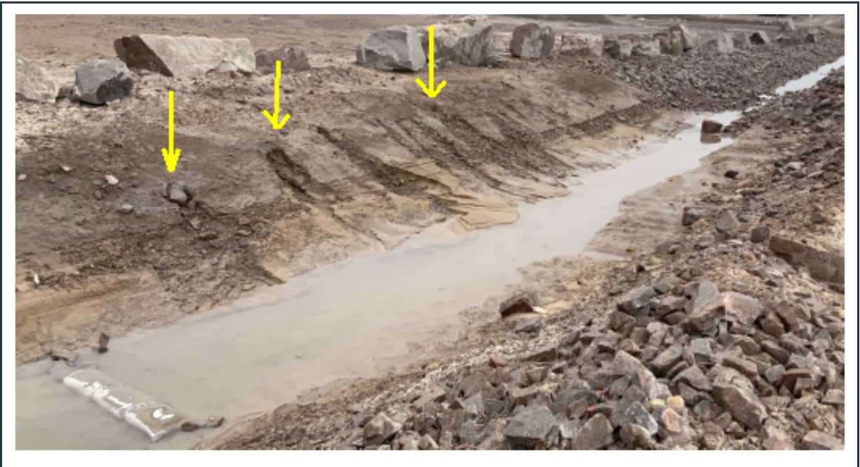
Figure 69: P-SWD-5 – “Q01-North” surface water collection ditch with missing riprap at one section of the ditch, where continuous seepage is noted from the side-slope.
