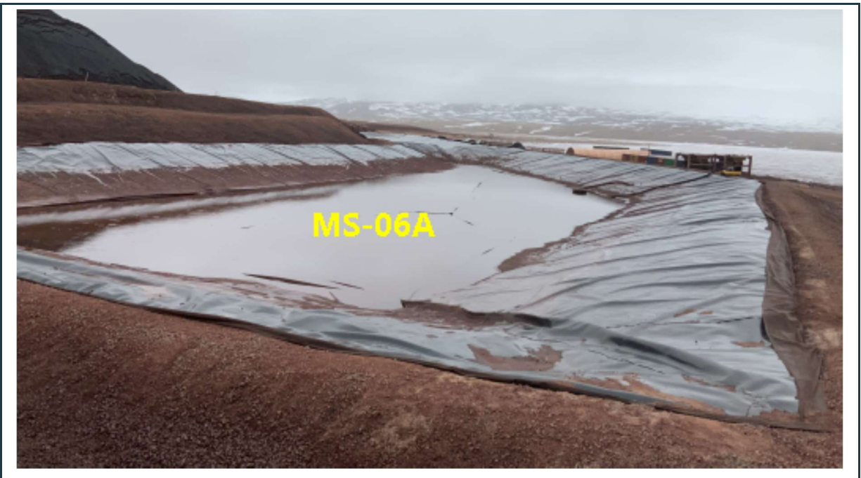
Figure 65: View of the lined MP-06A overflow pond with robust stable berms.
