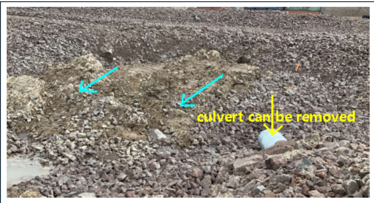
Figure 78: View of the "west end" of the PSC surface water collection ditch (red circle in Figure 7). Note the localized slope degradation due to frequent water seepage from the granular fill of the LP-2 laydown pad (blue arrows). The culvert in the area can be removed.
