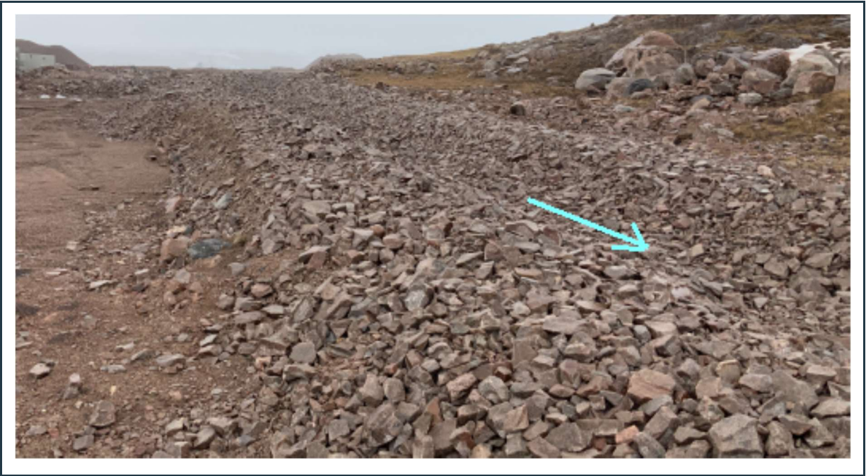
Figure 71: View of the now inefficient P-SWD-6 surface water collection ditch, due to over-blasting in the rock quarry.
