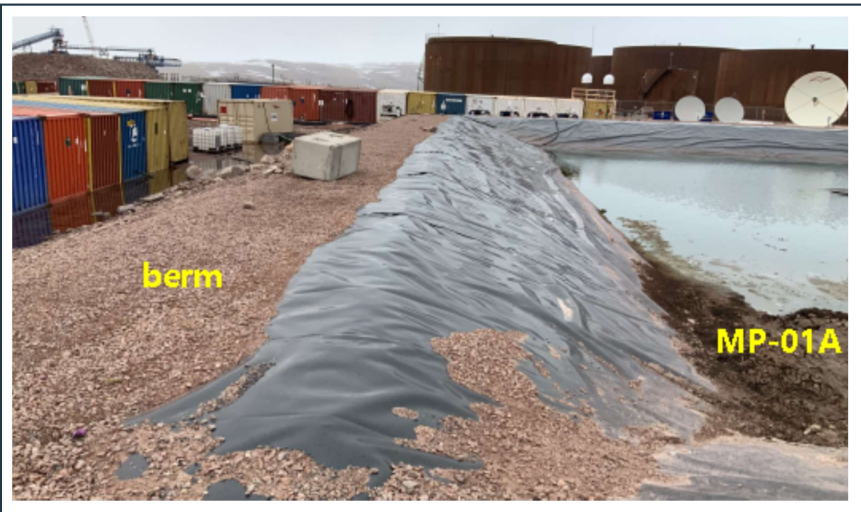
Figure 54: View of the robust, stable berms and intact liner in the MP-01A pond.
