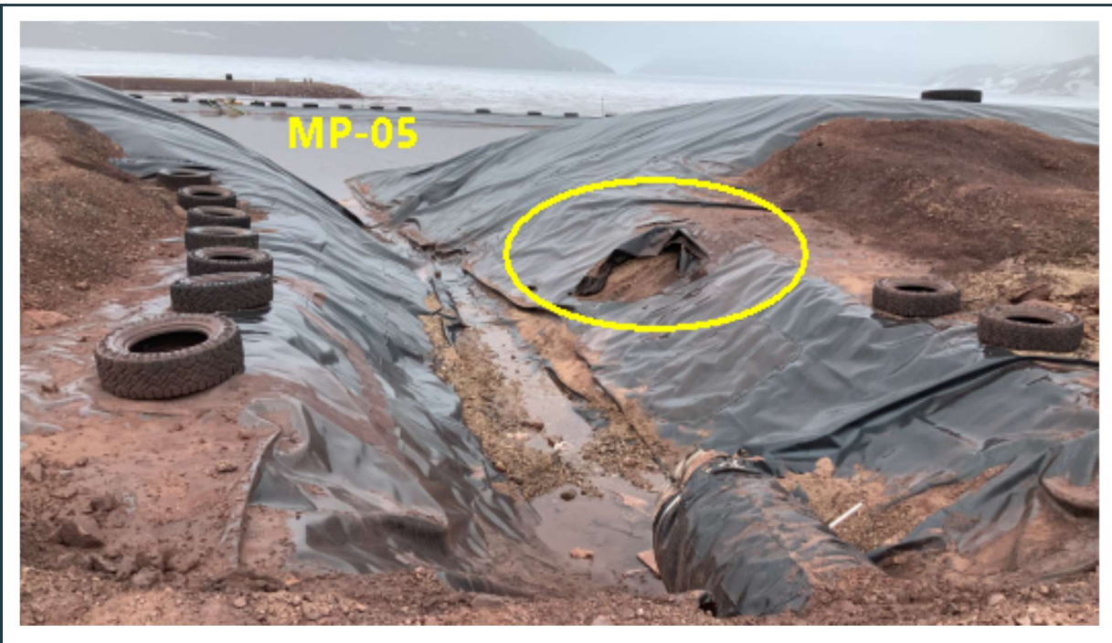
Figure 61: View of the inlet channel to the MP-05 pond, with the liner damaged at one location (yellow circle). The liner should be repaired as soon as practically possible.
