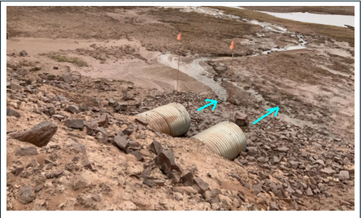
Figure 81: View of twin culverts, draining surface water from the quarry area (outlet).
