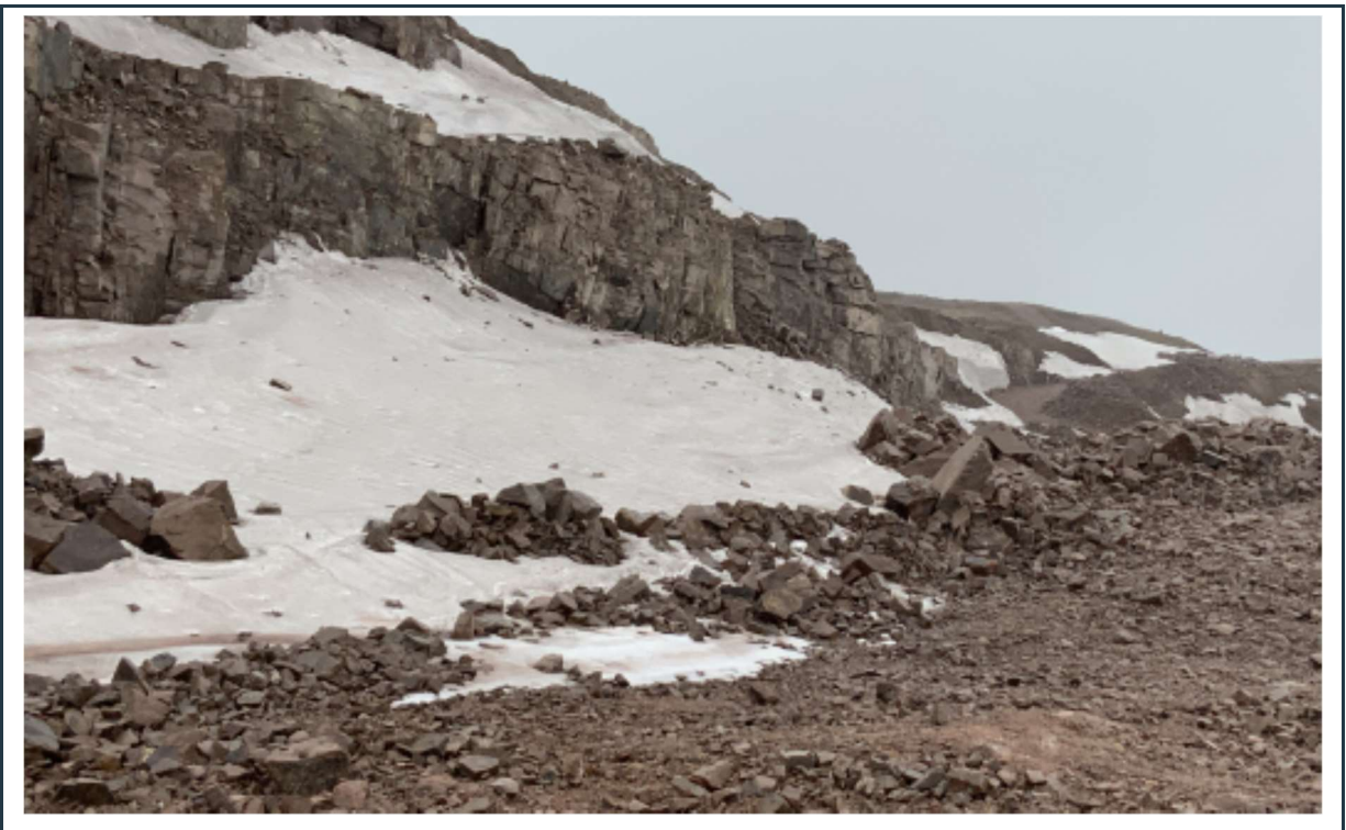
Figure 66: View of the snow-covered stable rock face with some weathering and bench erosion in the Q01 rock quarry. Currently there is no activity in this quarry.
