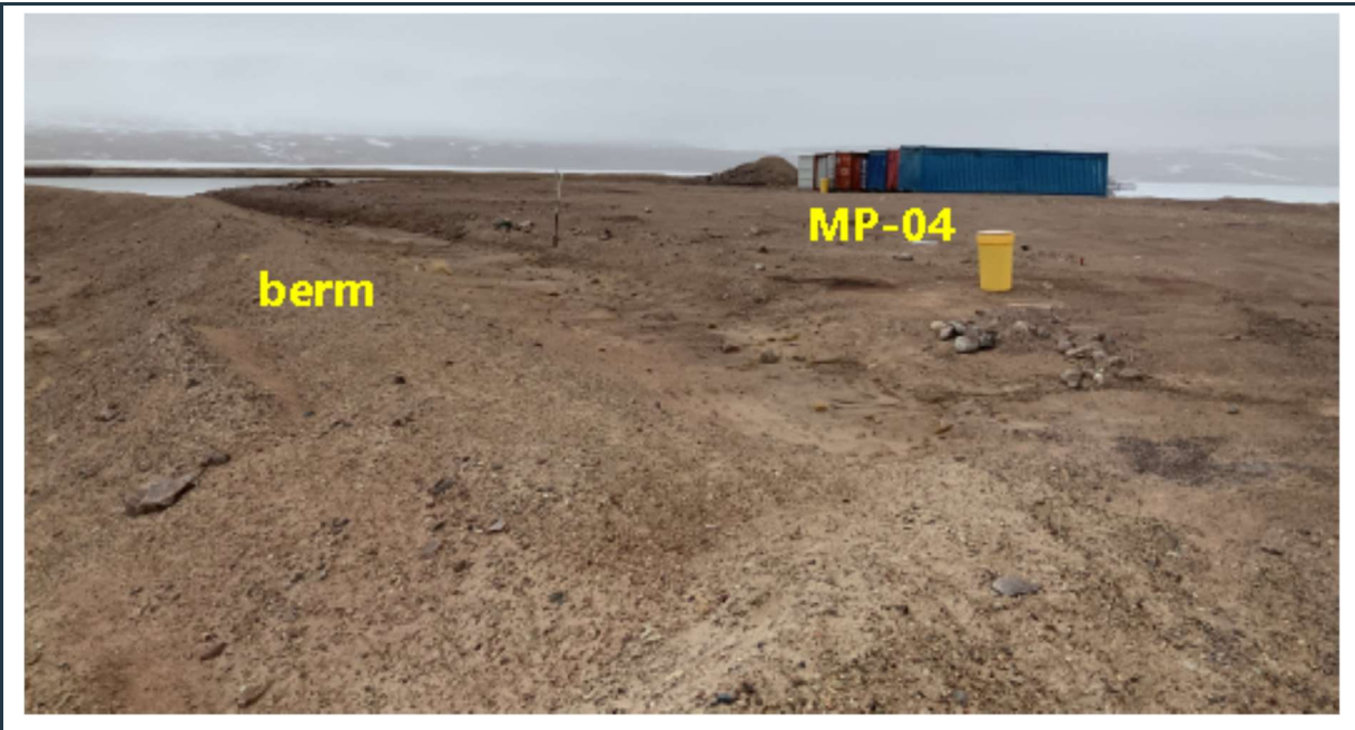
Figure 57: View of stable berm around the MP-04 land-farm, with ponding water in one corner of the cell.
