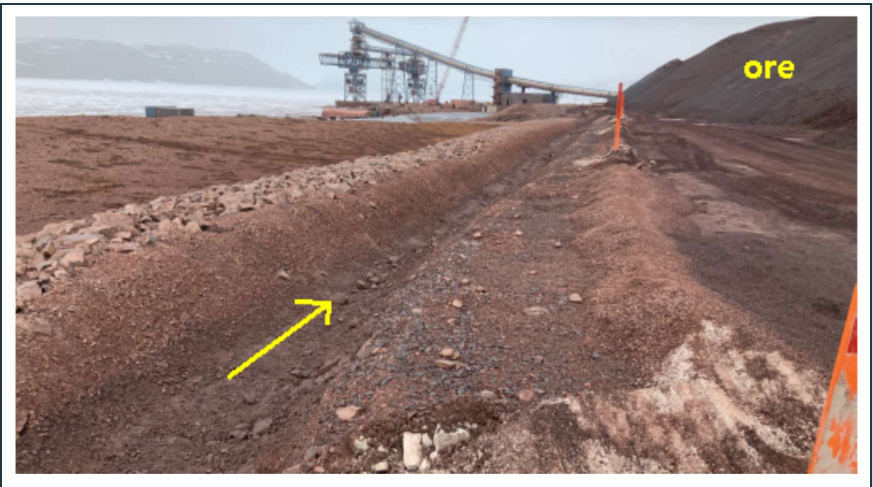
Figure 63: View of the well-maintained "west" surface water collection ditch adjacent to the ore storage, draining to the MP-06 pond.
