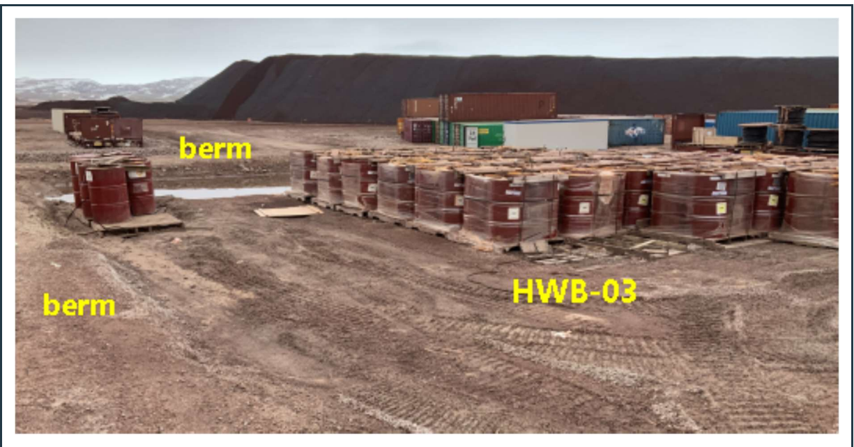
Figure 52: View of the HWB-03 cell with stable berms, containing fuel barrels. The interior subgrade has been regraded/lowered using clean sand and gravel fill, as specified in previous inspection report.
