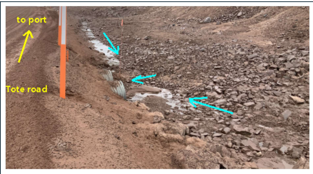
Figure 80: View of twin culverts, draining surface water from the quarry area under the tote road (inlet).
