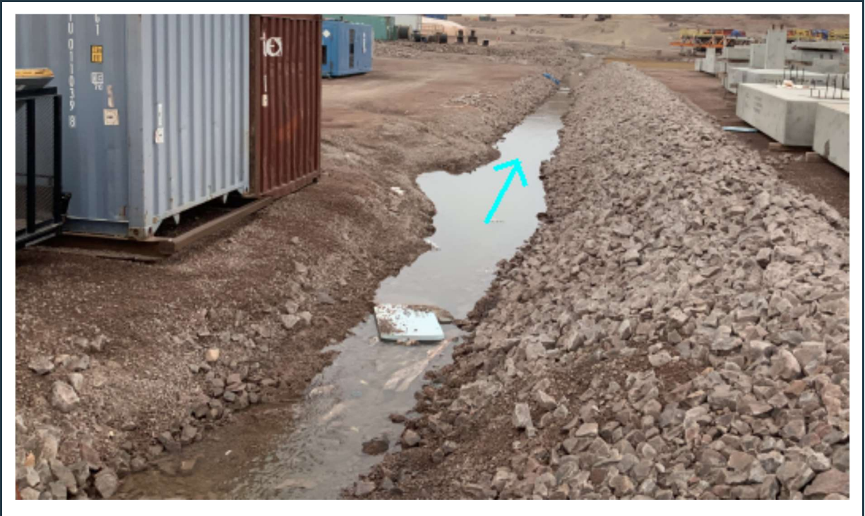
Figure 76: View of the south section of the 380-Person Camp surface water collection ditch. All debris (Styrofoam etc.) should be removed from the ditch.
