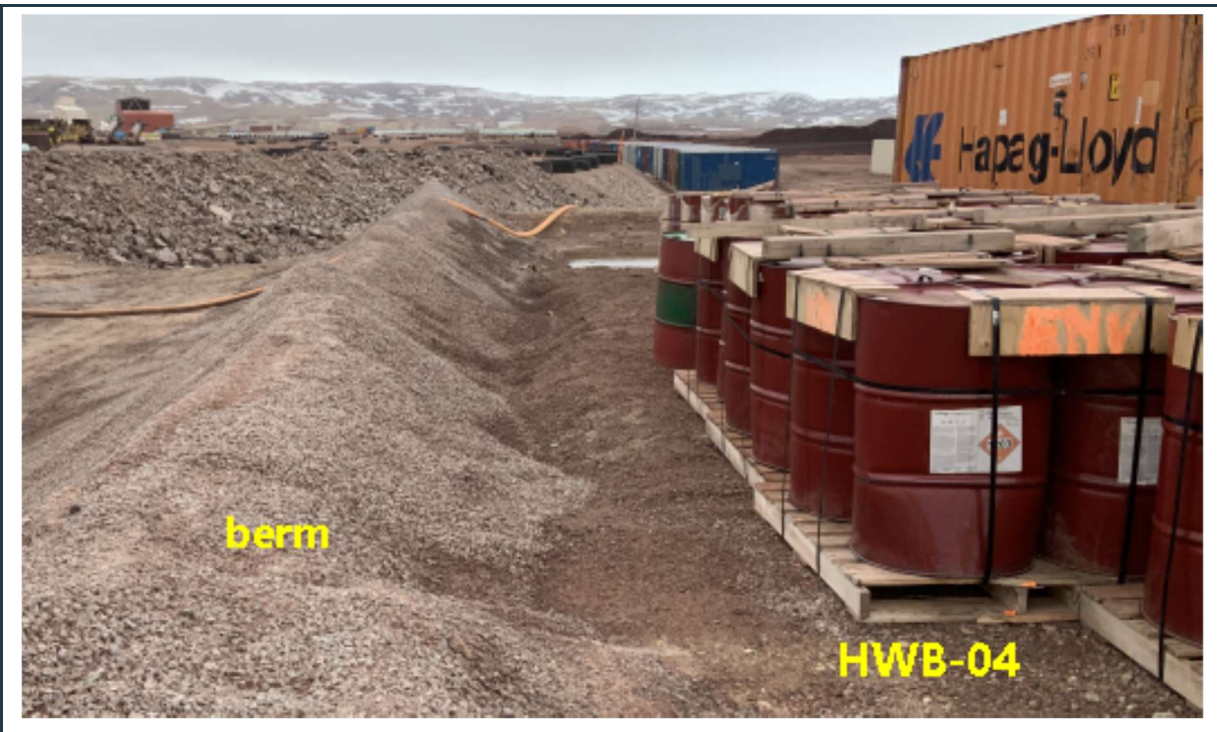
Figure 53: Recently improved (raised) berm at the HWB-04 cell, storing jet fuel and shipping containers.
