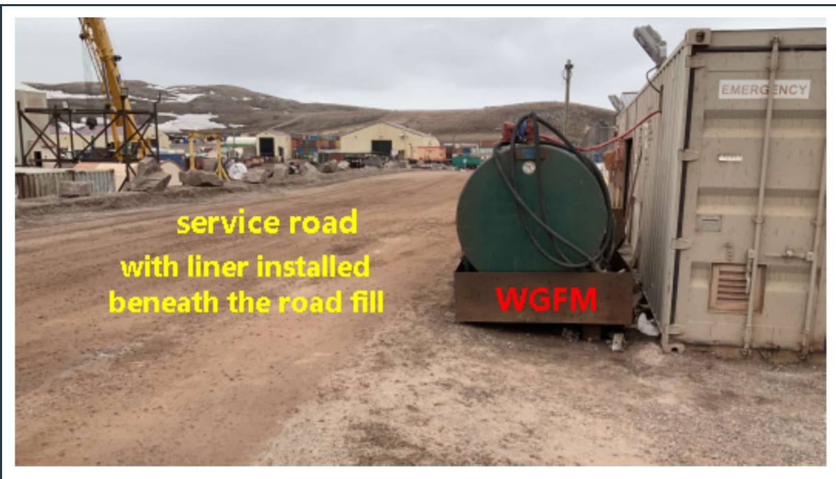
Figure 56: View of the Western Globe Fuel Module (WGFM) adjacent to MP-03 fuel tank farm. Based on site information, liner is present beneath the road fill and beneath the WGFM.
