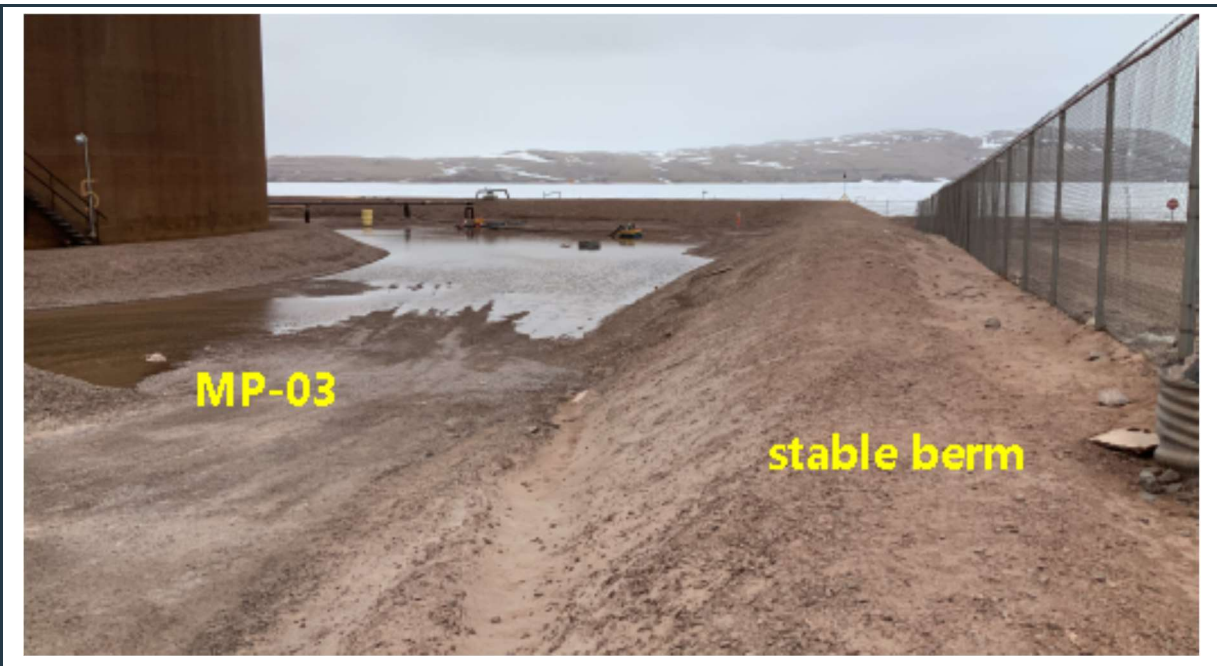
Figure 55: View of the well-maintained stable berms around the MP-03 fuel tank farm. The ponding water indicates good liner performance.
