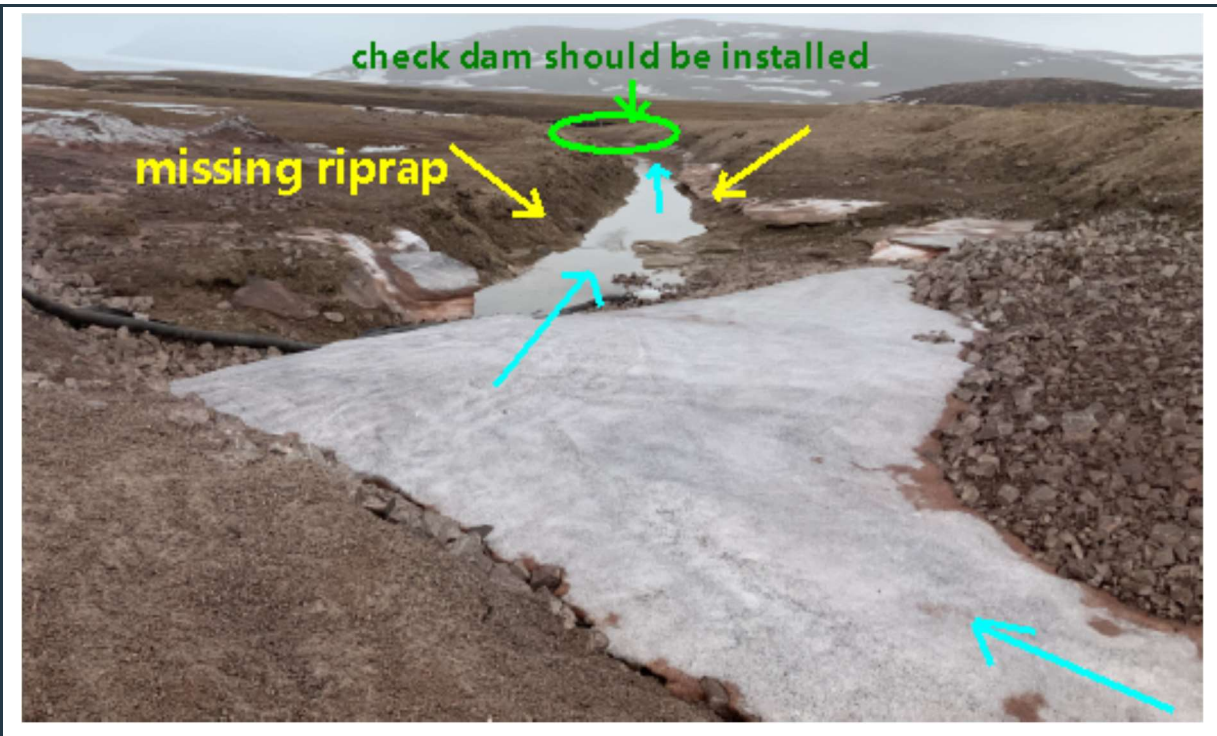
Figure 79: View of the unfinished “east end” of the PSC surface water collection ditch (green circle in Figure 7). Riprap and a check dam should be installed at this section if the ditch.
