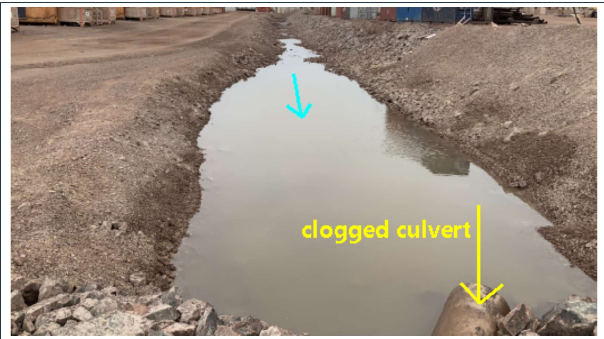
Figure 77: View of the east section of the 380-Person Camp surface water collection ditch with ponding water, due to the completely clogged culvert, which should be cleaned.
