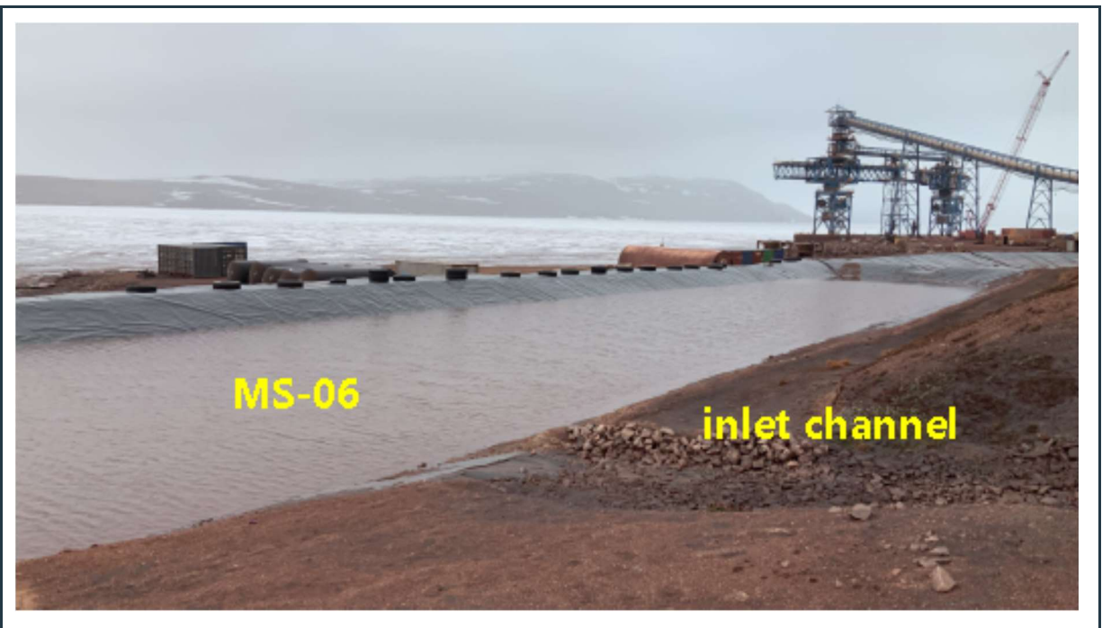
Figure 64: View of the lined MP-06 pond with robust, stable berms.
