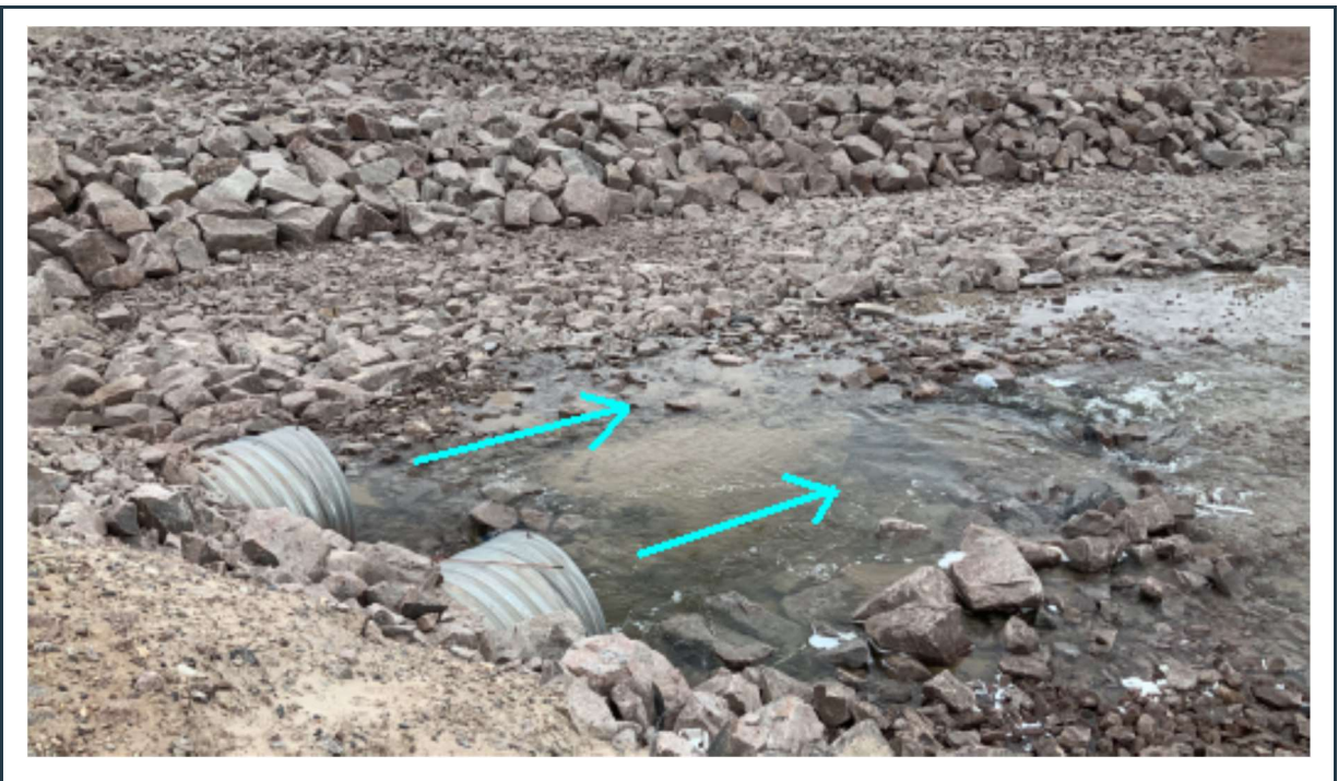
Figure 74: View of the well-maintained P-SWD-7 surface water collection ditch and culverts (outlet).
