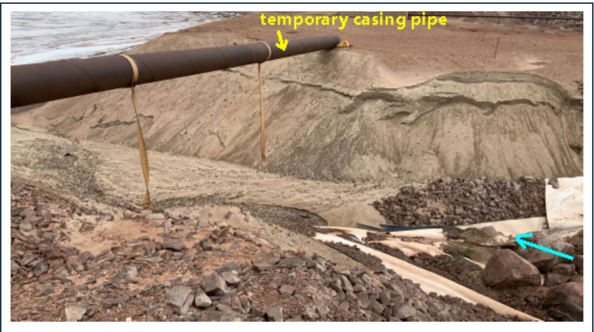
Figure 82: View of the end of the water discharge pipe (blue arrow) and deteriorating (eroding) slopes. This section of the valley should be filled with rock fill, placed over geotextile.
