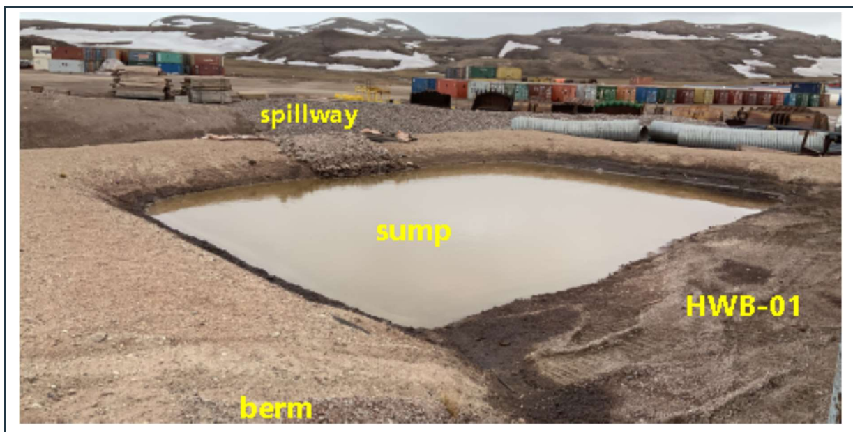
Figure 50: View of the sump and spillway at the back of the HWB-01 cell with stable berms.
