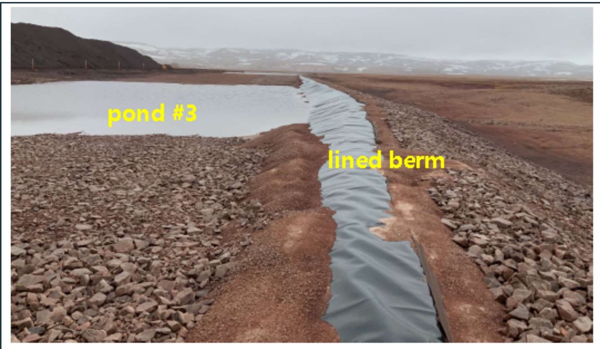
Figure 59: View of surface water management pond #3, with lined, stable berms.
