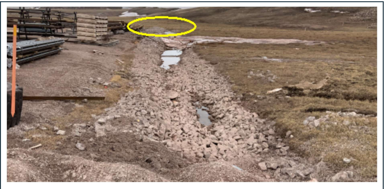
Figure 68: View of the northern part of the P-SWD-3 surface water collection ditch with failed slopes and some debris left in the channel, which should be removed. The ditch should be reconstructed.
