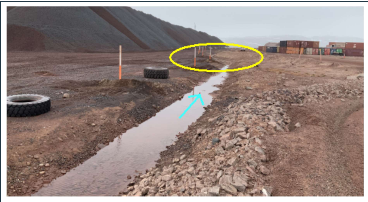
Figure 62: View of the "east" surface water collection ditch adjacent to the ore storage, draining to the MP-05 pond. Note the ponding water at the south end of the ditch. The ditch should be deepened/excavated in the area of the yellow circle to facilitate water flow to the MP-05 pond.
